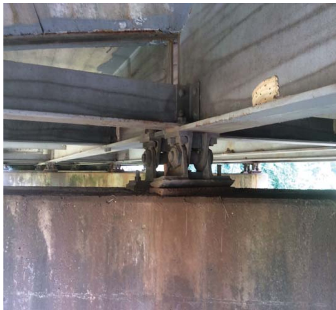
PHOTO 1 Description Span 1 beam 2 bearing shows some vertical movement 1/8" under heavy truck traffic. Sole plate are showing signs of wearing on rocker bearings typical all.. some bearing have heavy pack rust and anchor bolt are rusted into.....
