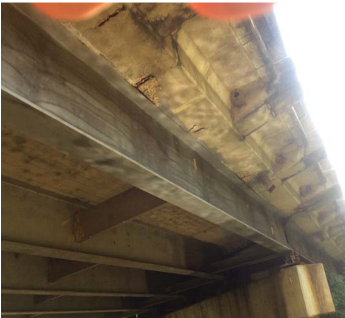
PHOTO 1 Description Bottom of deck span 3 right side spall with rebar exposed.
