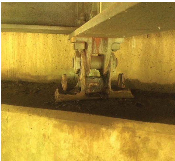
PHOTO 4 Description Abutment 2 beam 3 pack rust on bearings.
