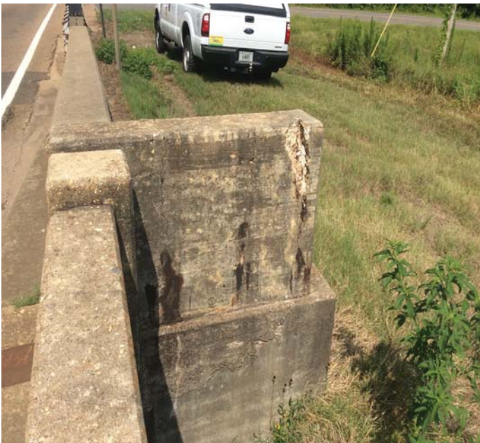
PHOTO 1 Description Left side top wing wall cracked and spalled beginning bridge.....
