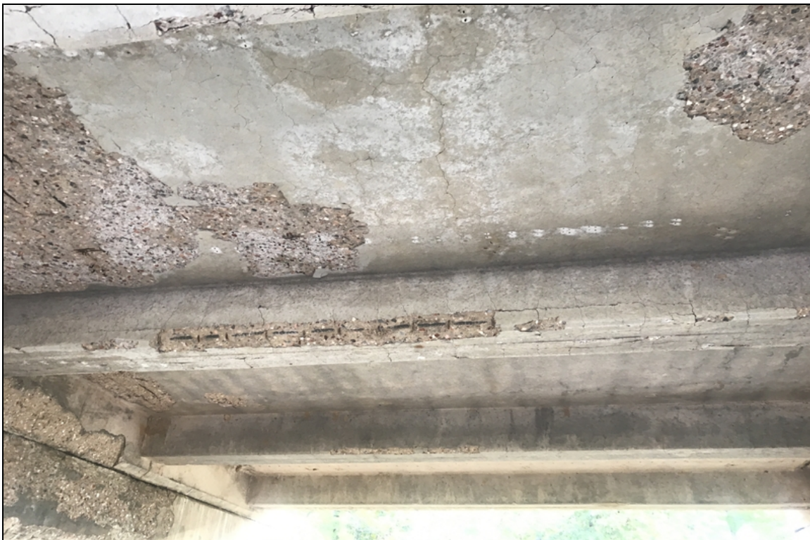
Under photo Span #13
