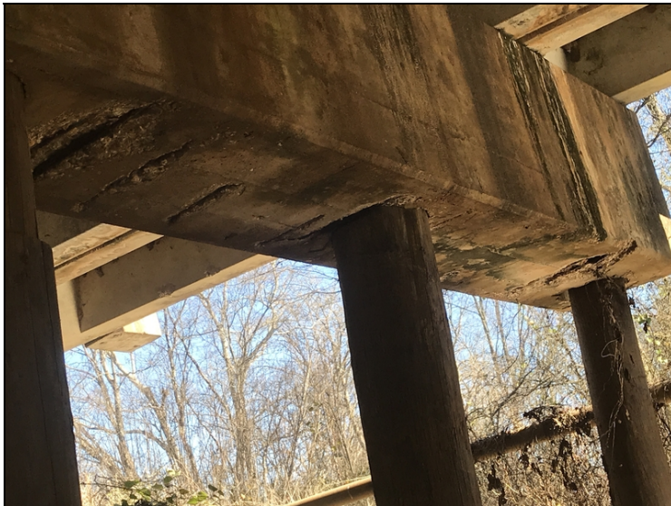
Bent 4 cap has spall with exposed rebar under and on edges of cap.
