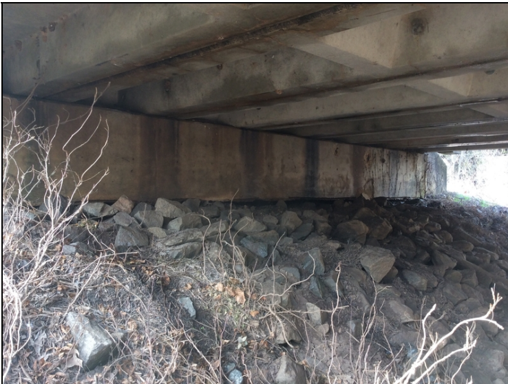
Endslope - Bent 1 (minor settlement)
