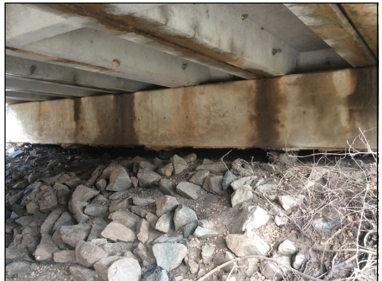
Endslope - Bent 5 (settlement)
