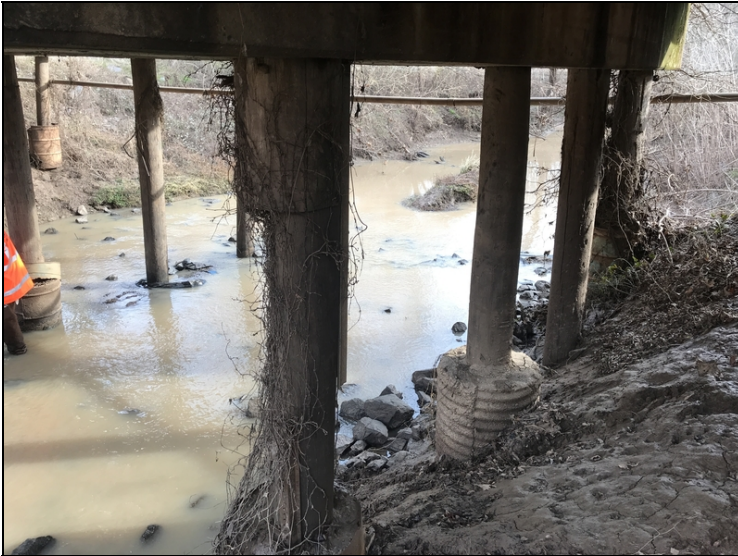
Bent 2 pile 2 no concrete collar on splice.
