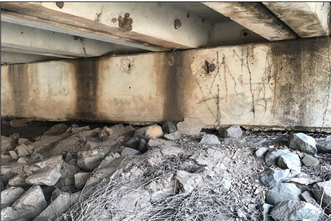
Bent 1 cap spalls with exposed rebar.
