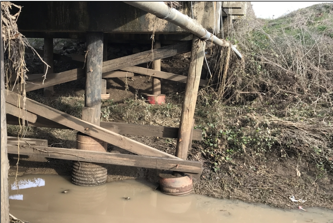
Ben 3 pile 5 has large checks.
