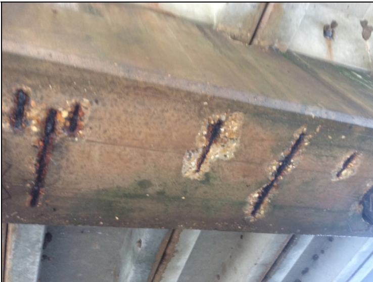
Cap - Bent 2 bottom face (corrosion)
