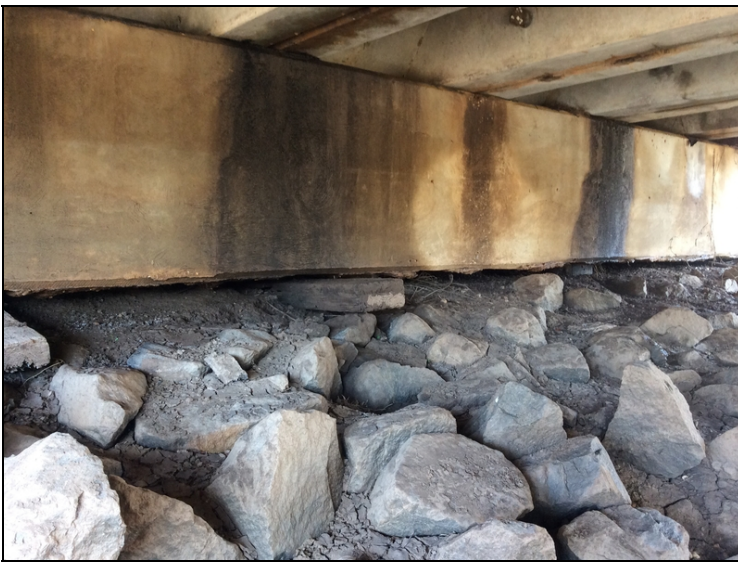
Endslope - Bent 5 (settlement)
