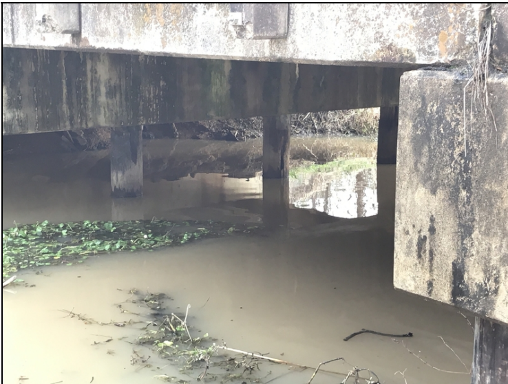
Bet 3 pile 3 hollow area 2' down from cap.
