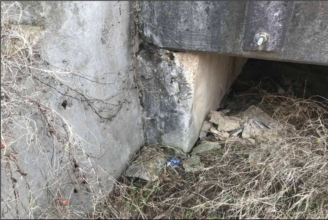
Bent 4 abutment left side has spall.
