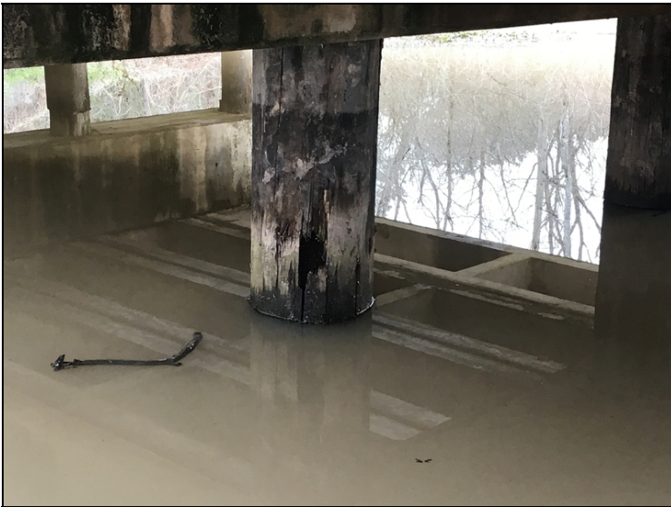
Bent 2 pile 2 hollow area 2' down from cap.
