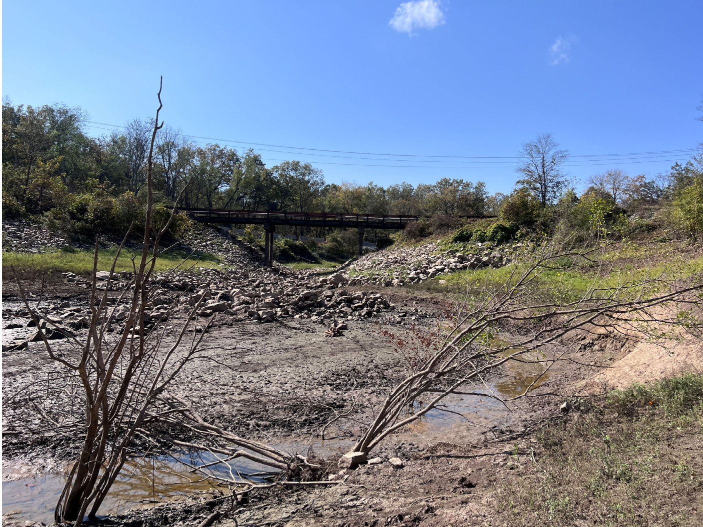
South side of bridge, looking upstream (October 2024)
