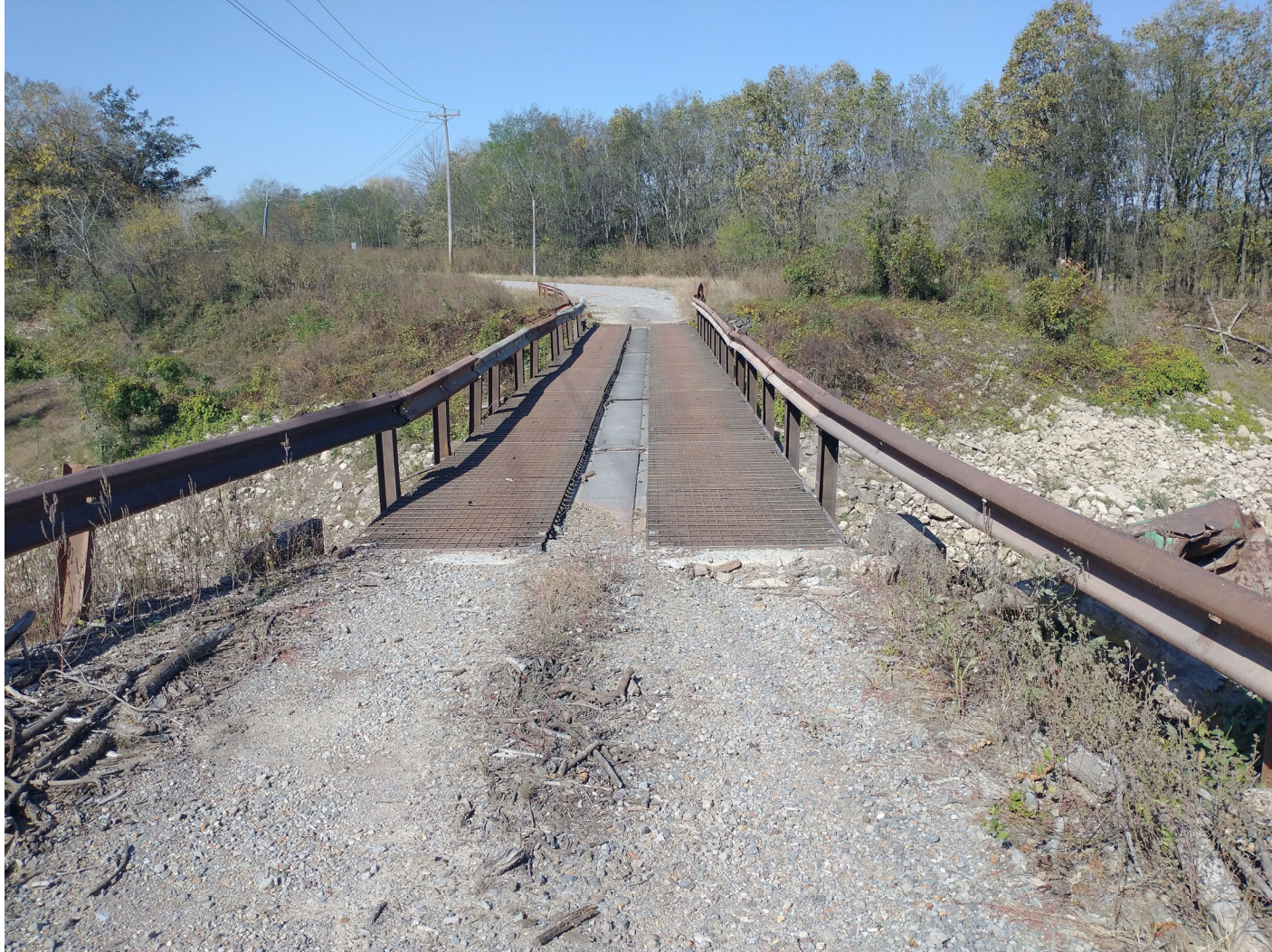
Looking at existing bridge from east bridge end (October 2024)
