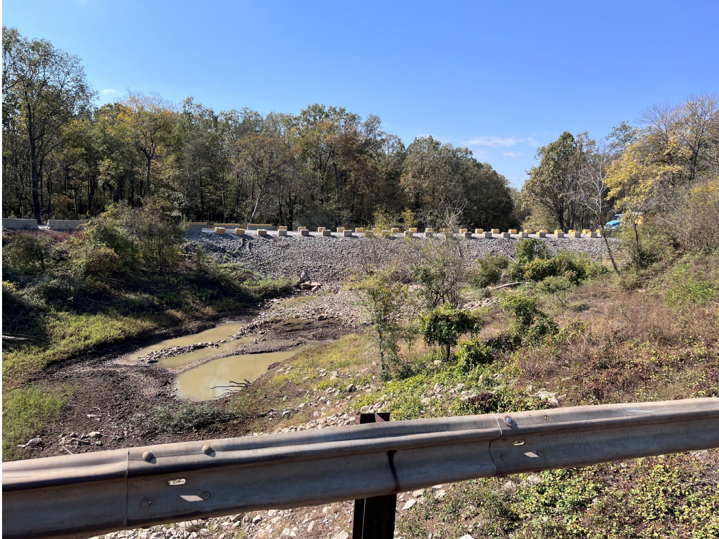
Looking south (upstream) from bridge at detour structure (October 2024)
