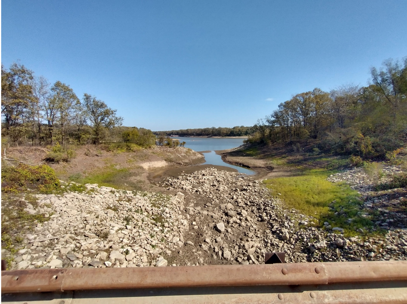
Looking north (downstream) from the bridge (October 2024)
