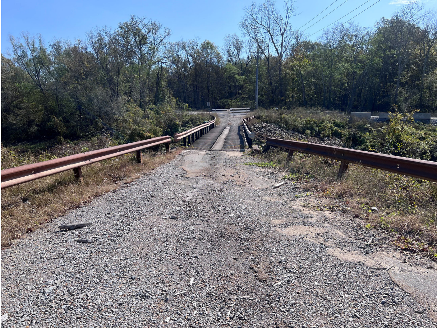
Looking at existing bridge from west bridge end (October 2024)
