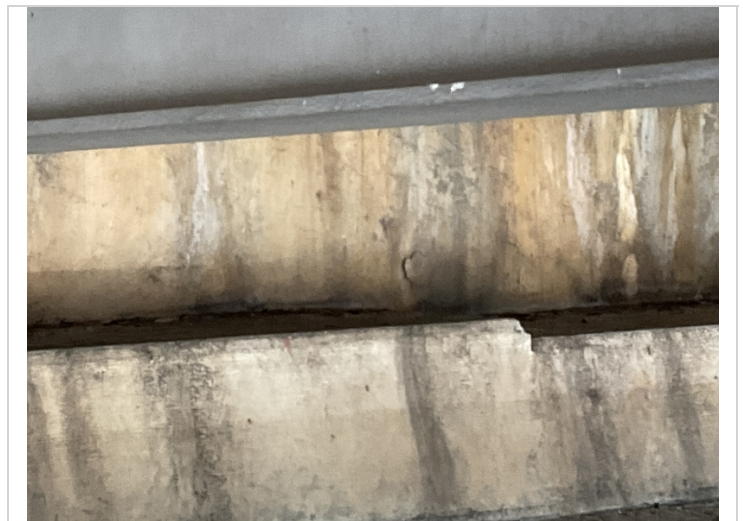
Bent 1 abutment has some cracking and a minor delam.
