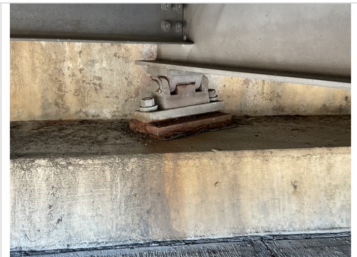
Bent 1 bearing 4 has corrosion common on all bearings.
