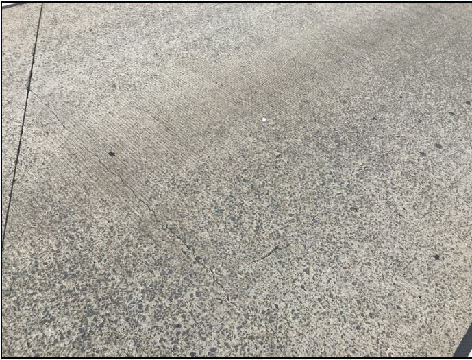
Deck - Span 2 : Cracking
