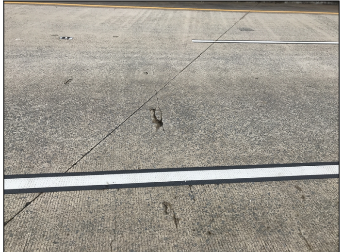
Deck - Span 2 : Spalling
