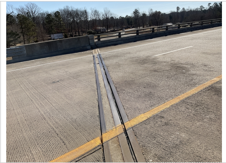
Bent 1 joint seal is torn and leaking.
