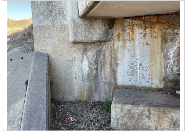
Bent 1 abutment right has cracking with delam.
