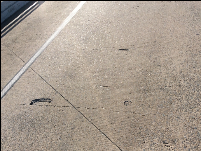
Deck - Span 1: Cracking/spalling
