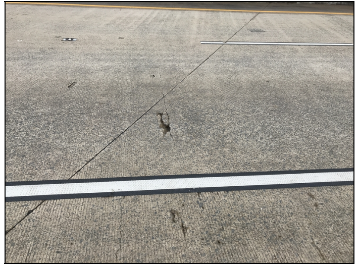
Deck - Span 2 : Spalling
