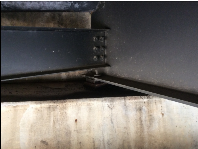
Bent 1 - Bearing 3: Missing nut
