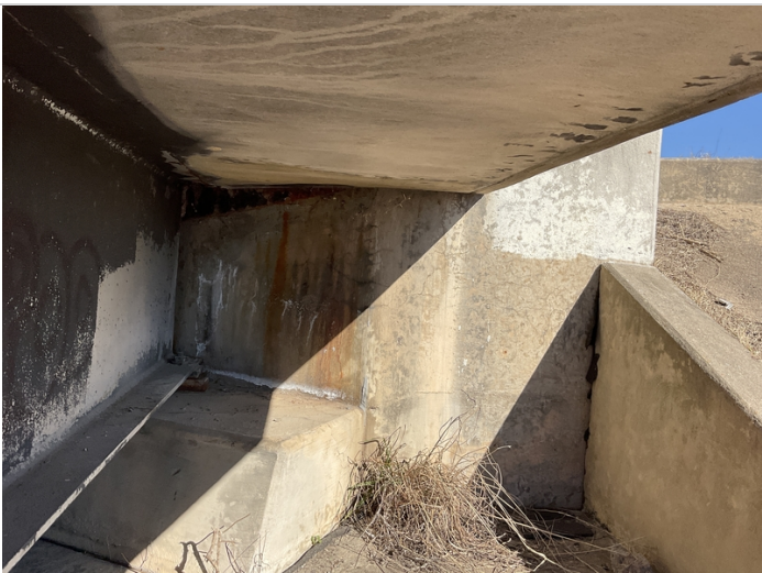
Bent 1 left at abutment has cracking with efflorescence.
