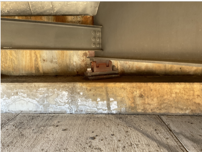
Bent 4 abutment at bearing 2 has corrosion.
