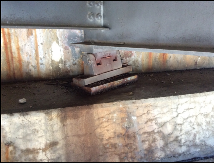
Bent 4 - Bearing 4: Missing bolt
