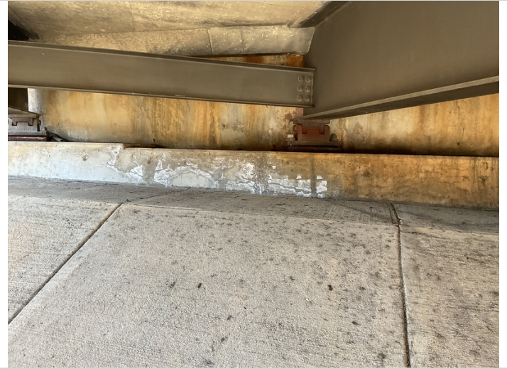
Bent 4 abutment has map cracking on step down.
