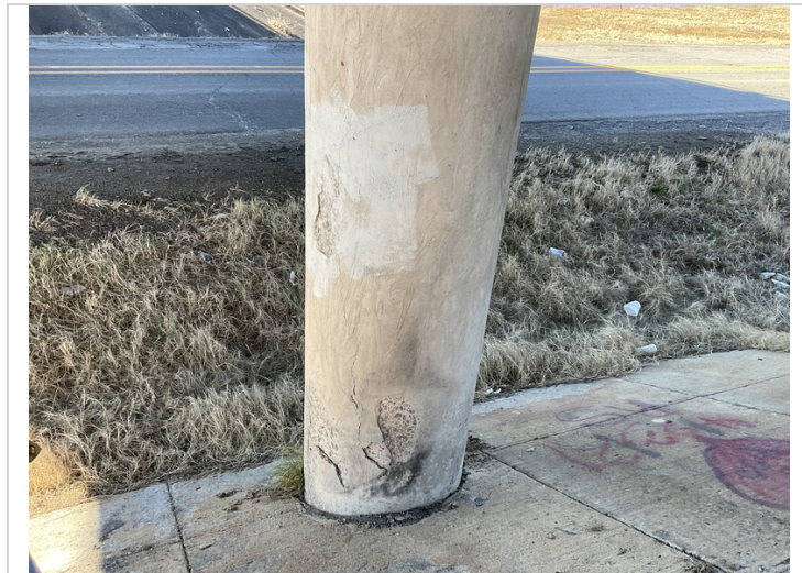
Bent 2 column 2 has cracking and spalls.
