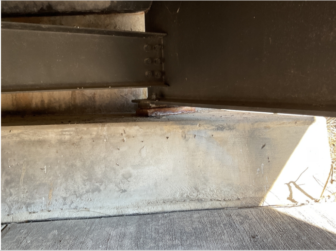
Bent 1 left bearing 1 has corrosion.
