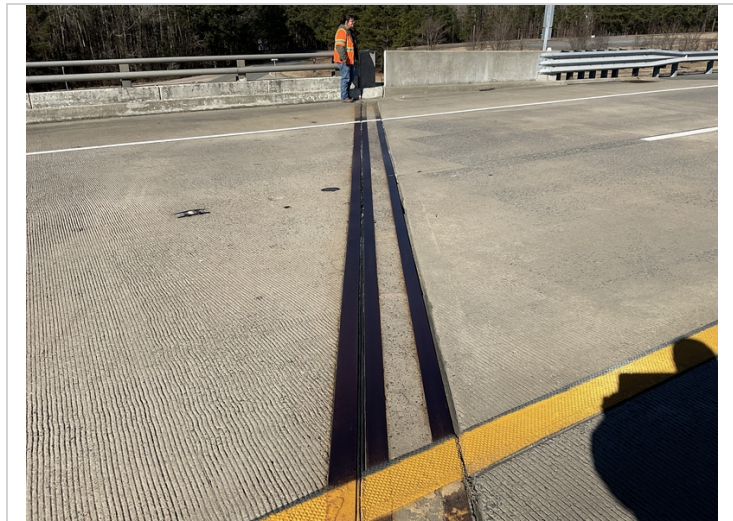
Bent 1 joint seals torn and leaking.
