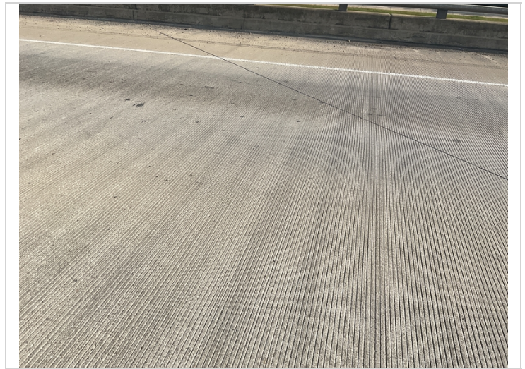
Span 3 near centerline has deck cracking.
