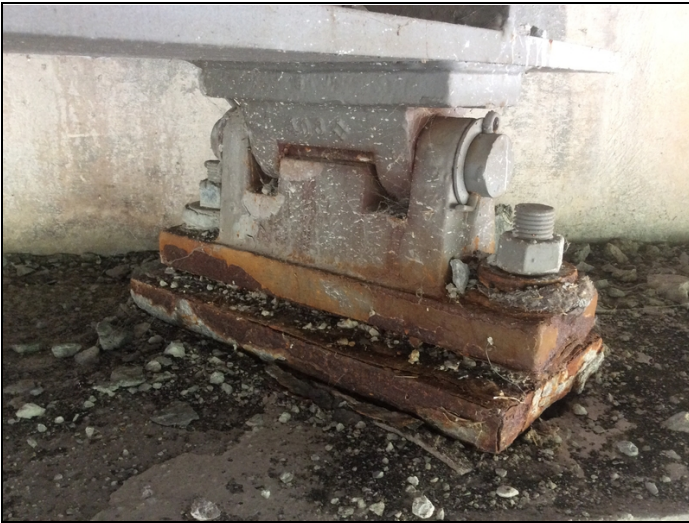
Bent 1 Bearing 2 (corrosion)
