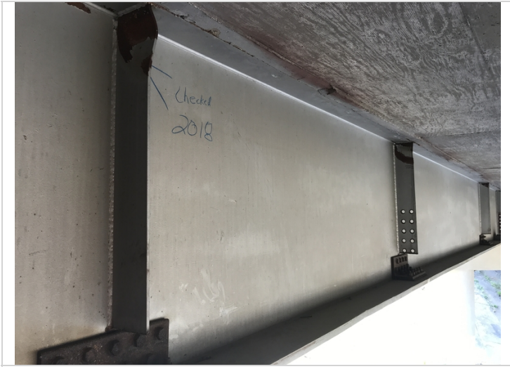
Span 2 Bay 2 left: Damage to stiffeners
