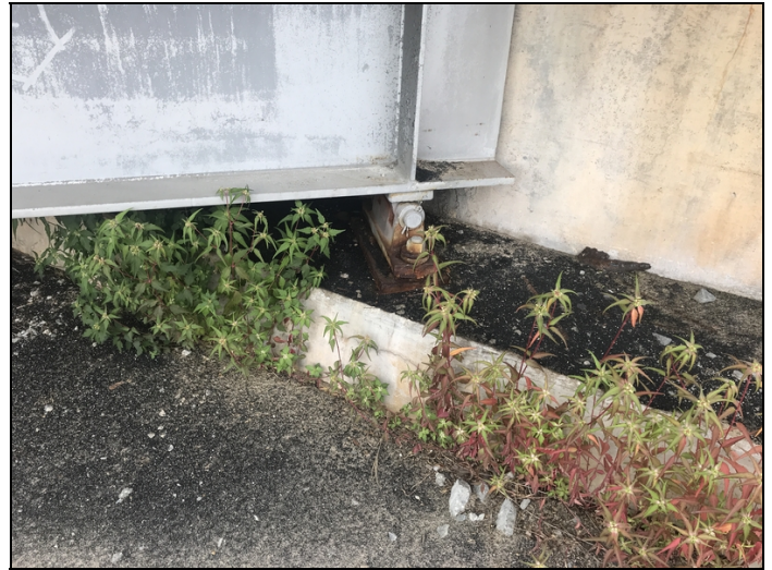
Bent 1 bearing 1 flaking rust.
