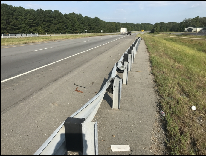
Approach railing - Bent 1 left: Impact damage
