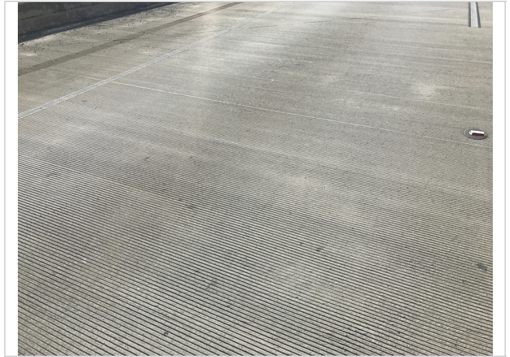
Deck - Span 2 over Girder 3: Longitudinal cracking
