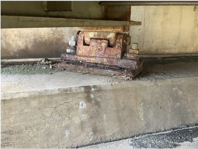
Bent 4 bearing 1 has heavy corrosion.
