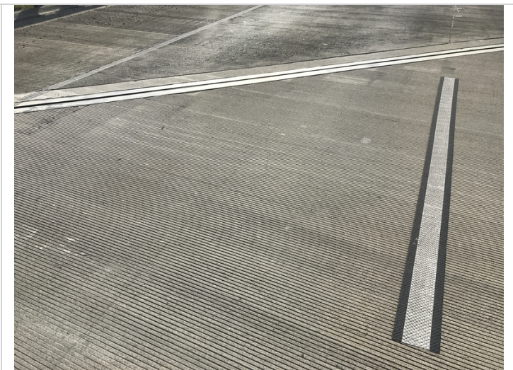
Deck - Span 1 @ Bent 1: Longitudinal cracking
