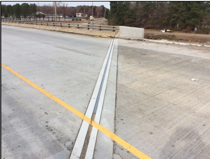
Approach slab/joint - Bent 4 (joint repaired)
