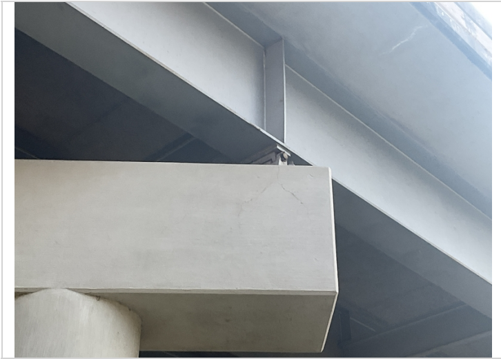
Bent 3 cap right near girder 5 has cracking.
