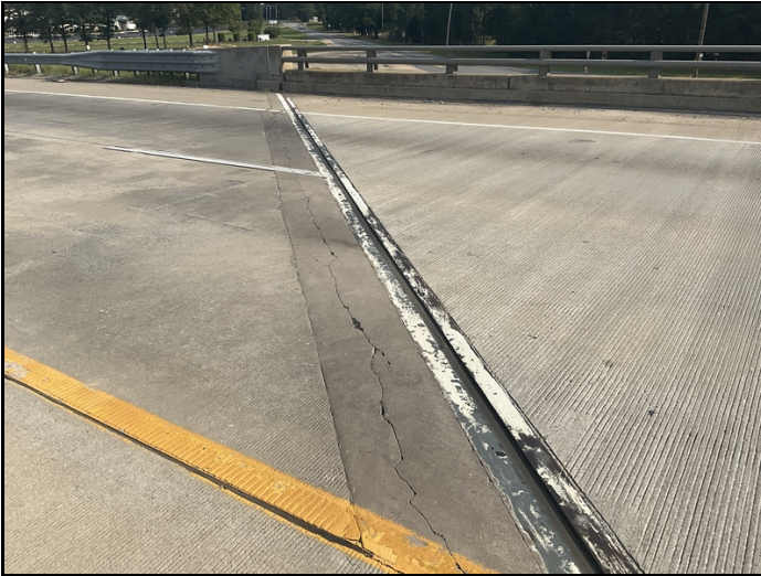
Bent 1 abutment at top of back wall has heavy cracking.
