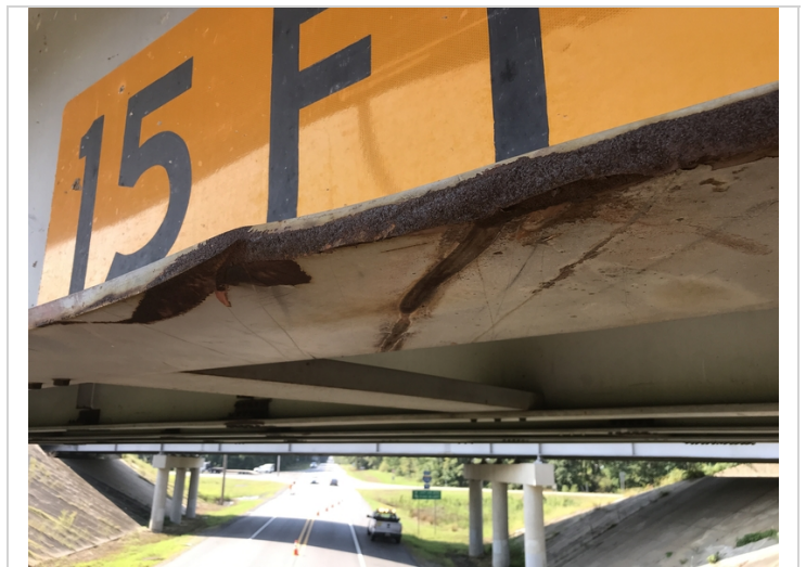
Span 2 Girder 1: Damage to bottom flange
