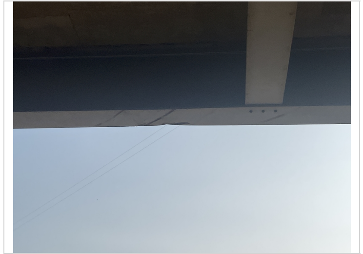
Span 2 girder 1 has traffic impact to lower flange. Damage is old.
