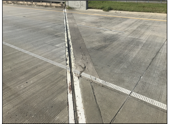
Approach slab/abutment - Bent 1 left: Cracking/spalling
