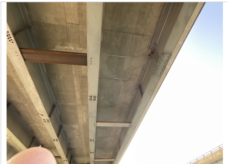
Span 2 bay 4 has cracking with efflorescence on soffit areas.
