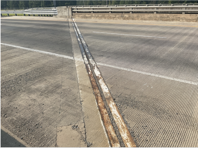
Bent 4 joint seals have some debris impaction.
