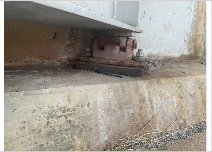
Bent 4 bearing 5 has moderate corrosion.
