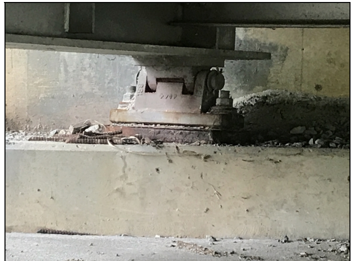
Bent 1 bearing 5 has flaking rust .
