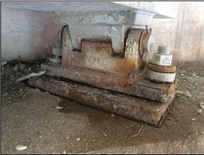
Bent 4 Bearing 4 (corrosion)
