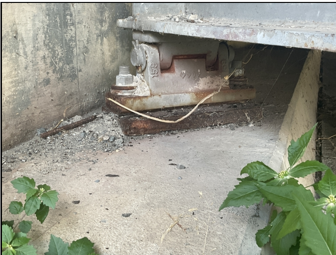
Bent 1 bearing 5 has pack rust under bearing. Common on all movable bearings.
