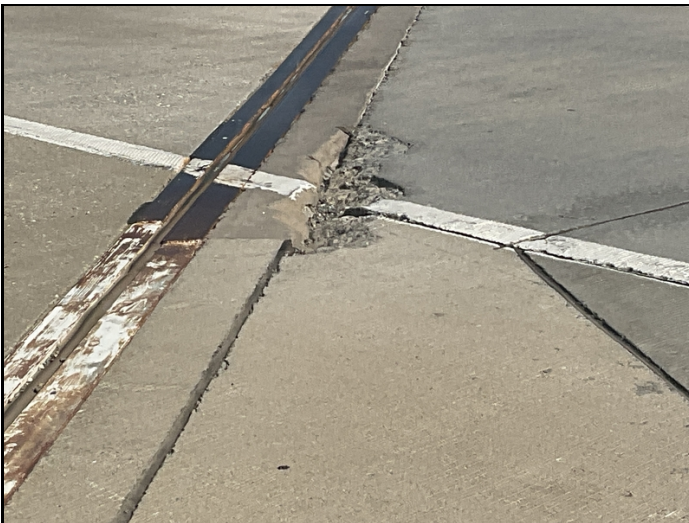
Bent 4 at end of header and approach slabs has spalls in concrete.
