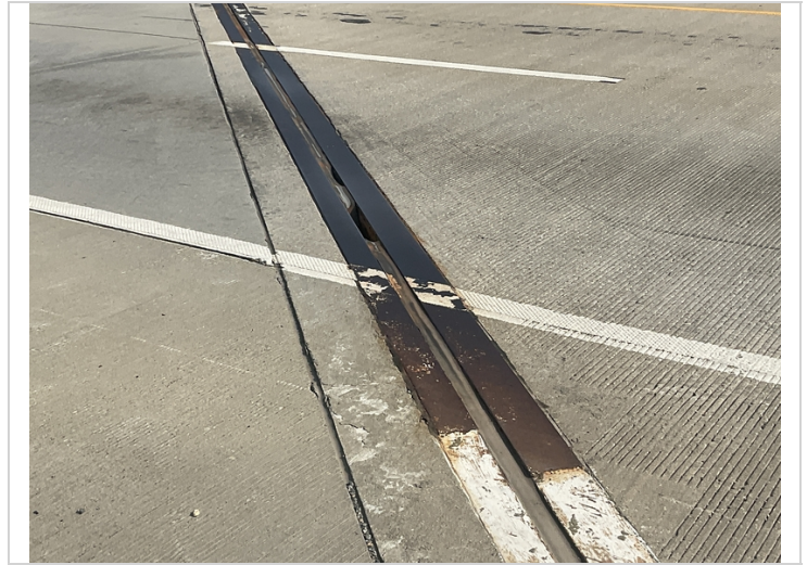
Bent 1 joint seal has loss of adhesion and is leaking.
