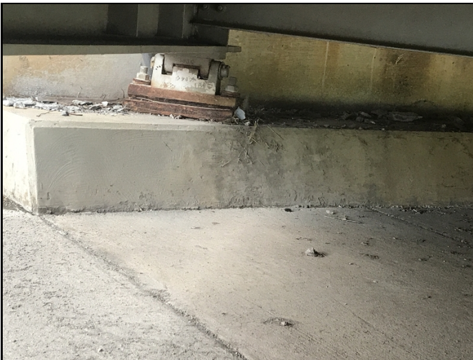
Bent 4 bearing 4 flaking rust common on bent 1 & 4 .
