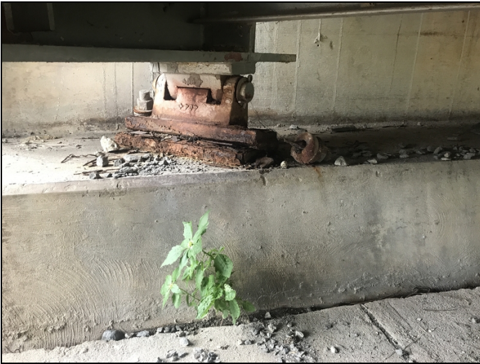
Bent 1 bearing 5 has heavy flaking rust and anchor bolt rusting away,
