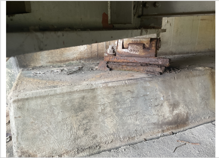
Bent 1 bearing 5 has heavy flaking rust.
