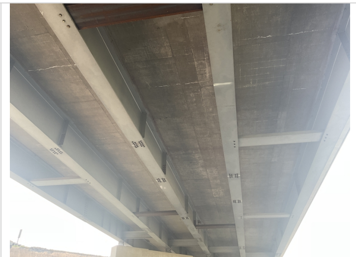
Under view of old repairs and cracking with efflorescence on soffit areas of deck.
