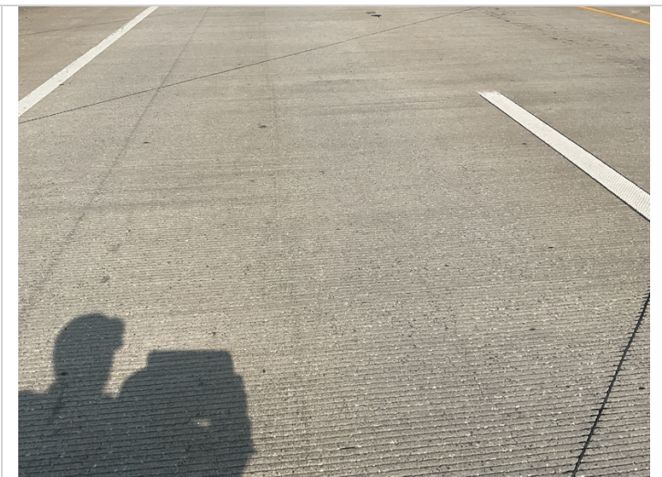
Span 2 near center line has longitudinal cracking in deck.
