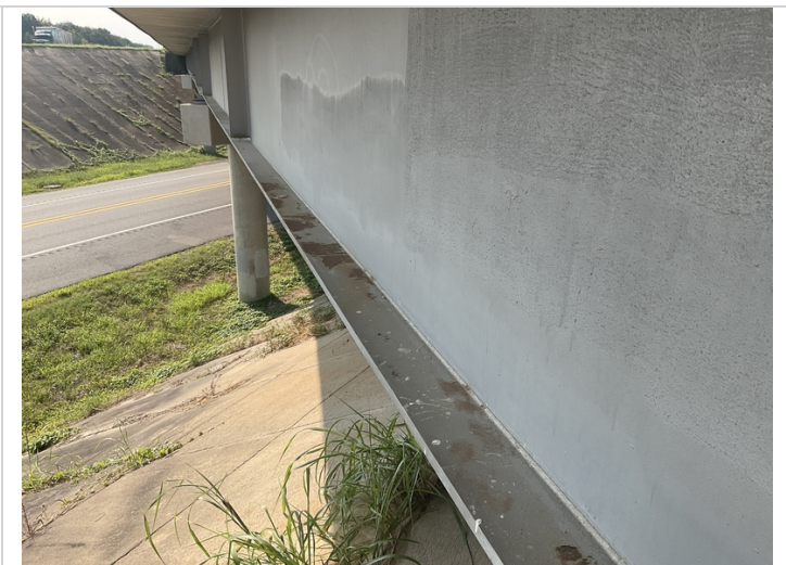
Span 1 girder 1 has peeling paint and some rust in areas on bottom flange.
