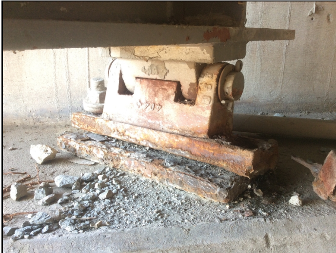
Bent 1 Bearing 5 (anchor bolt rusted away)
