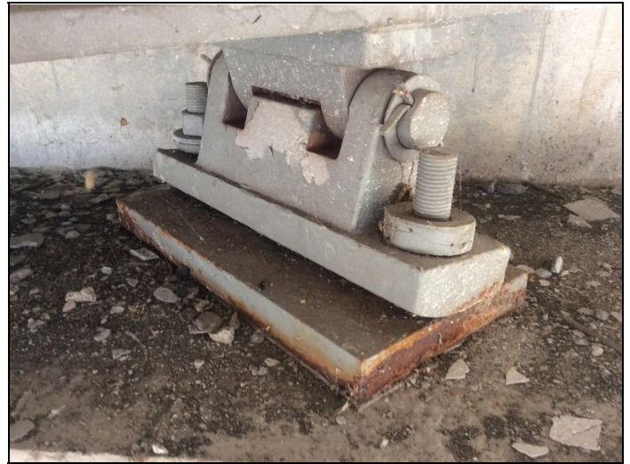
Bent 1 Bearing 2 (anchor nut missing)
