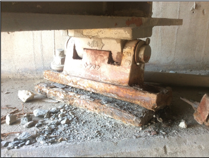
Bent 1 Bearing 5 (anchor bolt rusted away)
