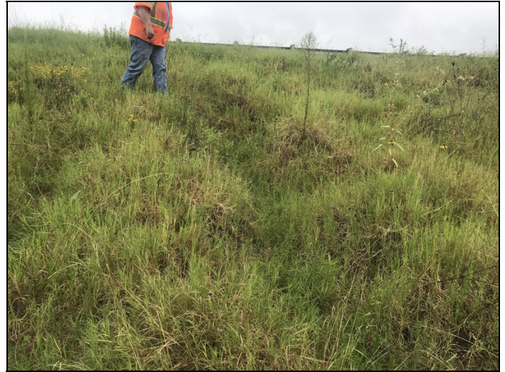
Approach roadway - Bent 1 right: Slope erosion
