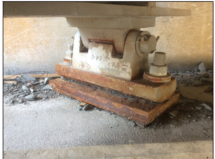
Bent 4 Bearing 1 (corrosion)
