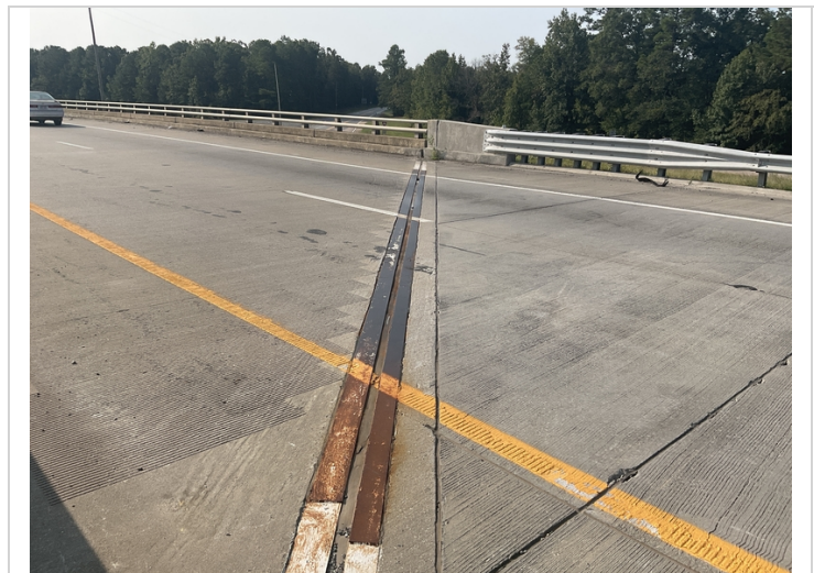
Bent 1 joint seal has small holes and seals and are leaking.
