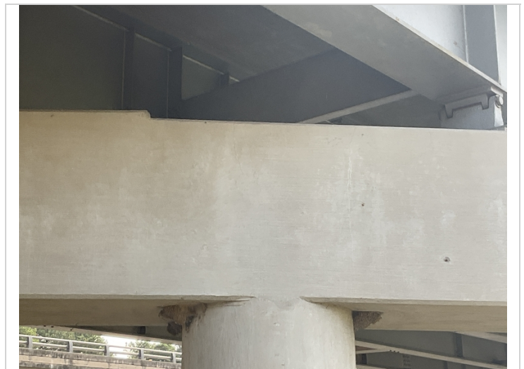
Bent 2 cap right back over column 3 has moderate cracking.
