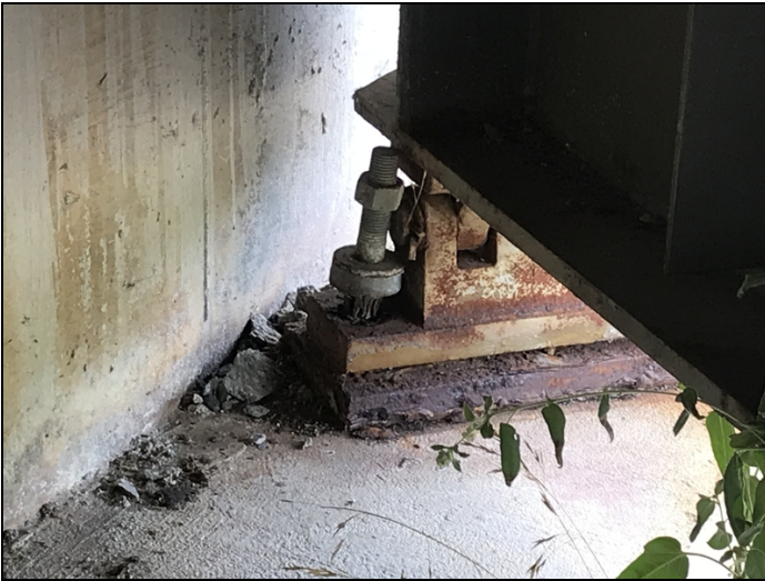
Bent 4 Bearing 5 left: Bolt corroded and worked out
