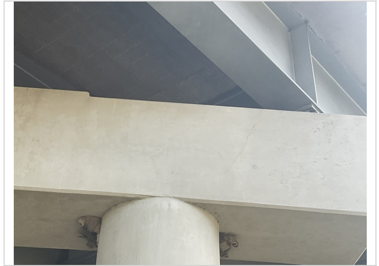
Bent 3 cap right behind has moderate sizes cracking
