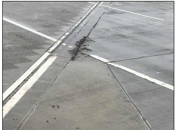
Bent 4 approach slab has potholes near joint armor .
