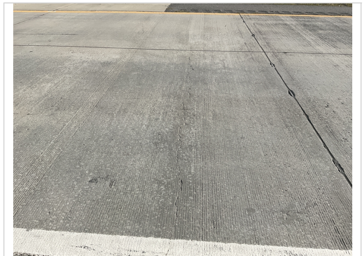
South end of approach slab has moderate cracking.
