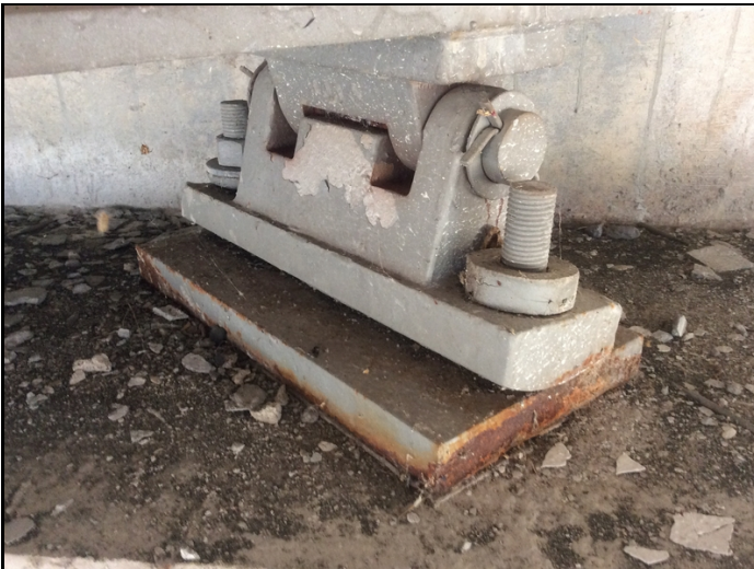
Bent 1 Bearing 2 (anchor nut missing)
