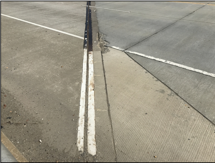
Approach slab - Bent 4 right: Spalling/potholes
