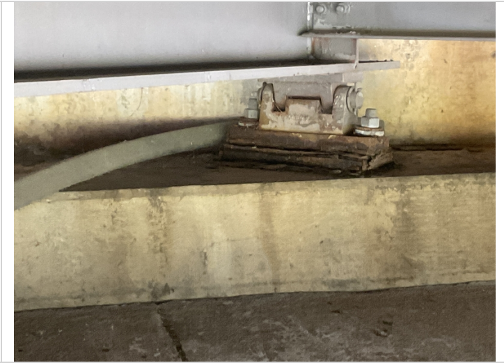
Bent 4 bearing 3 has heavy flaking corrosion.
