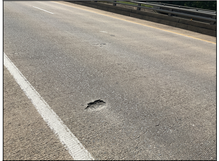
Spans 2 left has small spalls and heavy map cracking.
