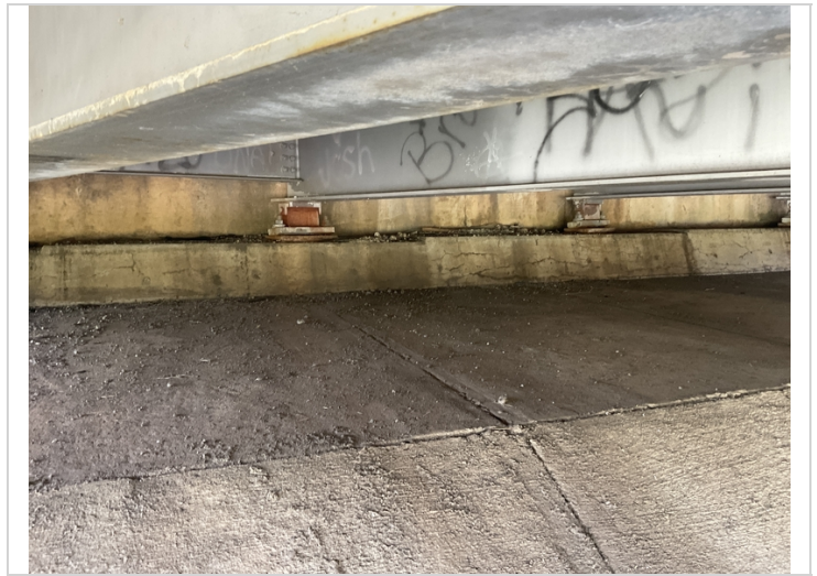
Bent 4 abutment has cracking.
