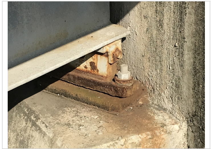
Bent 1 Bearing 1: Corrosion
