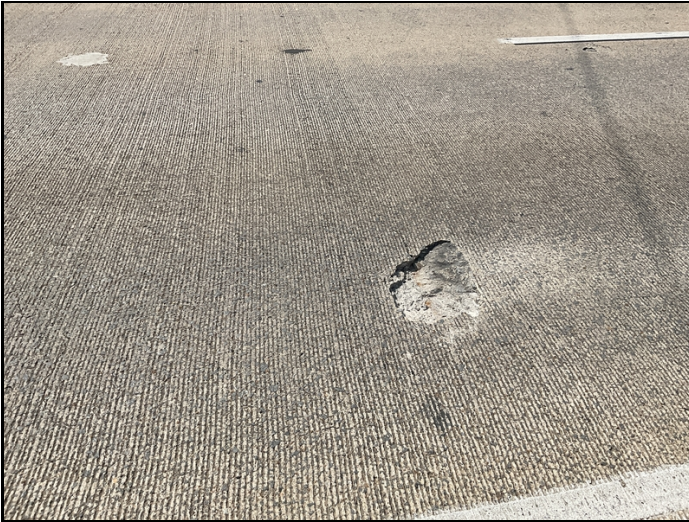
Span 1 left side as approach has small spalls.
