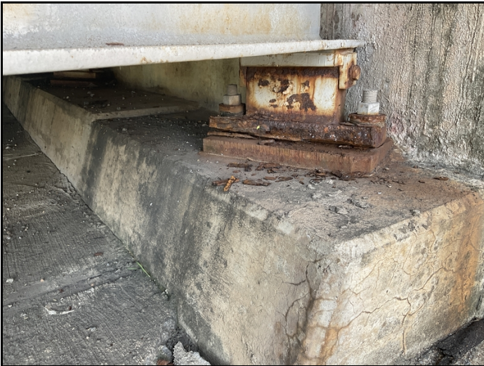
Bent 1 bearing 1 has heavy flaking rust.
