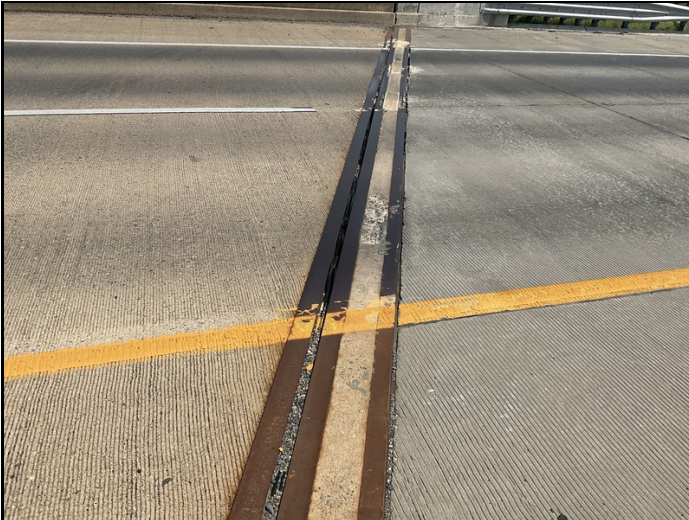
Bent 4 joint seal has loss of adhesion and is leaking.
