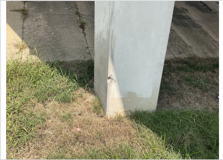
Bent 2 column 3 right has small spall.
