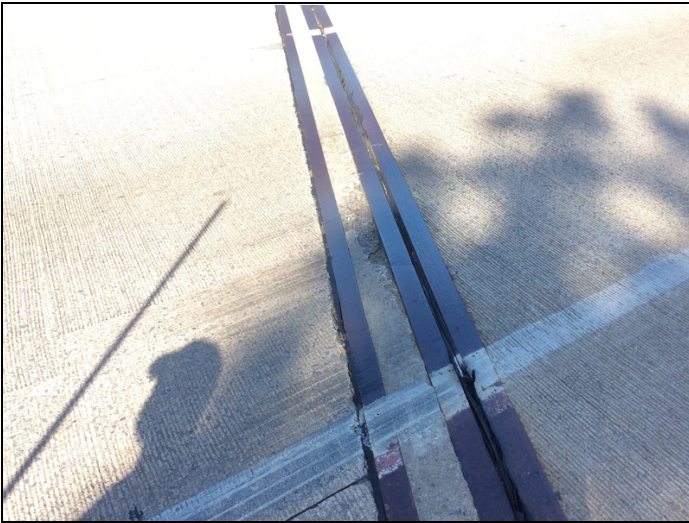
Joint - Bent 4 left (spalling of backwall)
