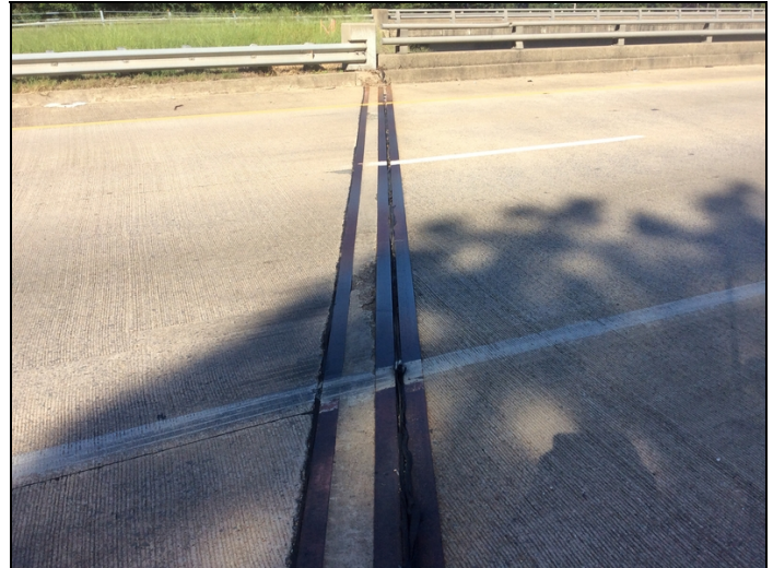
Joint - Bent 4 (tattering and loosing adhesion)
