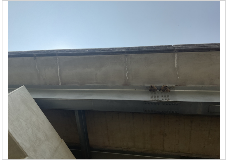
Cracks with efflorescence on soffit all spans mainly on outside areas.
