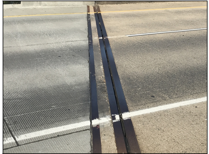
Joint - Bent 4 left: Spalling of adjacent deck/loose road iron
