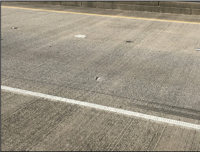
Deck - Span 1 left: Spall
