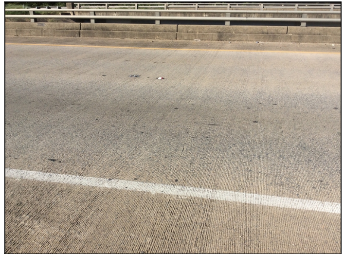
Deck - Span 2 (transverse cracking)
