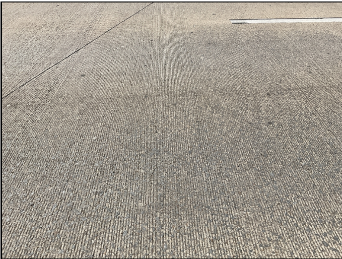
Span 2 left lane has heavy map cracking.
