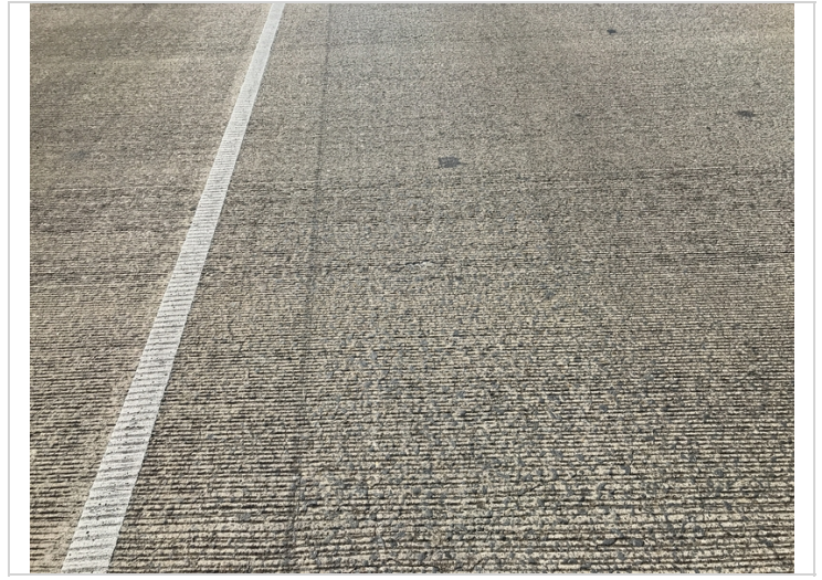
Deck - Span 1 left: Cracking
