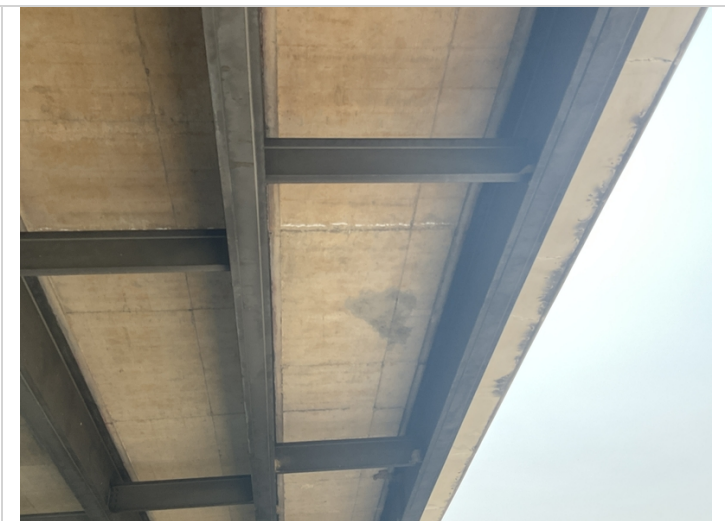
Span 2 bay 4 & 5 have cracking with efflorescence.
