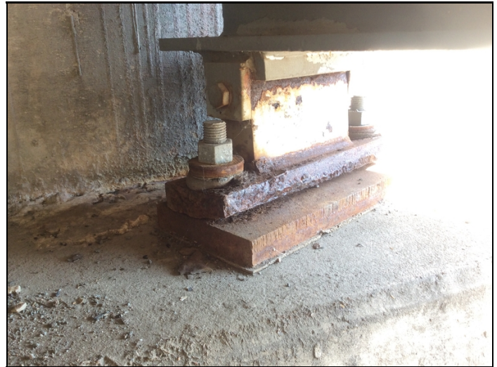
Bent 1 Bearing 1 (corrosion)
