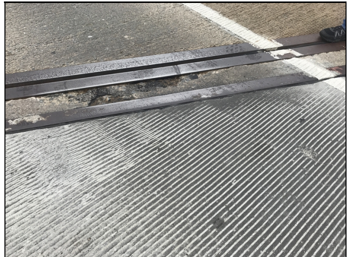
Bent 4 road iron is loose under traffic ( making noise)but still intact.
