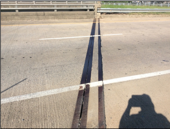
Joint - Bent 1 (loosing adhesion)
