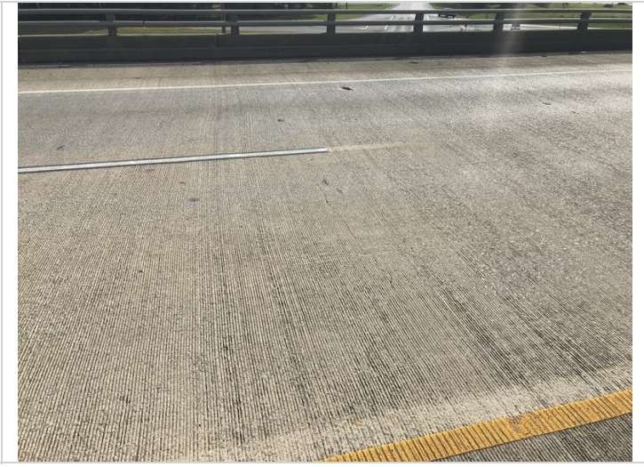
Deck - Span 2 @ midspan: Cracking
