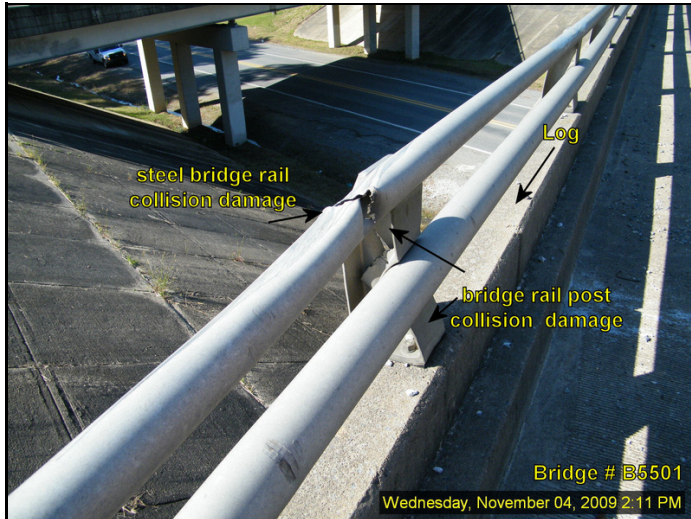
Railing - right side near Bent 4: Collision damage
