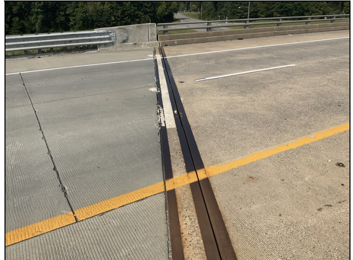
Bent 4 joint material missing.
