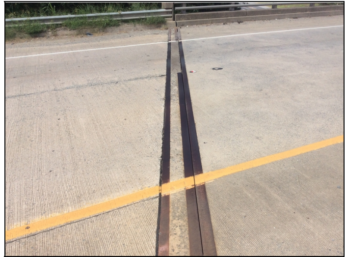
Joint - Bent 4 (material missing)
