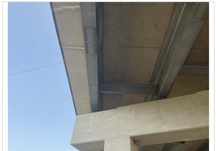
Span 1 underside of deck right side near bent 2 has cracking with efflorescence.
