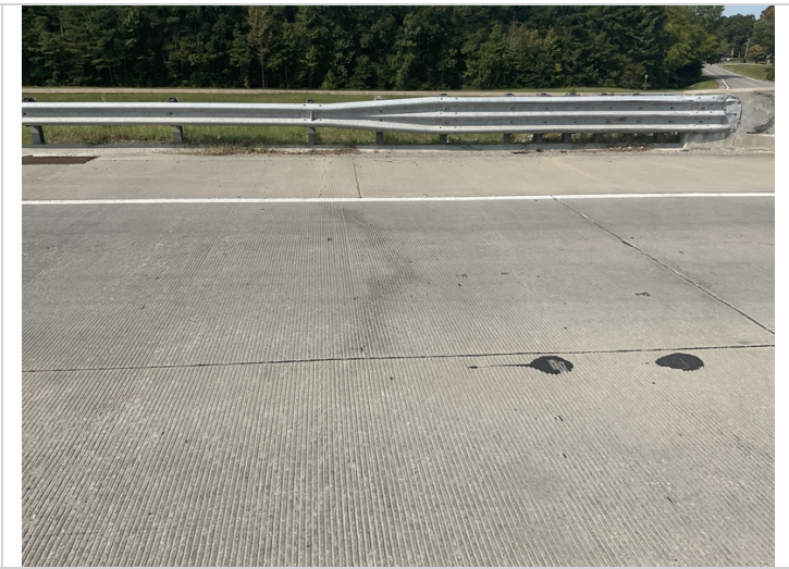
South approach slab has moderate to heavy cracking.
