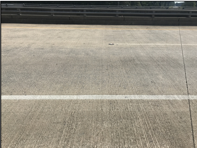
Deck - Span 2 right: Transverse cracking
