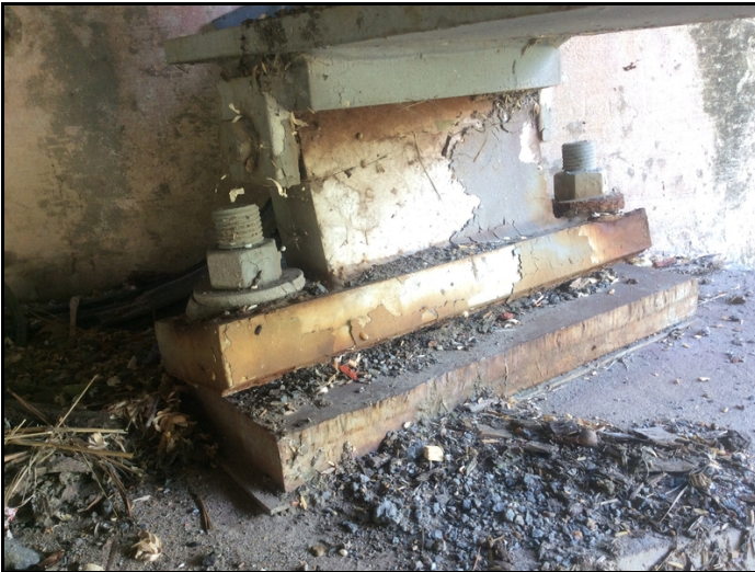
Bent 4 Bearing 6 (corrosion)
