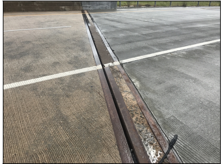
Bent 4 compression joint seal missing and road iron missing also.
