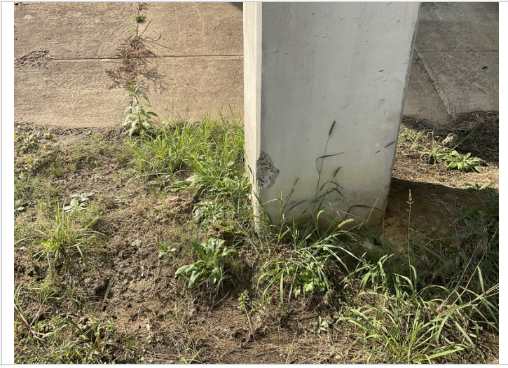
Bent 3 column 1 has minor spall.
