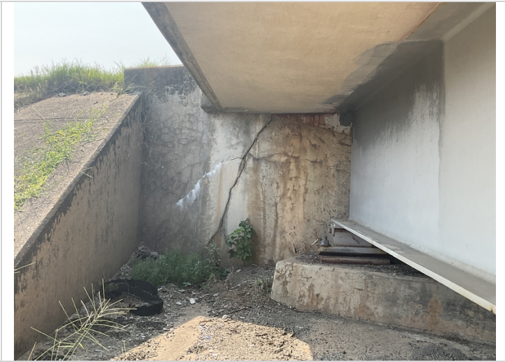
Bent 4 left at back wall has large cracks with efflorescence.
