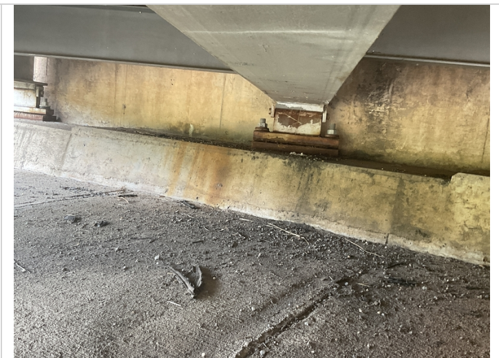
Bent 1 bearing 5 has heavy corrosion.
