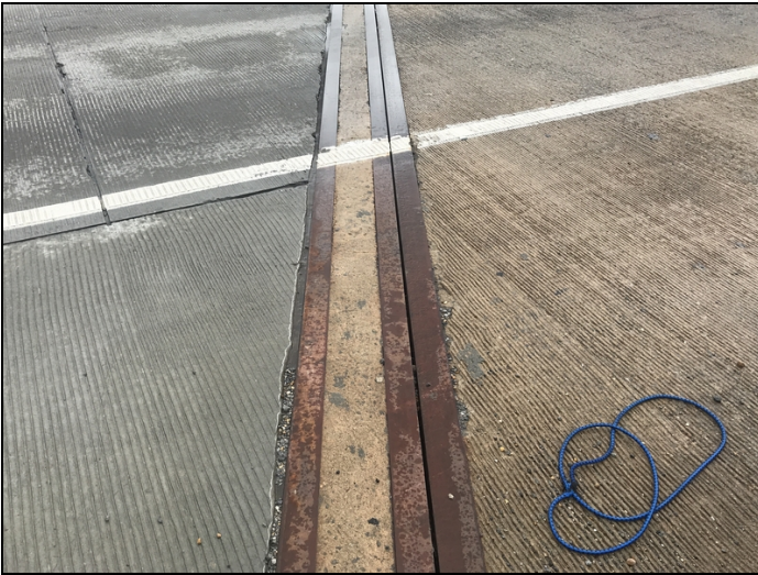
Bent 1 compression joint seal missing .
