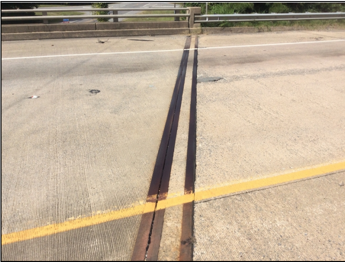
Joint - Bent 1 (material pinched)
