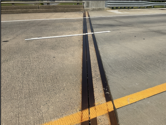
Bent 1 joint material missing.
