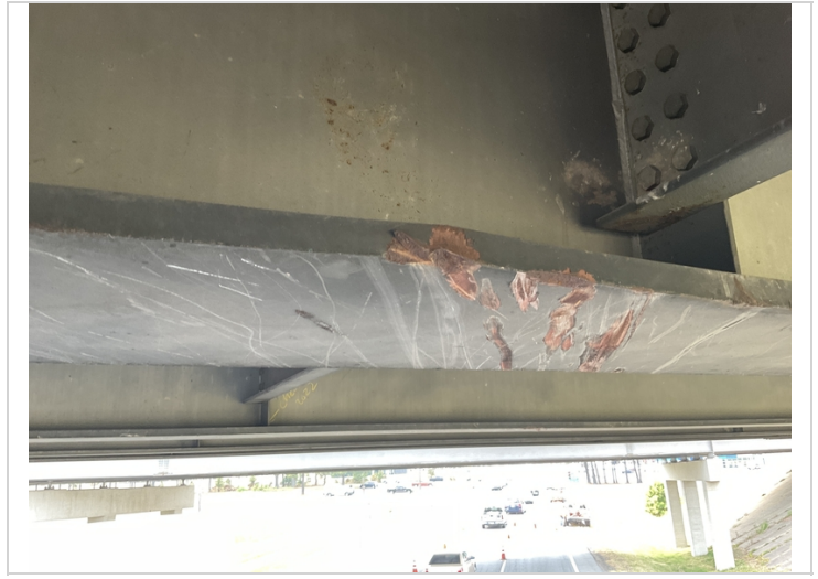
Span 2 girder impact damage.
