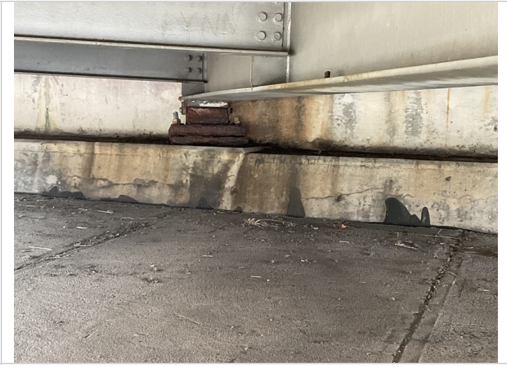
Bent 1 abutment has cracking.
