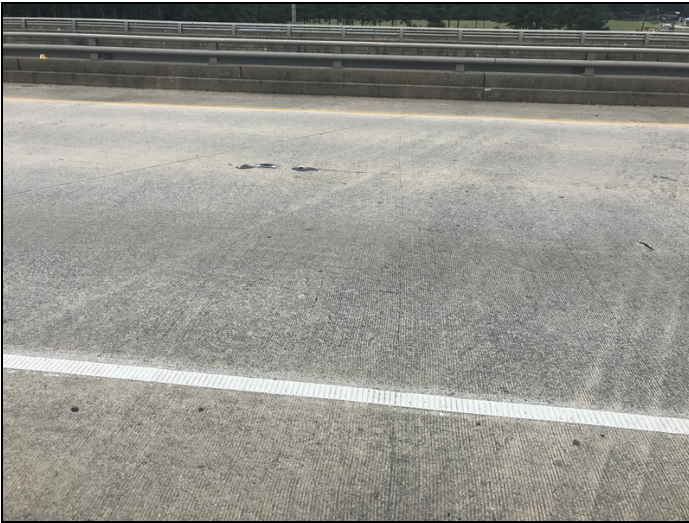
Deck - Span 1 left @ Bent 2: Cracking/minor spalling
