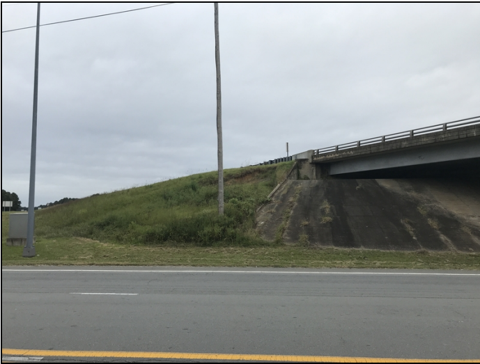
Roadway slope - Bent 4 left: Erosion/slope slumping
