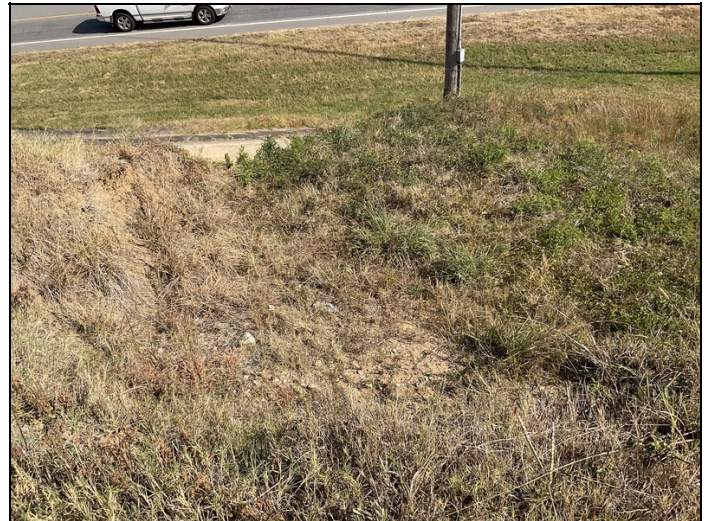
Erosion to South East side slope.
