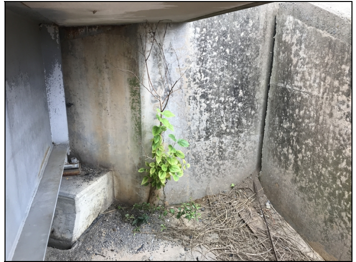
Slope paving - Bent 4 right: Moving/slumping
