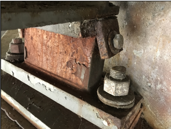
Bent 1 Bearing 2: Cracking of weld/bending out of hinge plate (ear)
