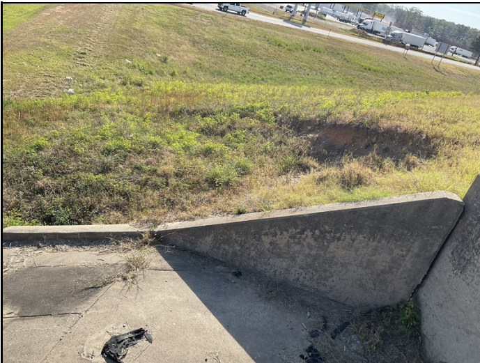
Erosion to South East side slope.
