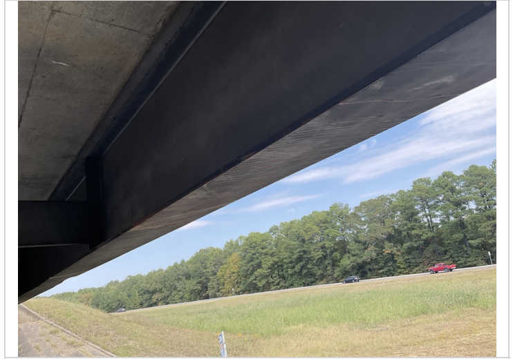
Span 2 girder 1 has scratches and scrapes.
