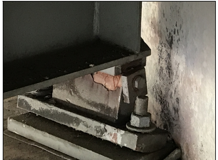
Bent 1 Bearing 4: Hinge plate (ear) broken loose
