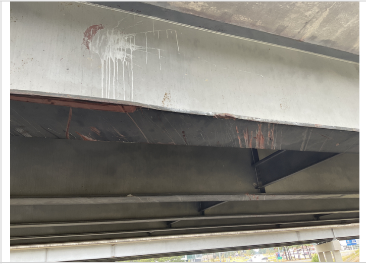
Span 2 girder 1 traffic impact.
