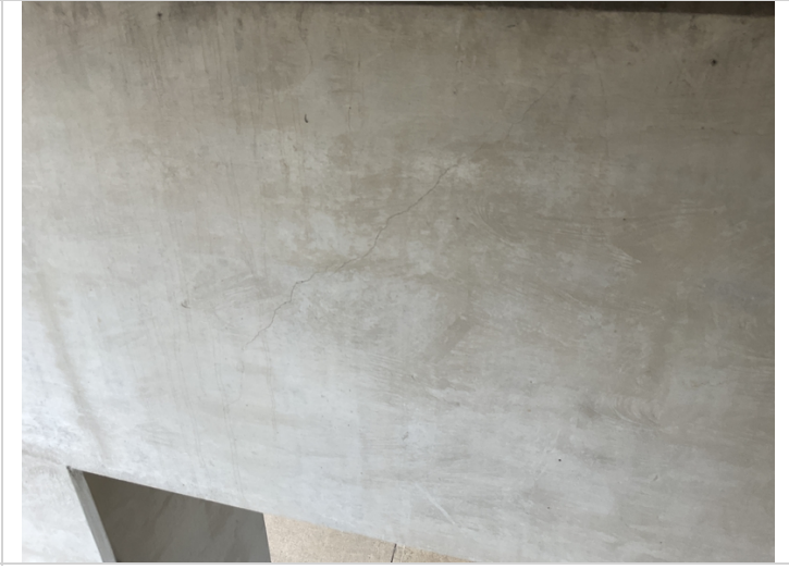
Bent 3 cap back has small diagonal cracks.
