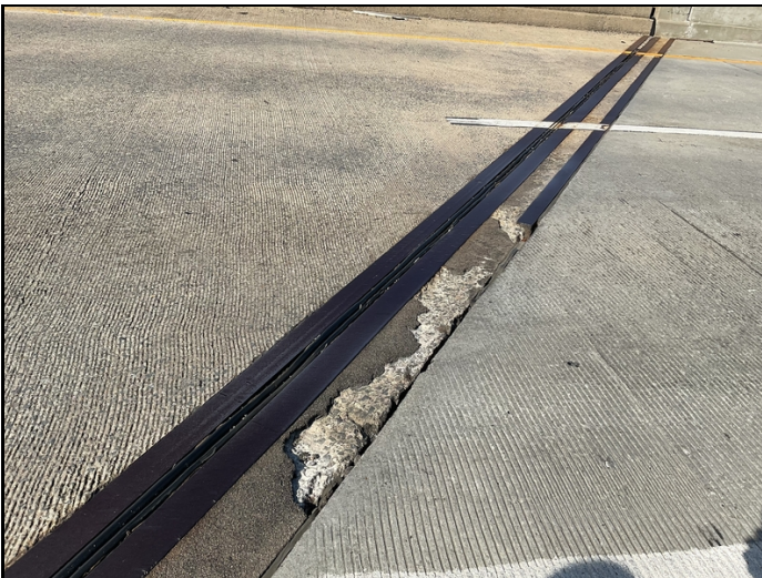
Bent 1 road iron has section missing. Common bent 4.
