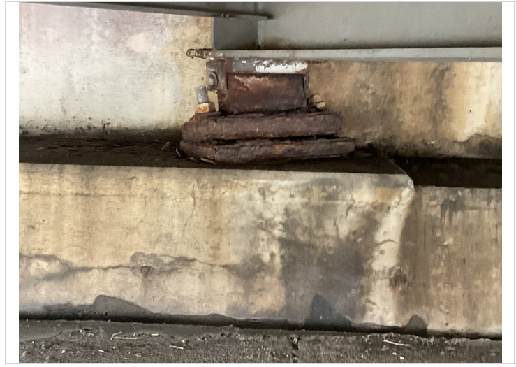
Bent 1 bearing 3 has heavy flaking corrosion..
