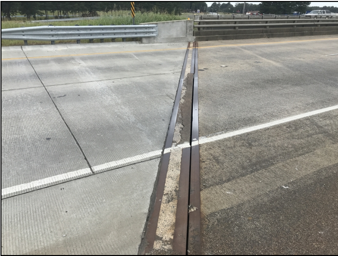
Abutment - Bent 4 left: Spalling on top of backwall
