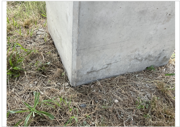
Bent 2 column 2 at ground level has cracking.
