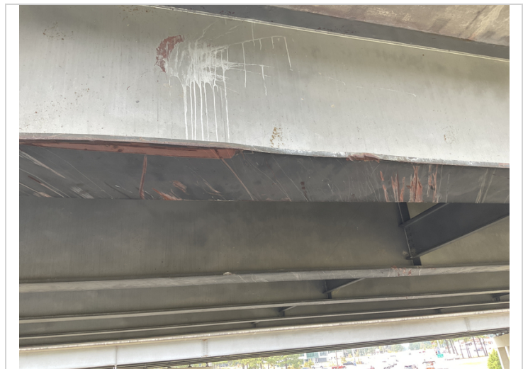
Span 2 girder 1 near mid span has previous traffic impact.
