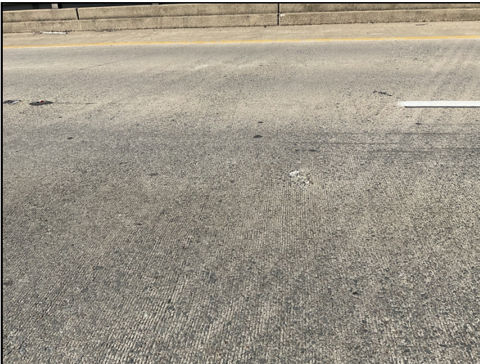
Deck span 2 has cracks and small spalls.
