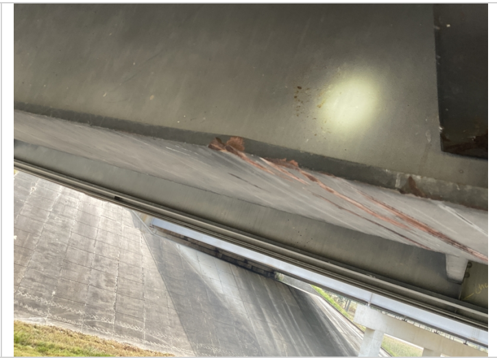
Span 2 girder 2 impact damage.
