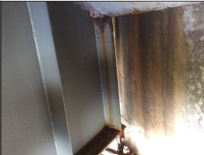
Span 1 Girder 3 @ Bent 1 (corrosion)
