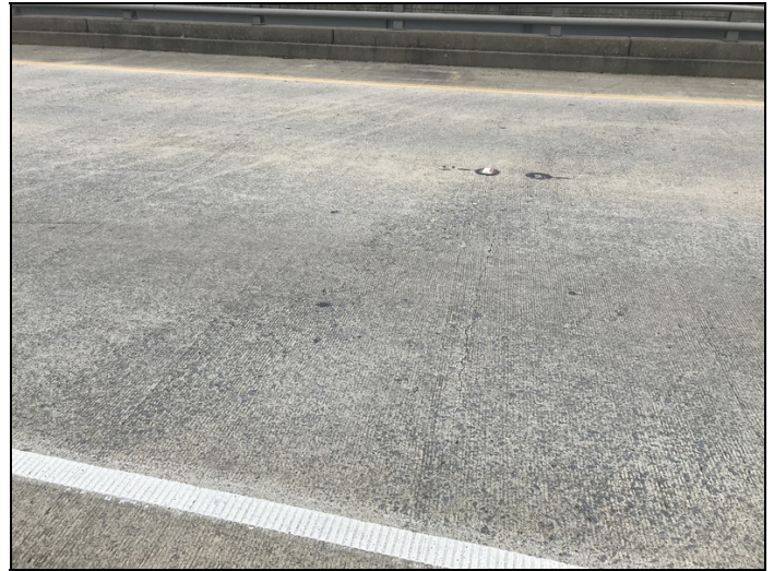
Deck - Span 2 @ midspan: Cracking/abrasive wear
