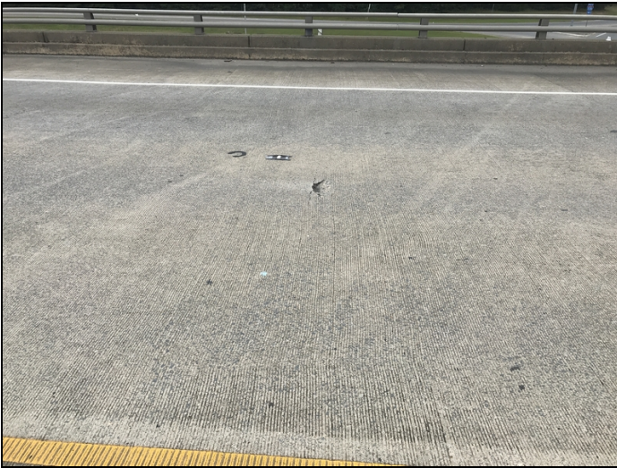
Deck - Span 2 right @ 3/4 span: Cracking/spalling
