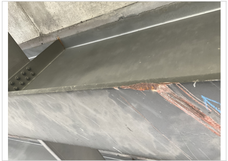
Span 2 girder 3 has traffic impact.
