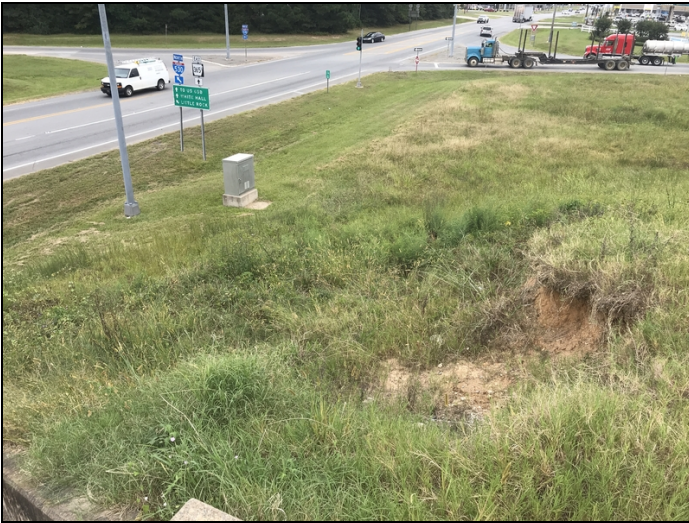
Roadway slope - Bent 4 left: Erosion/slope slumping
