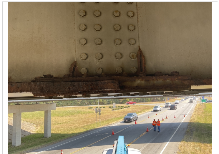
Span 2 girder 2 right at second splice plate ahead of Bent 2 has heavy rust and corrosion to lower web and flange. Pack rust forming between girders and built up members.
