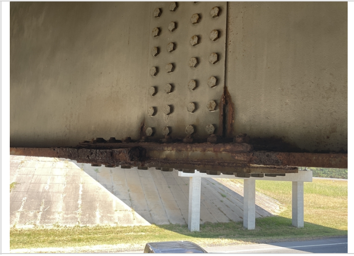
Span 2 girder 2 right at second splice plate ahead of Bent 2 has heavy rust and corrosion to lower web and flange.
