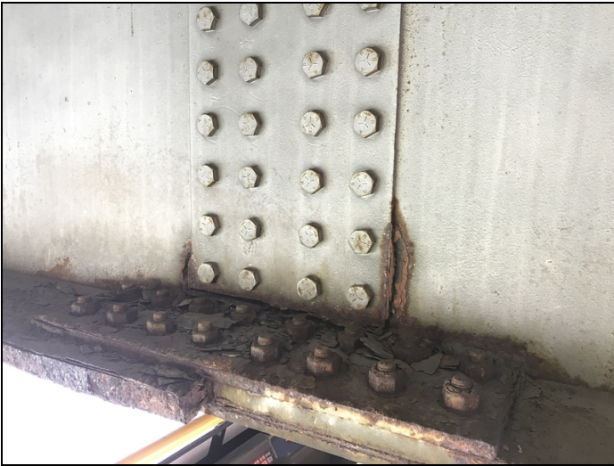
Span 2 Girder 2 @ Splice 2: Corrosion
