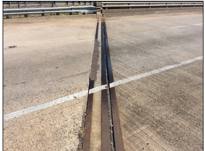
Joint - Bent 1 (leaking)
