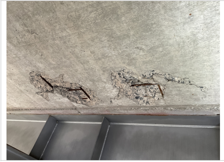
Span 1 at Bent 2 has spall with exposed rebar on under side of deck between girders 2&3.
