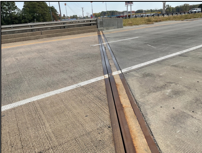
Bent 4 joints seal is missing.
