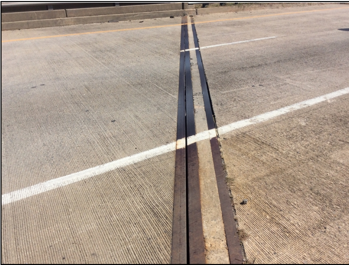
Joint - Bent 4 (loss of adhesion)
