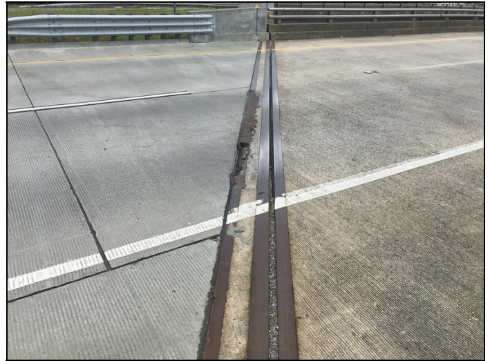
Abutment Bent 1 right: Spalling on top of backwall
