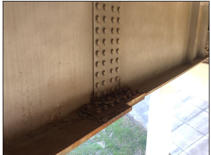
Span 2 Girder 2 @ Splice 2 (corrosion)
