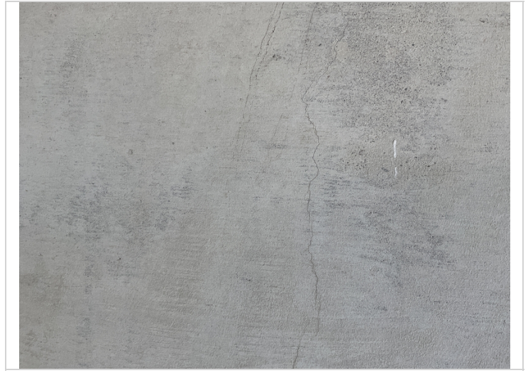
Bent 3 cap back has hairline vertical cracks.
