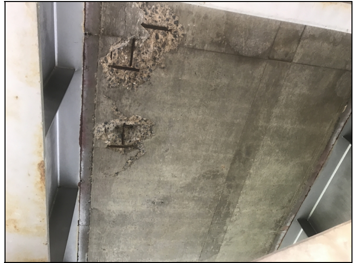
Span 2 soffit at bent 2 between girders 2-3 has spalling with exposed rebar.
