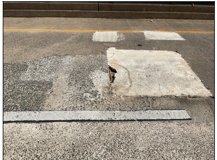
Span 2 left lane has spalls with exposed rebar and patched area.
