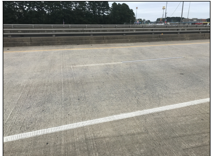
Deck - Span 2 @ midspan: Cracking
