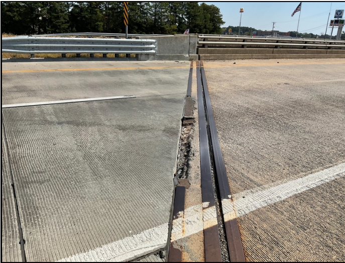
Bent 1 joint armor is missing. (with pot holes at the header).
