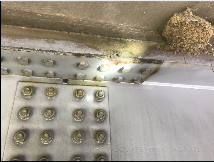
Span 2 second splice plate ahead of bent 2 girder 2 has moisture from deck.
