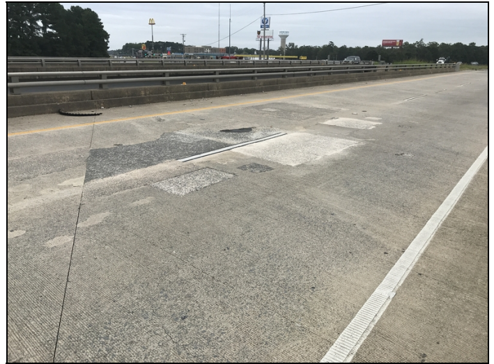
Deck - Span 2 @ Bent 2: Spalling/patches
