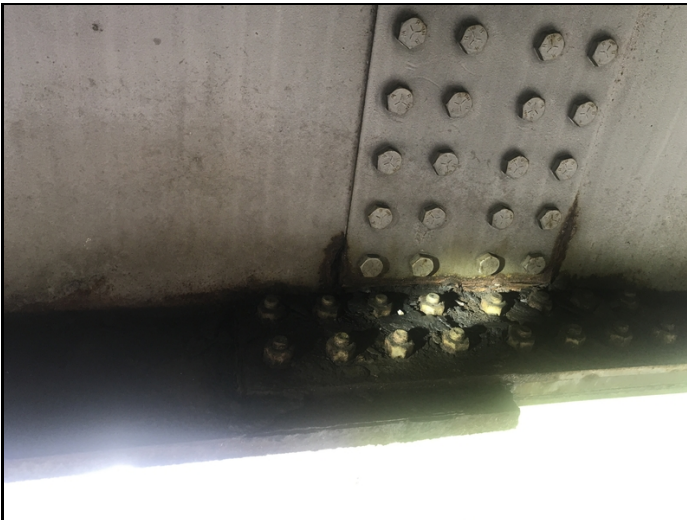
Span 2 girder 2 second splice plate ahead of bent 2 left has heavy rust with some flaking from moisture seepage.
