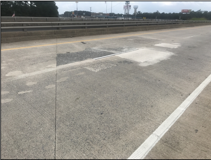
Spans 1&2 have spalls and repaired areas.
