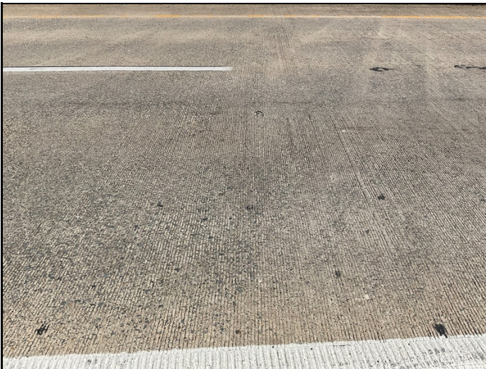
Span 2 has large unsealed cracks .
