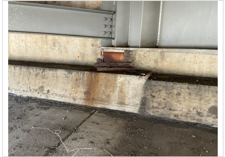
Bent 4 Bearing 3 has heavy flaking rust to masonry plate.
