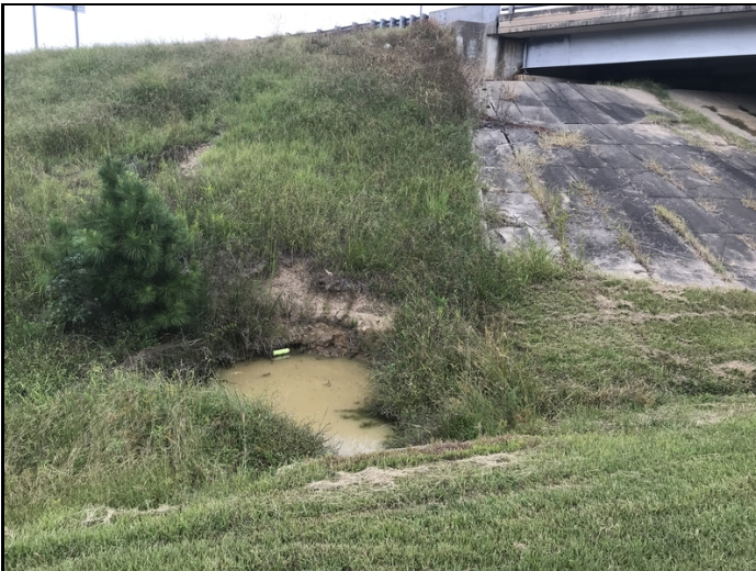
End-slope - Bent 1 right: Erosion
