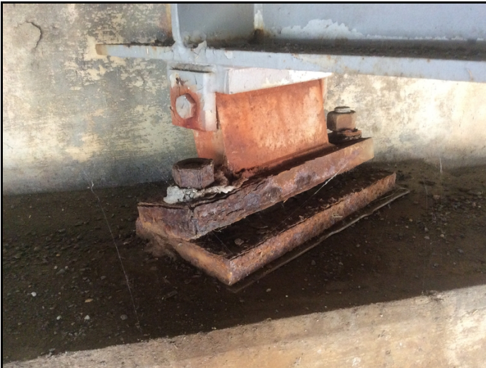
Bent 4 Bearing 3 (corrosion)
