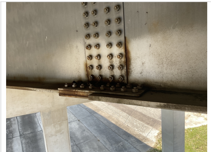
Span 2 girder 2 left at second splice plate ahead of Bent 2 has heavy rust and corrosion to lower web and flange.
