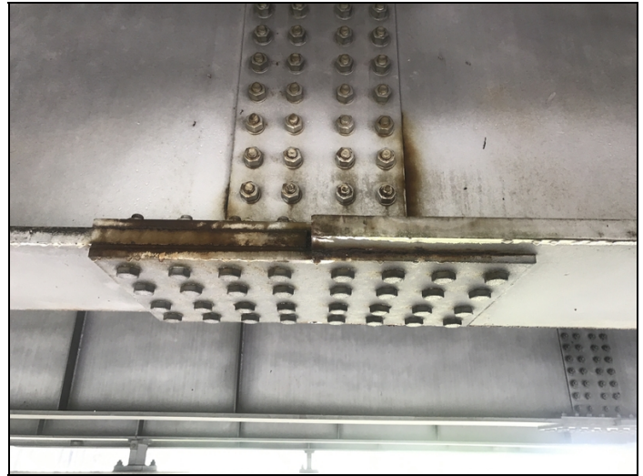
Span 2 second splice plate ahead of bent 2 girder 2 has moisture and rusting at splice plate with water running back down top of bottom flange.
