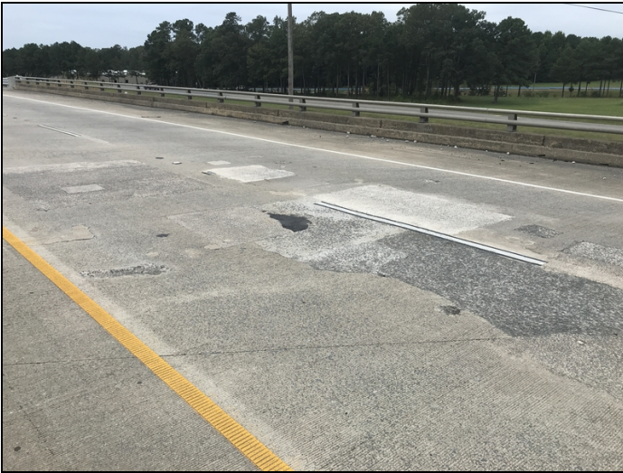
Deck - Span 2 @ Bent 2: Spalling/patches
