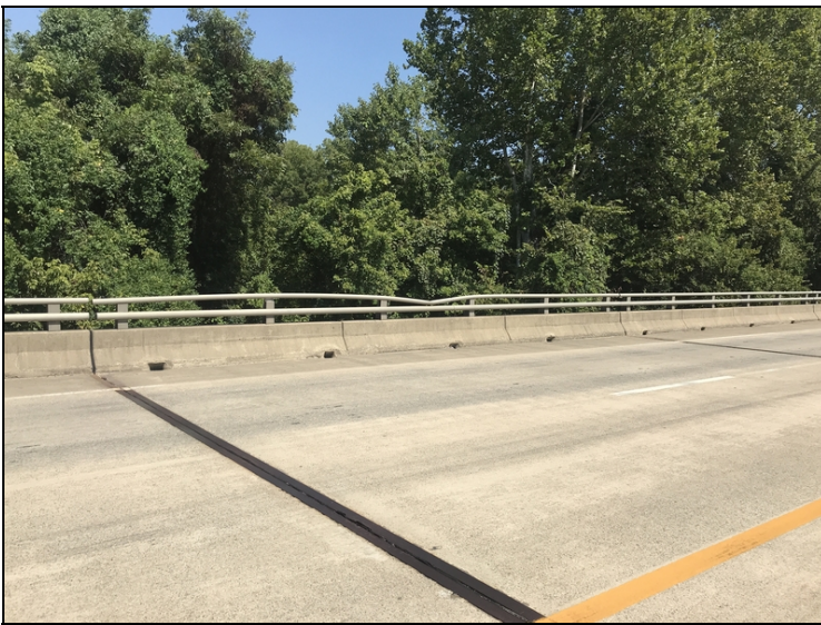
Railing - Bent 5 left: Damage
