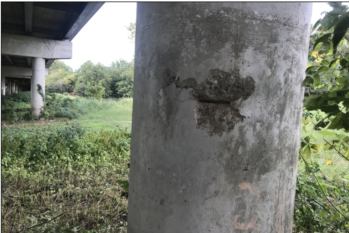
Bent 21 column 1 ahead has spall with exposed rebar.
