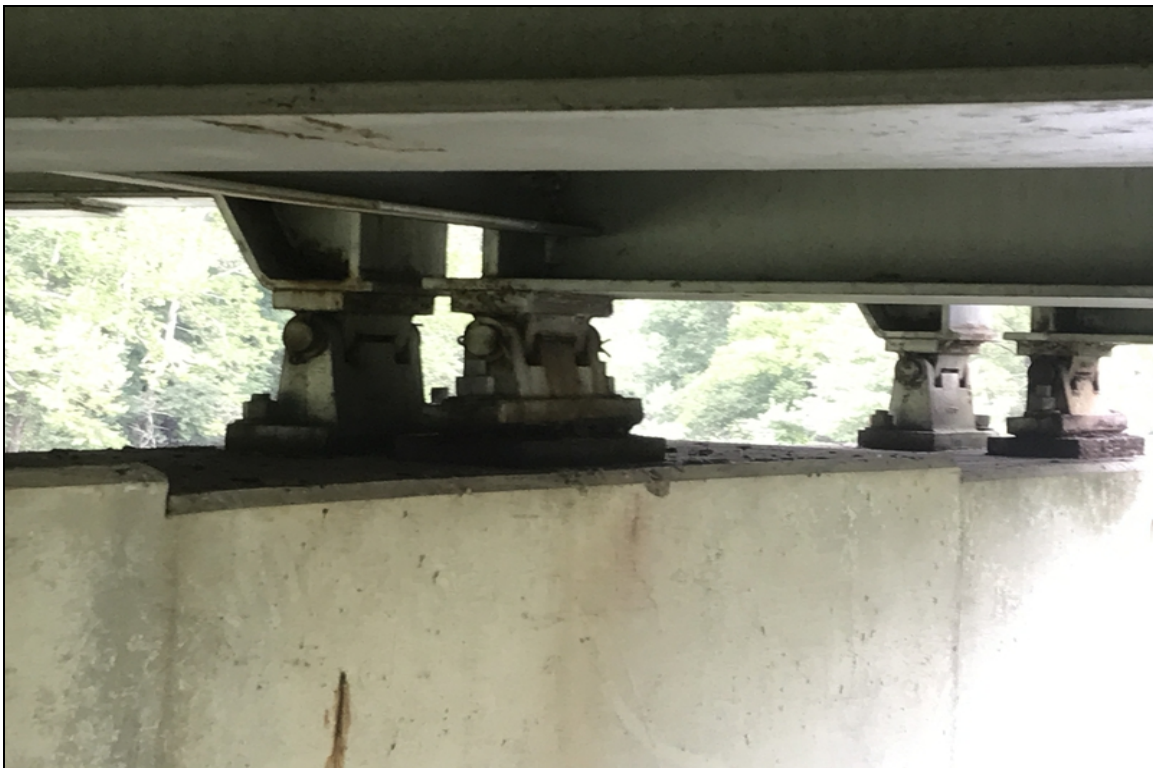
Bent 18 bearing 2 ahead is leaned back possibly due to pack rust.
