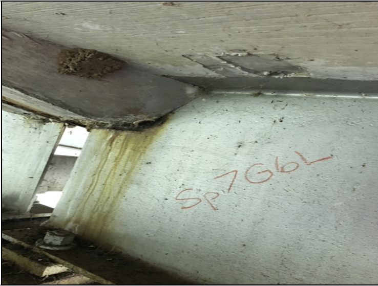
Span 7 - Girders 6 Left : Corrosion on haunch.
