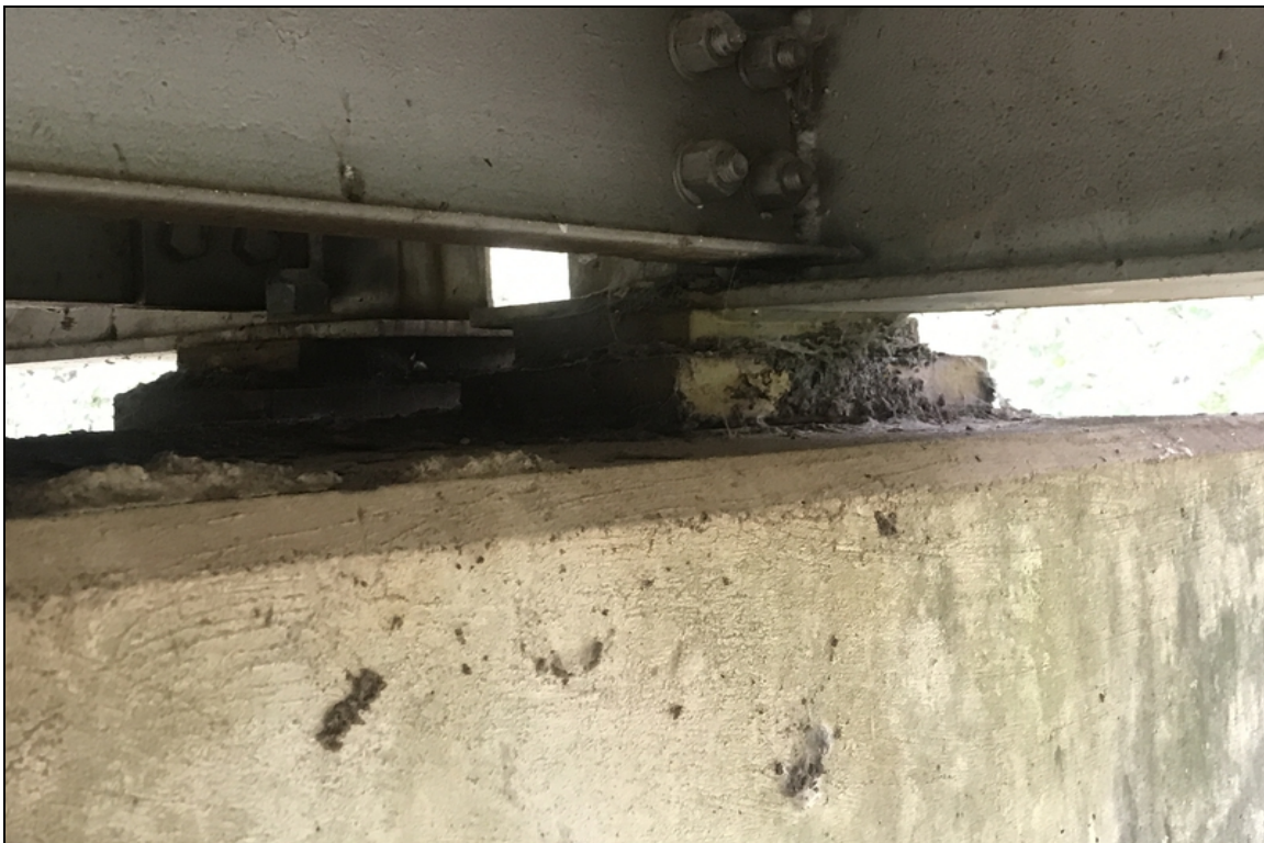
Bent 9 bearing 1 has flaking rust between bearing and plate.
