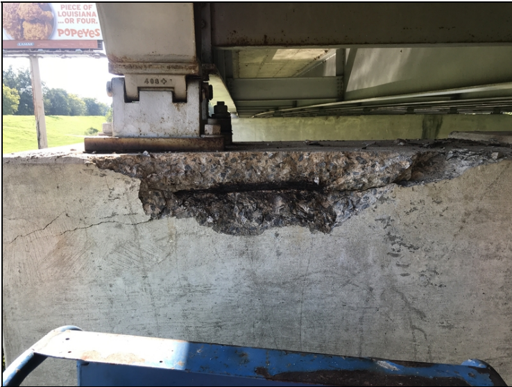
Bent 21 - Cap ahead side: Exposed rebar
