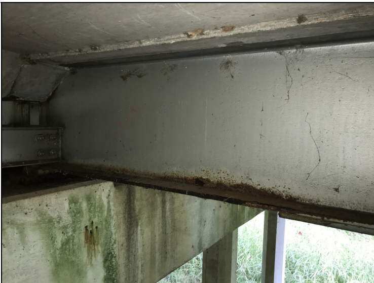
Span 9 Girder 3 right @ Bent 9: Corrosion
