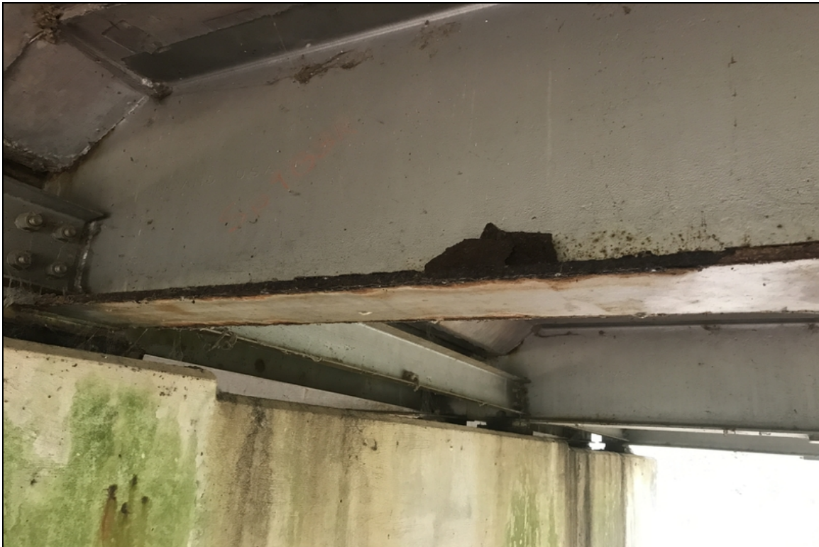
Span 9 girder 3 right has flaking rust.
