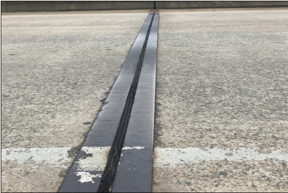
Bent 5 joint material is torn and leaking.
