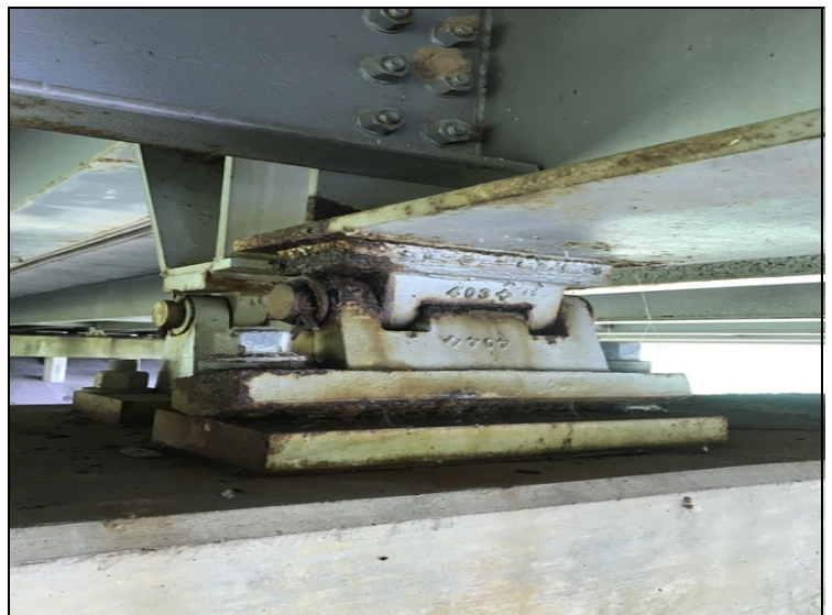
Bent 21 Back- Bearing 5 : Corrosion
