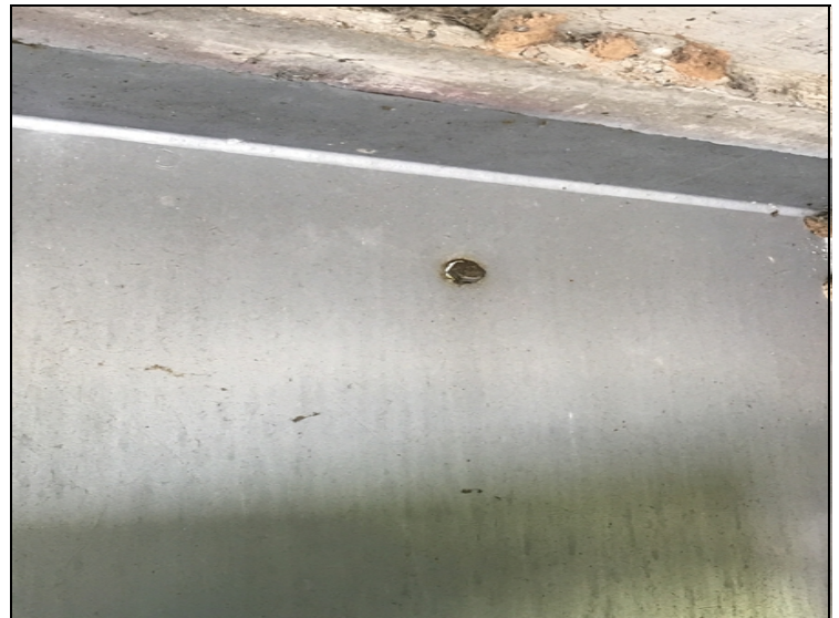
Span 19 - Girder 1 near Bent 20: Hole in web with loose bolt
