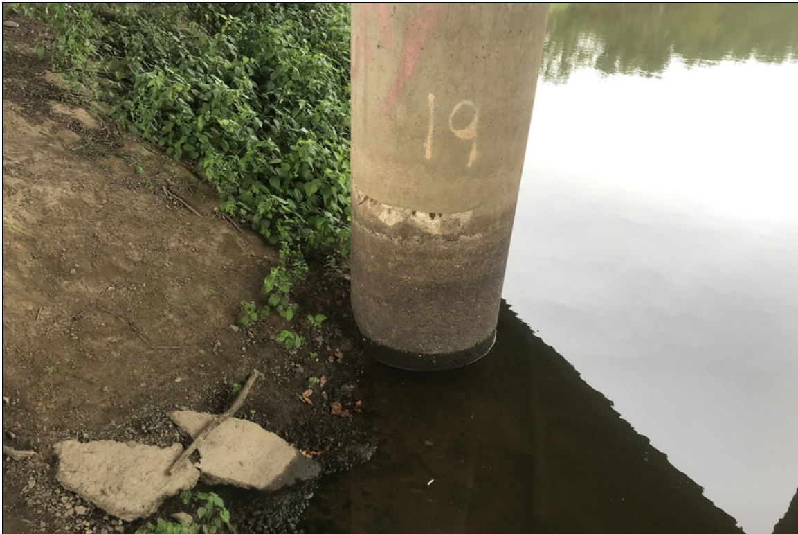
Bent 19 column 2 has spalling with exposed rebar.
