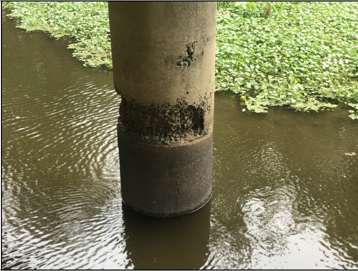
Bent 14 column 1 has spalling/ abrasion to lower 2' of column with exposed rebar
