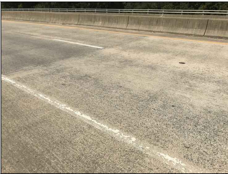
Deck - Span 19 right: Transverse cracking
