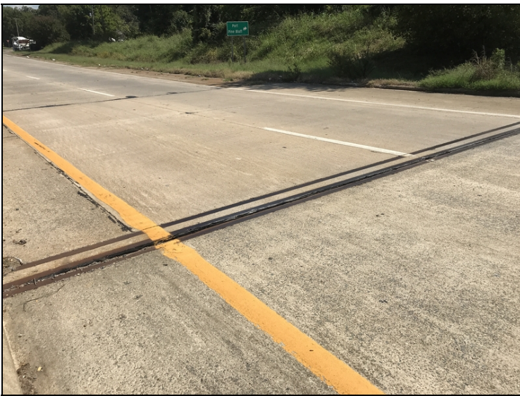
Joint - Bent 30 right: Backwall higher than deck
