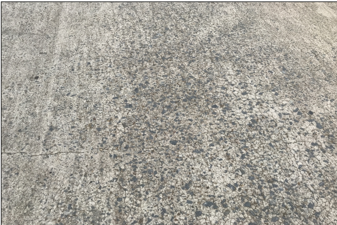
Deck span 11 map cracking.
