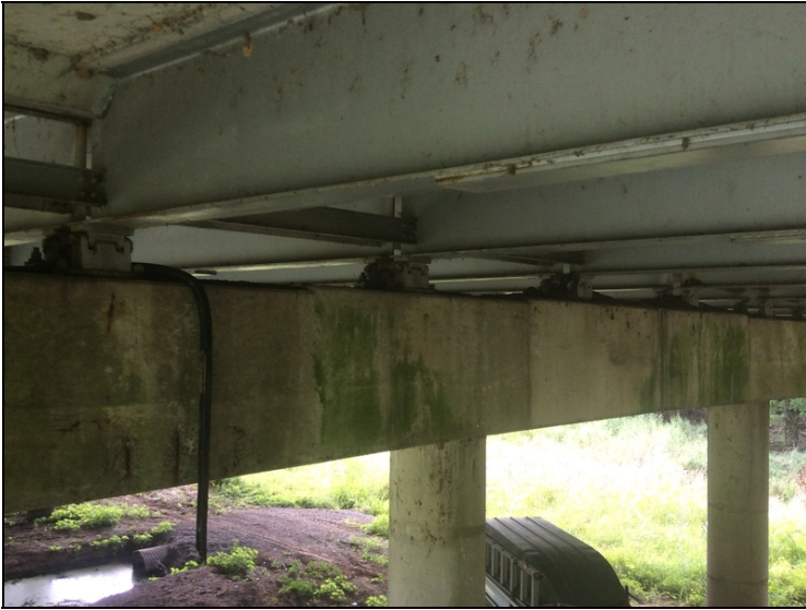
Bent 11 Joint material laying on cap with moisture and debris on cap
