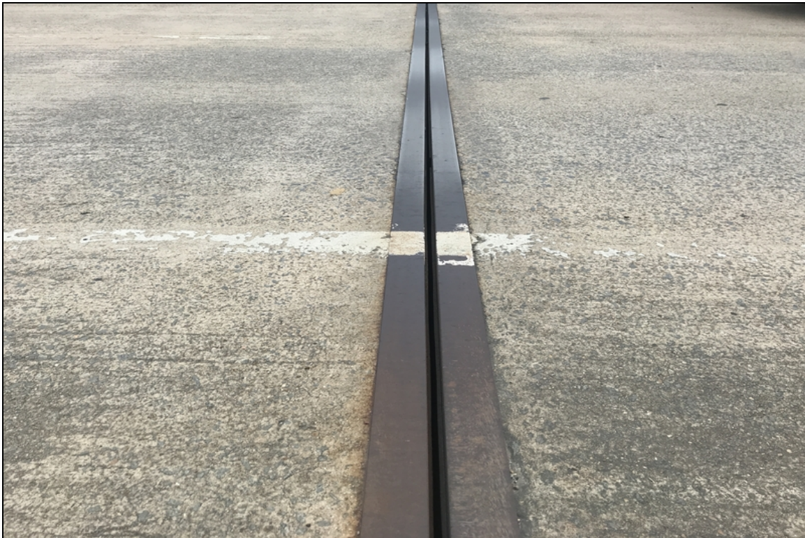
Bent 17 joint seal material missing.
