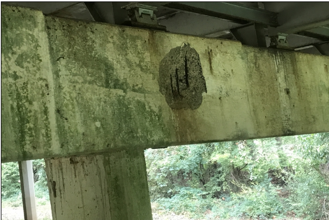
Bent 10 cap ahead has spalling with exposed rebar.
