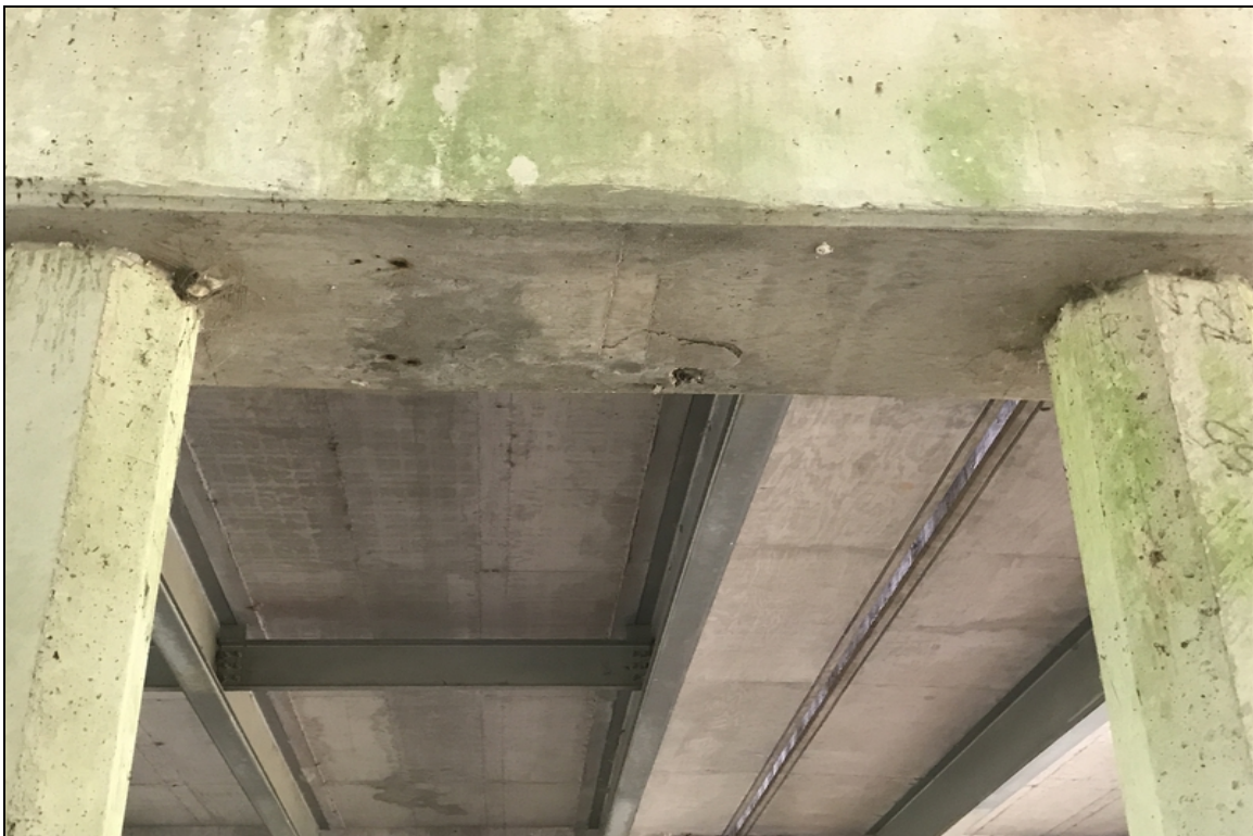
Bent 6 between piles 5 & 6 cap has small delam.
