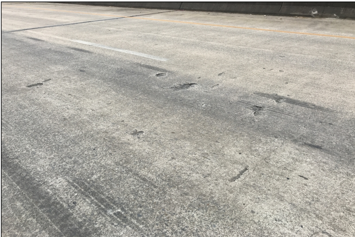
Span 4 north bound has small spall in deck.
