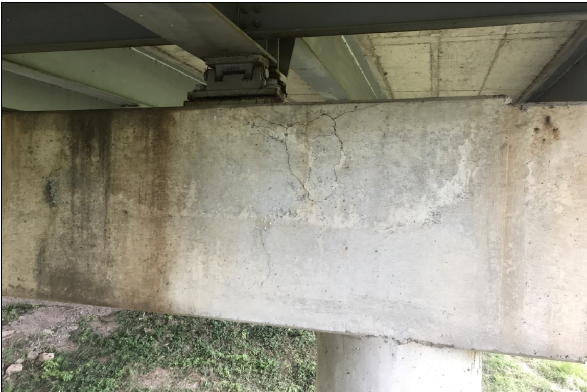
Bent 21 cap has cracking near girder 9.
