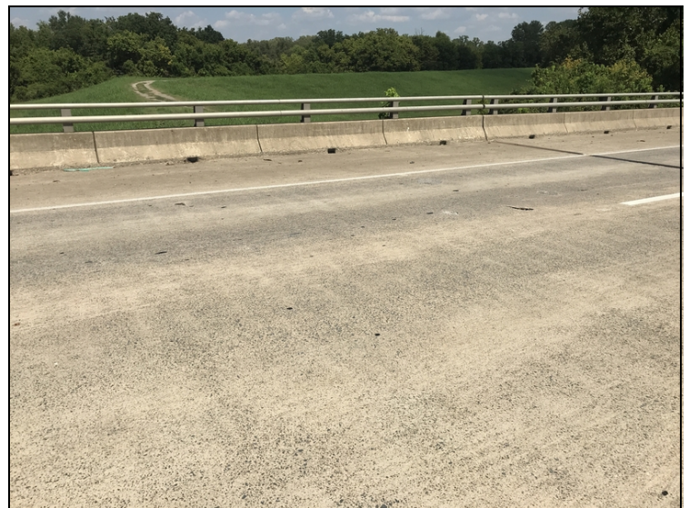
Deck - Span 22 left: Spalls
