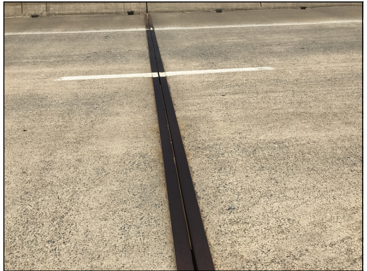
Joint - Bent 11 left: Material missing
