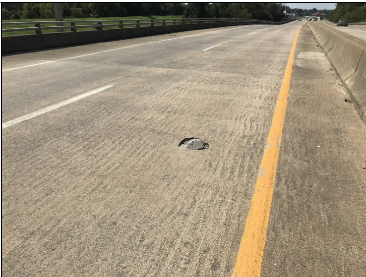
Deck - Span 20 right: Spall
