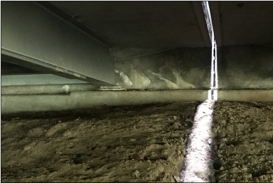
Bent 30 back wall has cracking with efflorescence.
