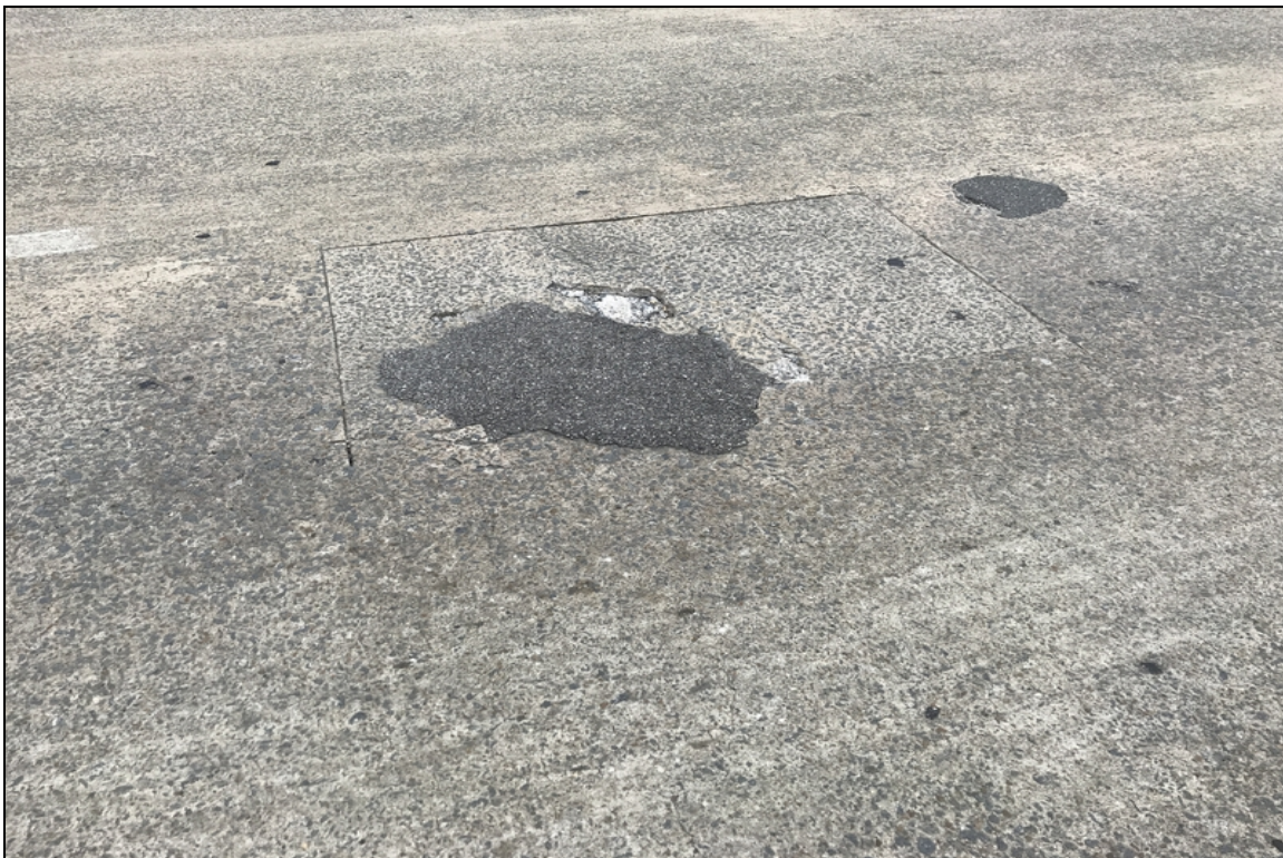
Deck span 25 north bound has spalling.
