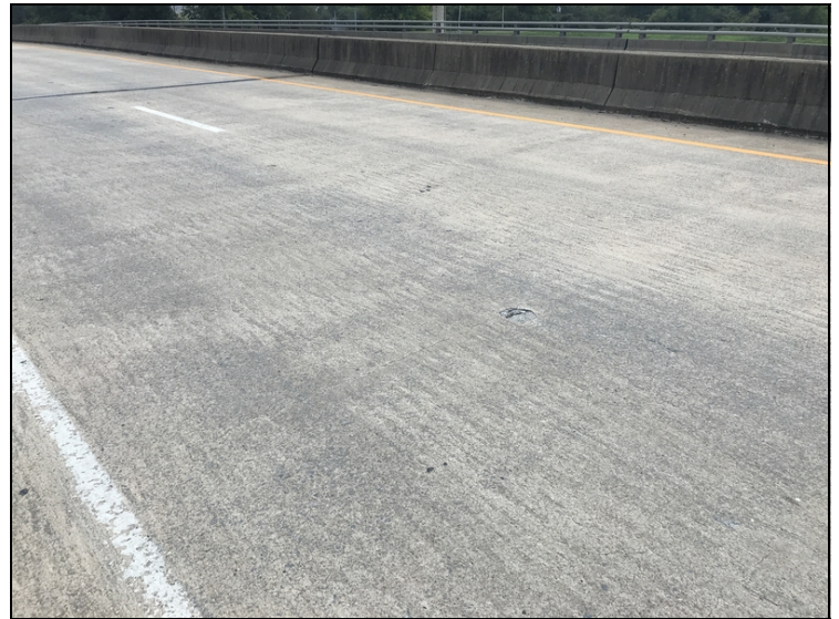
Deck - Span 17 left: Crack/spall
