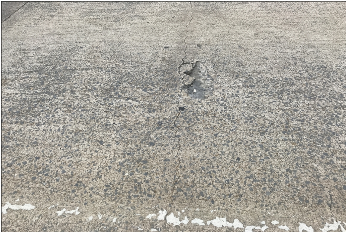
Deck span 19 south bound out side lane has 1' by 1' spall.
