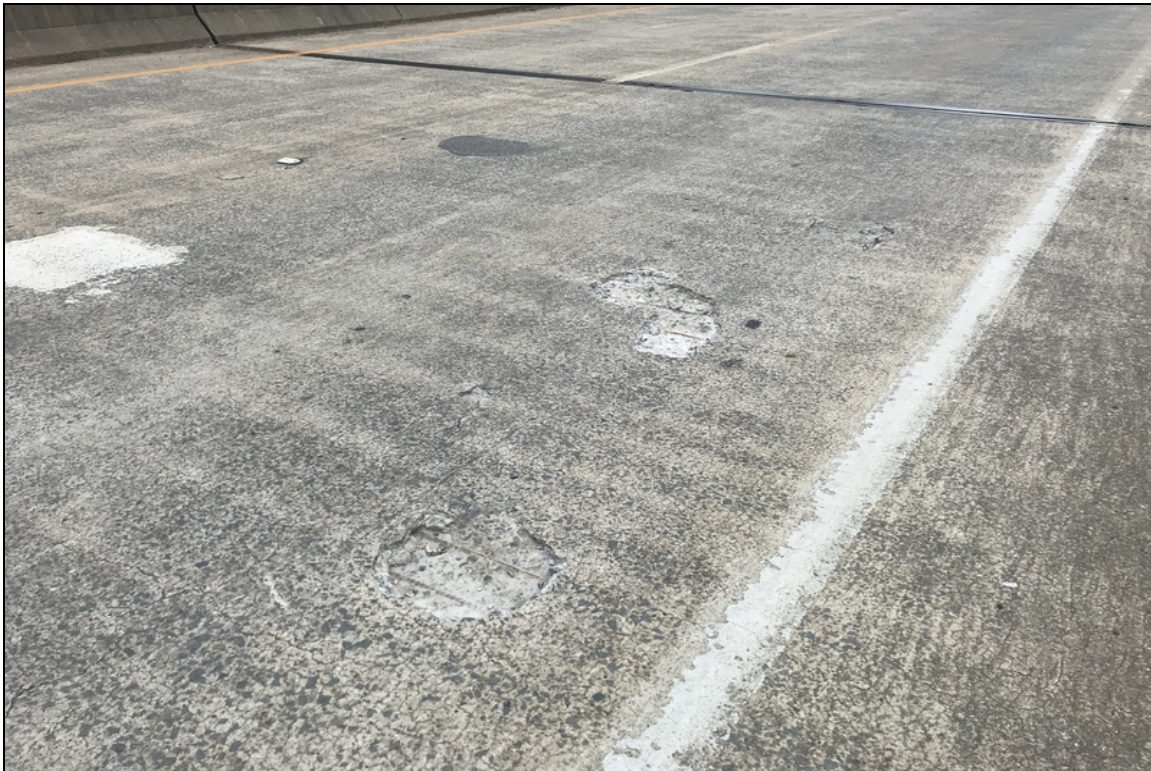
Deck span 27 right lane south bound has spalls with exposed rebar.
