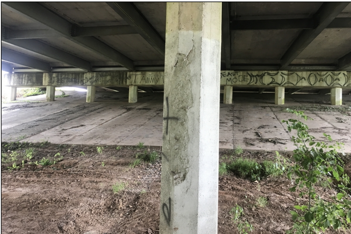
Bent 24 pile 5 has been repaired in past.
