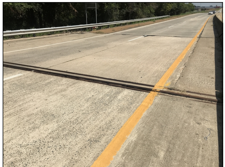
Joint - Bent 30 left: Backwall higher than deck
