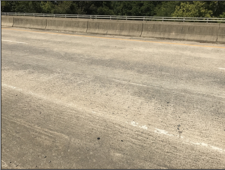
Deck - Span 11 right: Transverse cracking
