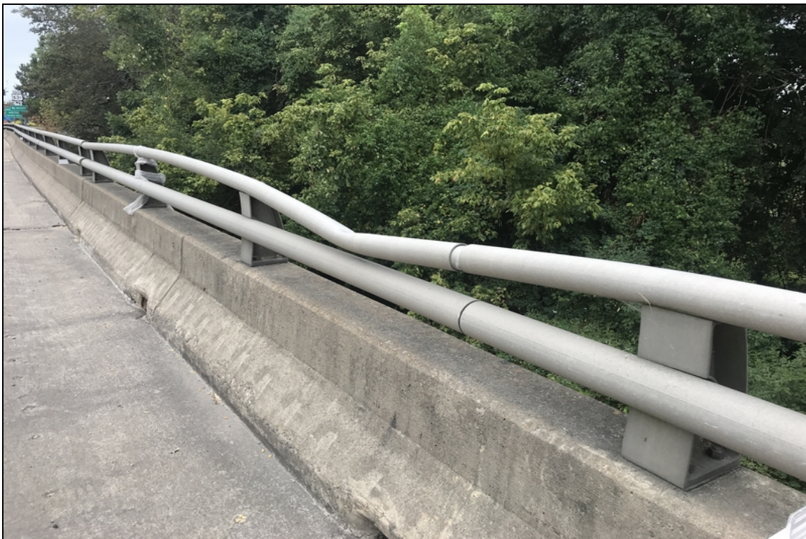
Span 5 north bound metal bridge rail damage.
