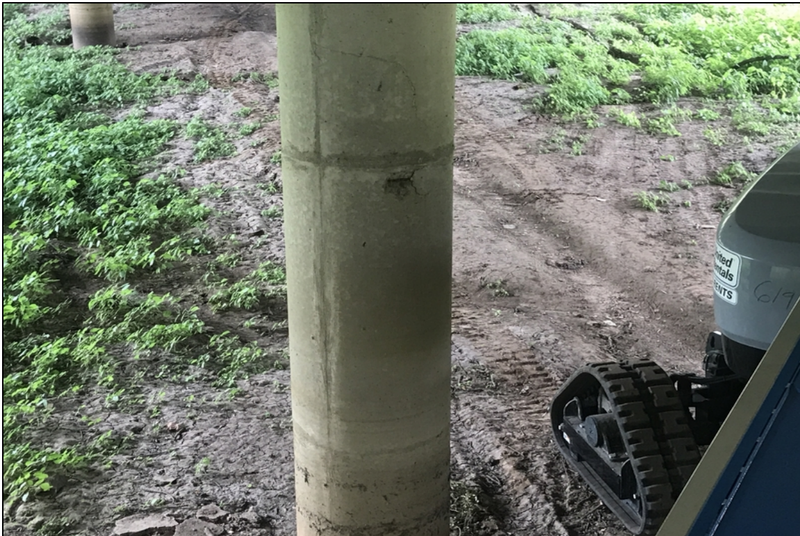
Bent 10 column 2 has spall with exposed rebar.
