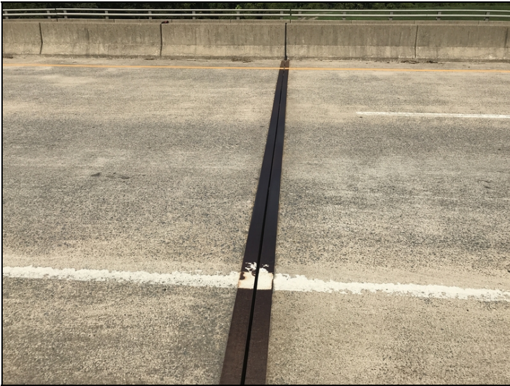
Joint - Bent 23 right: Material missing
