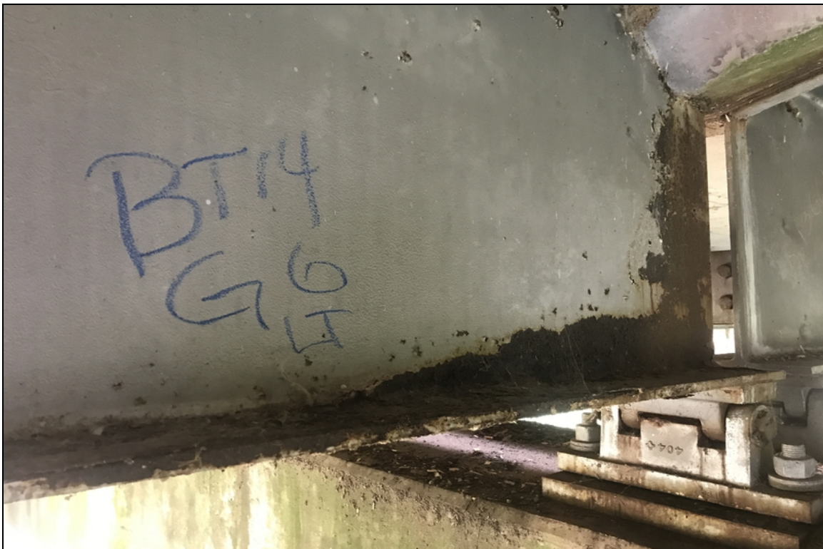
Bent 14 girder 6 left has corrosion with some flaking to web and lower flange.
