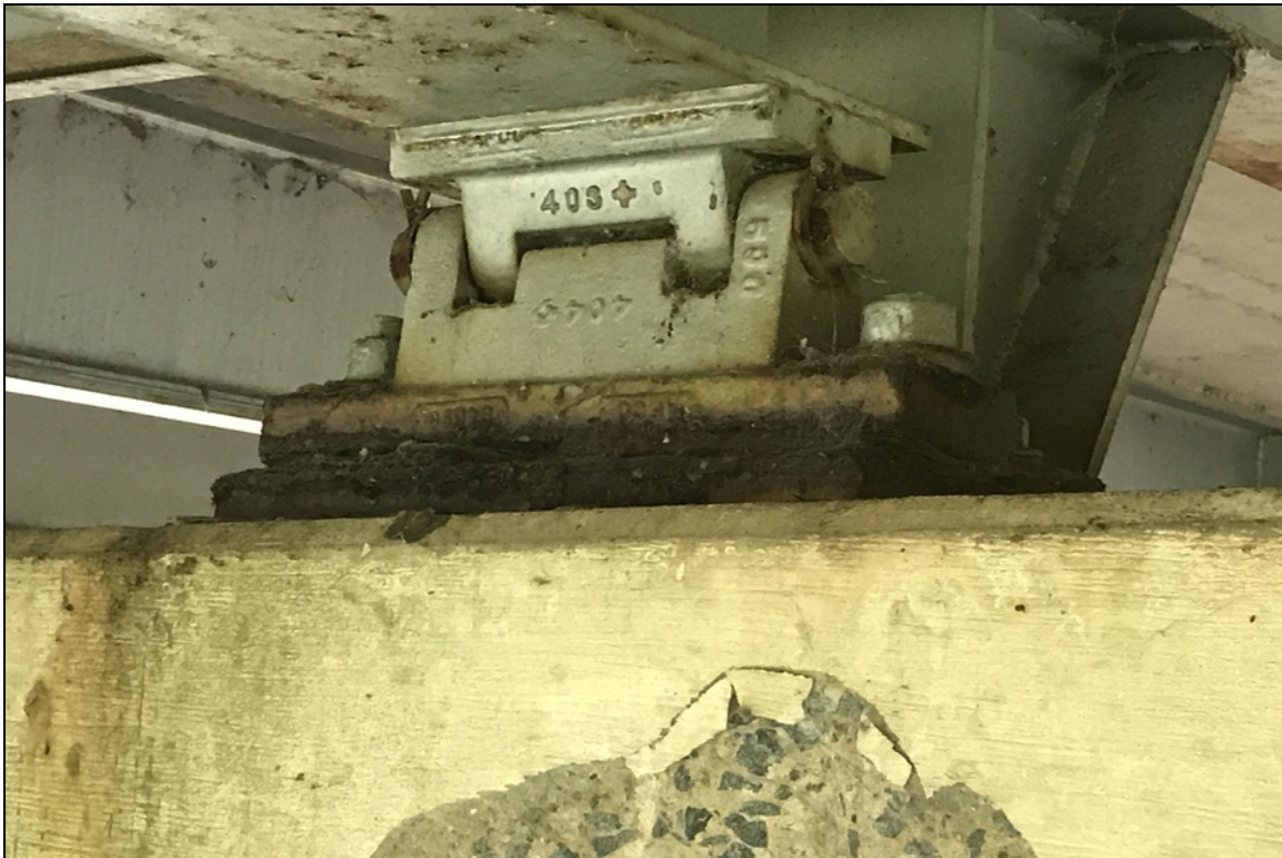
Bent 10 bearing4 ahead has heavy flaking rust. Common most bearing this bridge.
