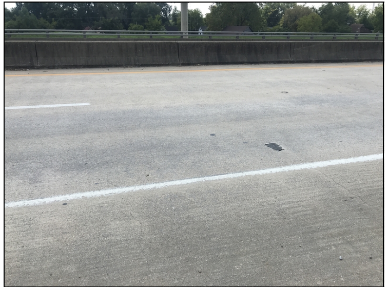
Deck - Span 19 left: Cracking/spall
