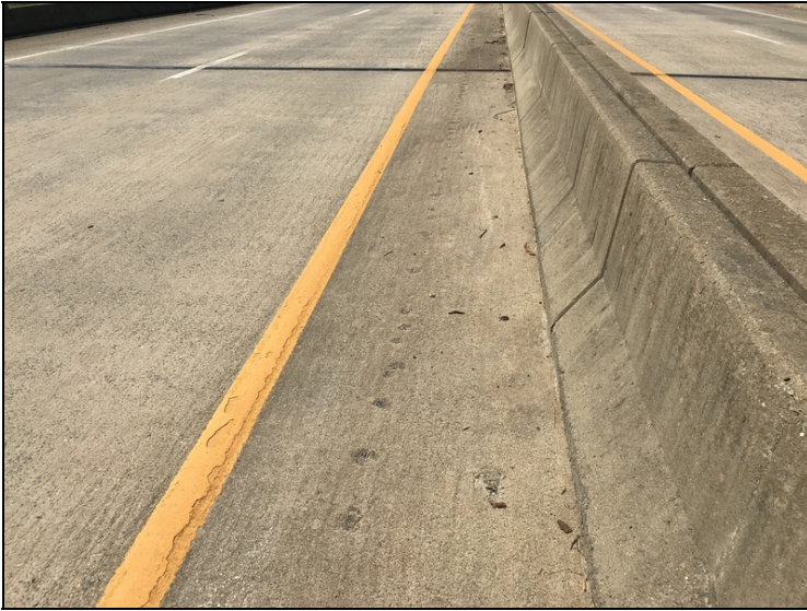
Deck - Span 21 right: Spalling over shear connectors
