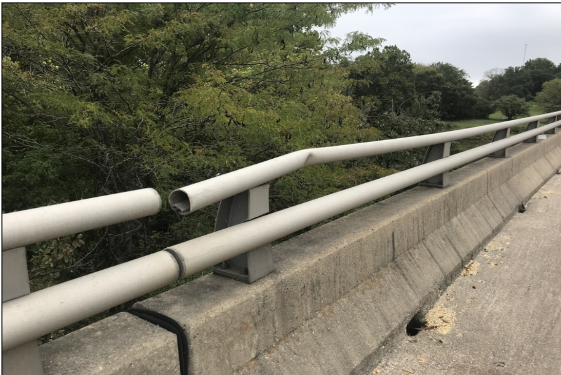
Span 13 metal rail damage north bound.
