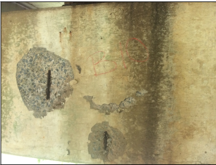
Bent 10 delam with exposed rebar over pile 2 and between piles 3-4
