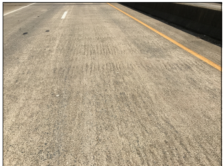
Deck - Span 11 left: Map cracking
