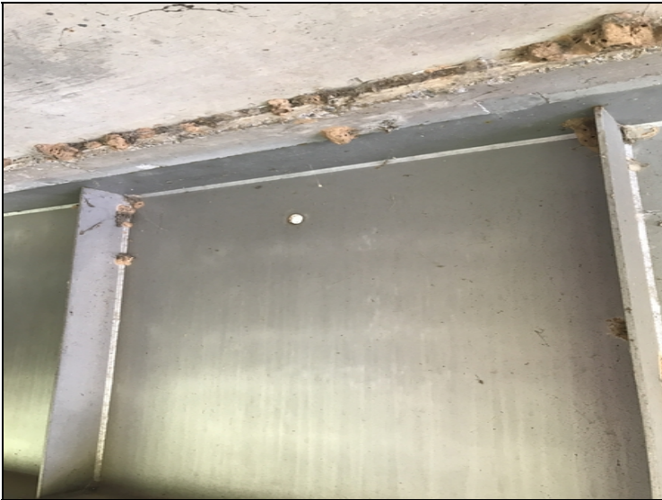
Span 19 - Girder 2 at Bent 20: Hole in web
