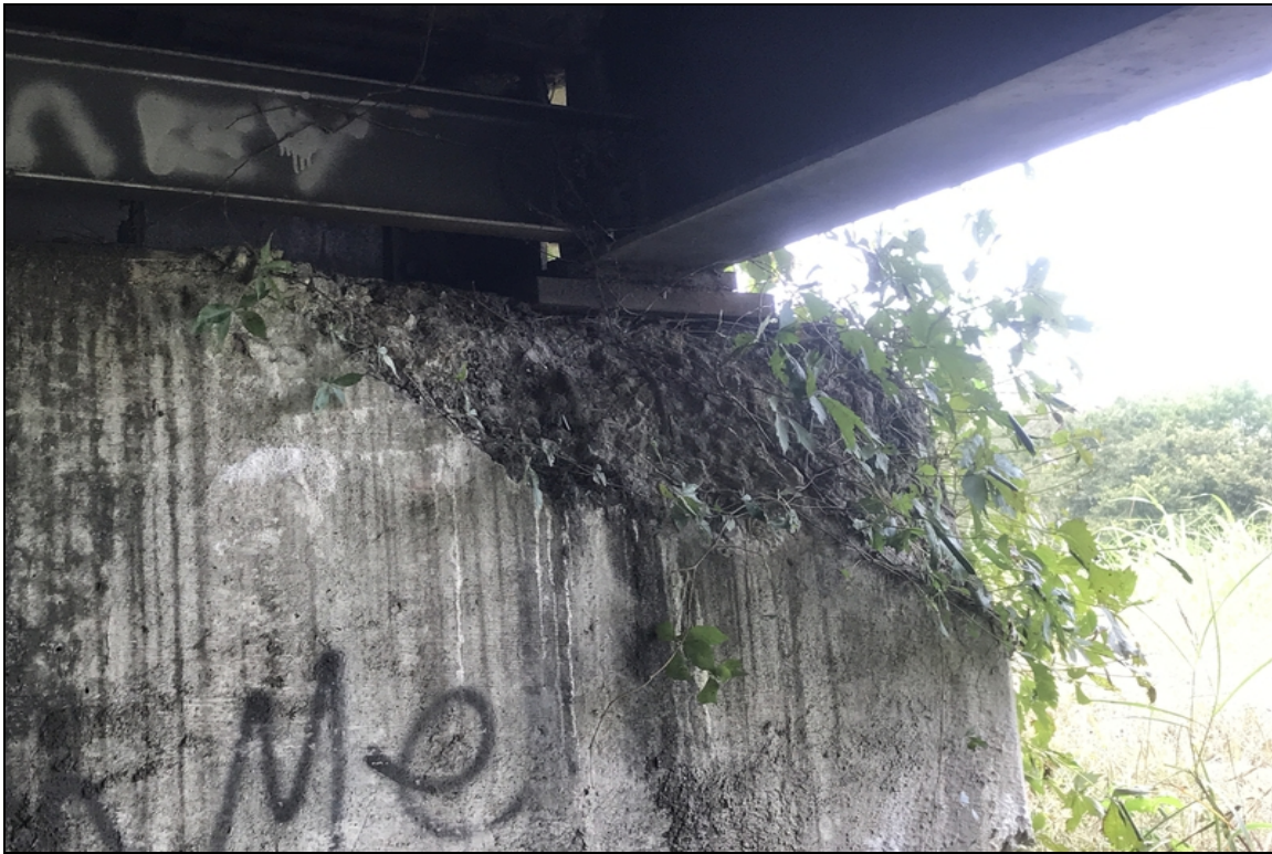
Bent 23 ahead face left end has large spall with exposed rebar encroaching on bearing area.
