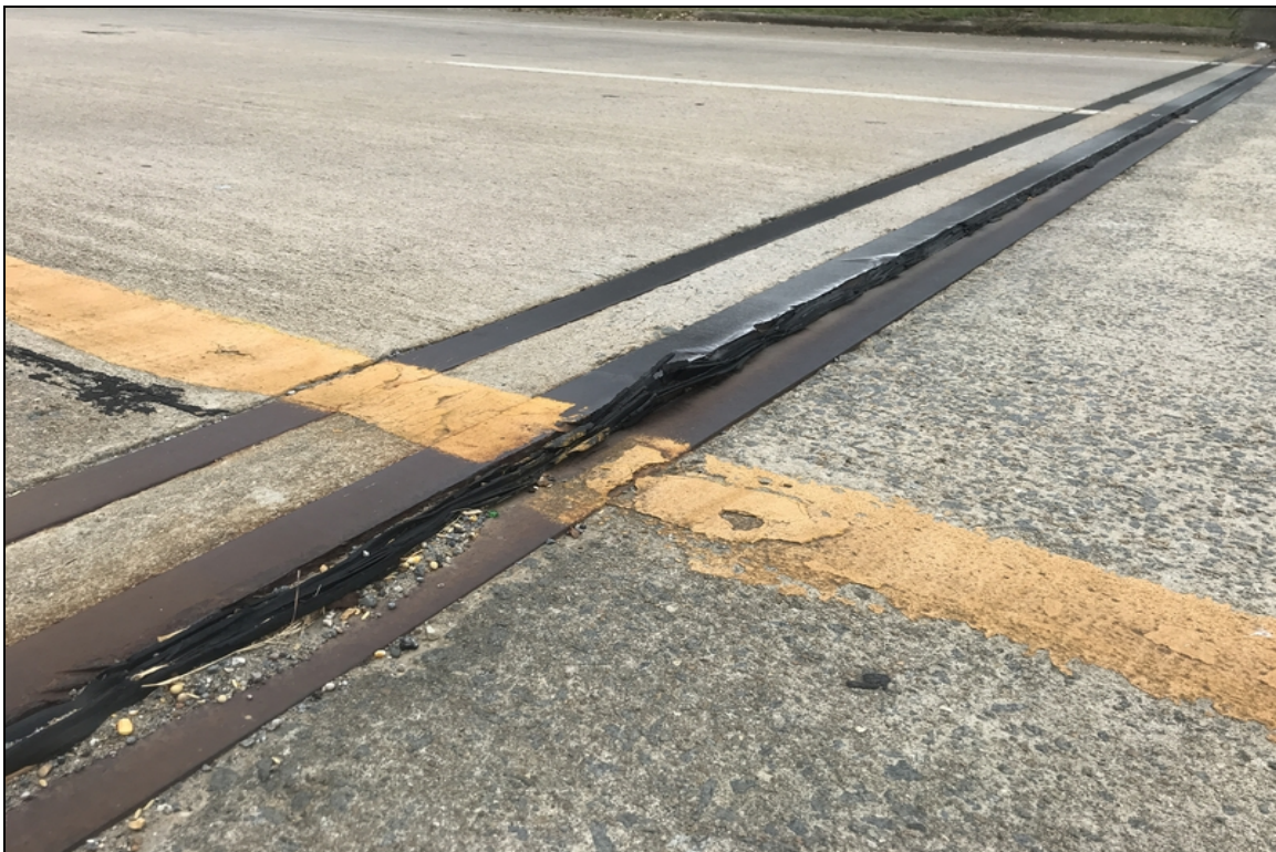
Back wall bent 30 south bound is higher than bridge deck
