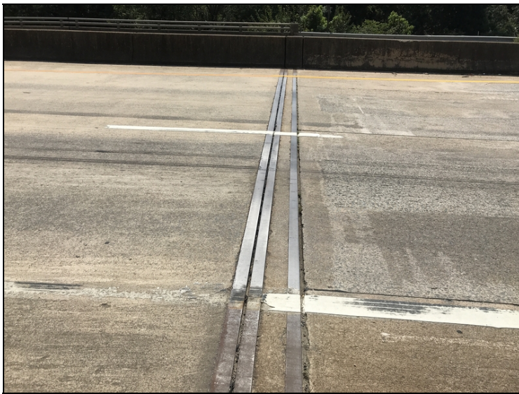
Joint - Bent 1 left: Damage
