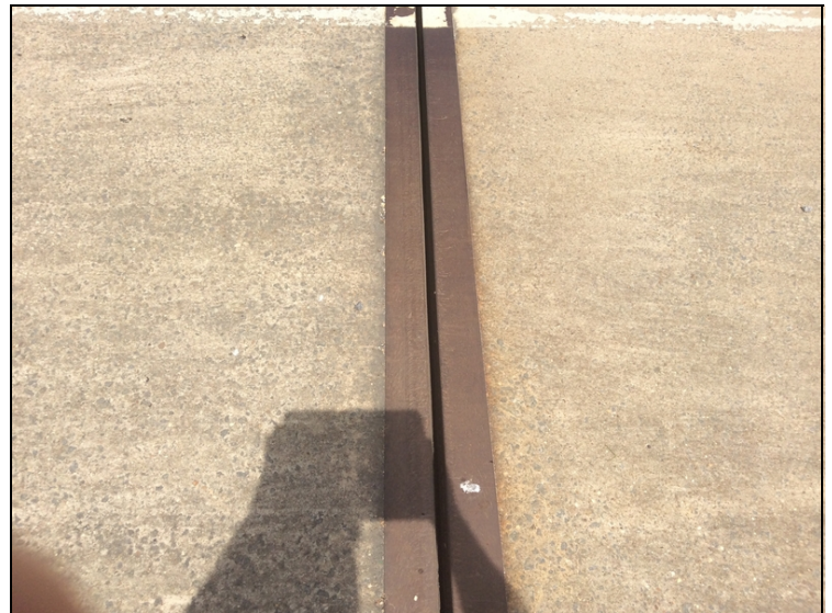
Span 23 expansion joint material missing in right hand lane and remaining joint torn and damaged.
