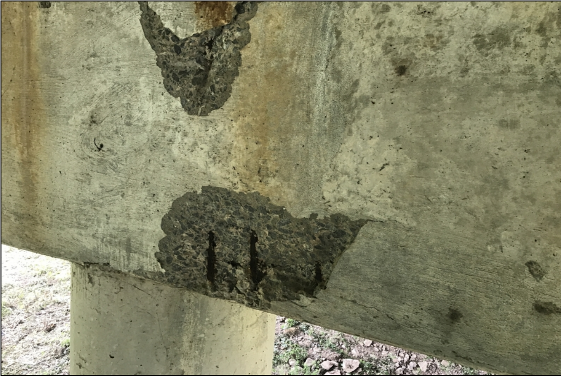
Bent 21 cap back spalls with exposed rebar.
