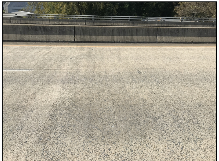
Deck - Span 5 left: Cracking/spalling
