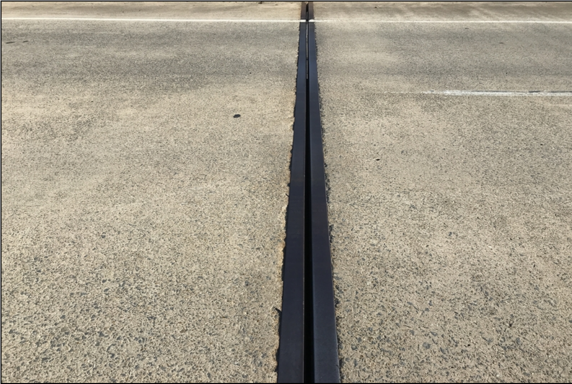
Joint - Bent 4 left: Material missing
