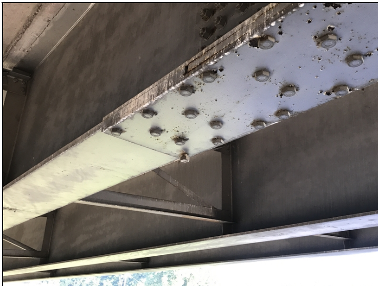
Span 4 girder 3 first splice plate near midspan has loose bolt.
