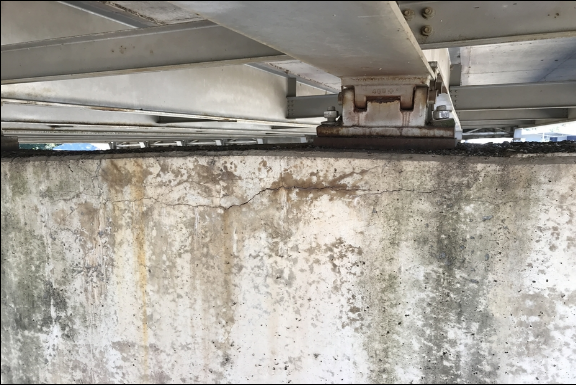
Cap - Bent 7 ahead left: Cracking
