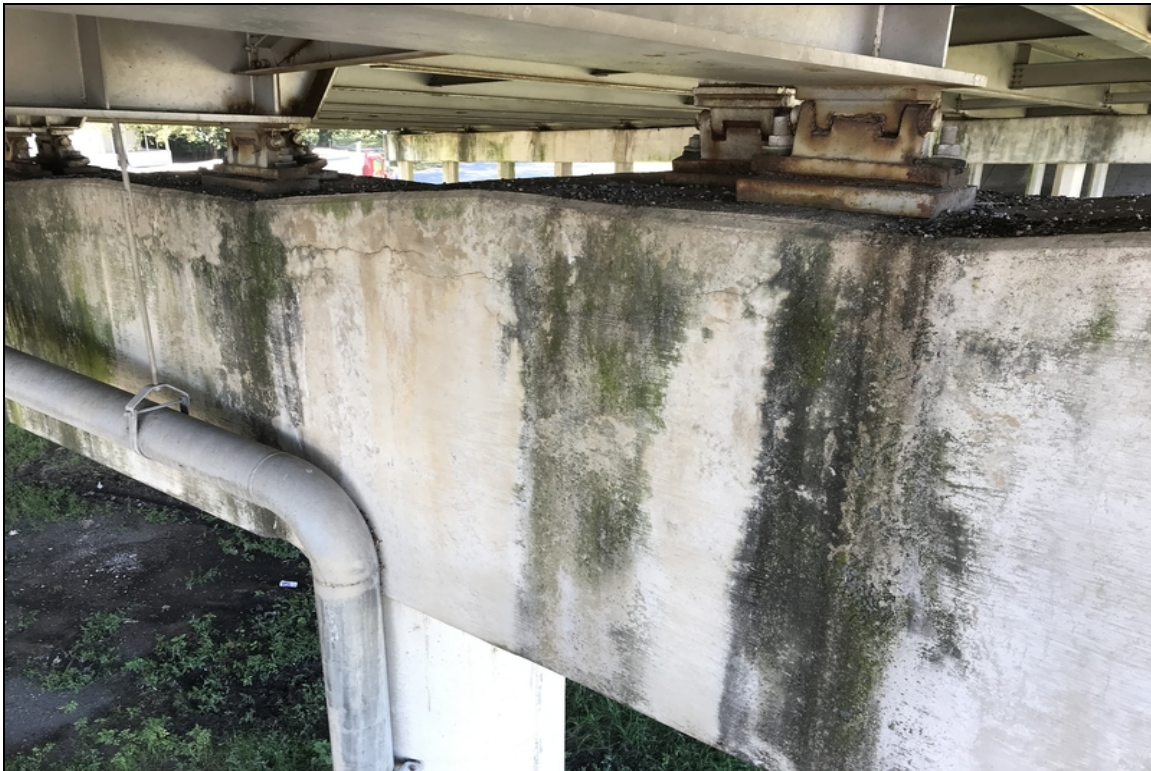
Cap - Bent 4 ahead: Cracking on top
