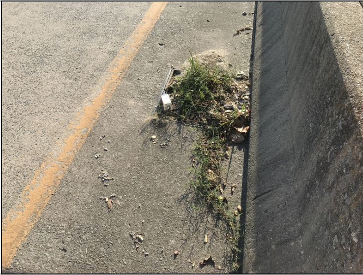
Drain - Span 4 left (inner gutterline): Stopped up
