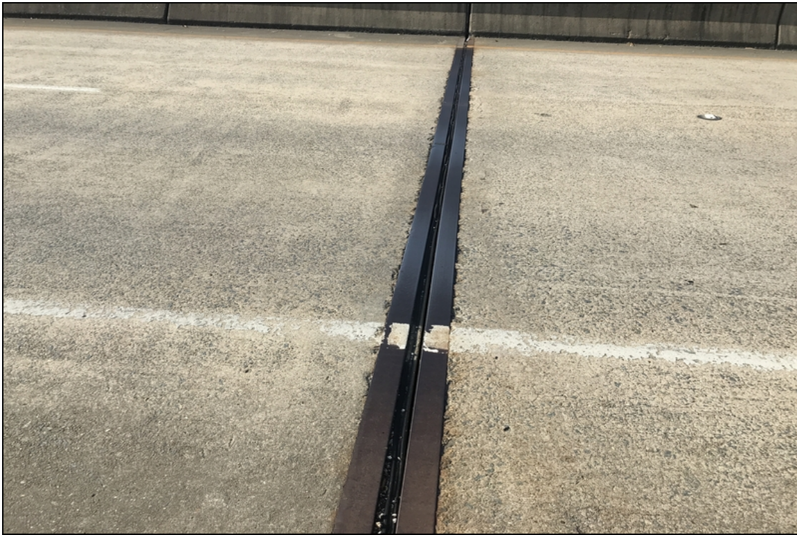
Joint - Bent 7 left: Loss of adhesion/adjacent deck Spalling ( deck Cracking)
