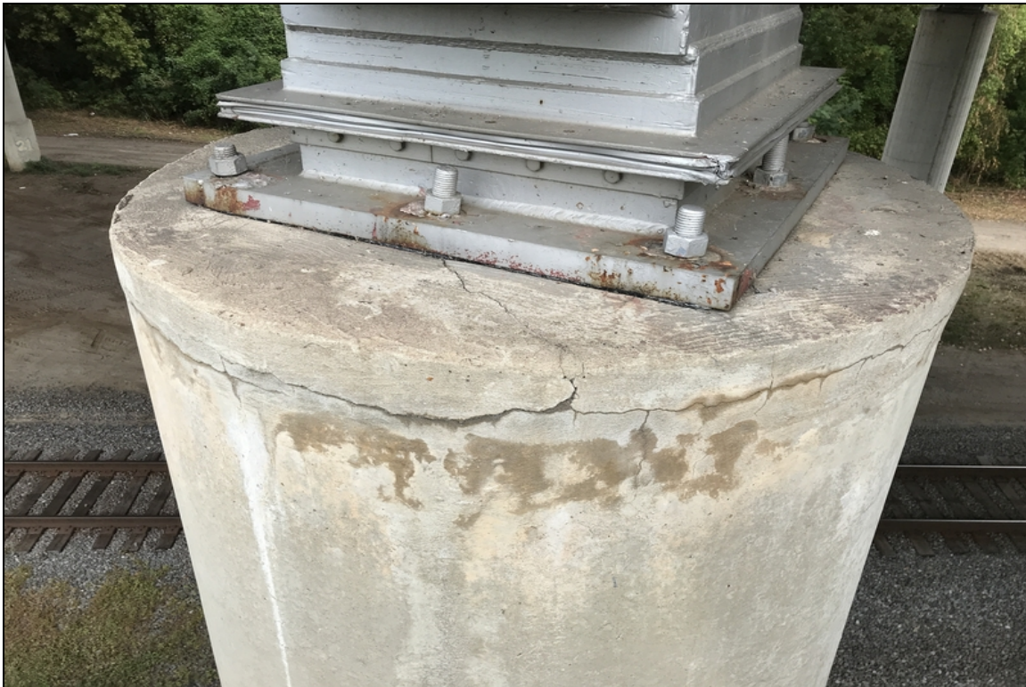
Bent 22 Column 2 right: Cracking
