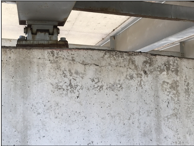
Bent 6 cap back has horizontal Crack under bearing 2. common bent 6 ahead at bearing 5,8 & 9.
