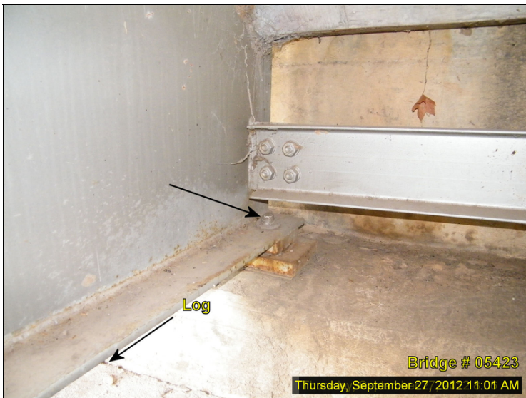
05423 09-27-2012 Bent 1 girder 11 - missing nut left side
