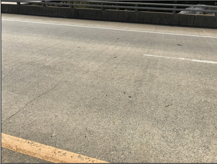
Deck - Span 5 right: Cracking
