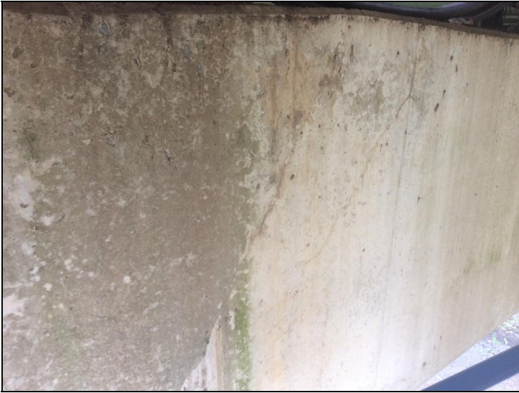
Bent 24 ahead has cracks with some light efflorescence. Common bent 25 back.
