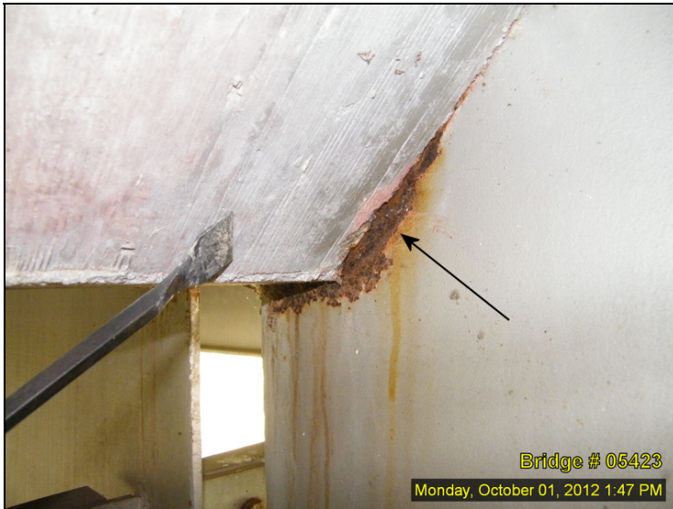
05423 09-27-2012 Bent 3 Girder 3 right side - some sec loss at the haunch area 10-15%
