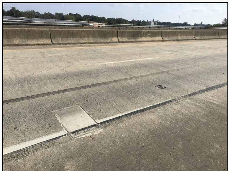
Deck - Span 14 right: Cracking/patch/rebar exposed
