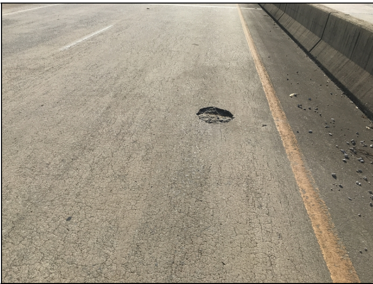
Deck - Span 6 left: Spall
