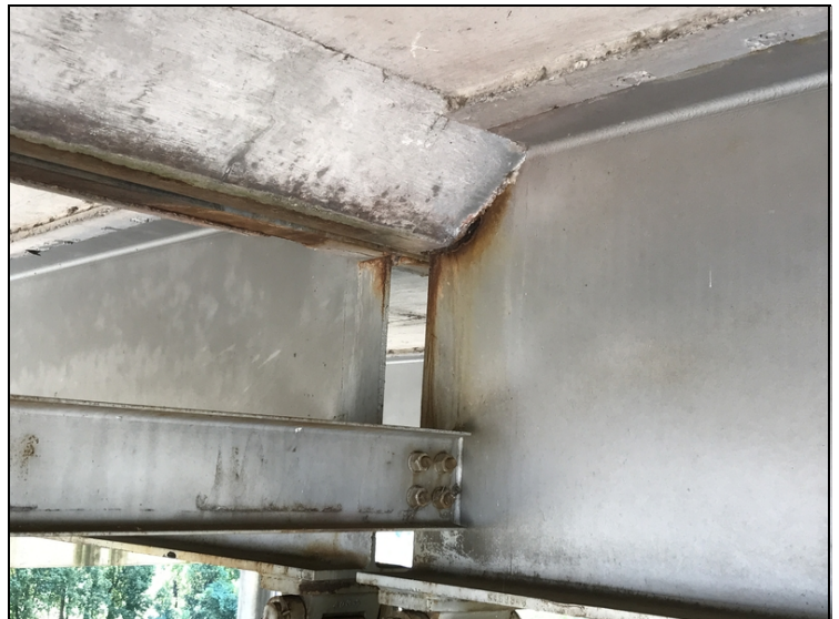
Span 16 Girder 2 left @ Bent 17: Corrosion @ haunch
