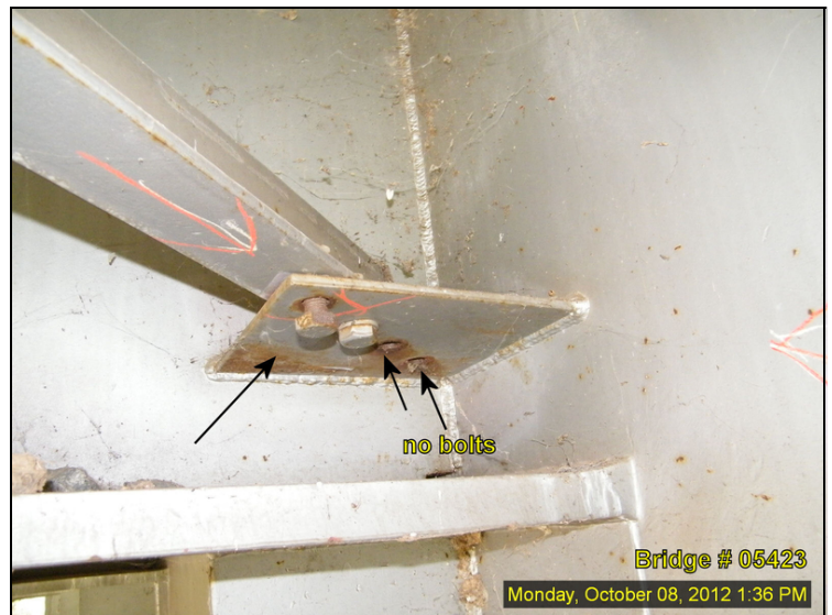
05423 09-27-2012 Bent 22 Cap - loose bolt at connection plate
