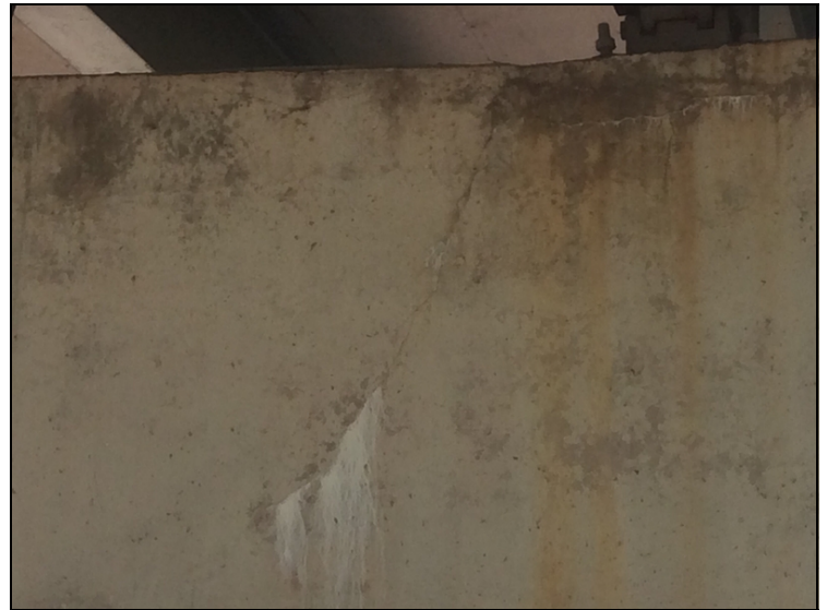
Bent 21 ahead , under beam 2 crack with efflorescence about 3 ft long
