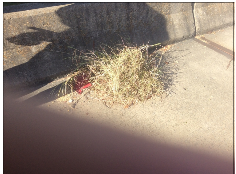
Drain opening near bent 4 right side completely full of debris with no drainage ability.
