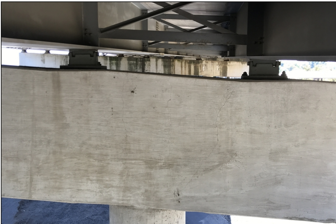
Cap - Bent 5 back: Cracking
