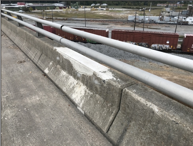
Railing – Span 18 left side: Post missing
