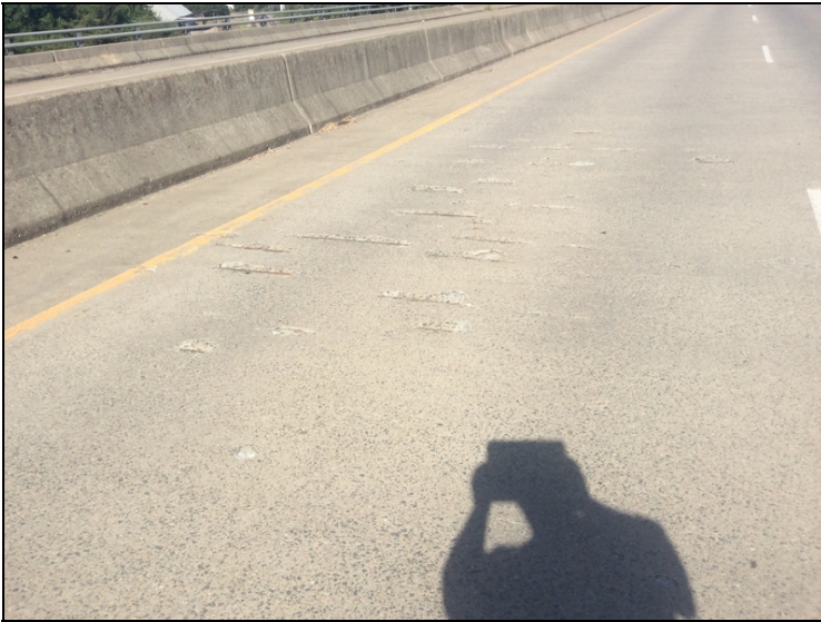
Span 14 north bound left lane spalls with exposed rebar.
