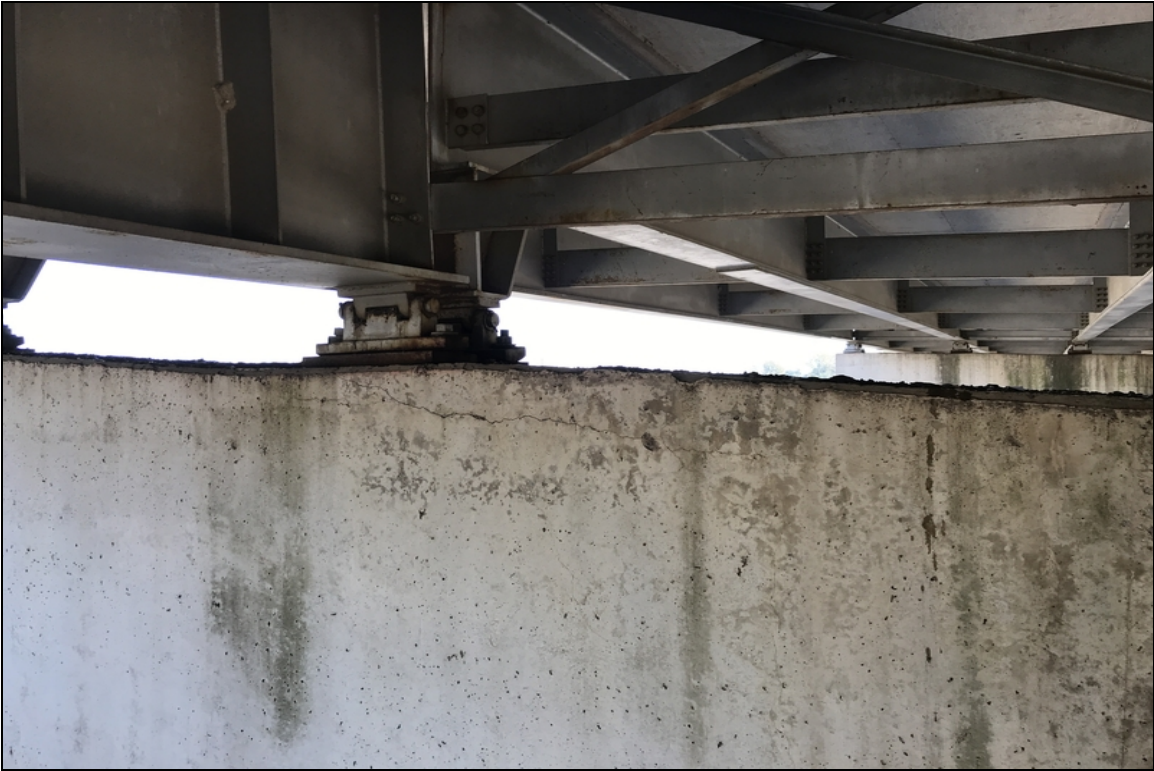
Cap - Bent 6 back left: Cracking
