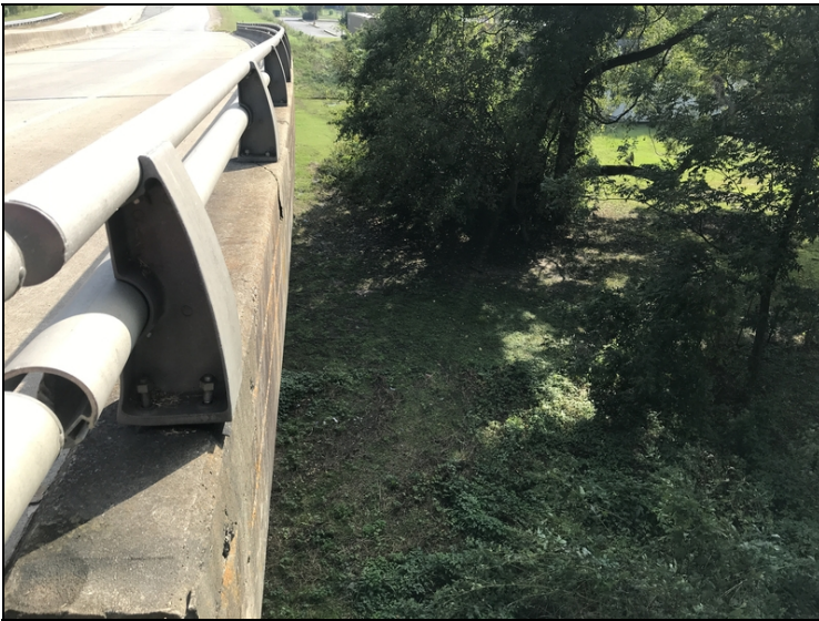
Railing - Span 26 right: Damage
