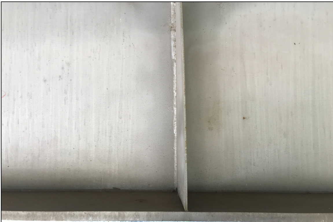
Cap - Bent 15 back @ Girder 6: Stiffener twisted to right at bottom
