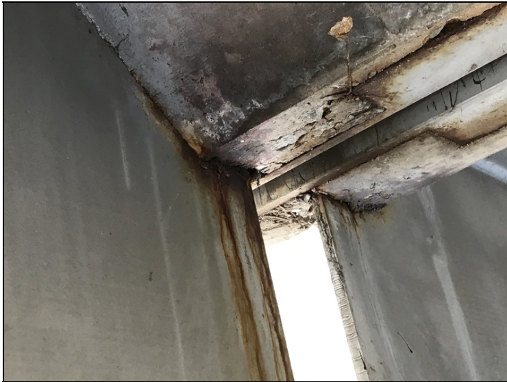
Typical haunch area with rust forming. Common throughout bridge.
