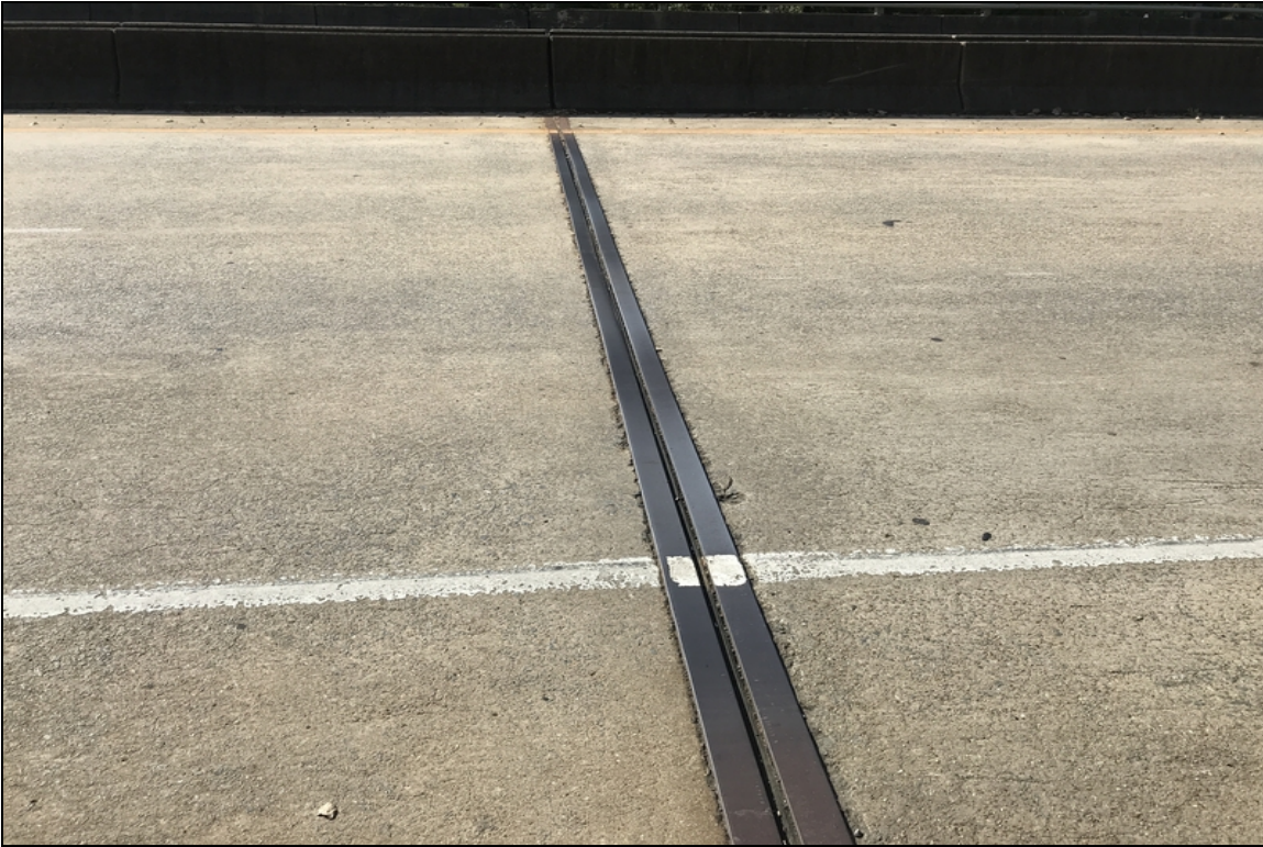
Joint - Bent 26 left: Adjacent deck spalling
