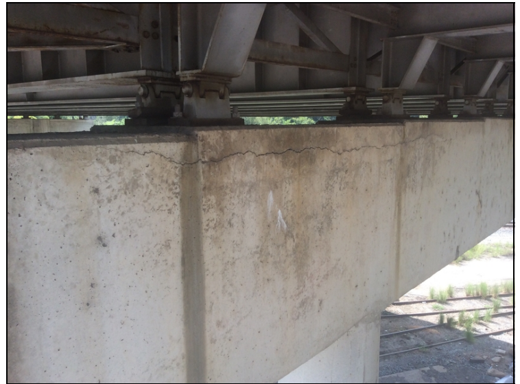
Bent 12 back crack in cap under beams 2-3
