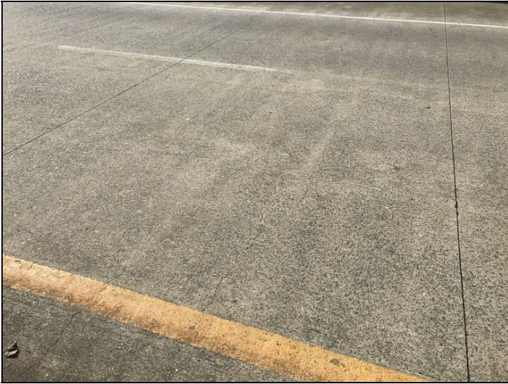
Deck @ Bent 23 right: Cracking along integral cap
