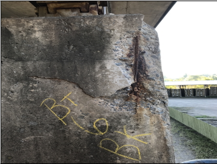
Bent 6 cap back has spalls with exposed rebar.
