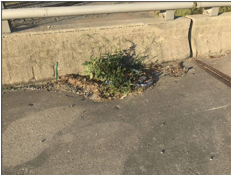
Span 10 south bound lanes drain opening completely stopped up with debris. Common several drains this bridge.
