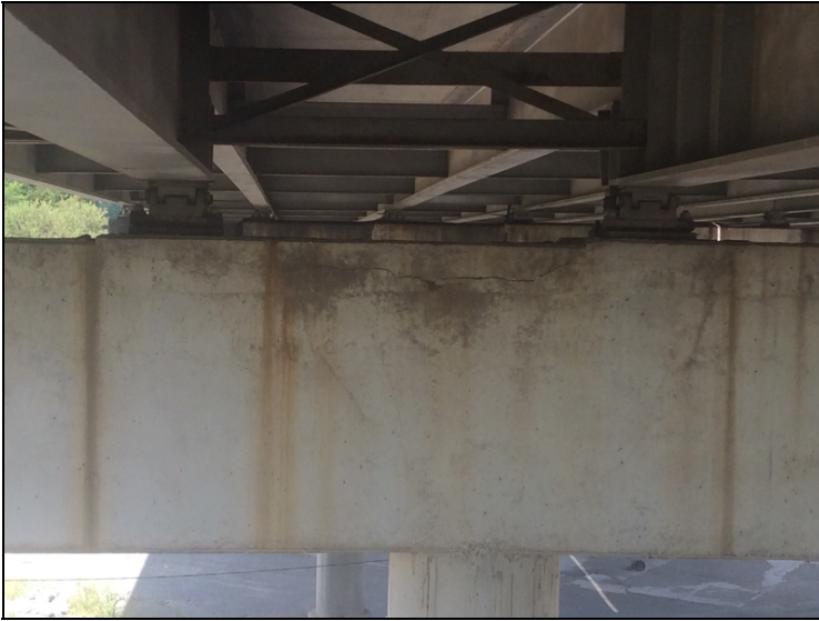
Bent 12 cap ahead Delams. under beam 2 and beams 8,9 , ends of cap
