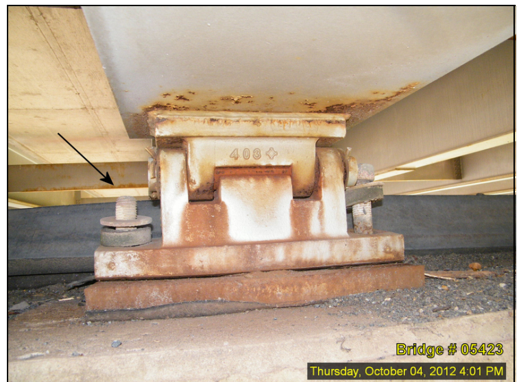
05423 09-27-2012 Bent 16 Girder 3 Bearing 3 - nut missing
