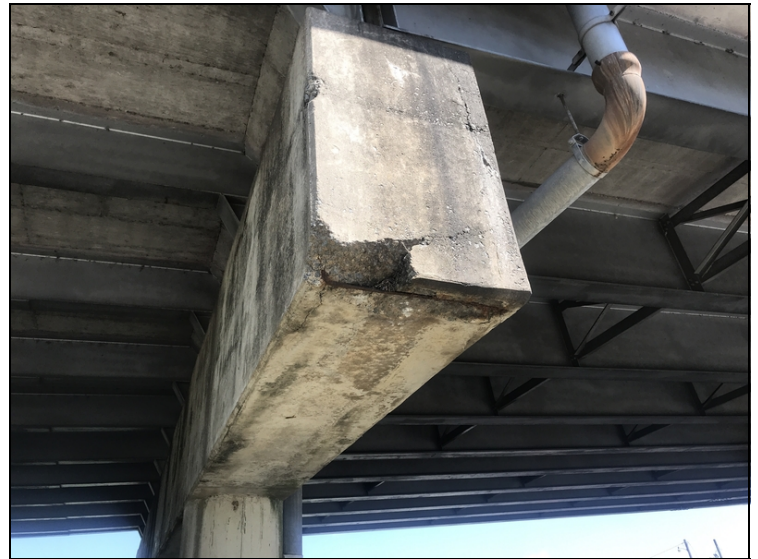
Bent 4 cap right side has spall with exposed rebar.
