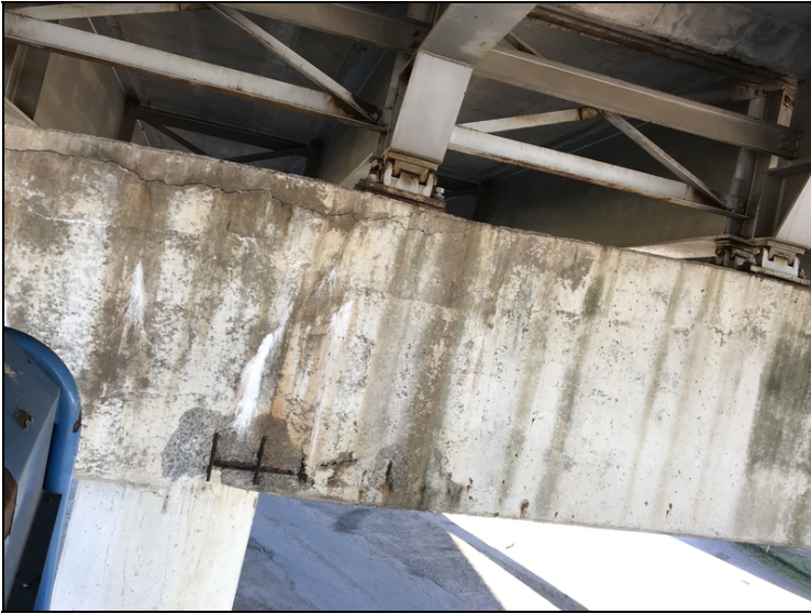
Bent 6 ahead has spalls with exposed rebar, cracking and cracking with efflorescence.
