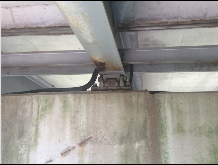
Bent 19 has some of the joint material missing, laying on cap from center line right. Common bent 18 left of center line.
