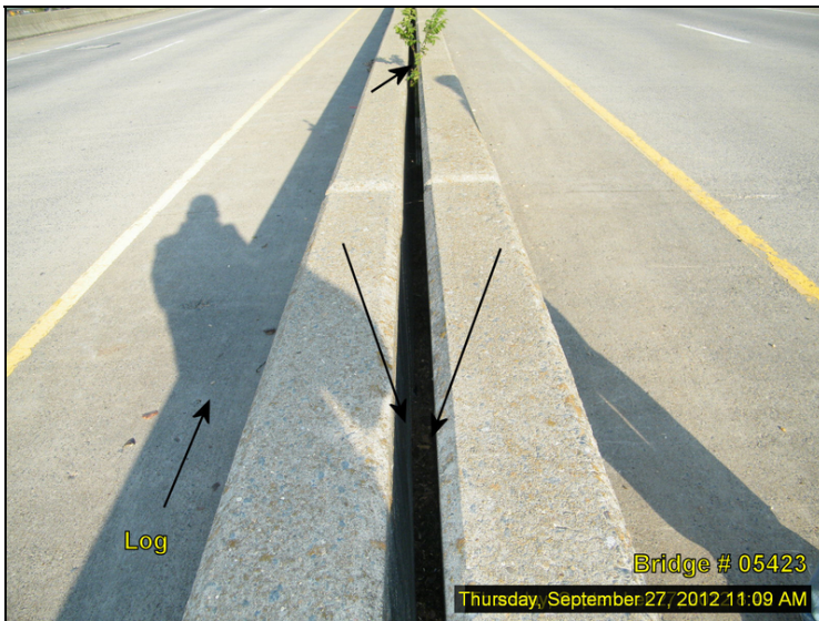
05423 09-27-2012 Bent 15 - center walls - debris on top of Bent 15 Cap
