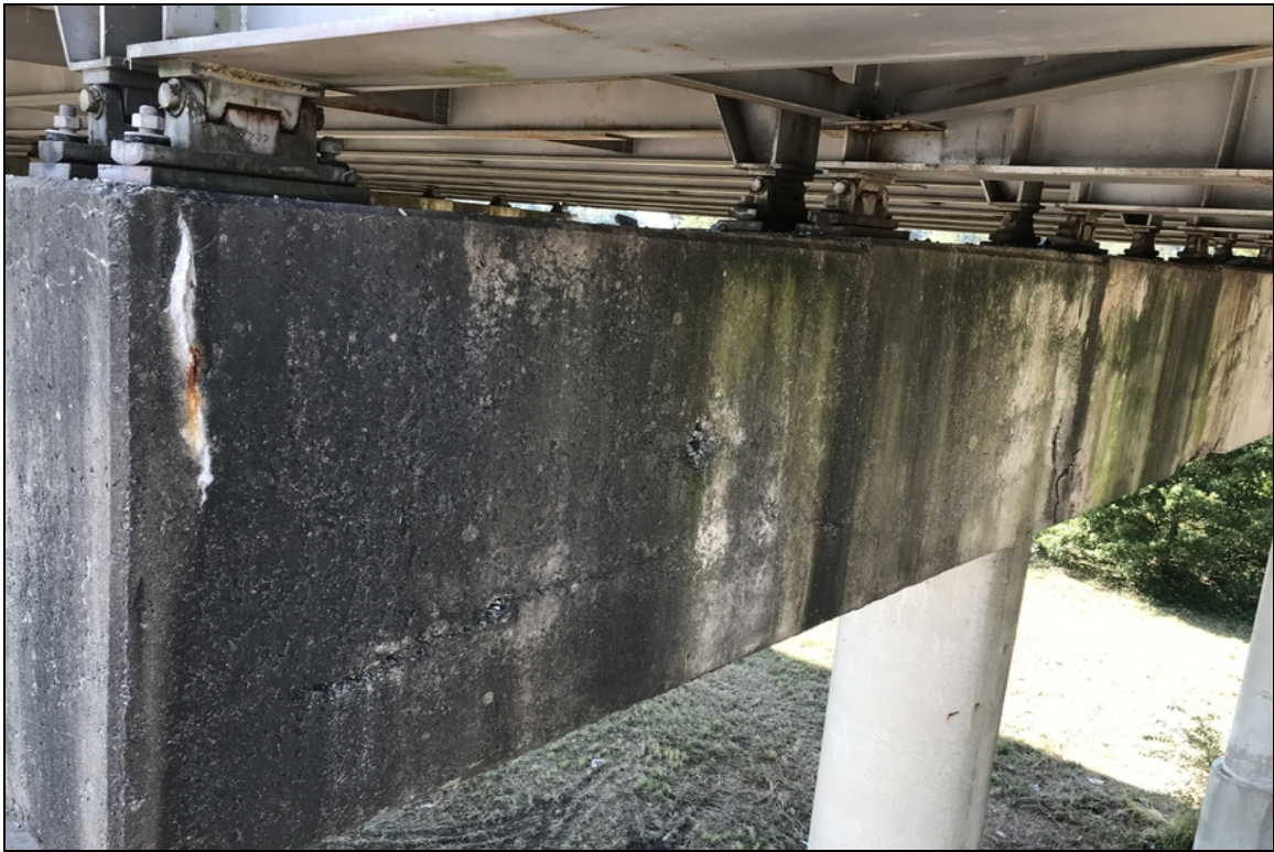
Cap - Bent 16 back left: Efflorescence/rebar exposed
