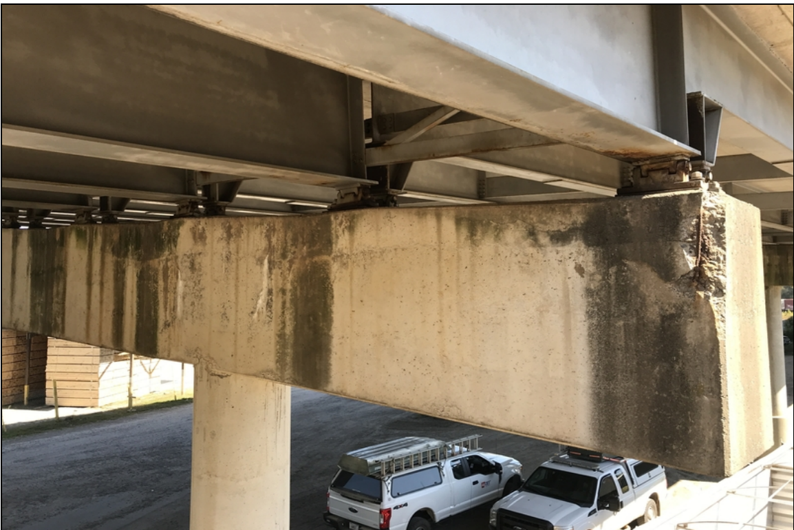
Cap - Bent 6 back right: Rebar exposed/efflorescence
