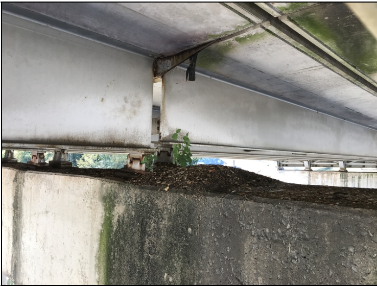
Cap - Bent 7 @ centerline: Debris build-up
