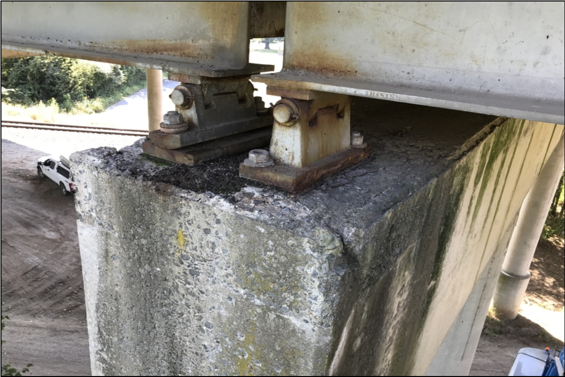
Cap - Bent 20 top face @ Bearings 1: Abrasive wear
