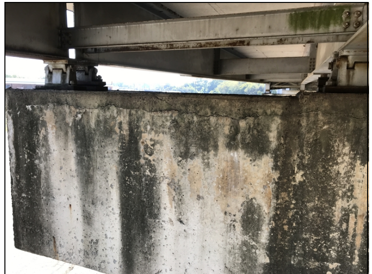
Bent 11 cap left side has large cracks from girder 1 -3.
