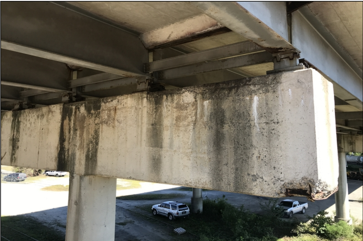
Cap - Bent 9 back right: Rebar exposed/efflorescence
