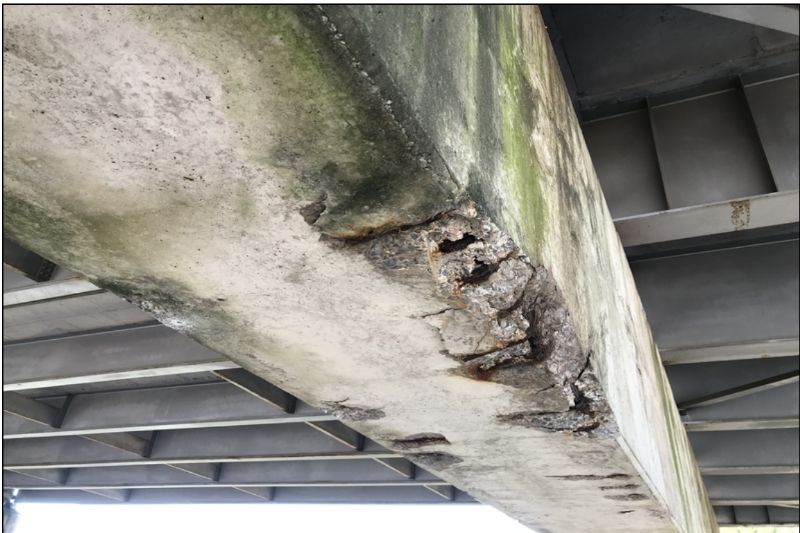
Cap - Bent 16 bottom face: Rebar exposed
