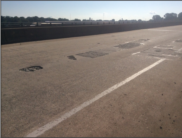
Span 9 deck has large spalls with some rebar exposed, asphalt patches and concrete patched areas. Approx 72'
