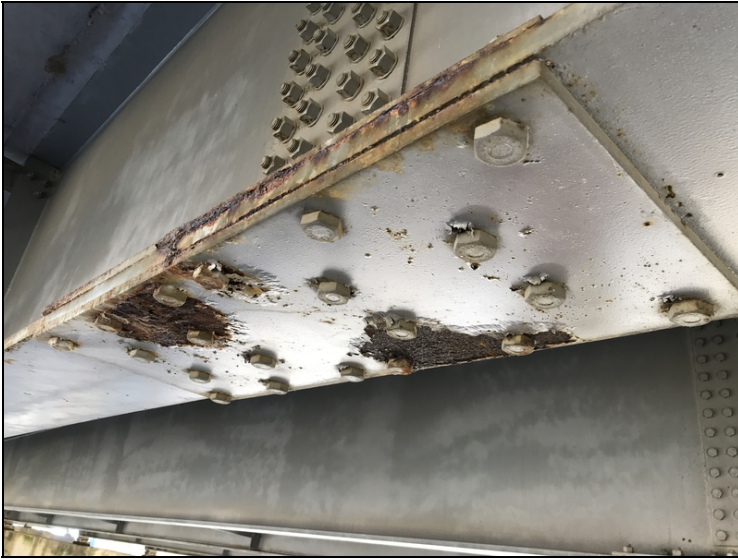
Span 5 Girder 5 @ splice: Corrosion
