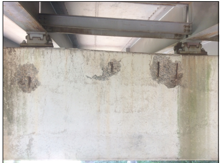
Bent 20 ahead about 5 ft of exposed rebar on cap
