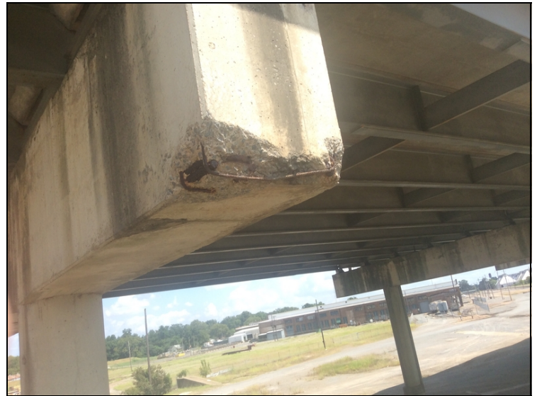
Large spall with exposed rebar on right side of cap 9 . Common on bents 4,5&6 all on the right sides .
