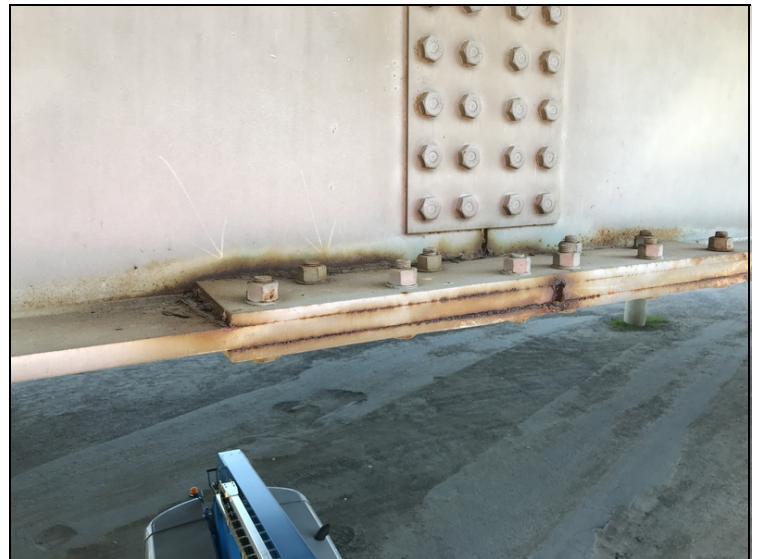
Span 5 Girder 10 right @ Splice: Corrosion
