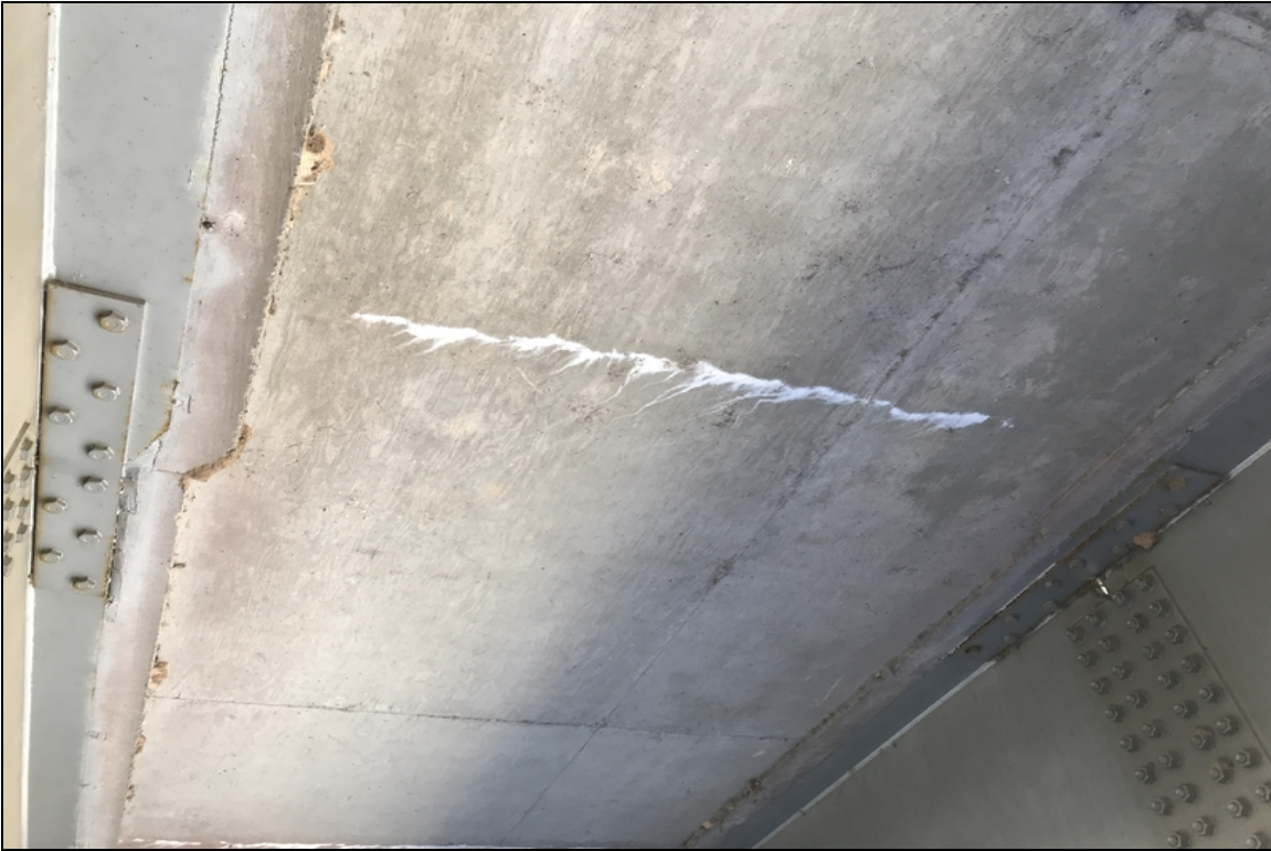
Soffit - Span 4 Bay 2: Efflorescence
