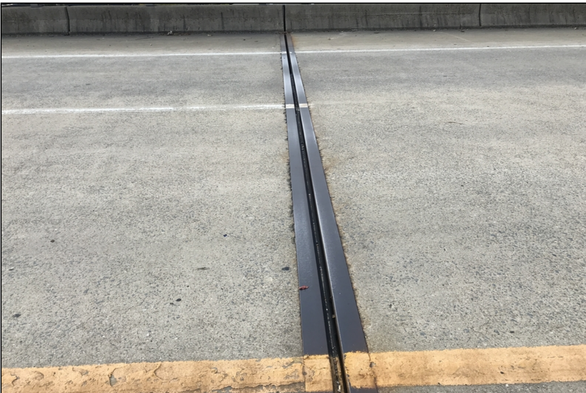
Joint - Bent 7 right: Loss of adhesion/spalling of adjacent deck
