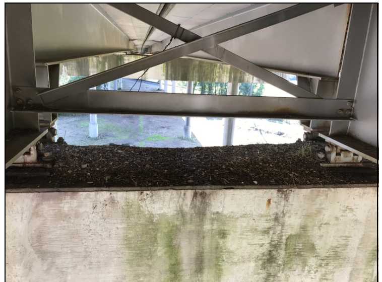
Cap - Bent 16 @ centerline: Debris build-up
