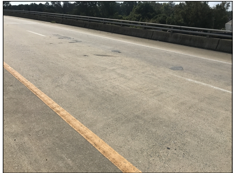
Deck - Span 7 right: Spalling/patches
