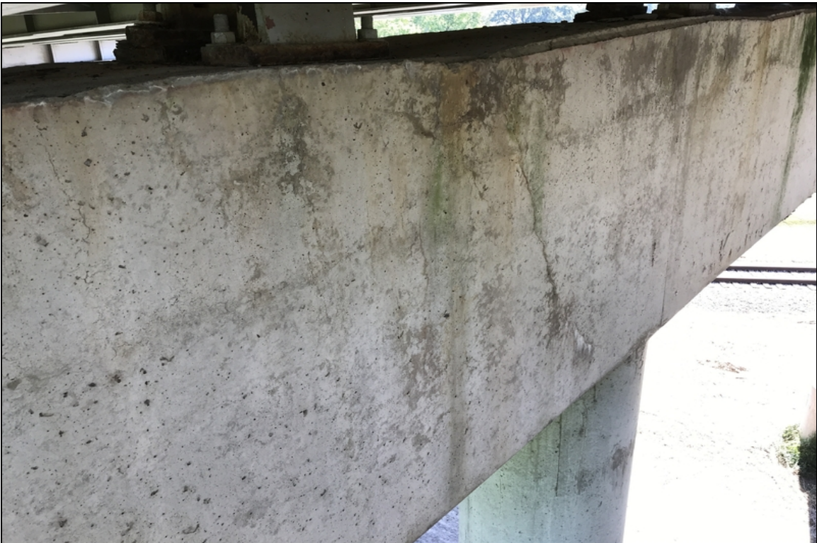
Cap - Bent 21 back left: Cracking
