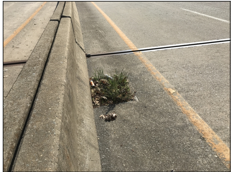
Drain - Span 24 right (inner gutterline): Stopped up
