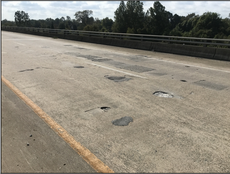
Deck - Span 9 right: Spalling/patches/rebar exposed
