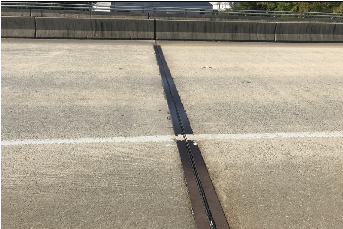
Joint - Bent 8 left: Adjacent deck spalling
