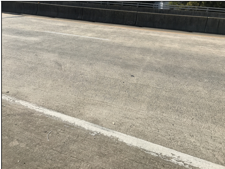
Deck - Span 2 left: Cracking
