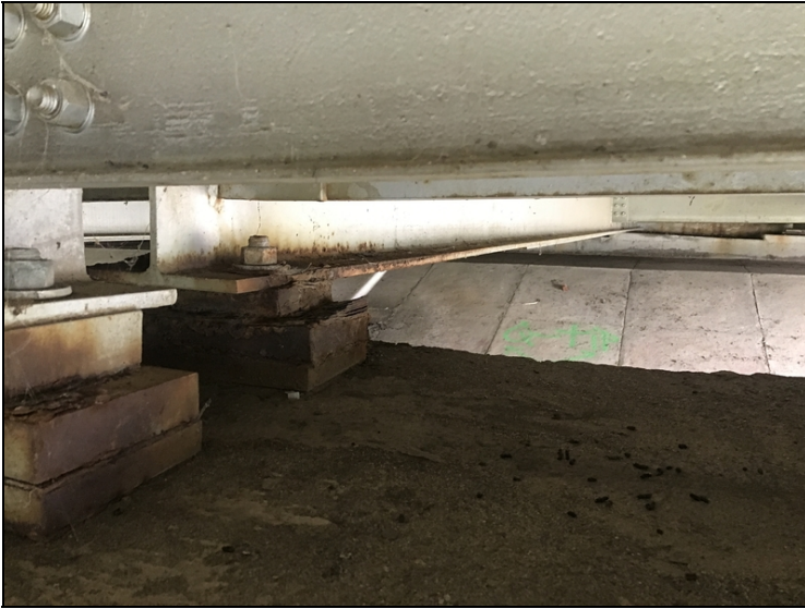
Span 31 Girder 7 right @ Bent 31: Corrosion
