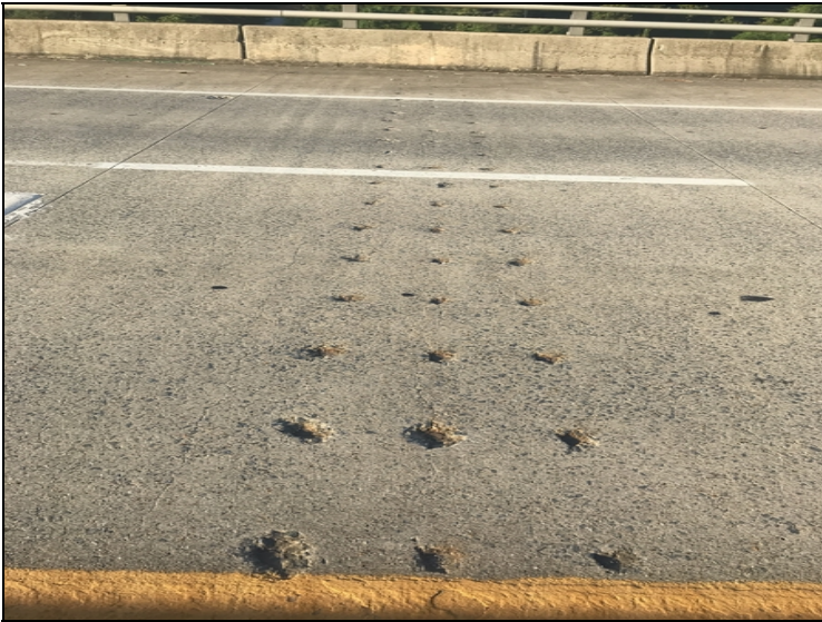
Deck bent 14 south bound small spalls at shear connectors of cap. Common bent 14 north bound.
