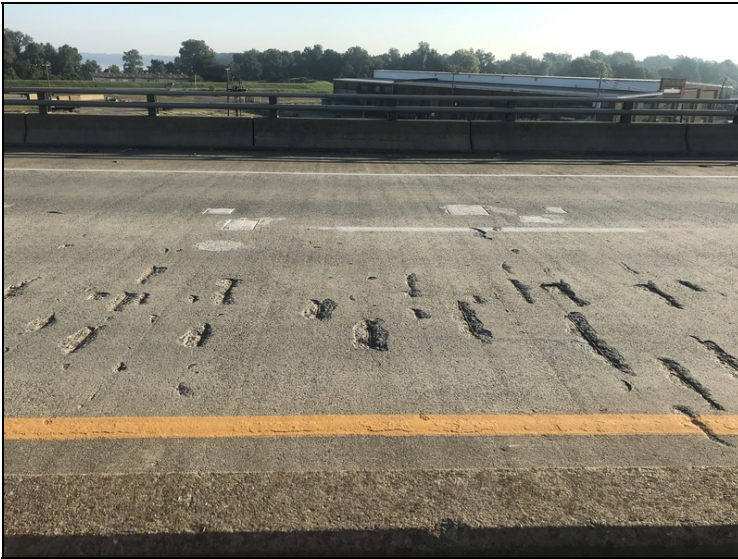
Span 14 north bound lanes have many small spalls with exposed rebar.
