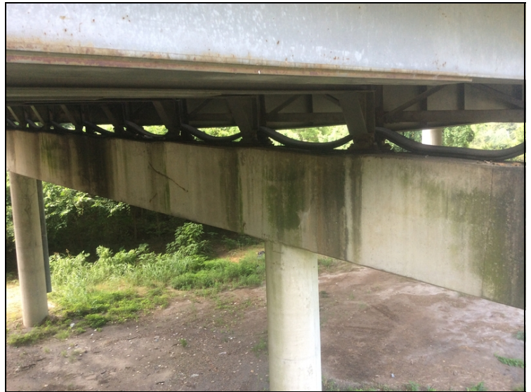
Bent 24 joint seal has fallen completely out and is laying on cap/ bearings.
