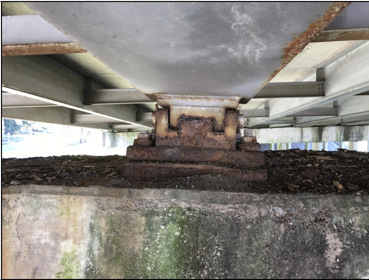
Bent 4 Bearing 8 ahead: Corrosion
