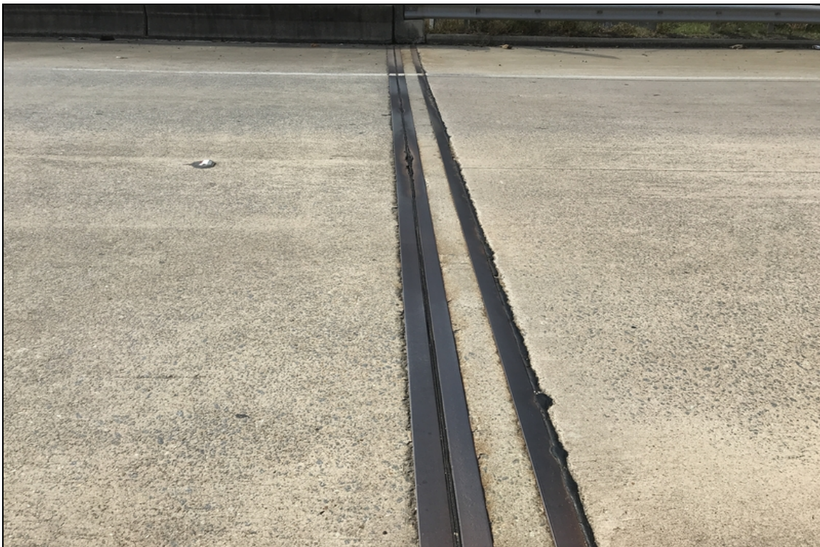
Joint - Bent 1 right: Damage
