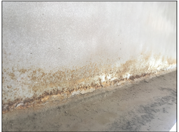
Span 5 Girder 10 left: Corrosion on bottom of web
