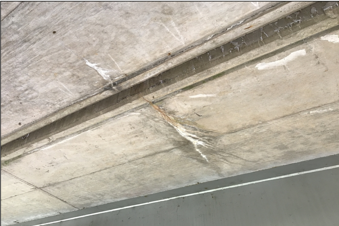
Soffit - Span 22 left: Efflorescence on center overhang
