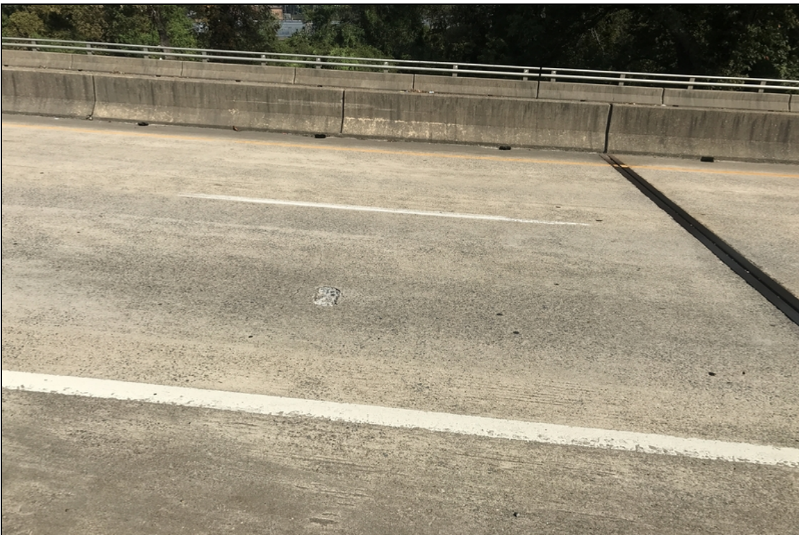
Deck - Span 25 right: Cracking/spalling
