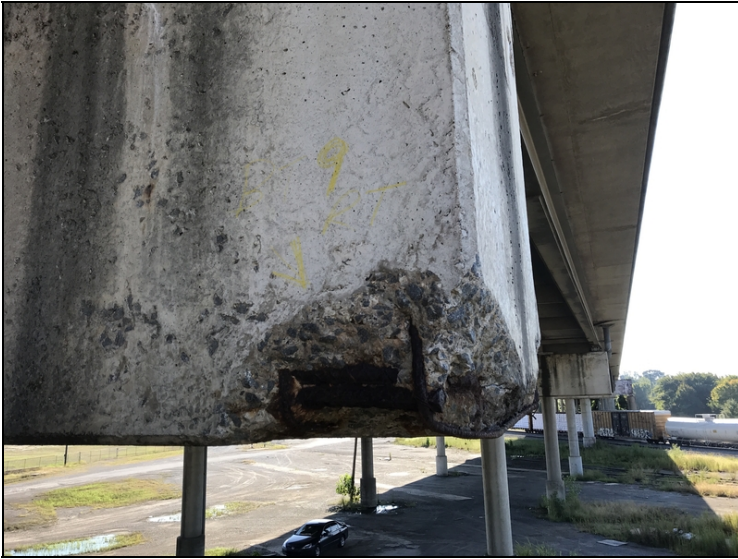
Bent 9 cap right side has spall with exposed rebar.
