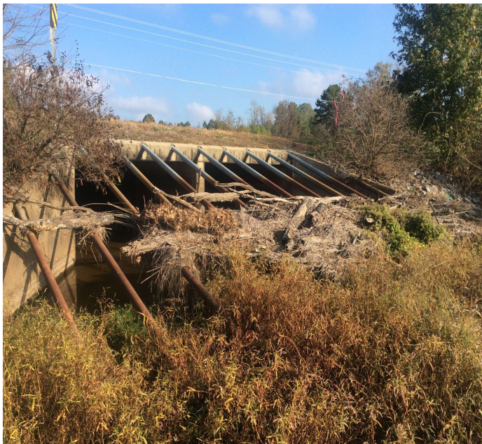
PHOTO 1 Description Channel - left end (debris build-up)
