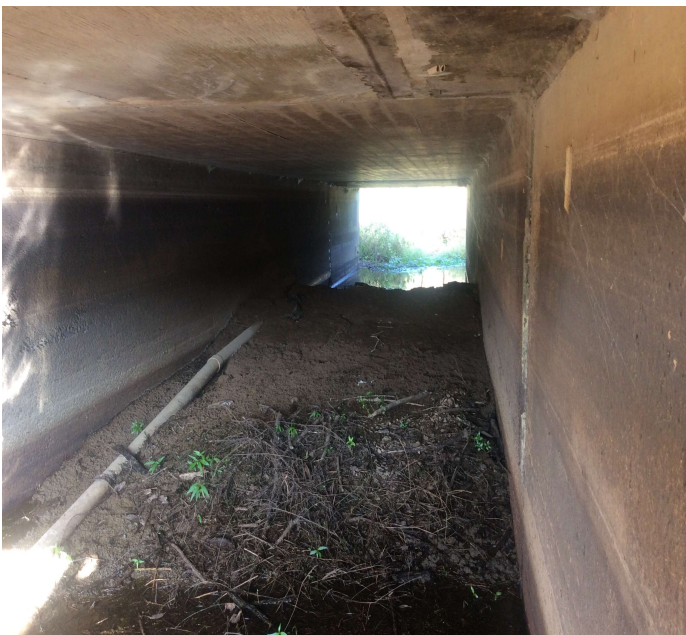
PHOTO 1 Description Channel - Barrel 2 (silt build-up)
