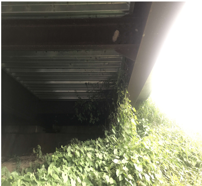
PHOTO 1 Description End-slope - Bent 4 right: Vegetation
