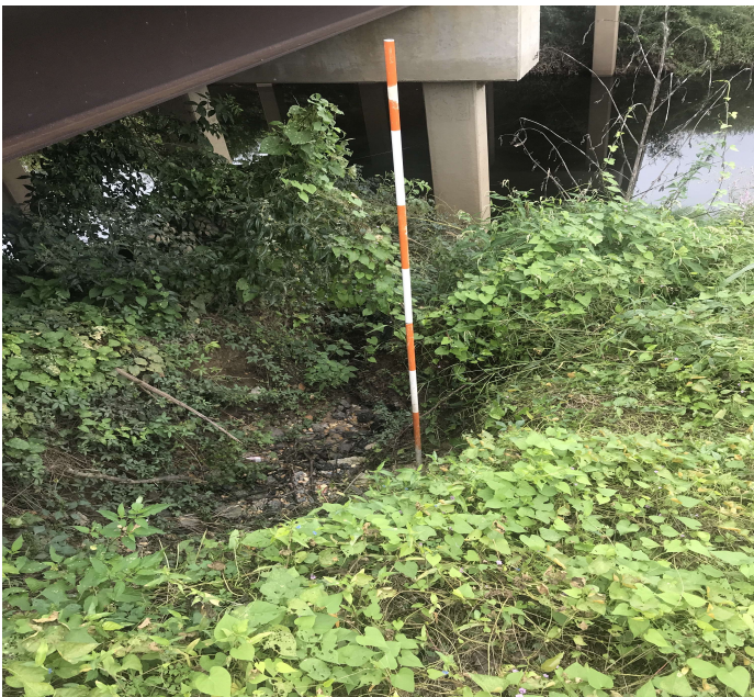
PHOTO 1 Description End-slope - Span 3 left : Erosion
