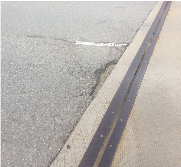
PHOTO 1 Description Pot hole on south end of approach in right lane heading north .
