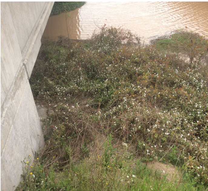
PHOTO 1 Description Bent 1 both sides of bridge Vines and vegetation growing along side .
