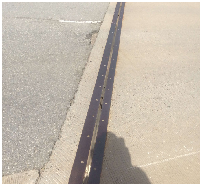
PHOTO 1 Description Bent 5 expansion joint has loss of adhesion and leaking . (Common at all expansion joints)
