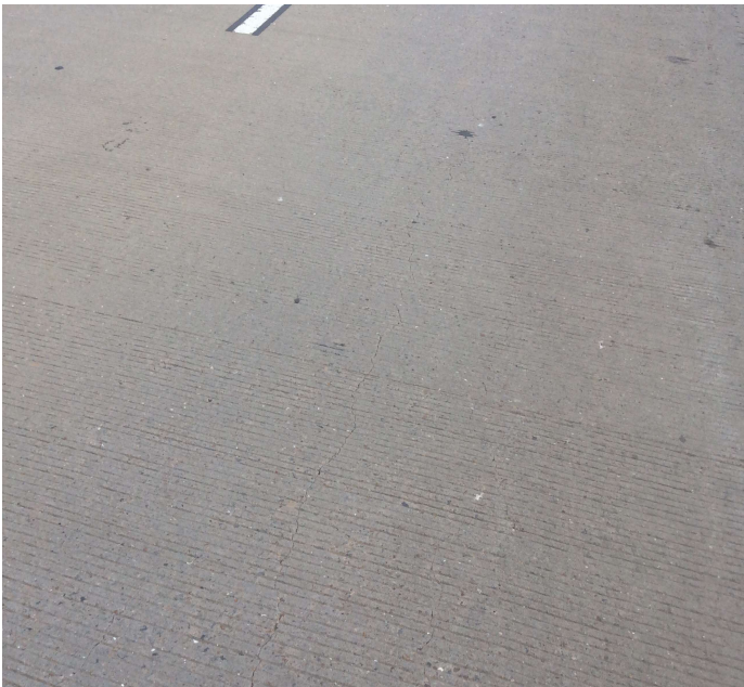
PHOTO 1 Description Longitudinal cracking at span 4 but common on all deck spans .
