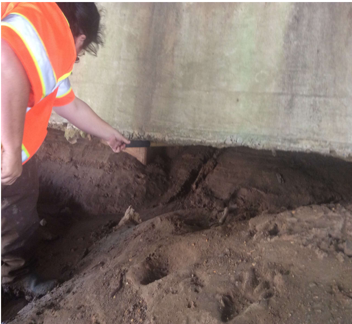
PHOTO 1 Description Erosion under abutment at bent 1 between girders 2 -5( is 4' back is exposing pile and to approach roadway .)
