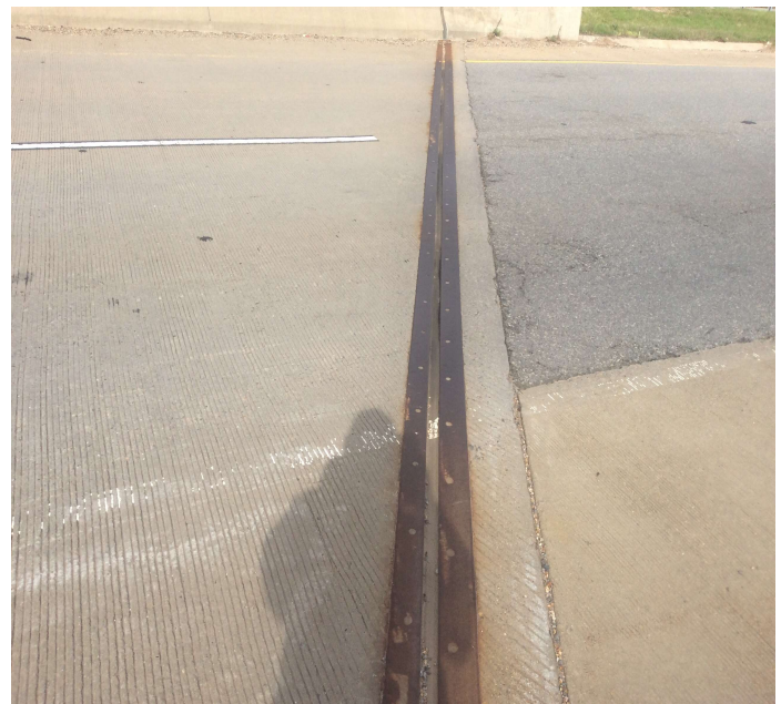
PHOTO 2 Description Expansion joint at bent 1 has some loss of adhesion , debris impact and leakage .
