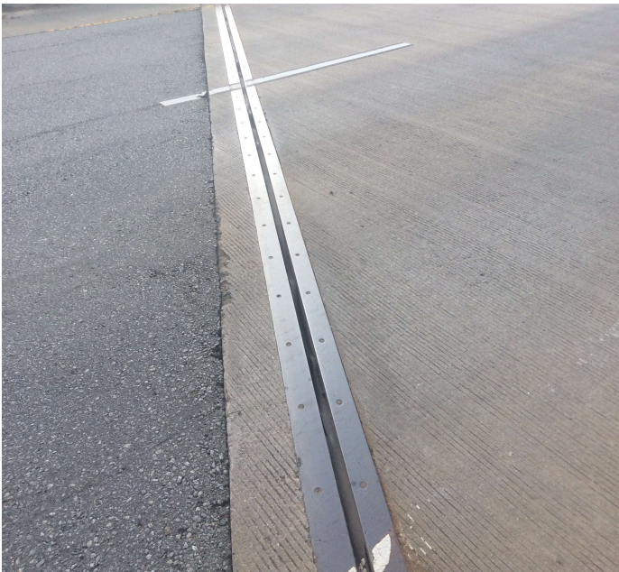
PHOTO 1 Description Bent 1 abutment pourable joint seal has loss of adhesion and are leaking .
