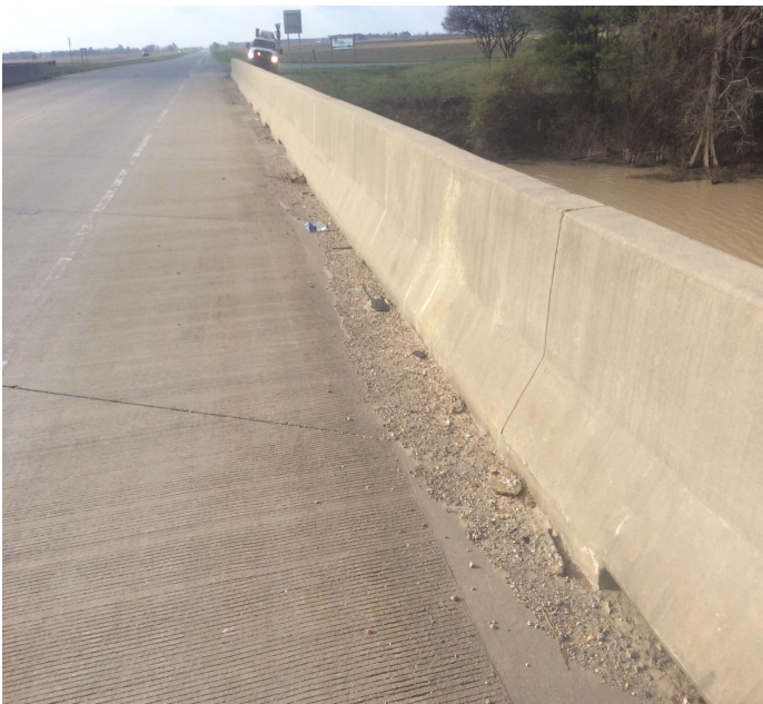
PHOTO 1 Description Gutter line have debris impeding waters flow mainly on right side of deck .
