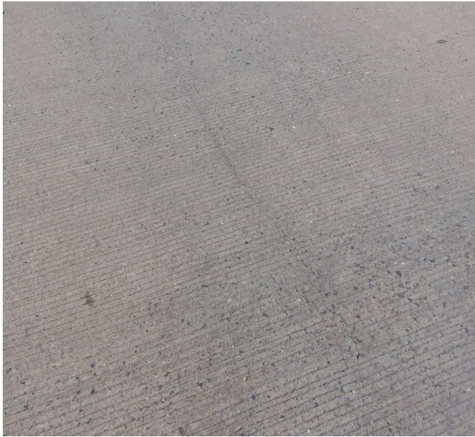
PHOTO 1 Description Longitudinal deck cracking at bent 4 near mid span in right lane but common on all spans .
