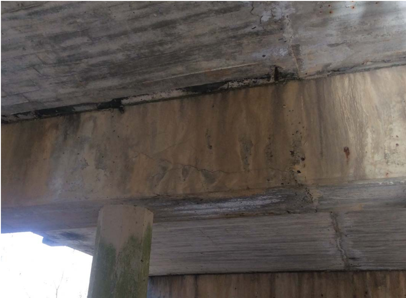
Bent 6 - cracking
