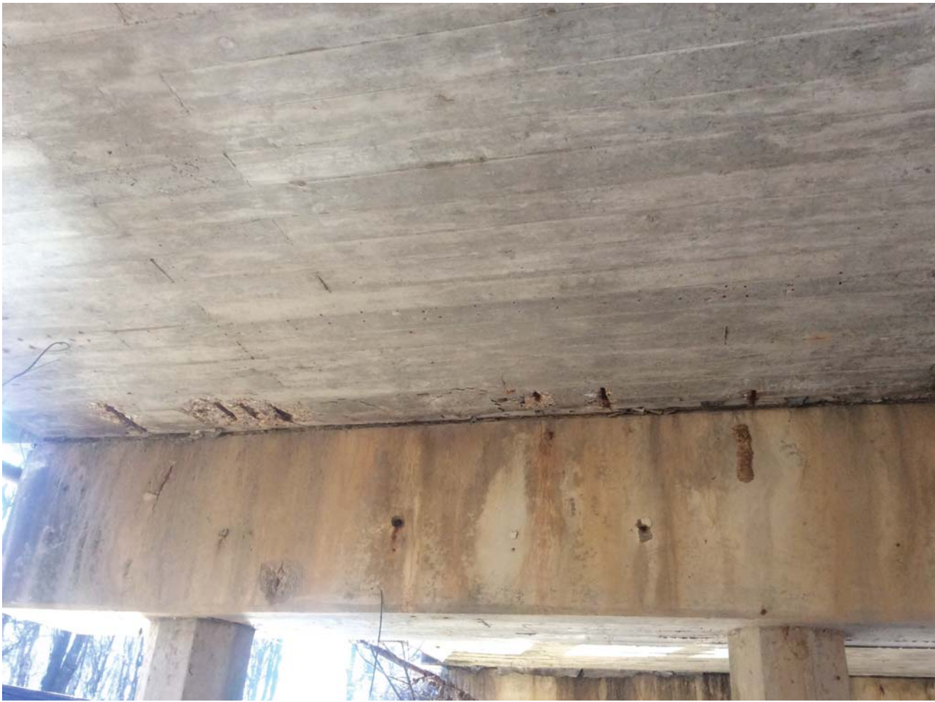
Soffit - Span 6 - exposed rebar
