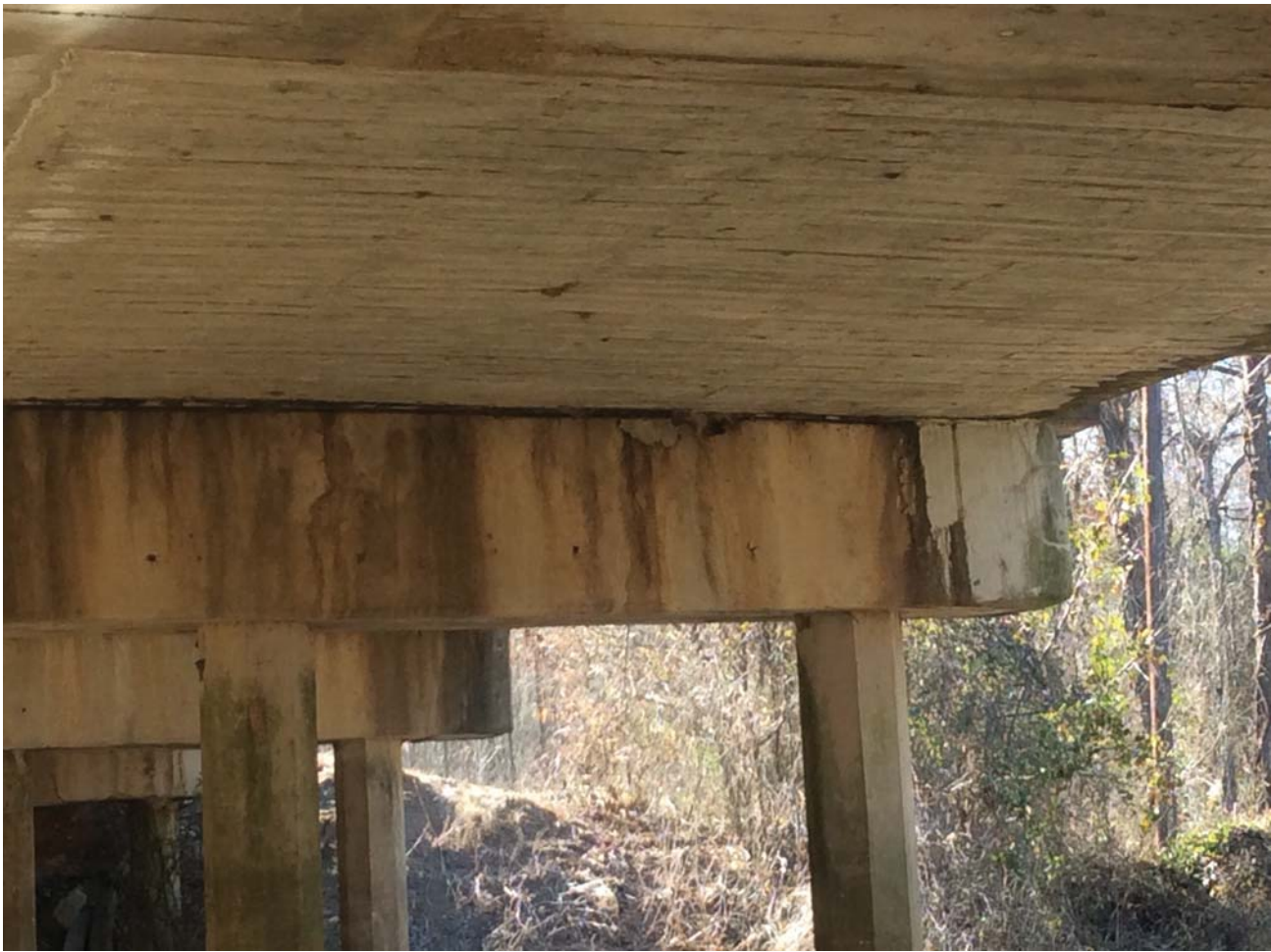
Bent 4 - delamination
