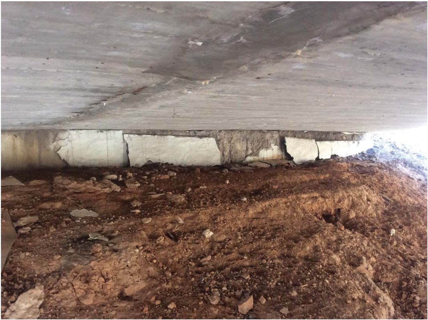
Abutment Bent 1 rebar exposed
