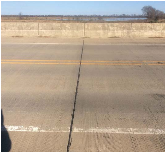
PHOTO 1 Description Joint - Bent 2: Loss of adhesion
