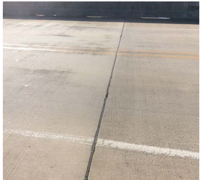
PHOTO 2 Description Joint -Bent 4: Loss of adhesion
