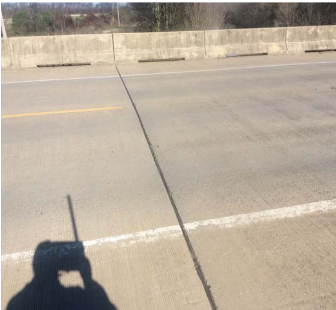
PHOTO 1 Description Joint - Bent 2: Loss of adhesion
