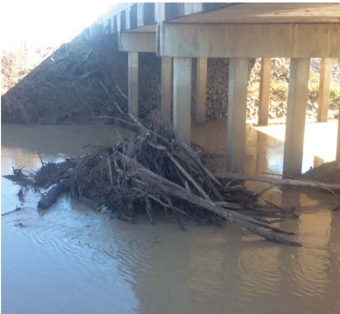
PHOTO 1 Description Channel - Bent 3 left: Debris build-up
