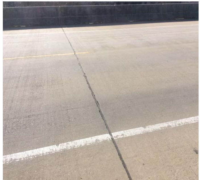
PHOTO 2 Description Joint - Bent 4: Loss of adhesion
