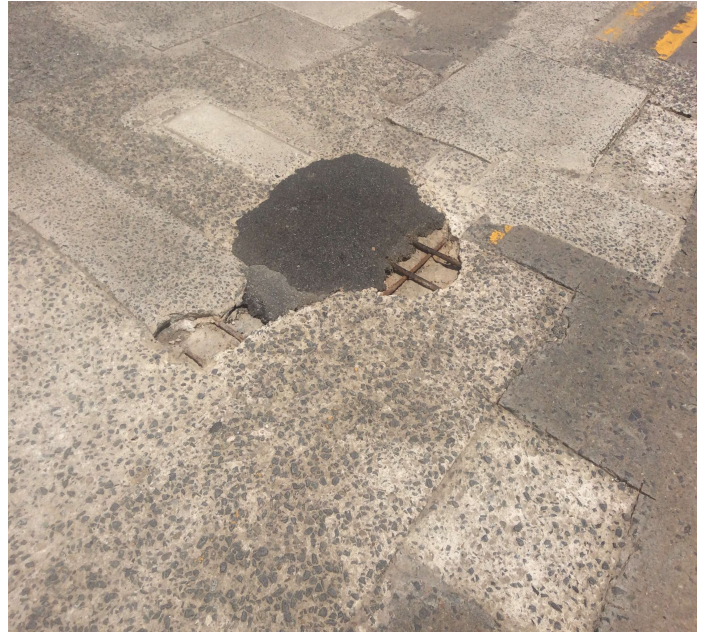
PHOTO 5 Description Span 1 near bent 1 spall with exposed rebar
