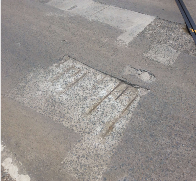
PHOTO 3 Description Spall with exposed rebar span 3 near bent 3
