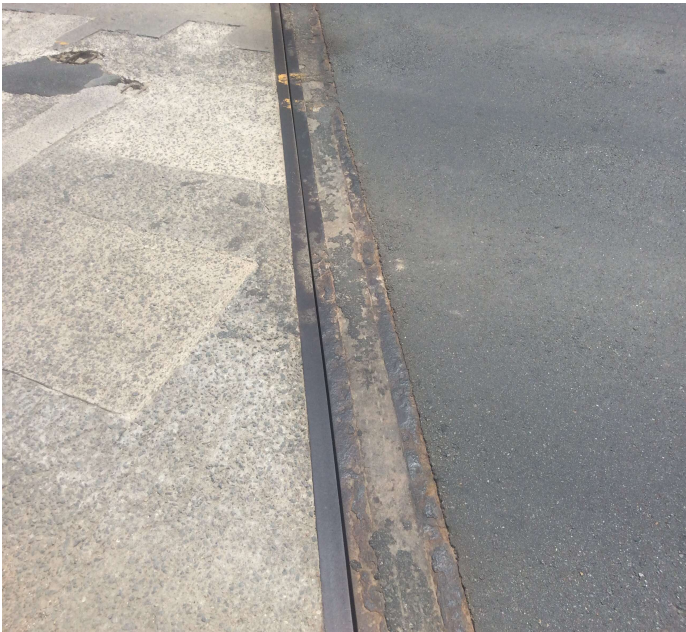
PHOTO 1 Description Open joint seals at span1 bent 1
