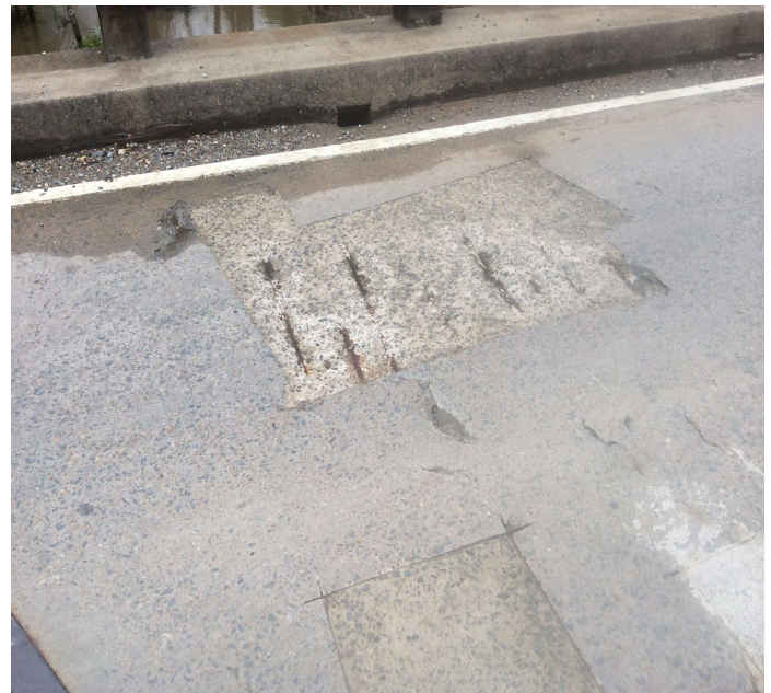
PHOTO 2 Description Span 3 left lane near bent 3 spall with exposed rebar in previously patched area.
