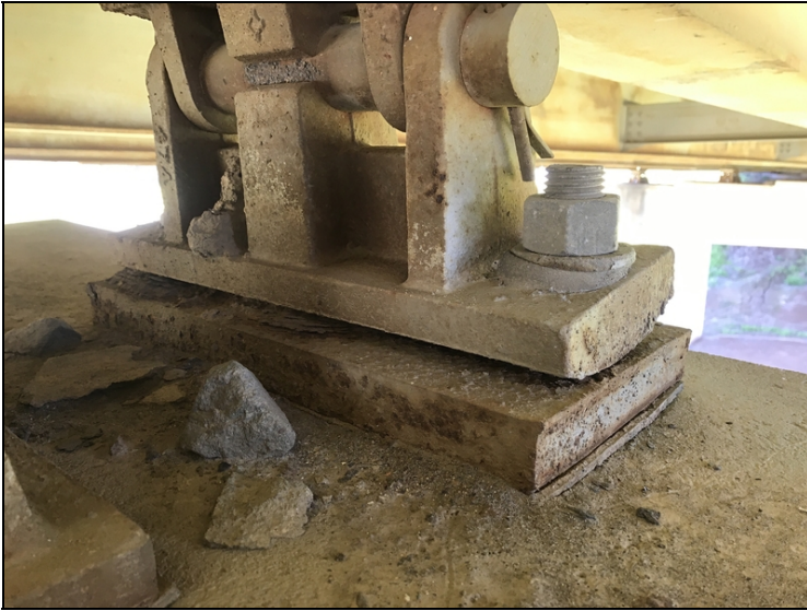
Bent 17 ahead bearing 4 has some pack rust between plate and bearing.
