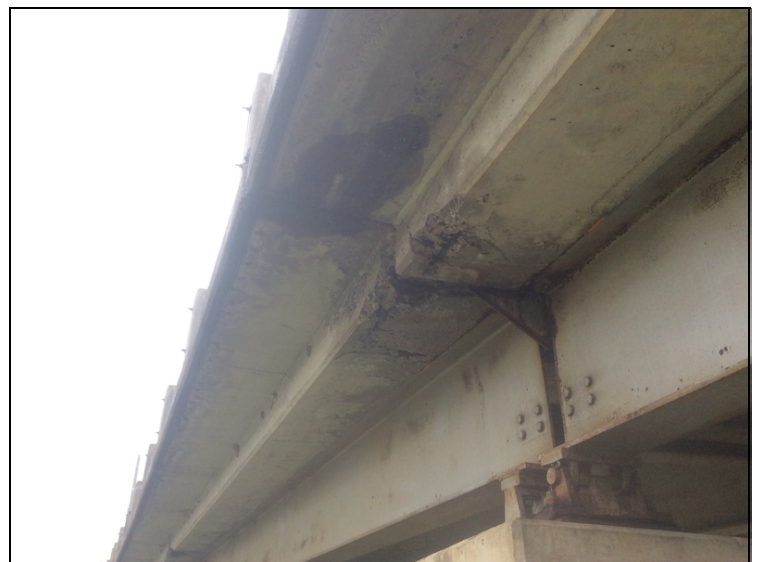
Deck soffit at bent 3 left spalls with exposed rebar near joint armor.
