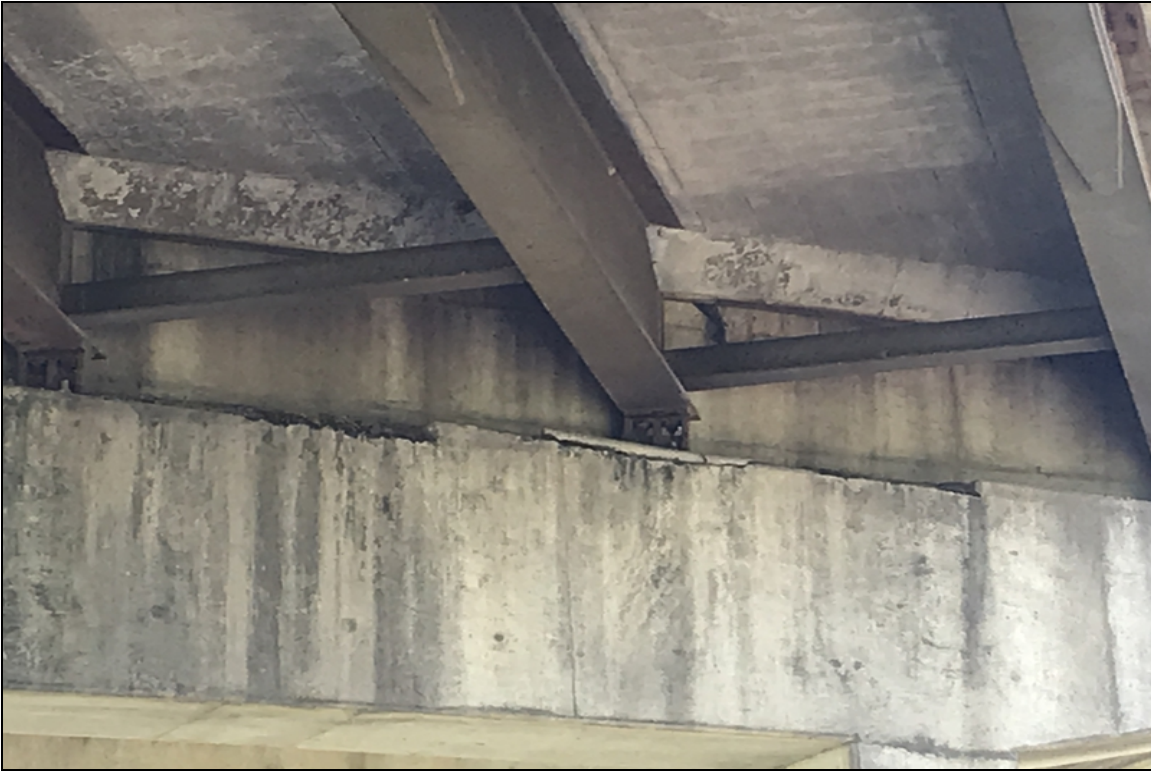
Cap - Bent 10 @ Bearing 4: Spall
