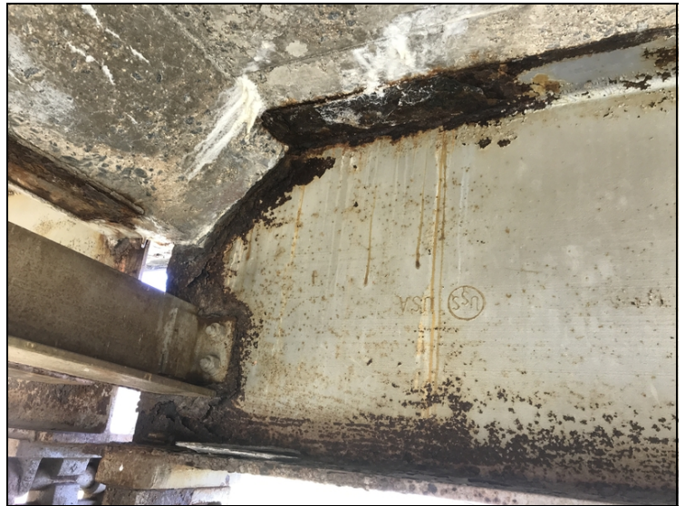
Bent 5 span 5 girder 1 has heavy flaking rust with section loss to top flange and lower web and flange.
