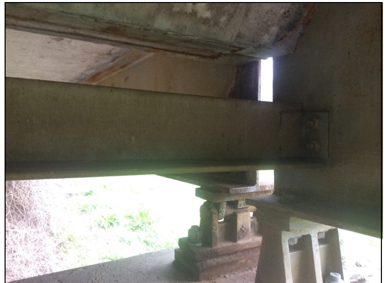
Span 1 bent 2 girder 1 has some light flaking rust to end 1'
