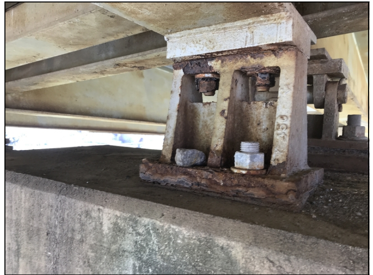
Bent 15 bearing 3 back has heavy flaking rust.
