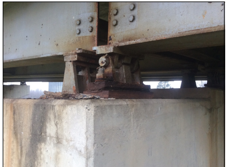
Bent 4 bearing 1 heavy flaking rust.
