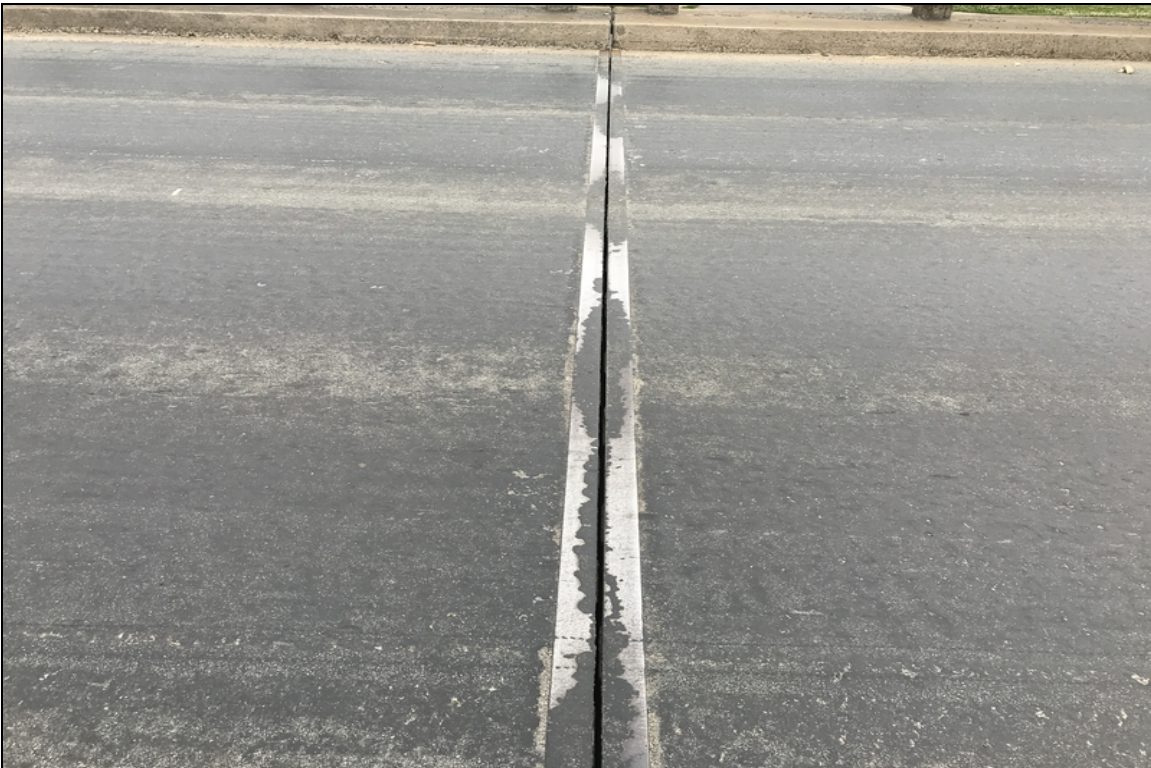
Joint - Bent 16: Material missing
