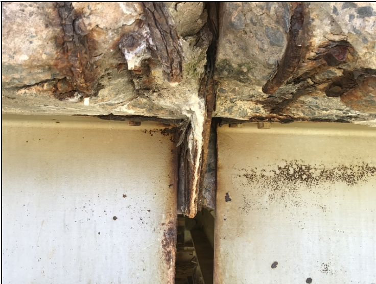
Bent 4 joint armor left side is completely closed due to pack rust.
