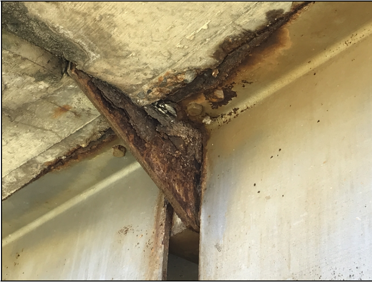
Bent 18 left has heavy flaking rust to joint armor and girder ends.
