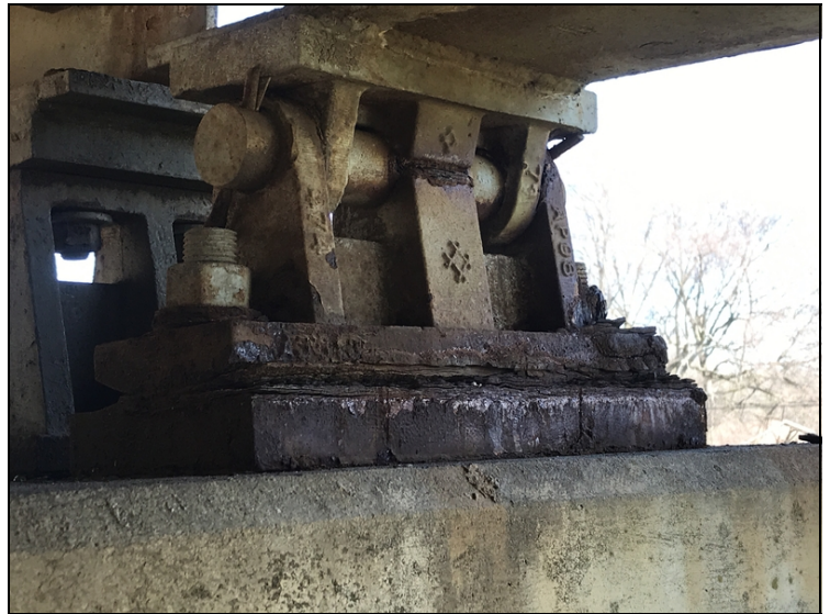
Bent 15 ahead bearing 1 has heavy flaking rust and pack rust..
