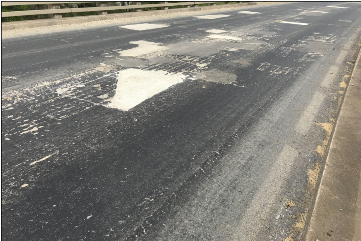
Deck - Spans 1-2: Spalling/patches
