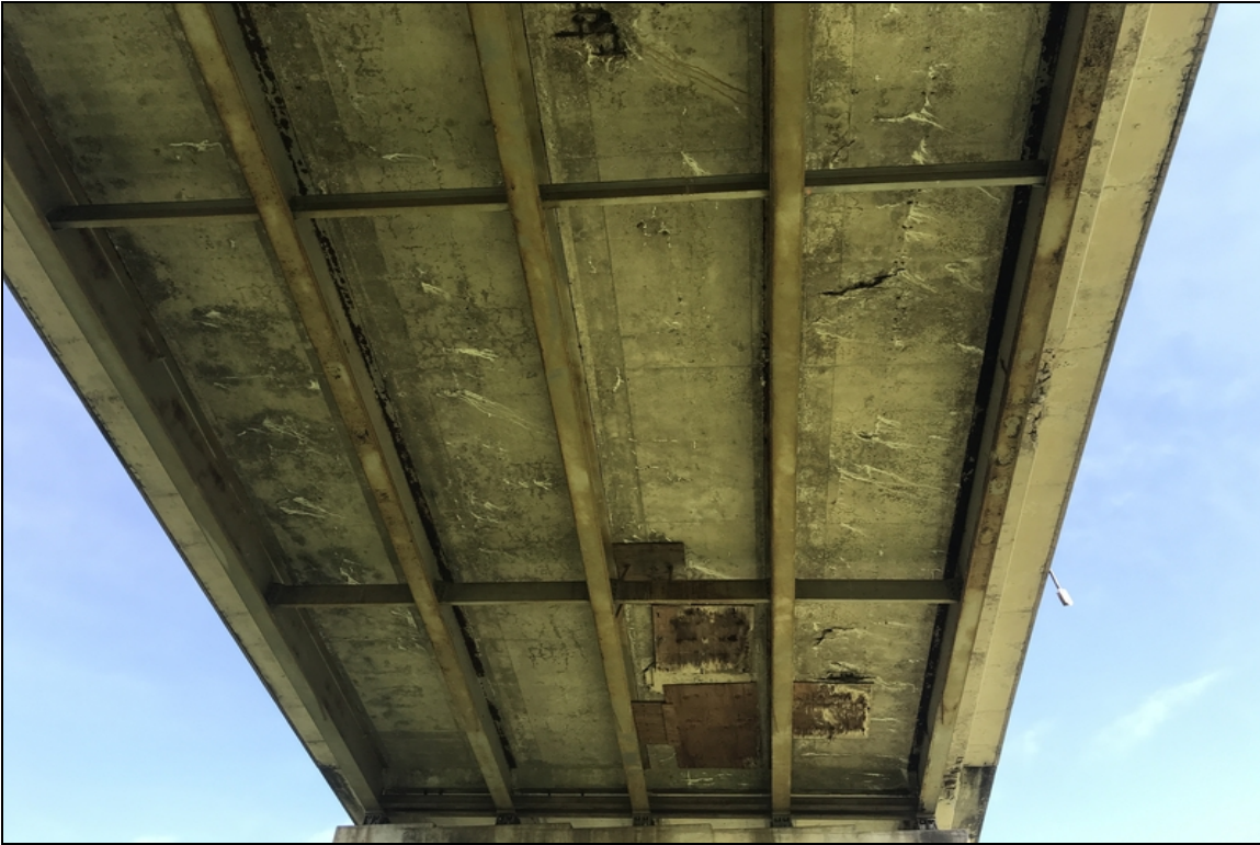
Soffit - Span 5: Efflorescence/patches
