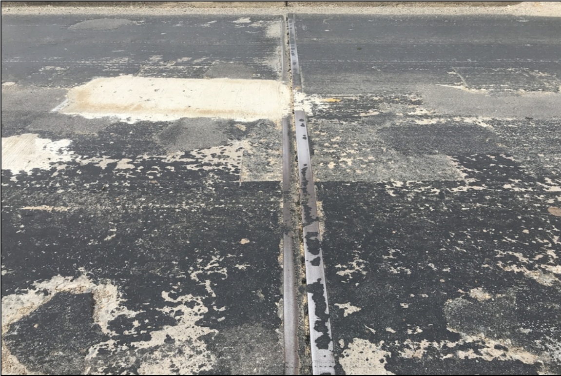
Joint - Bent 4: Loss of adhesion
