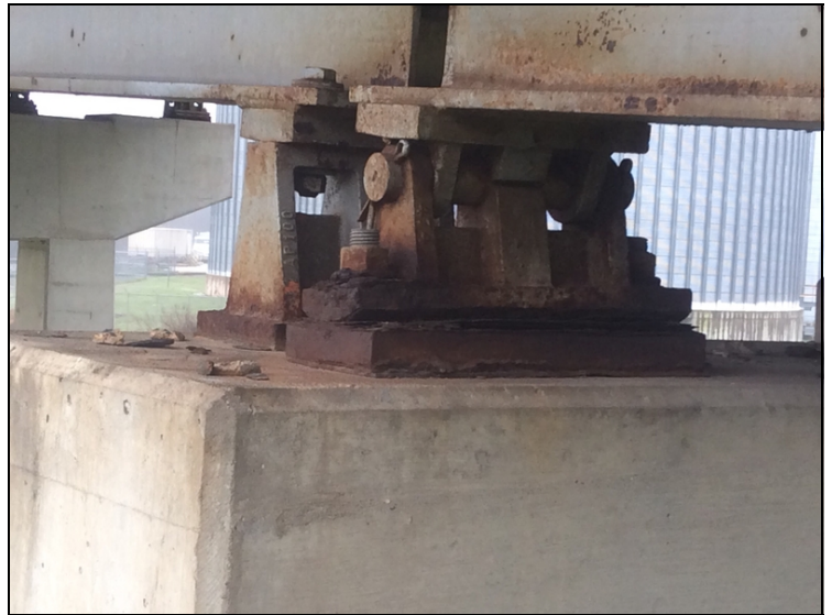
Span 2 bent 3 bearing 1 heavy flaking rust to bearing and masonry plate. Common on all bearings this bent to a lesser extent.
