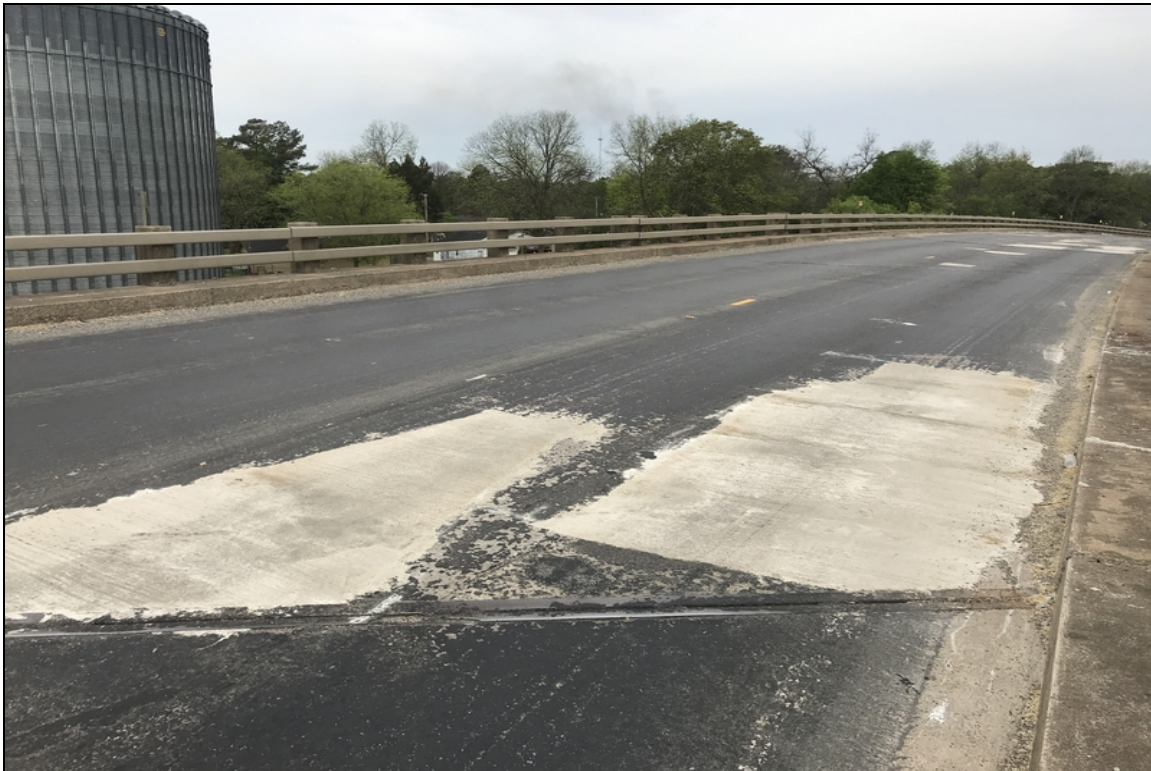
Deck - Span 10: Patches
