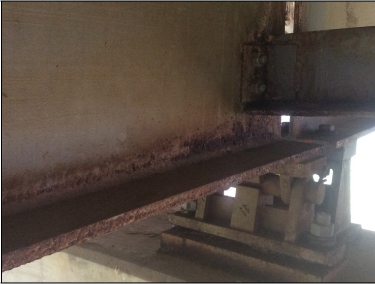
Span 2 bent 3 girder 2 has some light flaking rust to lower web and flange.
