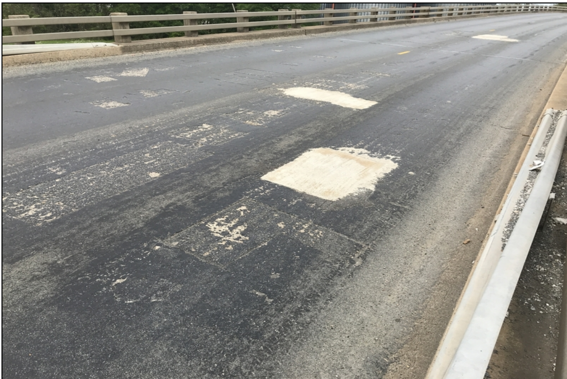
Deck - Spans 17-18: Spalling/patches
