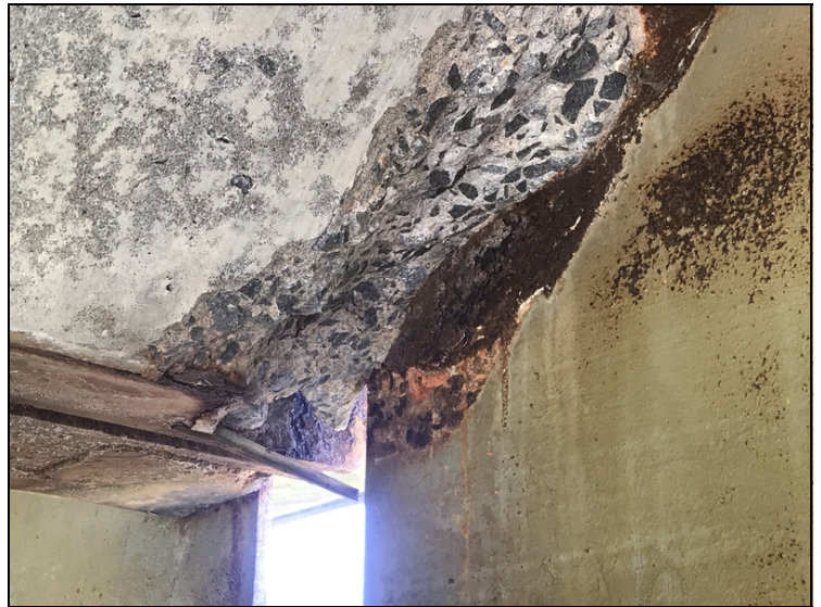
Bent 16 back left side of girder 5 has flaking rust in hunch area. Common in many locations.
