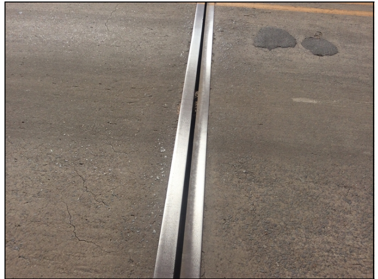
Bent 13 joint seal missing .
