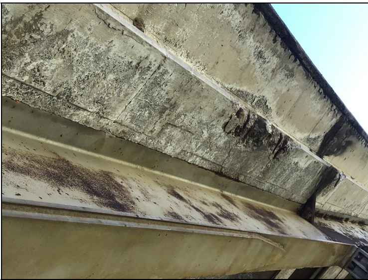
Span 6 left soffit at overhang drain opening spalling with exposed steel to bottom of deck.
