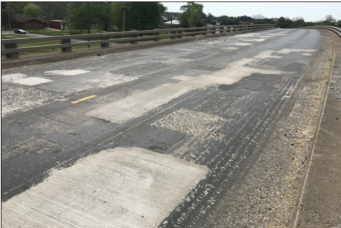
Deck - Spans 5-6: Spalling/patches
