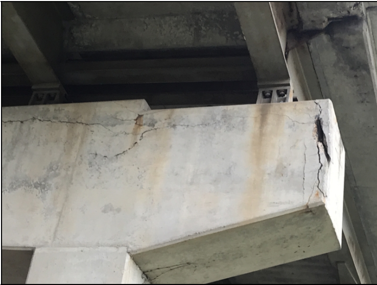
Bent 2 cap ahead face left has spall with exposed rebar and delamination with cracking.
