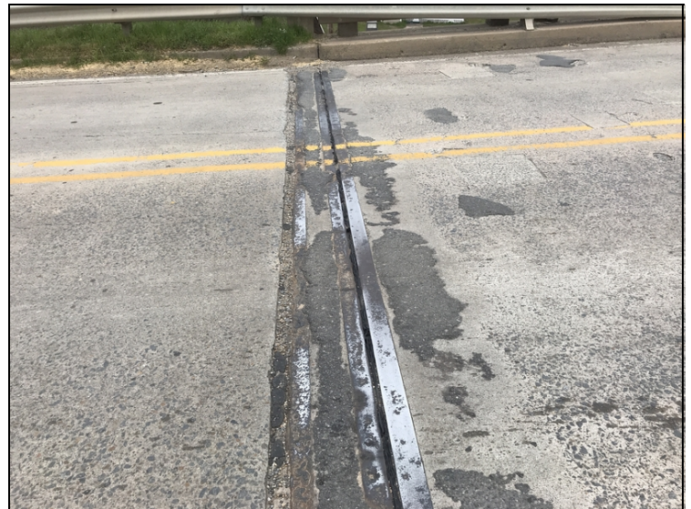
Bent 1 expansion joint damaged. This is Common at all joint.
