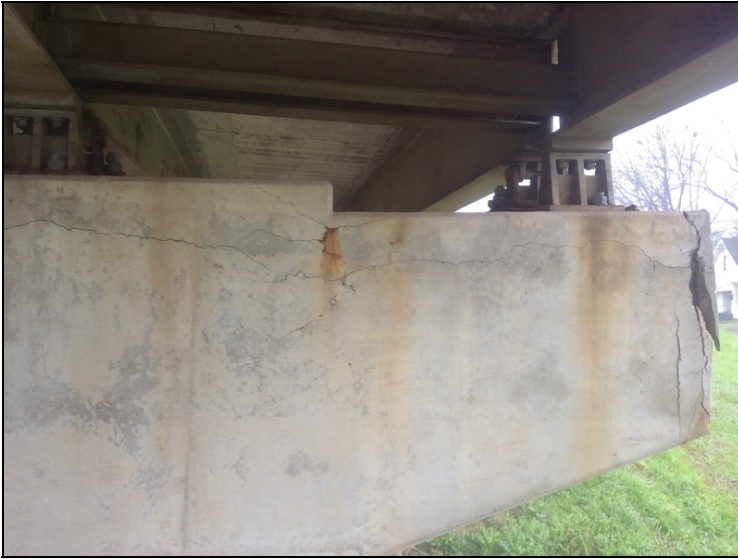
Bent 2 cap ahead has large horizontal cracks with some rust staining. Cap ahead left end has spall with exposed rebar.
