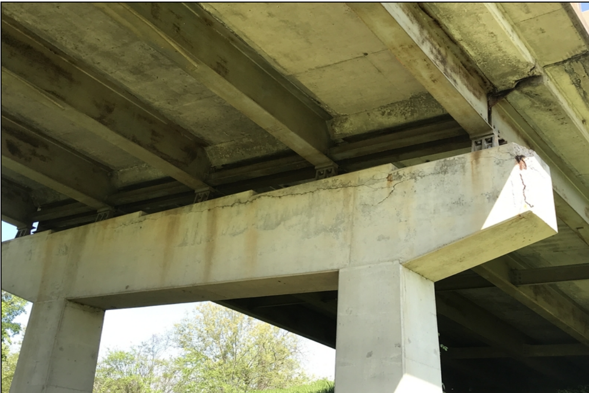
Cap - Bent 2 back: Cracking/spalling
