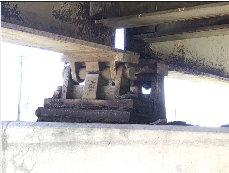
Bent 5 bearing 1 back has heavy flaking rust.
