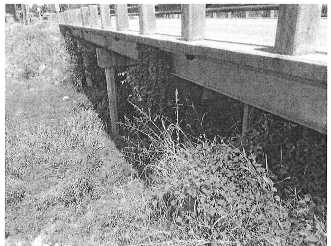
Figure 2. Bridge over outlet canal looking northeast.
