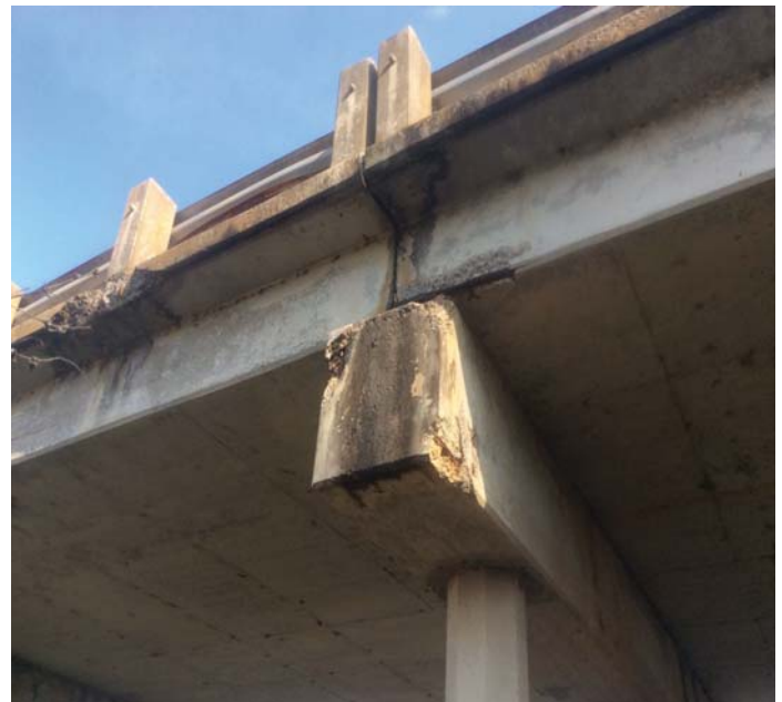
PHOTO 2 Description Cap - Bent 9 right end: Rebar exposed
