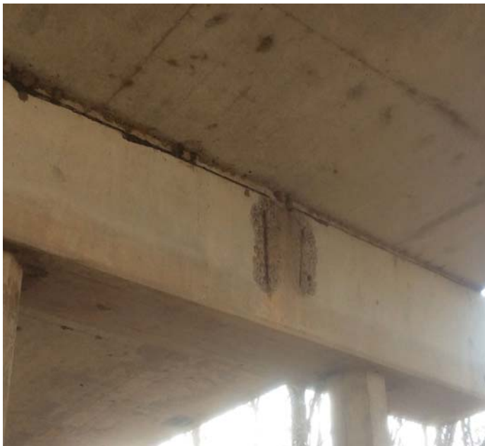
PHOTO 1 Description Caps - Bent 10 back: Rebar exposed
