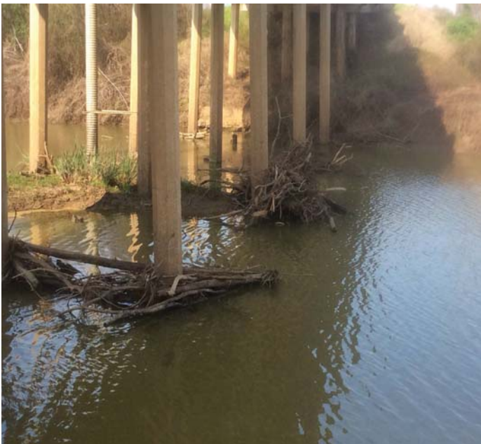
PHOTO 1 Description Channel - Bents 5-7: Debris build-up
