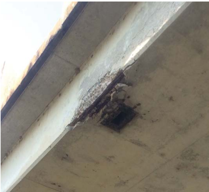
PHOTO 1 Description Soffit - Span 8 right: Rebar exposed
