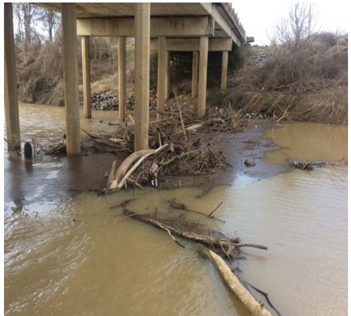
PHOTO 2 Description Channel - Bents 3-4 left (debris build-up)
