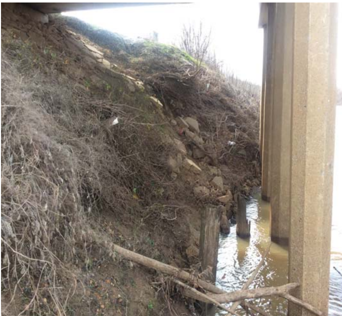
PHOTO 1 Description Endslope - Span 5 (erosion)
