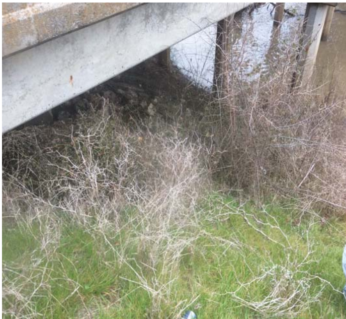
PHOTO 1 Description Span 1 small trees and vines along side of bridge.
