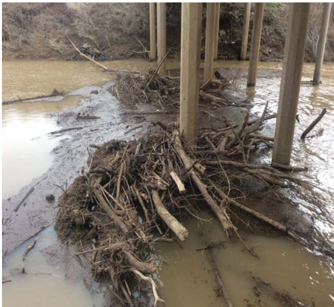
PHOTO 1 Description Channel - Bents 3-4 left (debris build-up)
