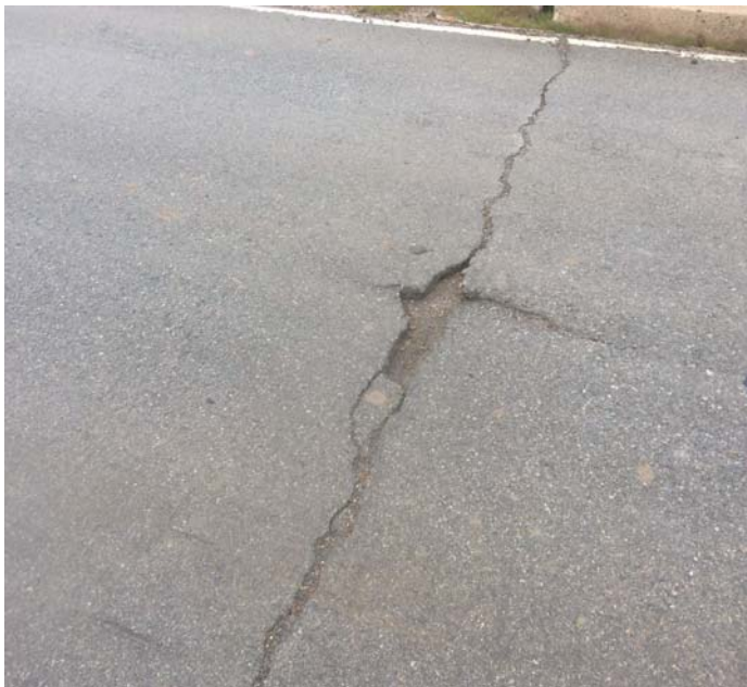
PHOTO 1 Description Beginning of bridge small pothole in roadway approach near center line.
