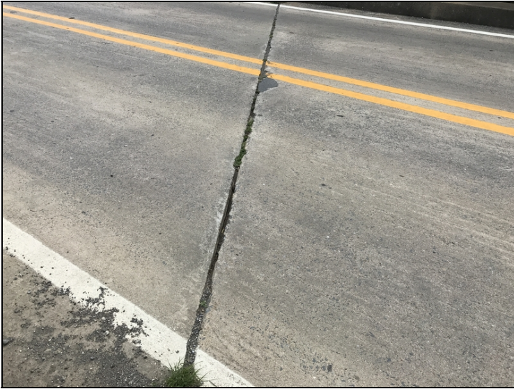
Joint - Bent 2: Material missing/debris filled
