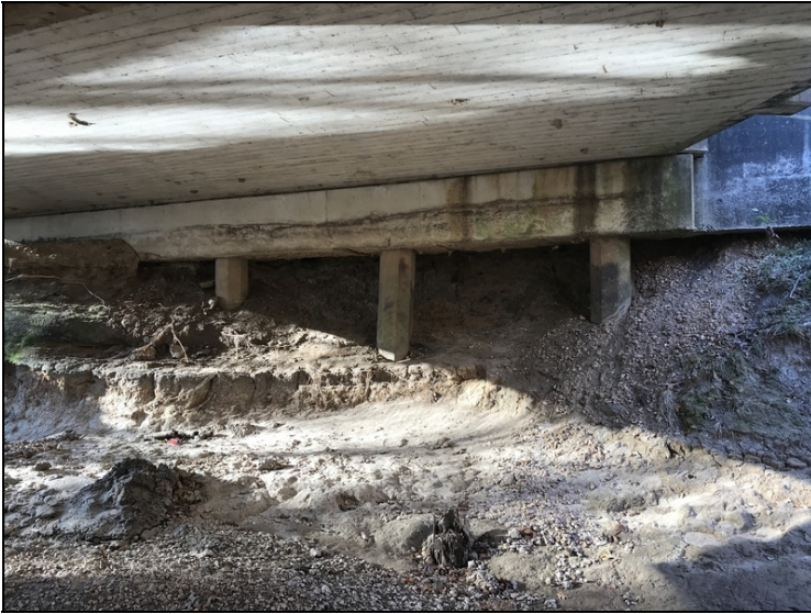
Bent 4 erosion 2020
