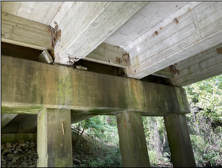
Loss of bearing area @ ends of Girders 1, 2 & 3 @ beginning of Span 2.
