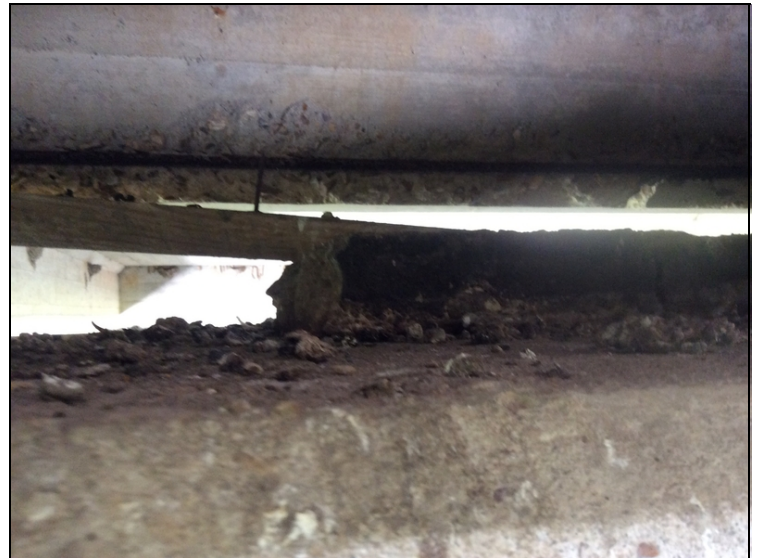
Cracking & spalls with rebar exposed to diaphragms between Girders 1-4 @ Bent 1.
