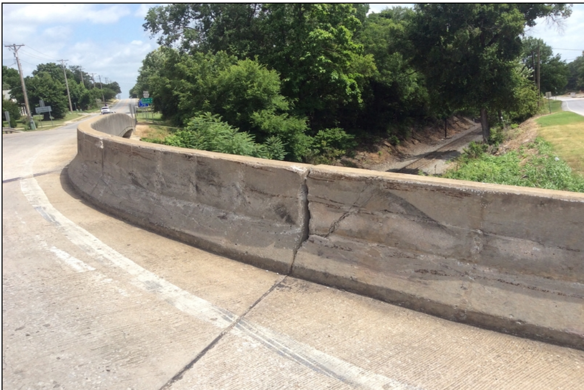
Railing left in spans 3 and 4 has Collision damage.
