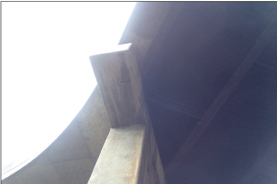
Bent 2 underneath cap left side has spalling with steel exposed.
