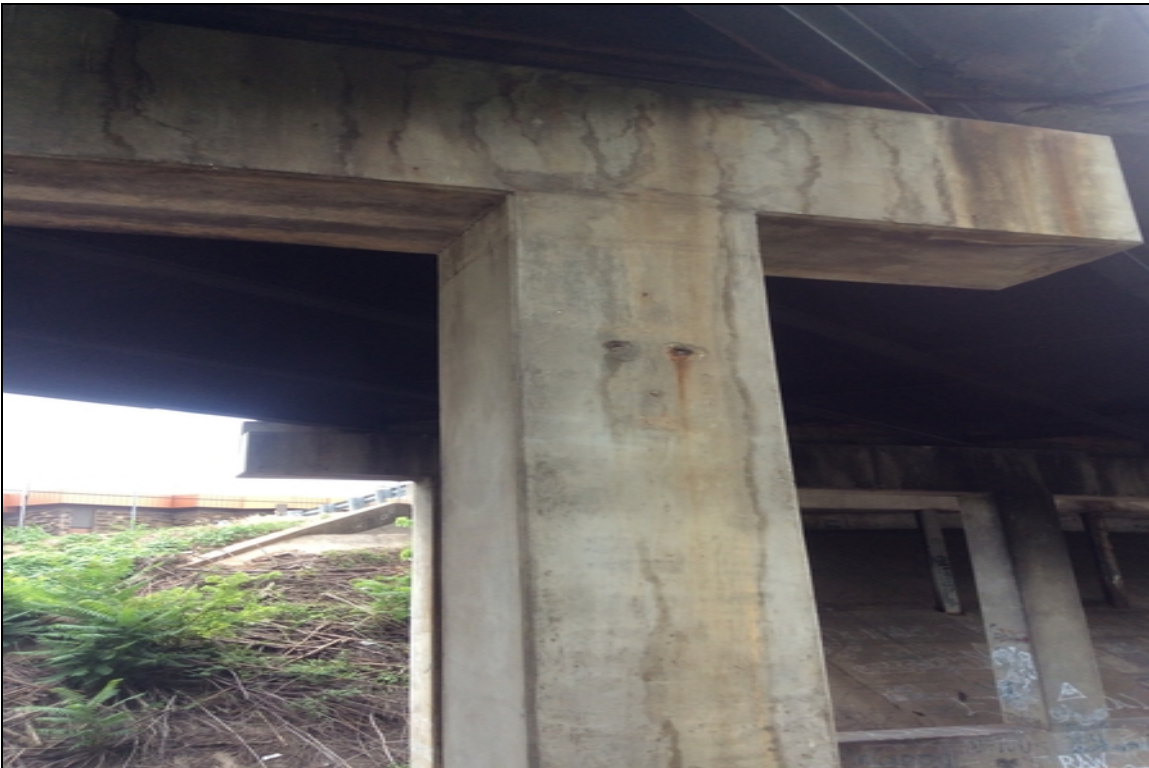
Bent 1 column 3 behind side has minor spalls with steel exposed.
