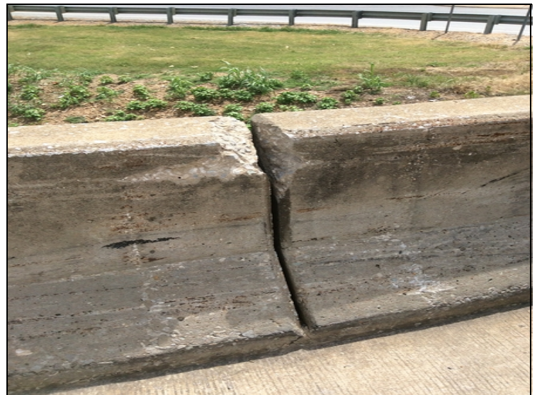
Large spall due to collision damage on railing left side span 3.
