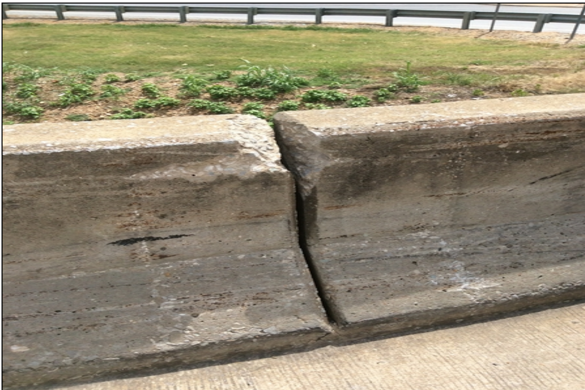
Large spall due to collision damage on railing left side span 3.
