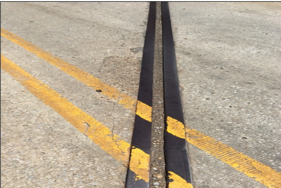
Span 1 spalling adjacent to road iron at bent 2.
