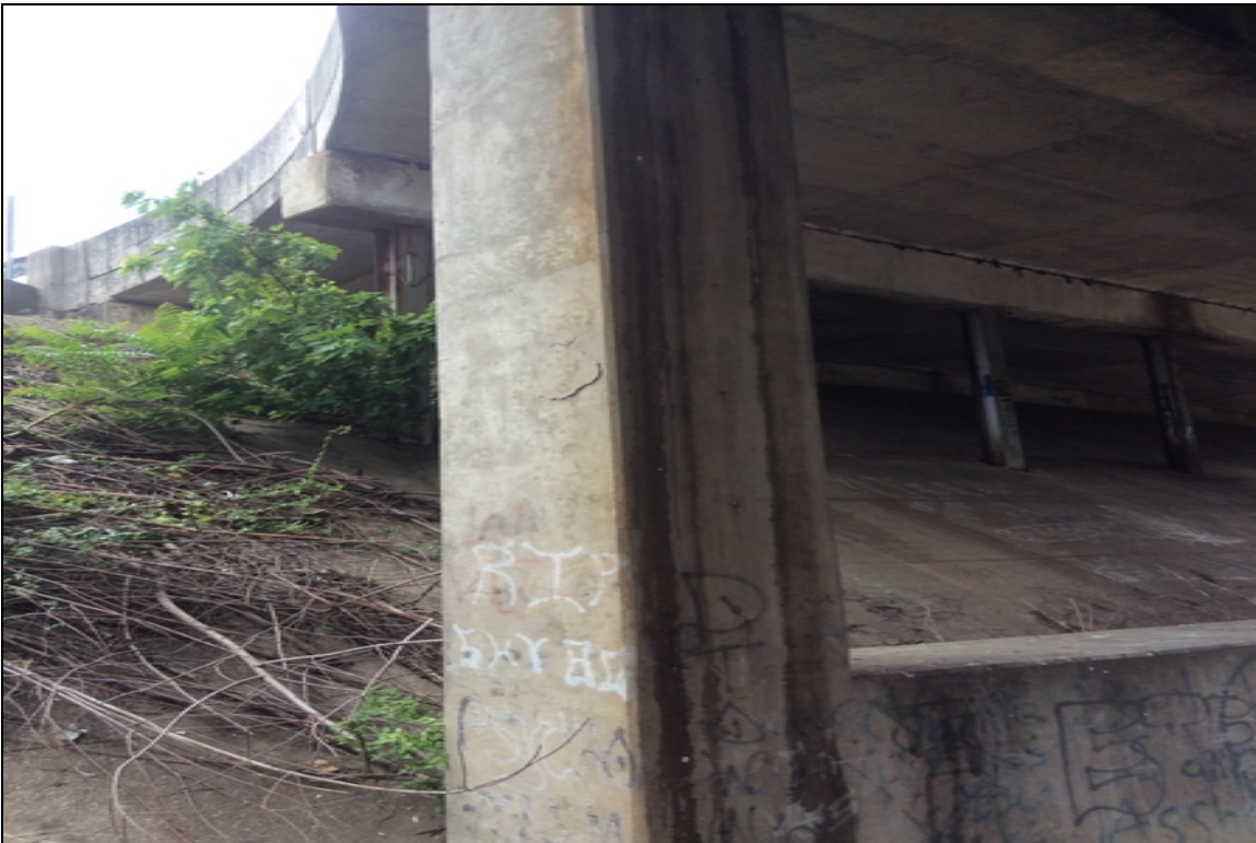
Bent 2 column 1 left side has a delaminated area.
