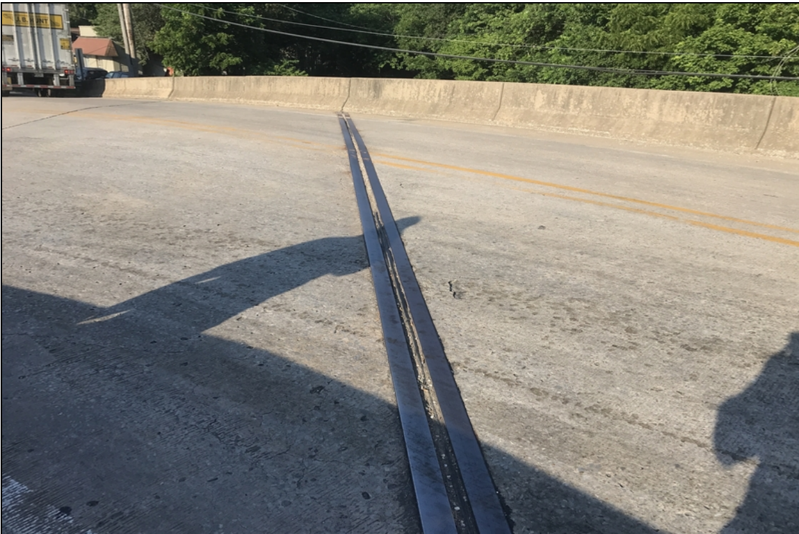
Bent #2 joint debris impaction.
