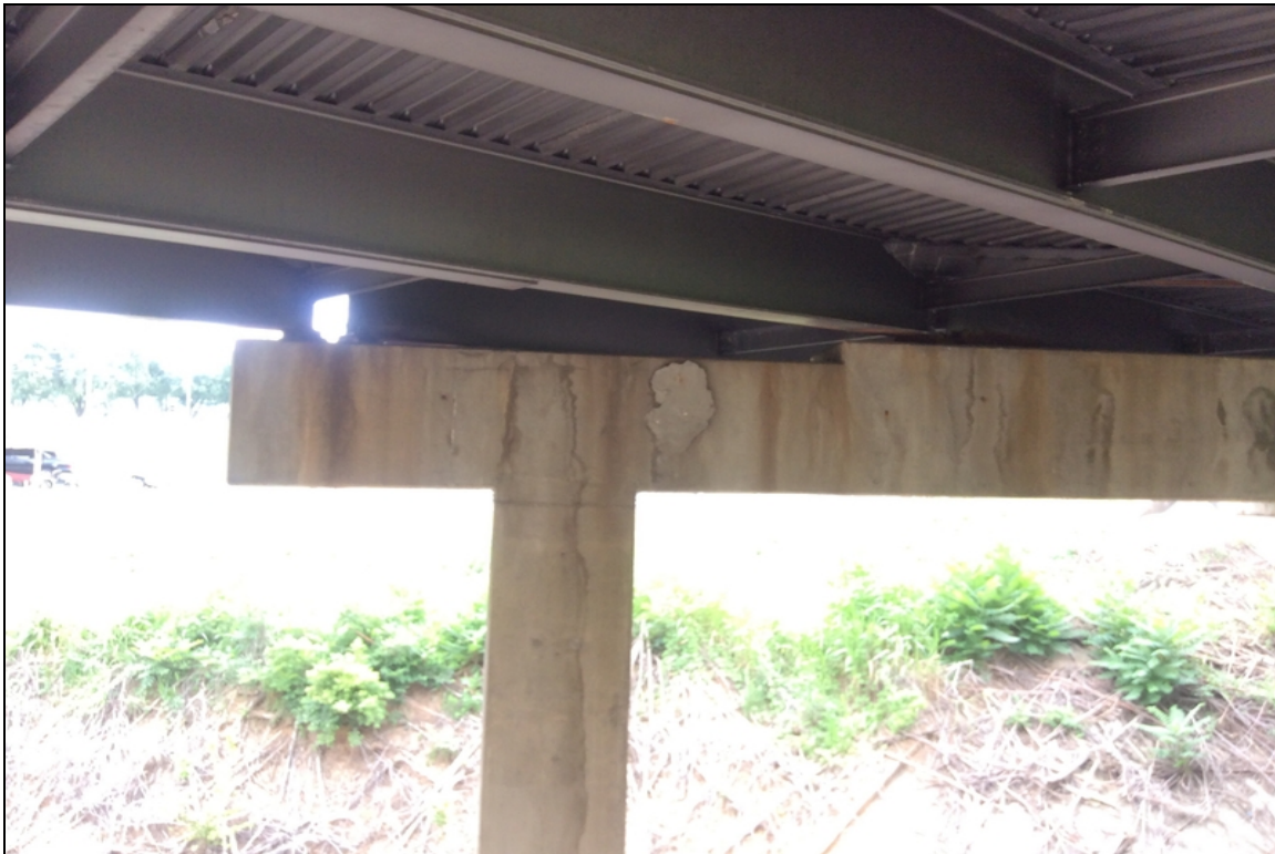
Bent 1 cap behind side left has large delaminated area.
