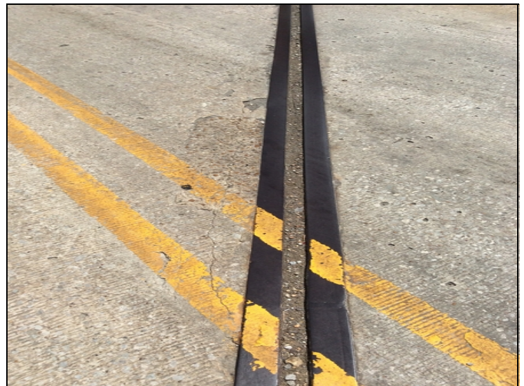
Span 1 spalling adjacent to road iron at bent 2.
