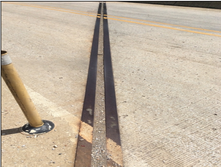
Bent 2 joint material has debris impaction
