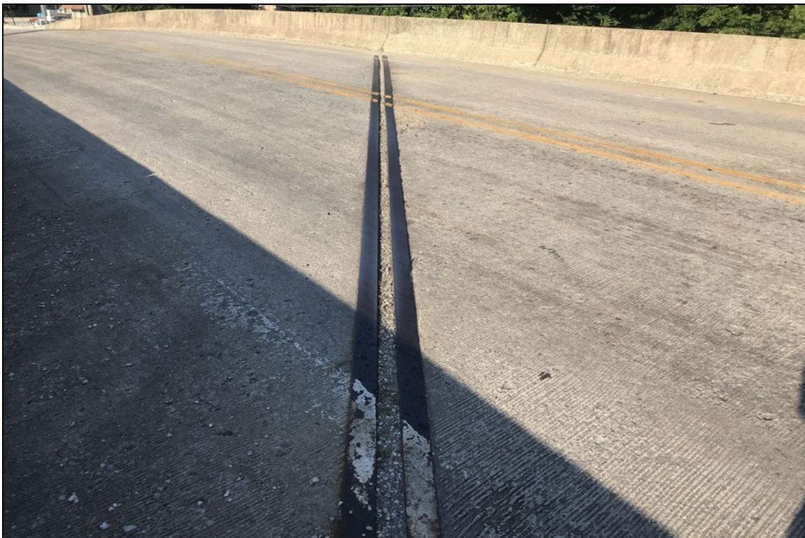
Bent #1 joint debris impaction.
