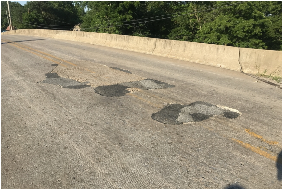
Span #1 large spalled patched areas near centerline.
