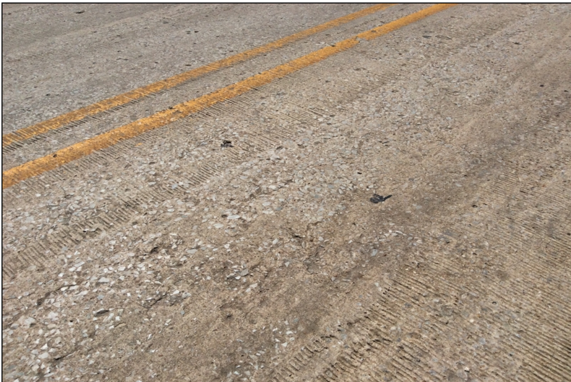
Span 1 typical wearing of driving surface.
