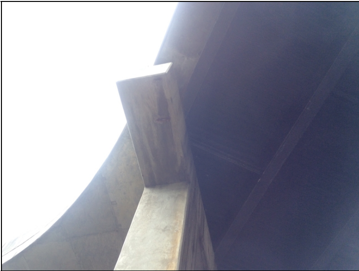
Bent 2 underneath cap left side has spalling with steel exposed.
