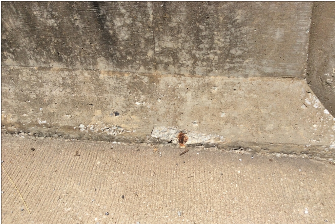
Span 1 right railing has spalling with steel exposed.
