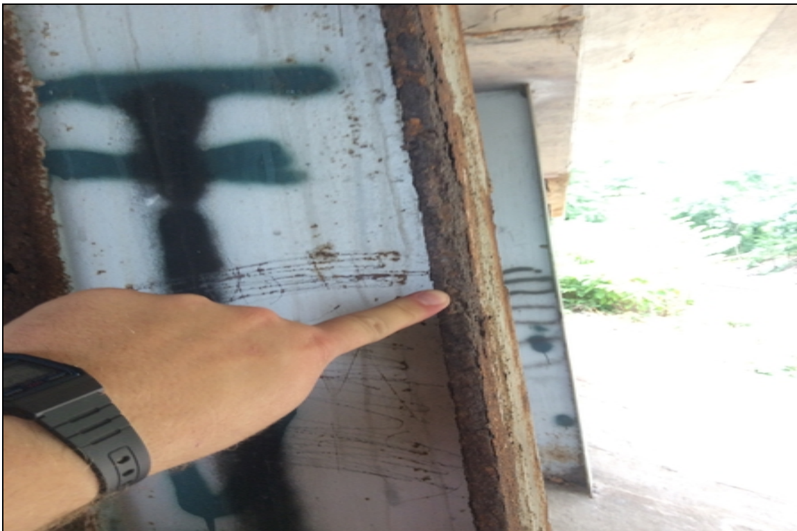
Bent 3 piling number 4 has active corrosion with minor section loss.
