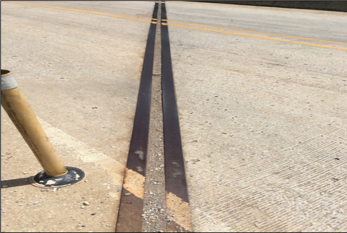
Bent 2 joint material has debris impaction
