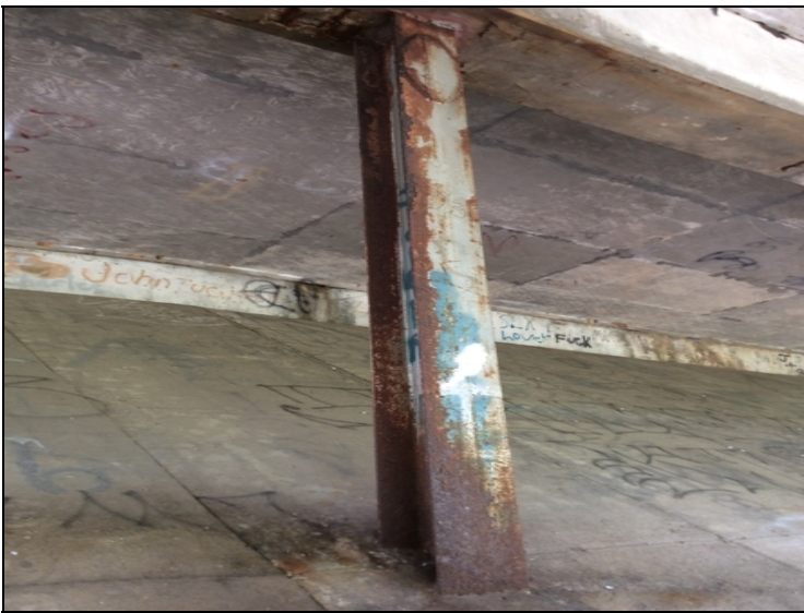
Bent 4 piling 4 - active corrosion and pitting.
