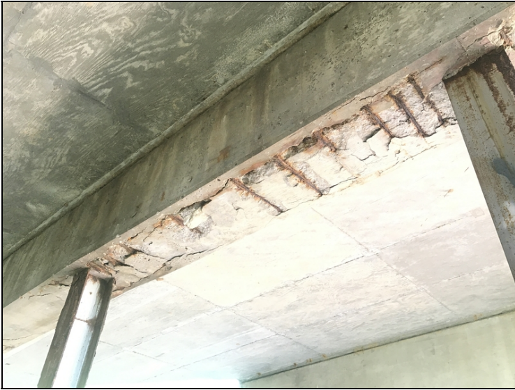
Bent #3 cap undersurface spalling with steel exposed section lose present in steel.
