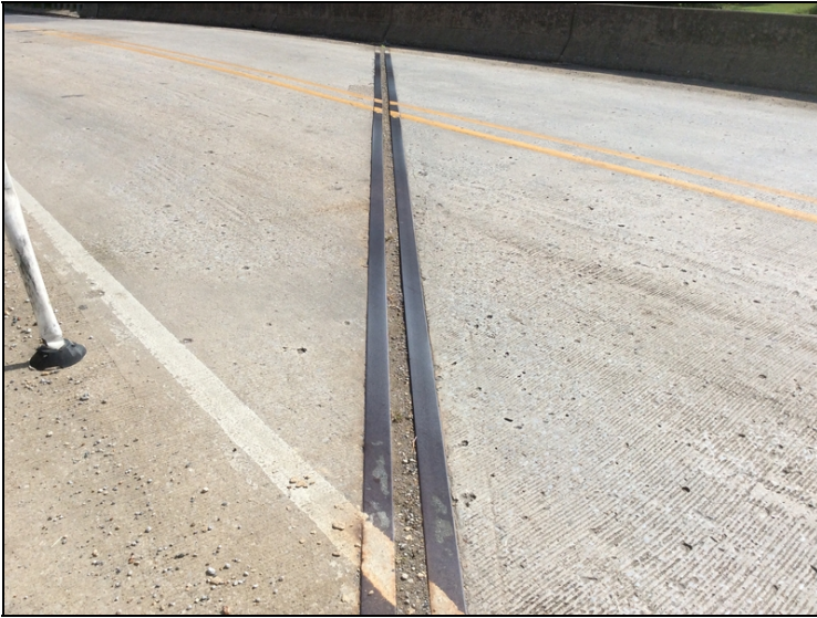
Deck joint bent 2 - debris impaction.
