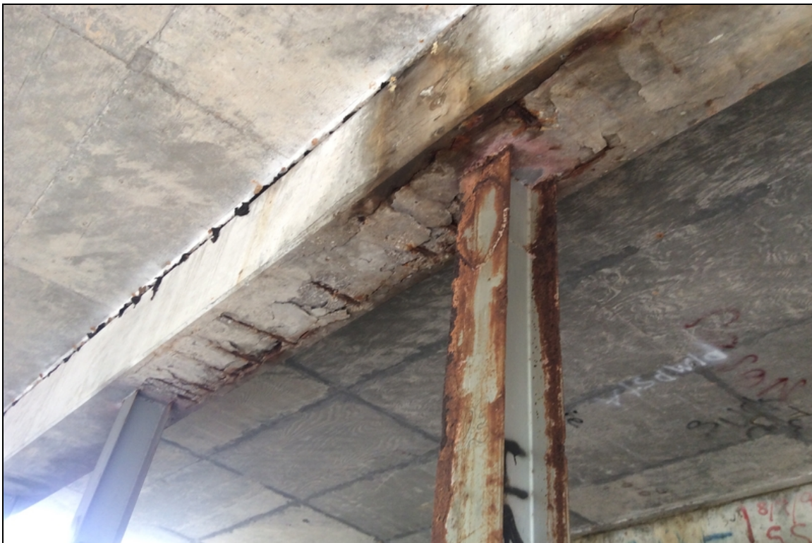
Bent 3 cap between steel piling 3 and 4 has spalling with steel exposed.
