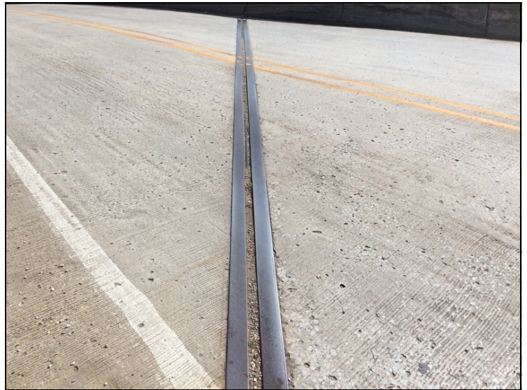
Deck joint bent 3 - debris impaction.
