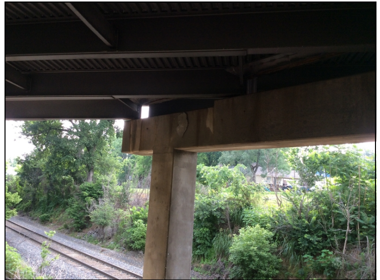
Bent 2 cap behind left - delaminated area.
