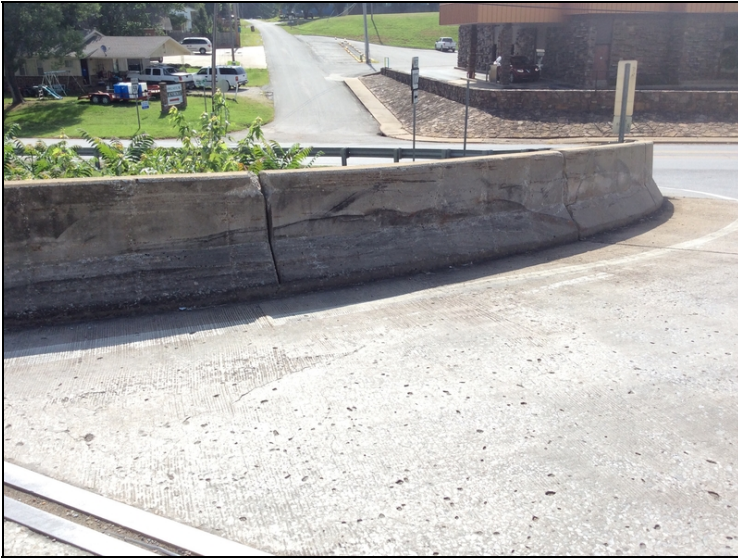
Concrete bridge railing span 4 left - collision marks.
