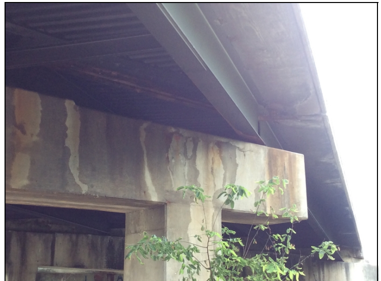
Bent 2 cap right behind - vertical cracking.
