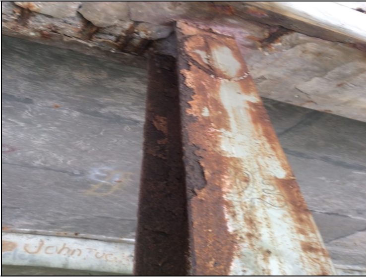
Bent 3 piling number 4 has active corrosion with minor section loss.
