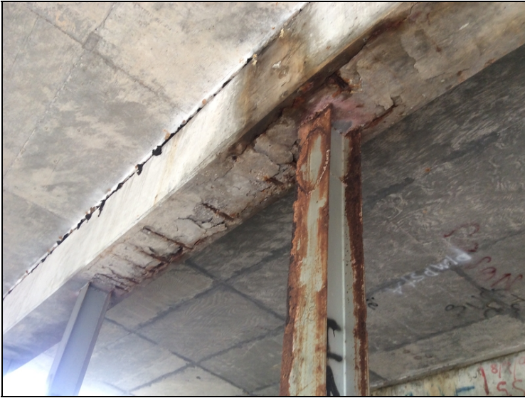
Bent 3 cap between steel piling 3 and 4 has spalling with steel exposed.
