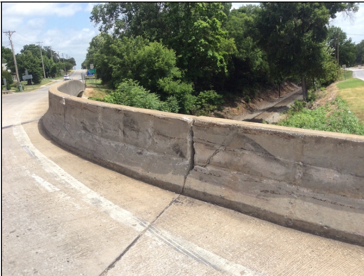
Railing left in spans 3 and 4 has Collision damage.
