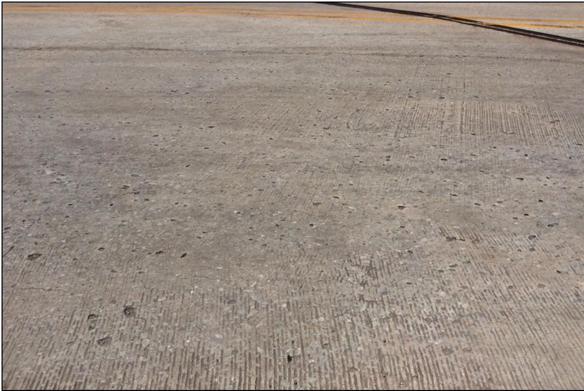
Span 3 left lane typical view of map cracking.
