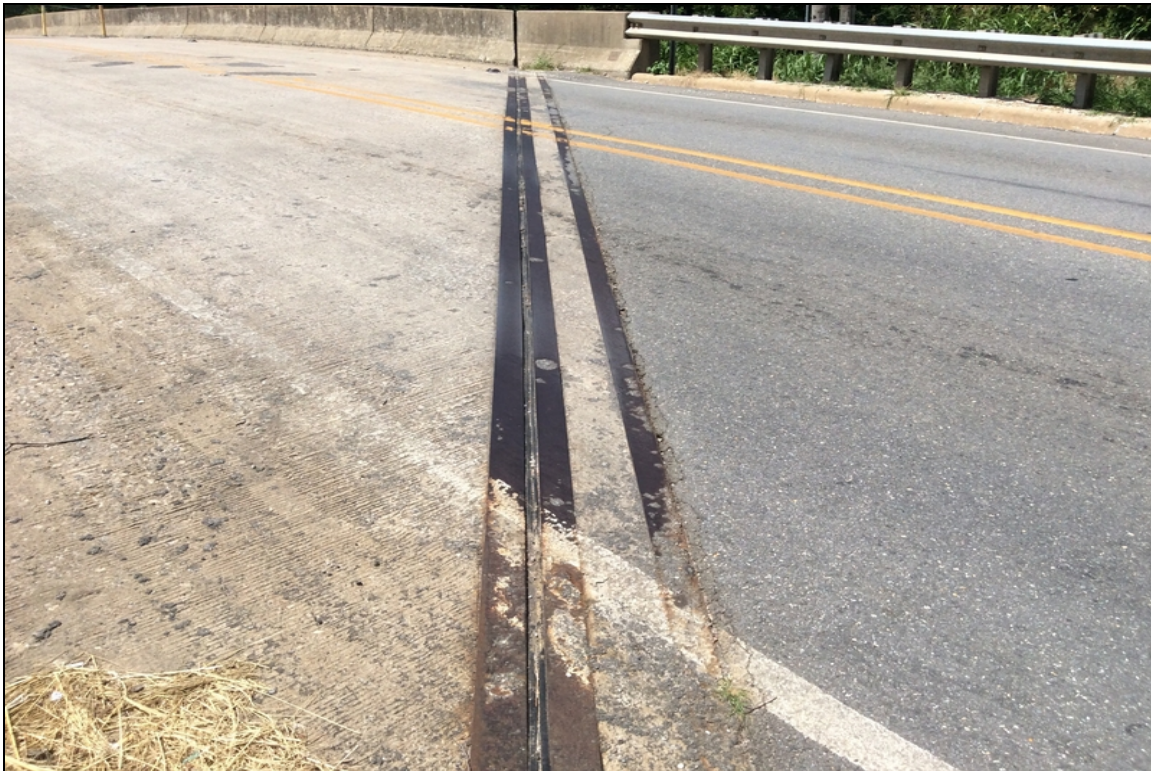
General view of abutment 1 joint material.
