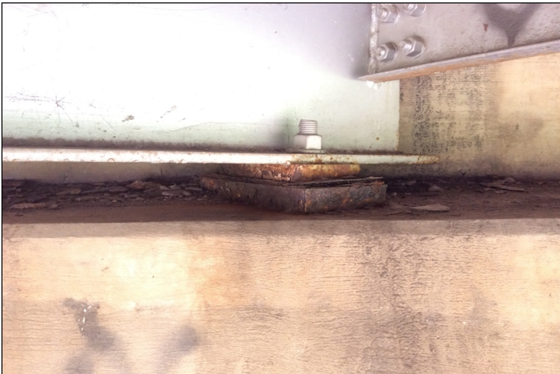
Typical view of bearing corrosion.
