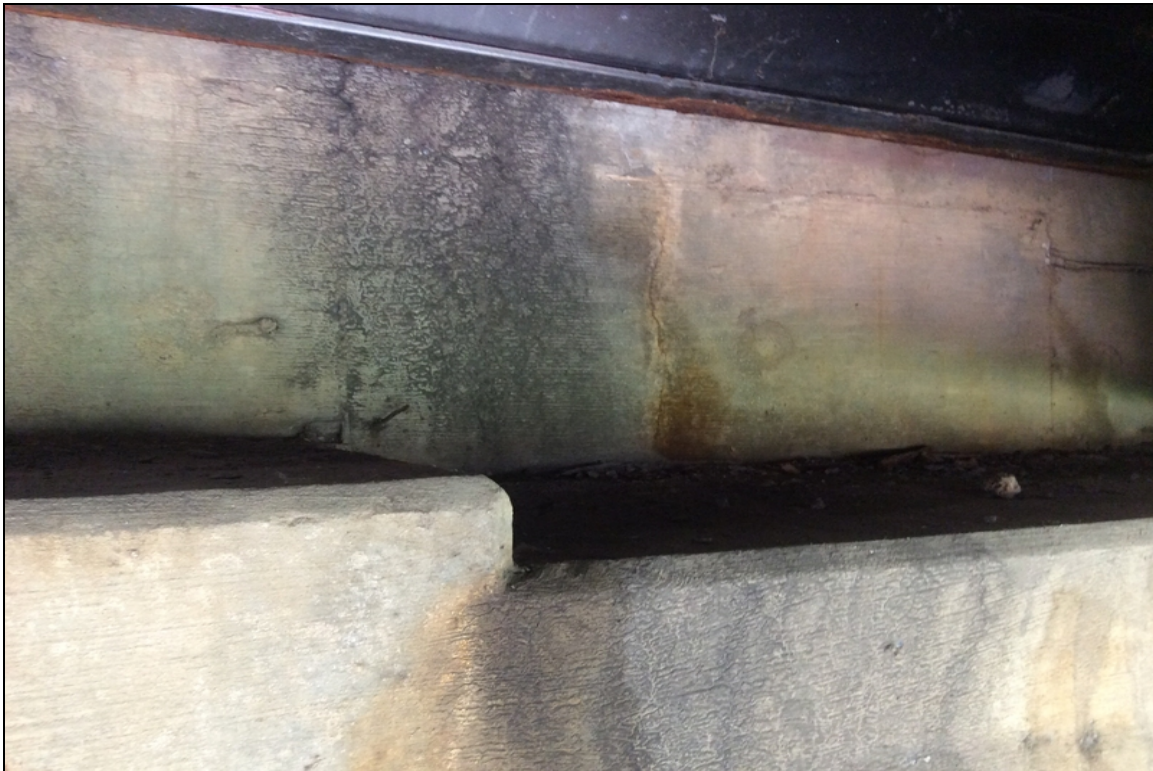
Abutment 1 bay 3 backwall has vertical cracking.
