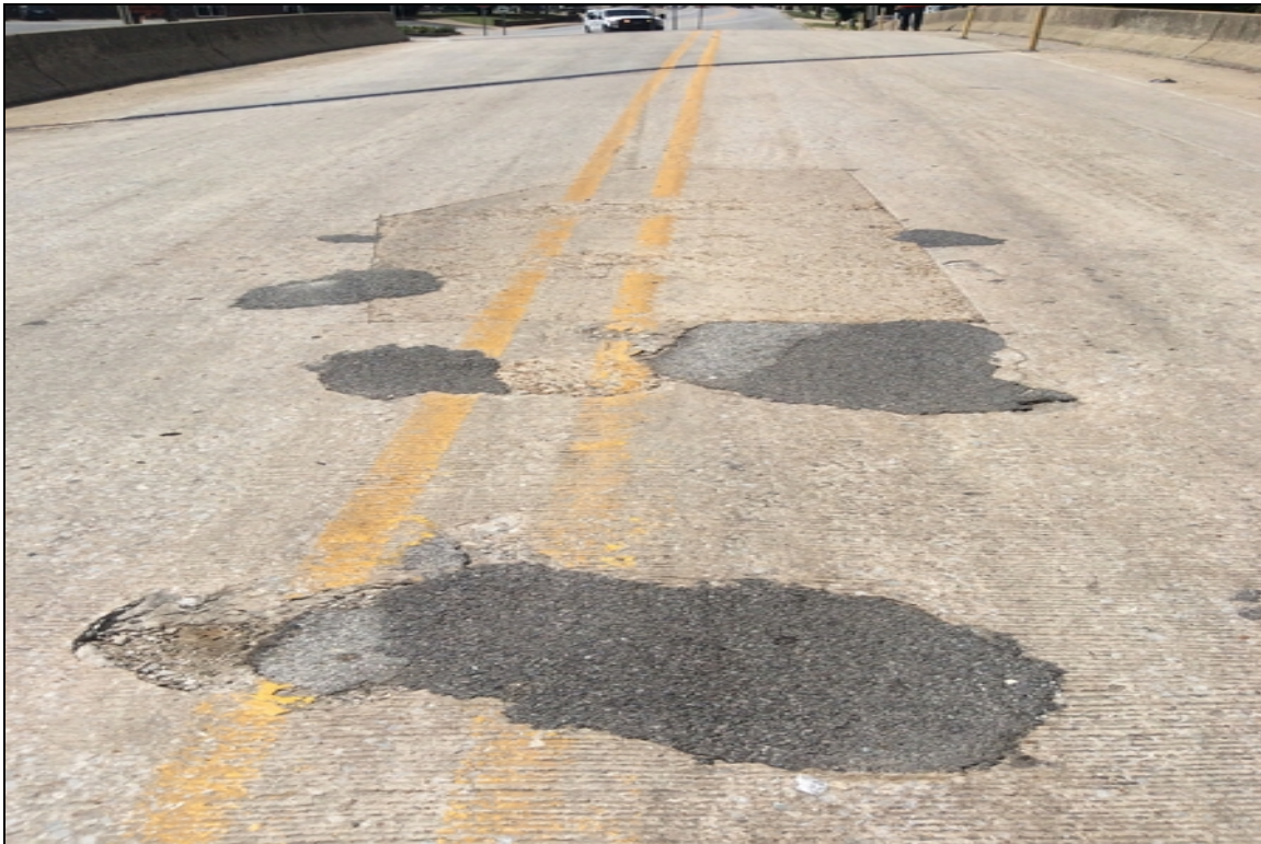
Span 1 has spalled patched areas.
