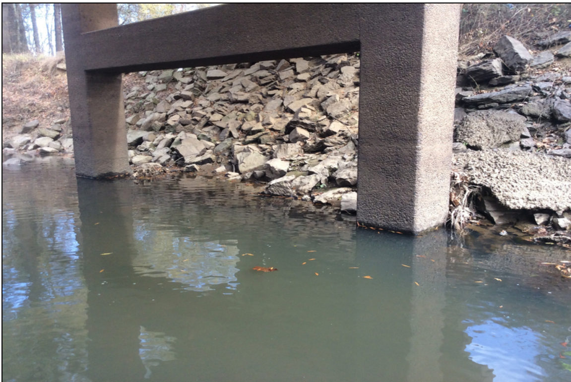
Columns at piers 3 and 4 has moderate abrasion below the R/C pier walls.
