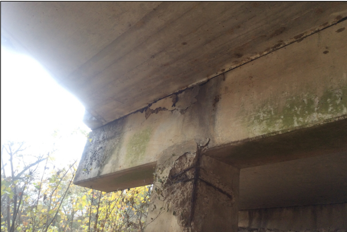
Right ahead side of pier #2 has moderate delam above column #2.
