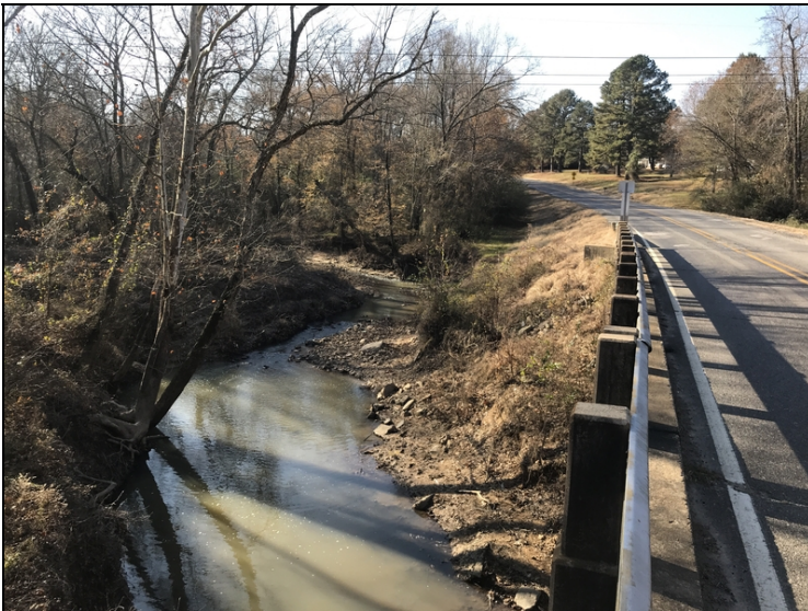
Embankment Erosion Behind Abutment 1 on Rt. (UP) Side. Channel on skew to Bridge.
