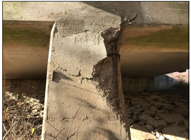
Delam, Cracking & Spalling W / Rebar Exposed in Column 2 at Pier 2.
