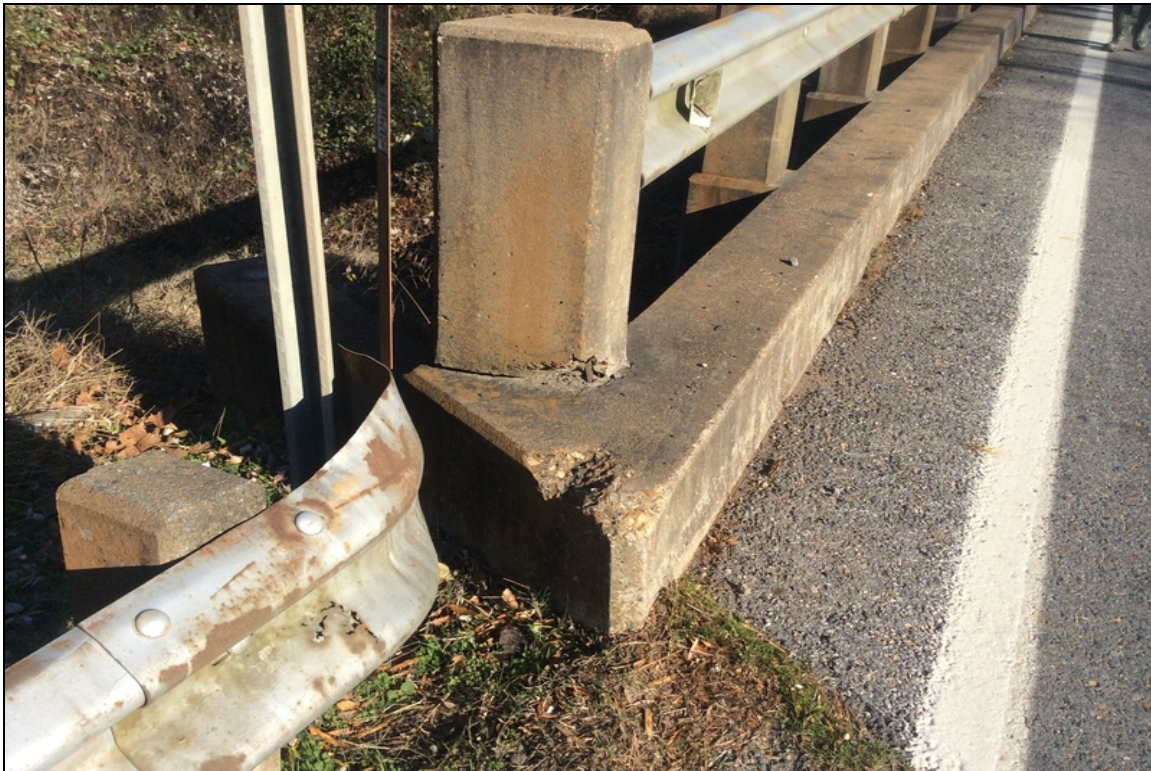
Left side post #1 has old impact damage.
