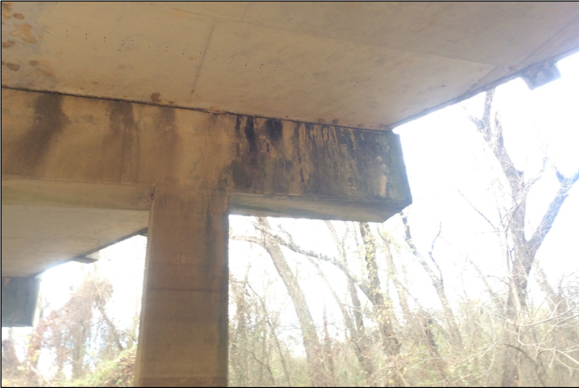
Pier #4 left ahead side has exposed rebar due to being too close to the surface.
