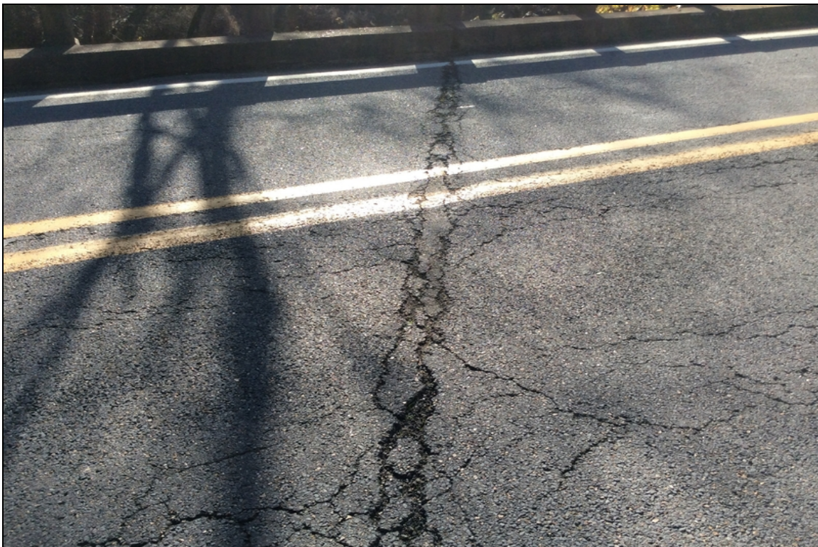
Joint #1 has complete debris impact (asphalt) the full length. All joints are typical.
