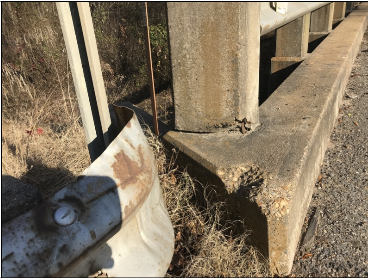
End Post at Abutment 1 Lt. Side Broken due to Impact.
