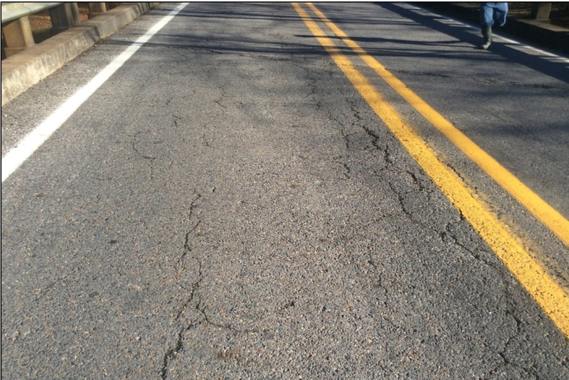
Moderate to large longitudinal cracks in wearing surface throughout.
