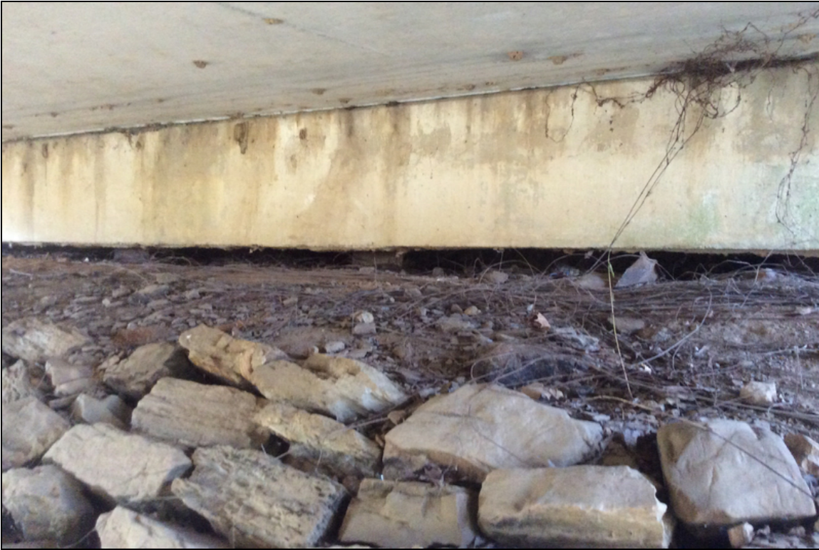
Piles are exposed at abutment #1 and have minor corrosion with minor section loss.
