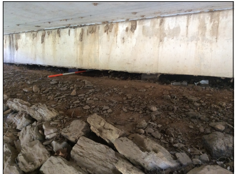
Abut. #1 - Erosion extends the full length of abutment and extends back 2 foot under abutment. All piles are exposed.
