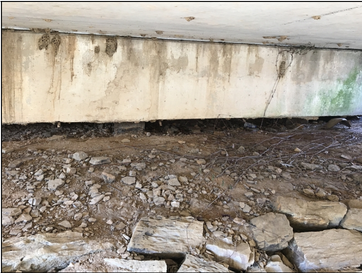
Erosion at Abutment 1.
