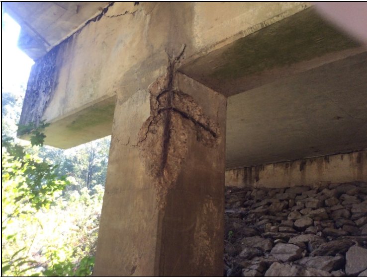
Pier #2, column #2 - Ahead side has major spall with rebar exposed, rebar has section loss. Cond. 3 for spall.
