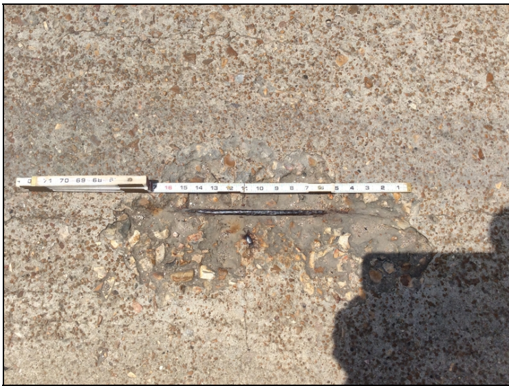
Exposed rebar in span #1 right whiteline
