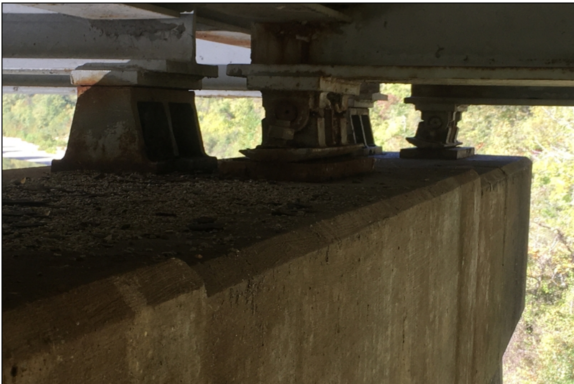
Bearing 5 tilt at the end of span #1.
