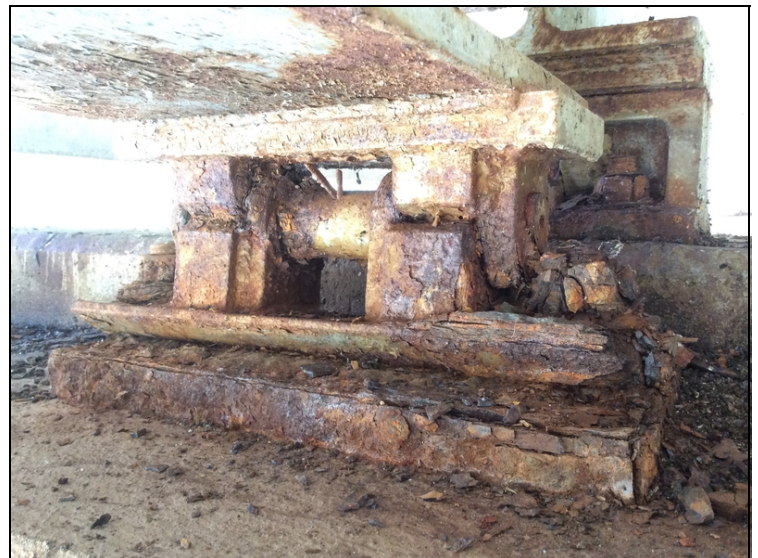
Corrosion to moveable bearings.
