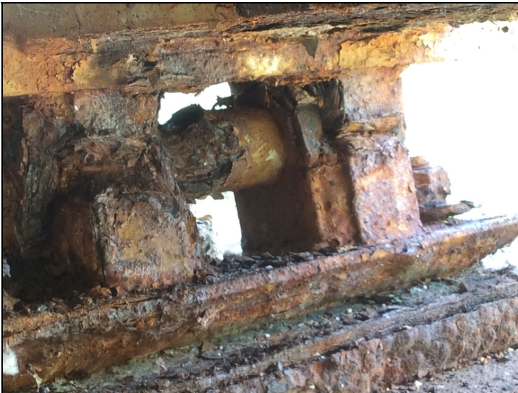
Corrosion to moveable bearings.
