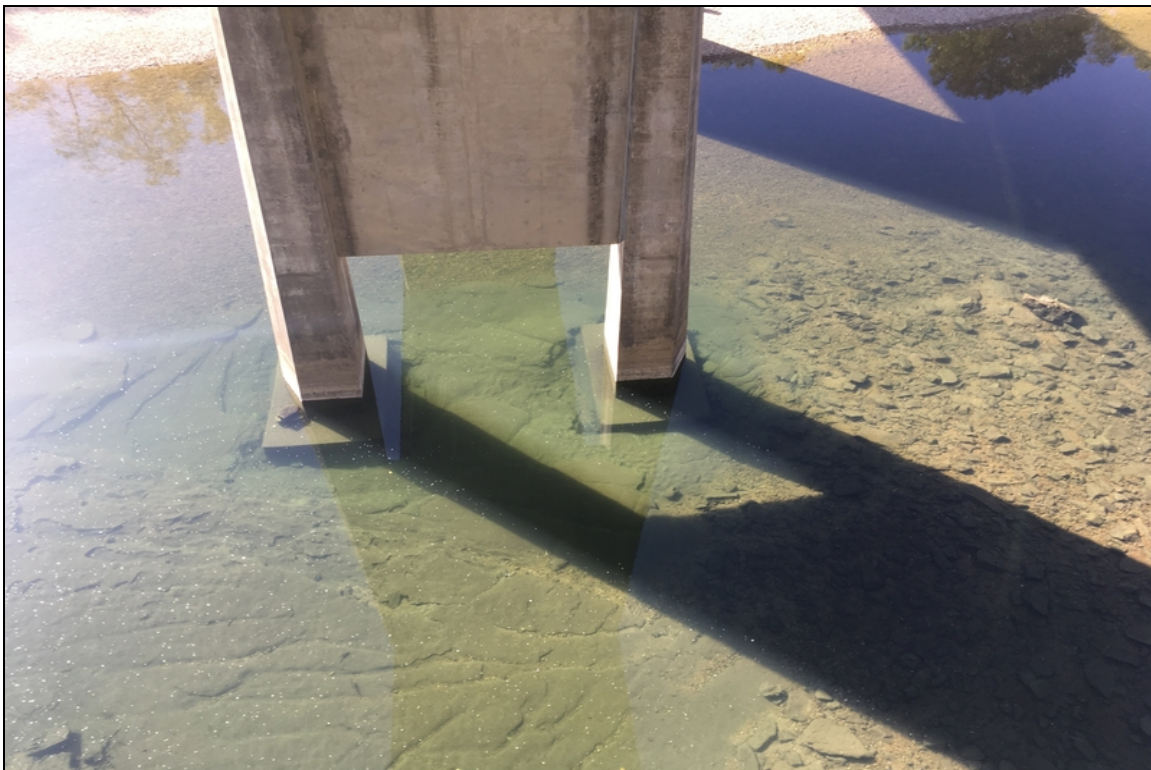
Exposed footings at the pier #2 columns.
