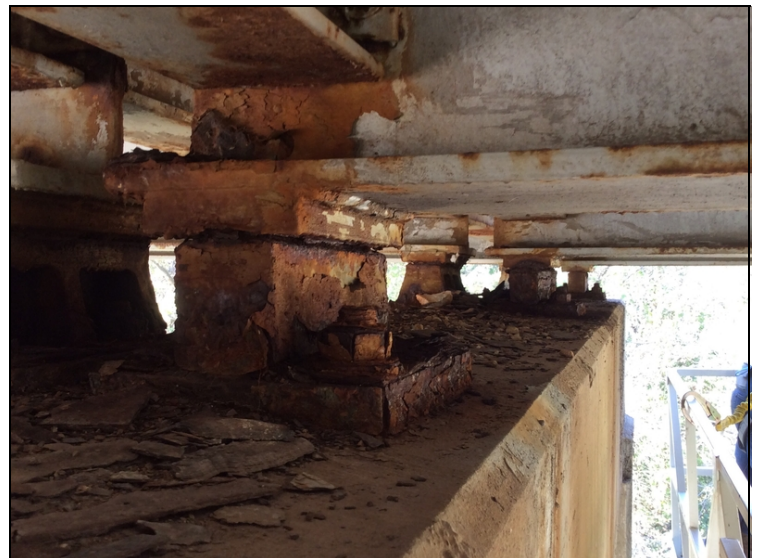
Corrosion to beam ends and bearing devices.
