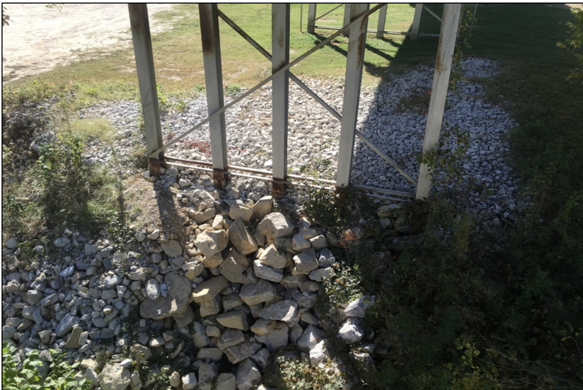
Repaired scour area around steel bent #4 is still holding at the 2020 inspection.
