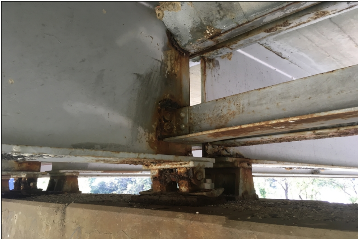
Beam end condition at the end of span #2.
