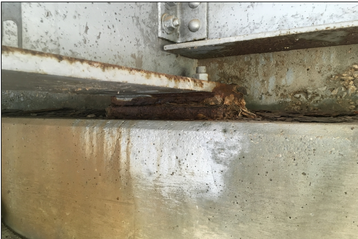
Abutment #1 bearing corrosion. Typical except bearing #4.
