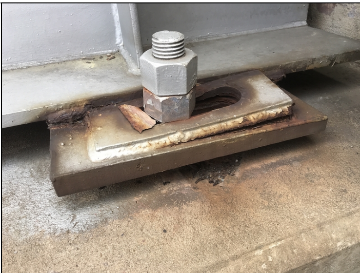
Bent 6, girder 4: weld broke due to pack rust
