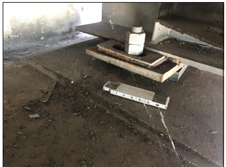
Pack rust has swelled between the bearing and the bottom flange, causing the welded connection to break. North abutment girder 1.
