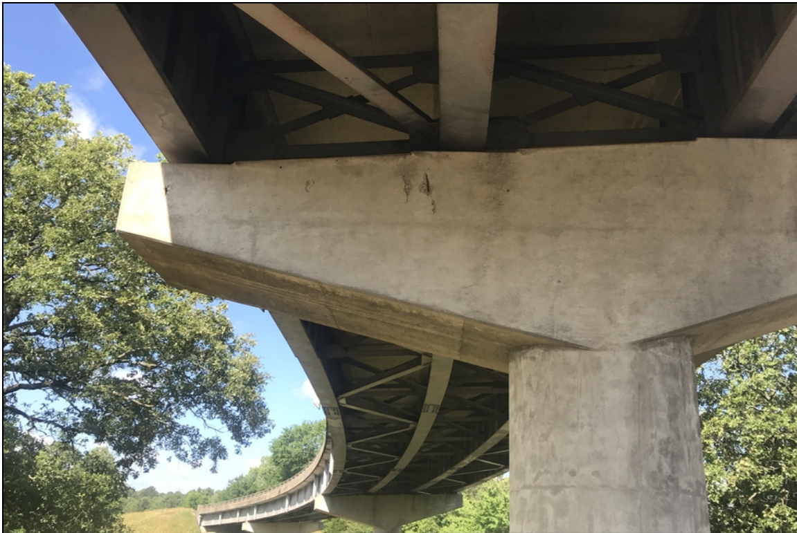
Bent 3 small spalls with exposed rebar on cap
