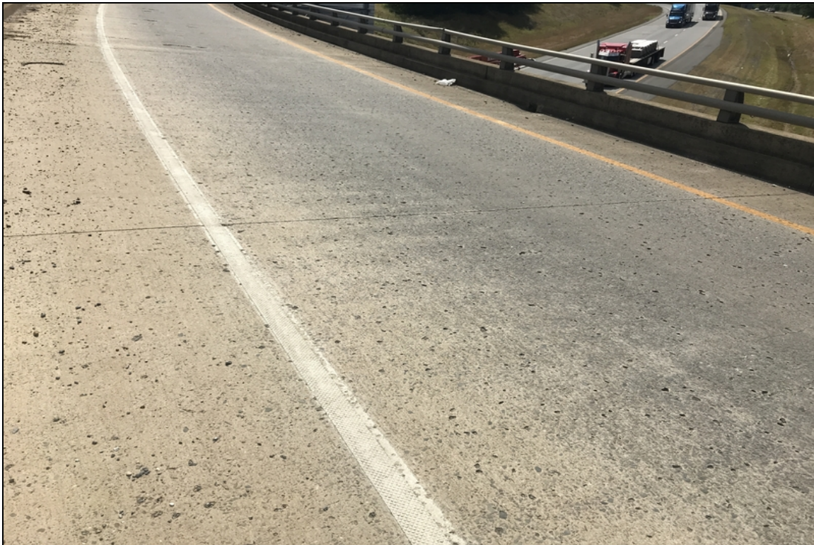
Span 3 abrasion
