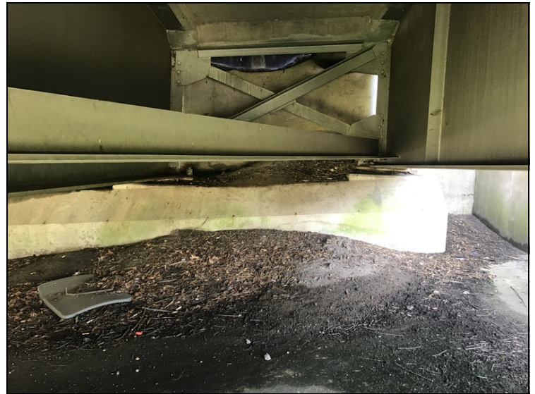
Bent 6, debris on the beam seat and beam ends due to open joint.
