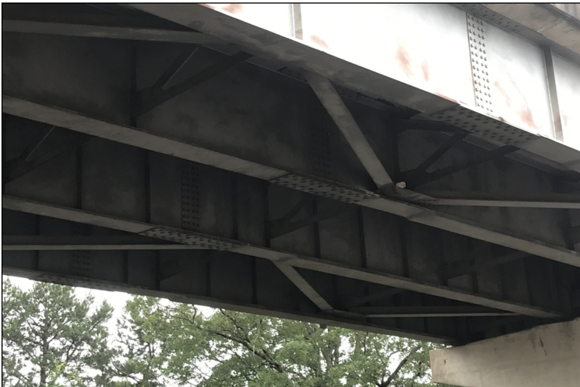
Span 4, girder 2 left side, at diaphragm 3: moderate sized piece of concrete is sitting on top of the diaphragm gusset about to fall off. This chunk of concrete is above I-40 west bound left lane.
