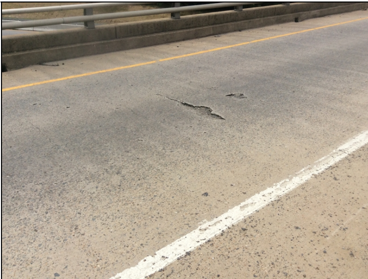
Spall in he deck at span 1.
