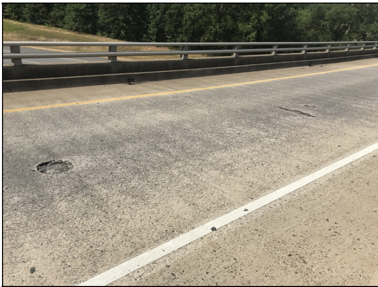
Span 5: large open spalls with exposed rebar in the deck surface
