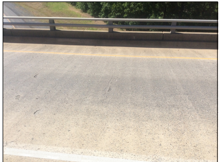
Span 5 transverse unsealed cracking up to 1/8" on three to four foot centers. Common in all spans.
