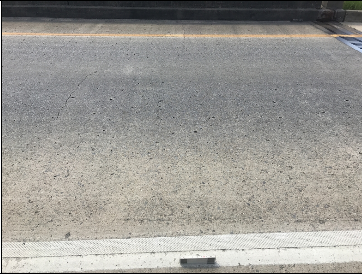
Typical deck cracking
