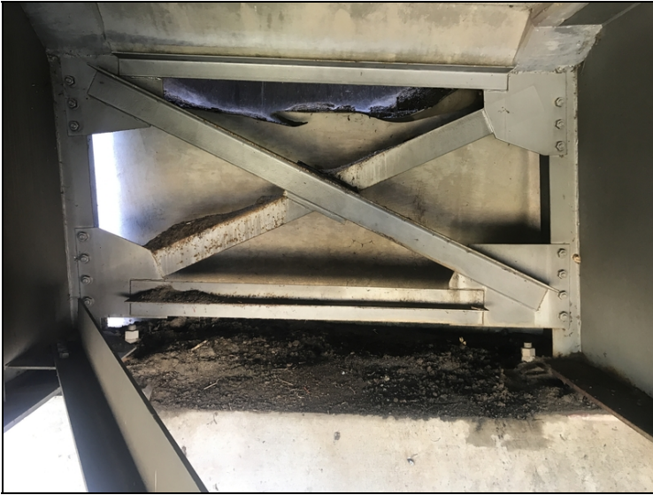
Bent 1: joint seal is open allowing debris to rest upon beam seat and bearings between girders 1 & 2. Similar condition at opposite abutment.
