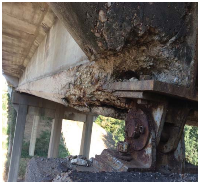
PHOTO 4 Description Typical spalls and cracking to Girder 1, 2 & 5 @ end of Span 3.
