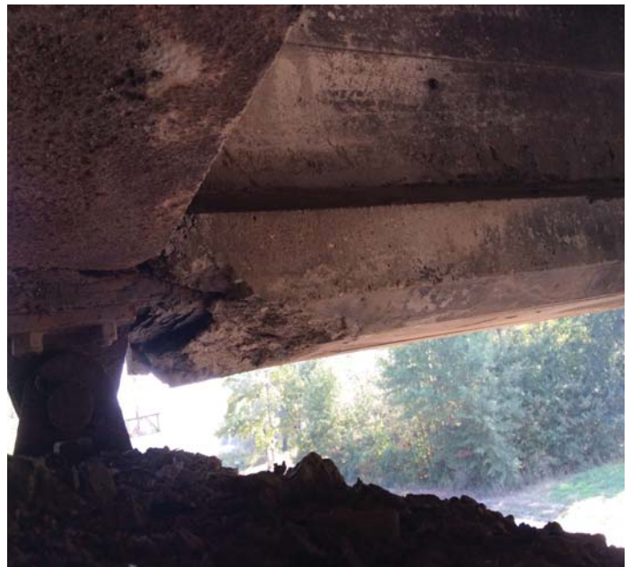
PHOTO 2 Description Typical condition of ends of all Girders @ beginning of Span 3.
