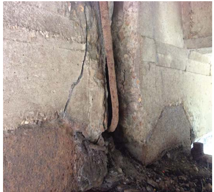
PHOTO 5 Description 100% Section Loss to Rebar @ End of Girder 3 @ Span 4.
