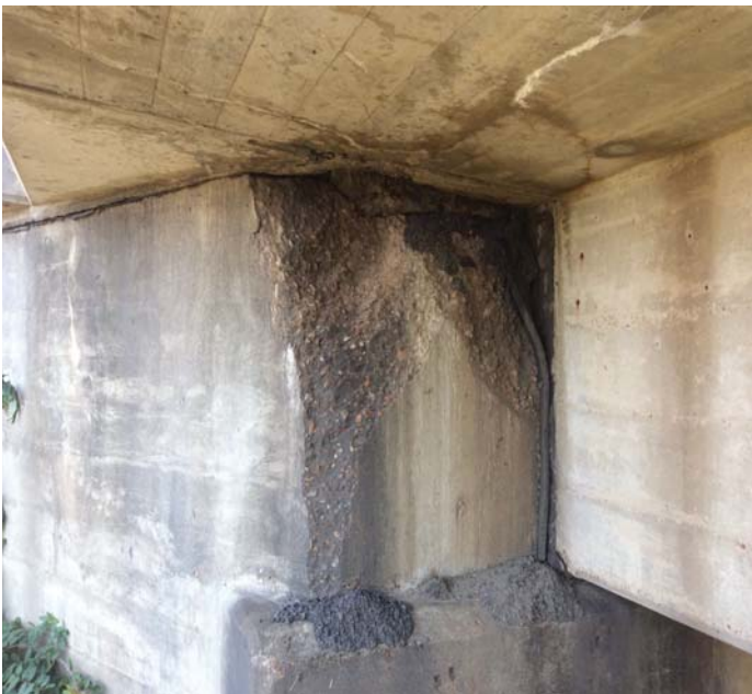
PHOTO 1 Description Spalls with Rebar Exposed to Left & Right ends of Abutment 1.
