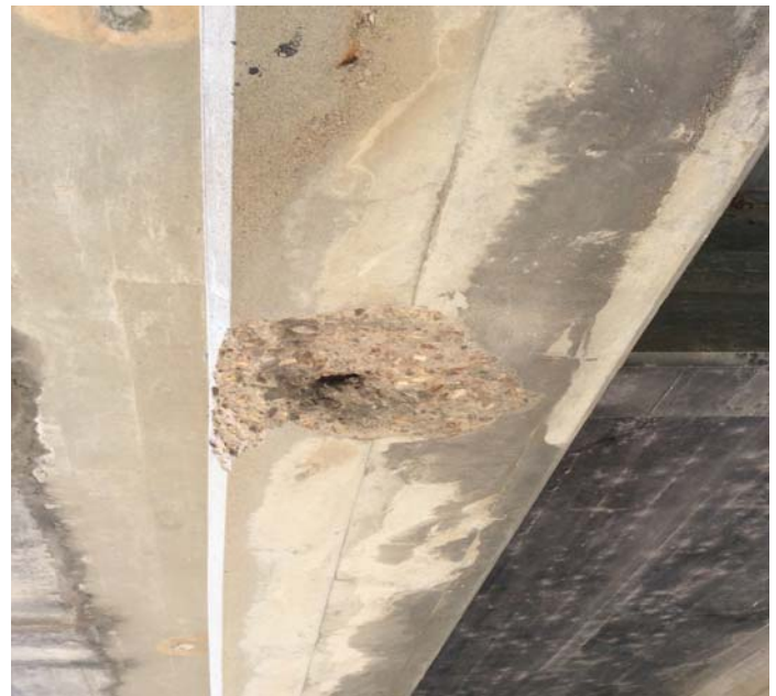
PHOTO 6 Description Girder 3 @ Span 4 has Spall with 4" Rebar Exposed.
