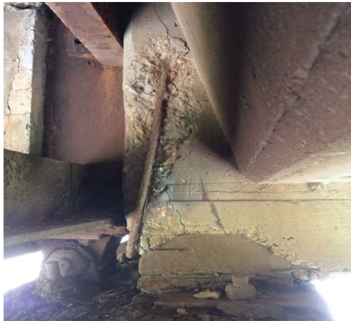
PHOTO 3 Description Spall with large area of Rebar Exposed to Girder 2 @ beginning of Span 4, Typical condition of Girders 2 & 3.
