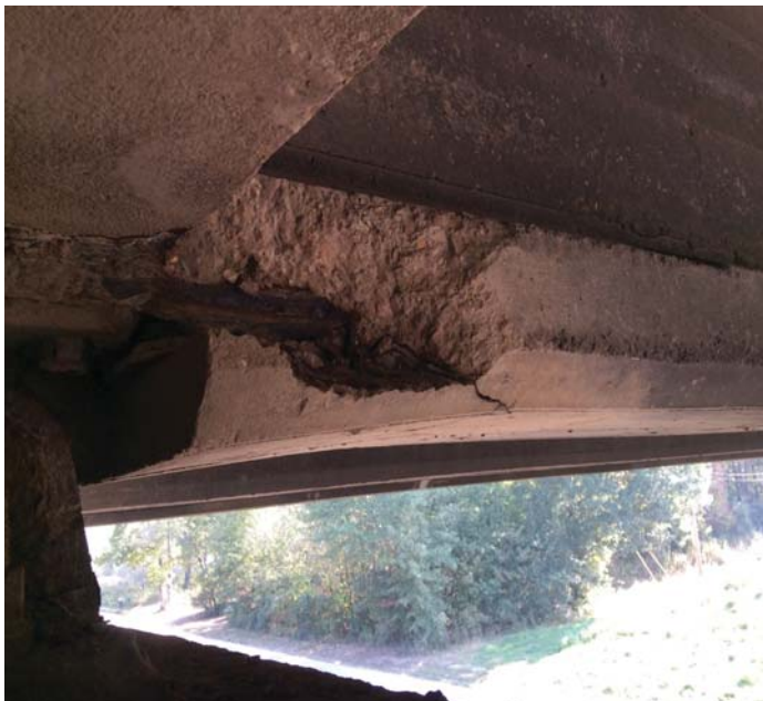
PHOTO 1 Description Typical condition of ends of all Girders @ beginning of Span 3.
