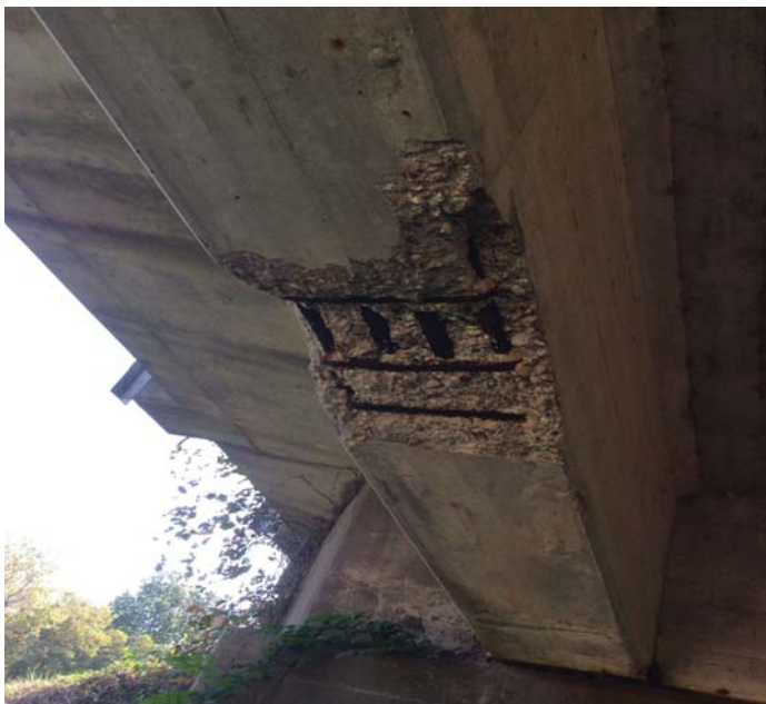
PHOTO 7 Description Girder 1 @ Span 5 has large spall with 5' rebar exposed near mid span.
