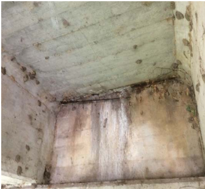
PHOTO 1 Description Typical exposed rebar in soffit
