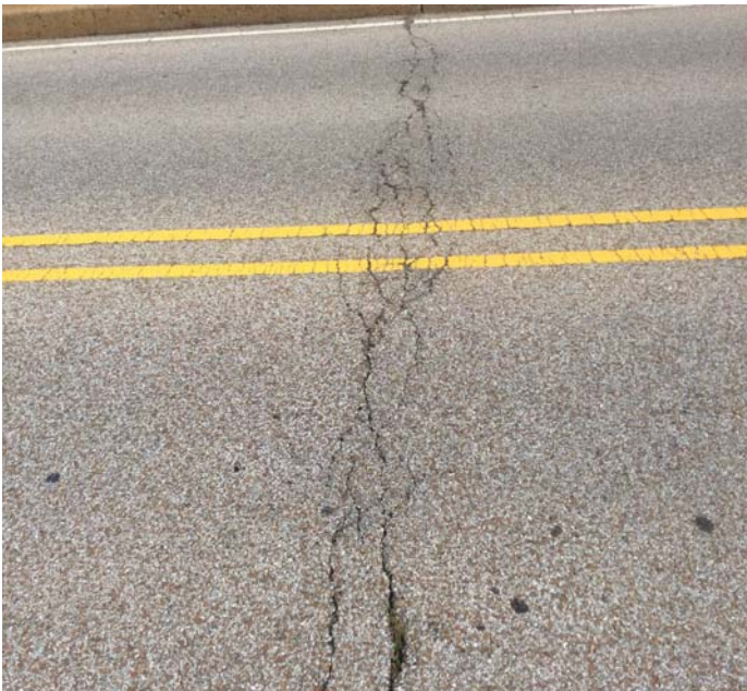
PHOTO 1 Description Typical cracks in asphalt at joints.
