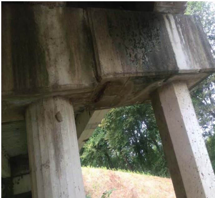
PHOTO 1 Description Typical spall bottom of cap.
