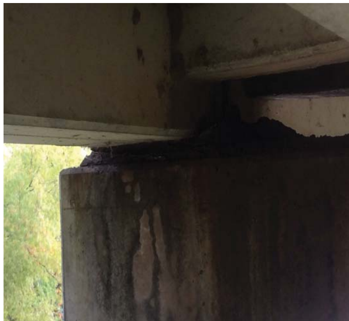
PHOTO 1 Description Typical bearings on outside girders.
