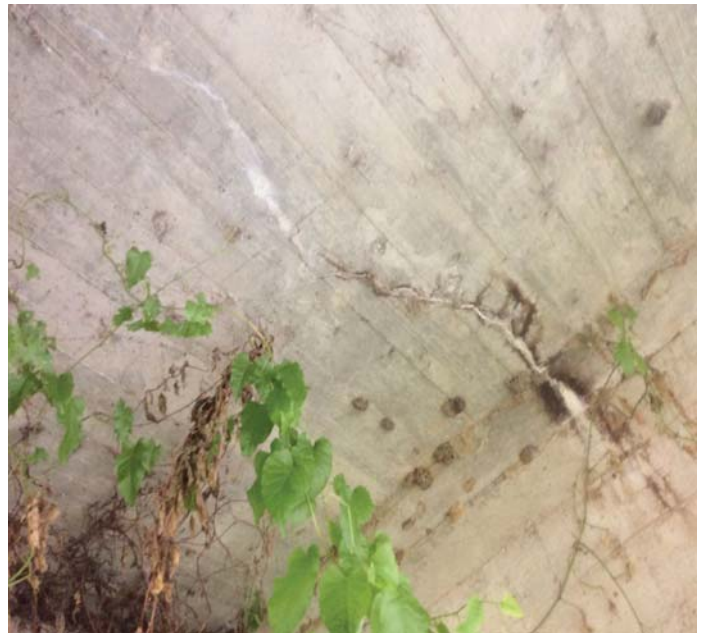
PHOTO 2 Description Typical soffit crack with efflorescence.
