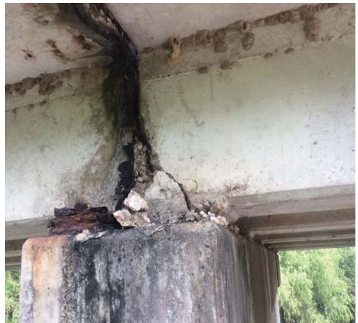
PHOTO 2 Description Typical girder end spalled.
