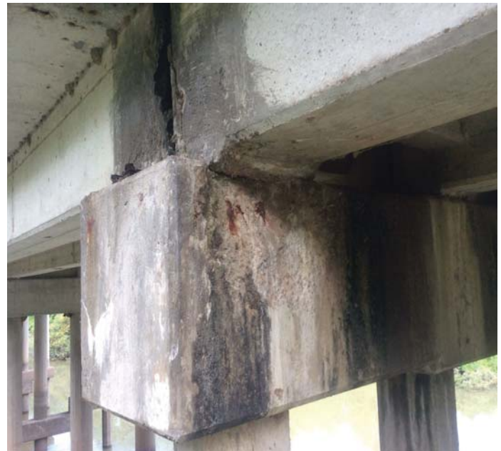
PHOTO 2 Description Bent 13 cap ahead face right end 2' spall under bearing area 6
