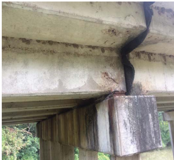
PHOTO 1 Description Typical light spalling on girder ends.
