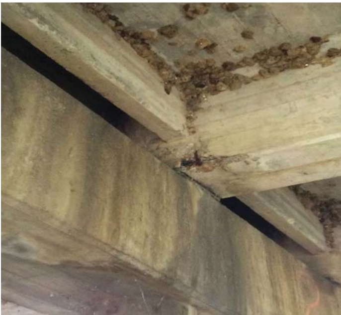
PHOTO 1 Description Cracks, delaminating &/or spalls with rebar exposed to concrete girders at Spans 2 - 7.
