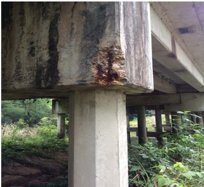
PHOTO 1 Description Bent 2 Right Side. Cracks, delaminating &/or spalls with rebar to caps at Bents 2 - 6.
