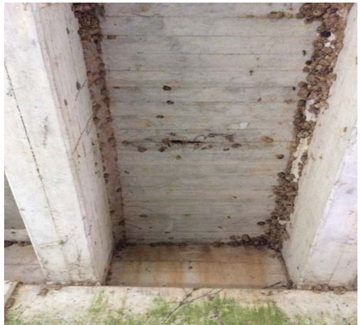
PHOTO 2 Description Span 3. Spall with corroded rebar exposed to deck below at Spans 2 & 3.
