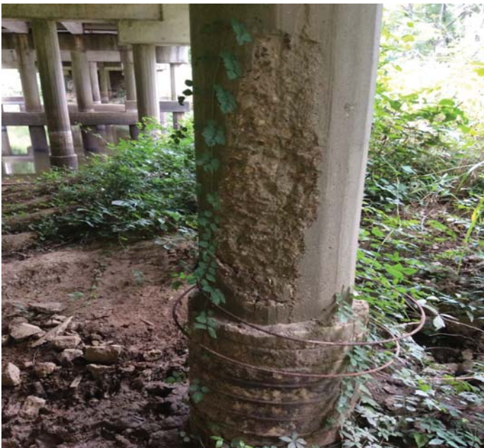
PHOTO 1 Description Large spall no rebar exposed to Pile 5 at Bent 2.
