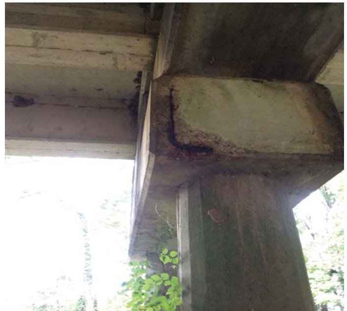
PHOTO 2 Description Bent 2 Right Side. Cracks, delaminating &/or spalls with rebar to caps at Bents 2 - 6.
