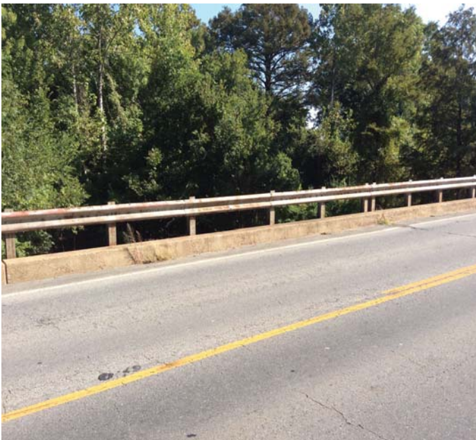
PHOTO 1 Description All Guard Rail is rusting & areas of peeling paint.
