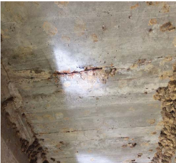
PHOTO 1 Description Spalls with rebar exposed to Deck below @ Spans 1, 2, 3, 4, 6, 7 & 8.
