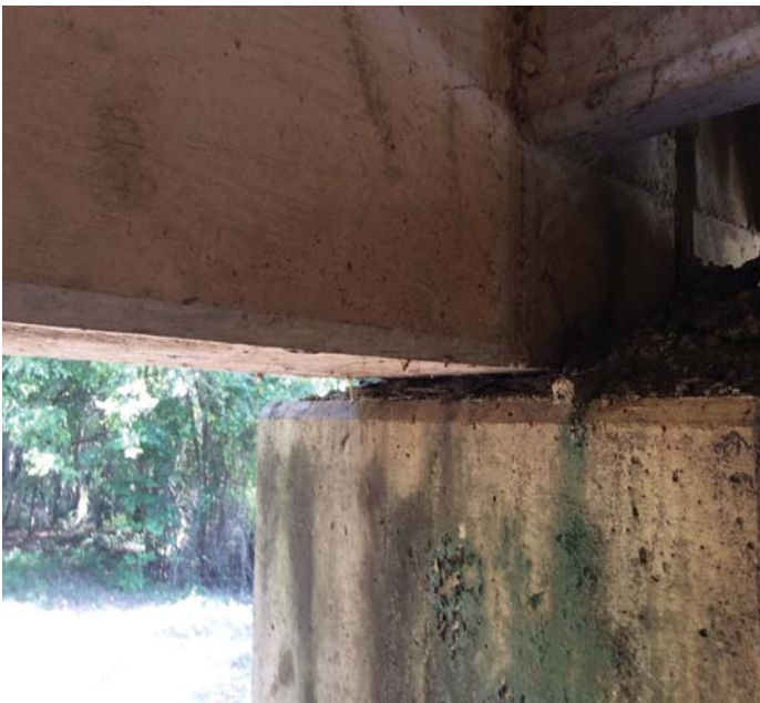
PHOTO 1 Description Rust & section loss to Bearings 1 & 6 @ Bents 2, 4 & 6
