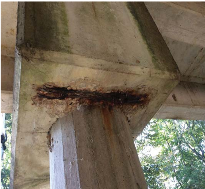
PHOTO 1 Description Spalls with rebar exposed to Caps @ Bents 1, 2, 3 & 6.
