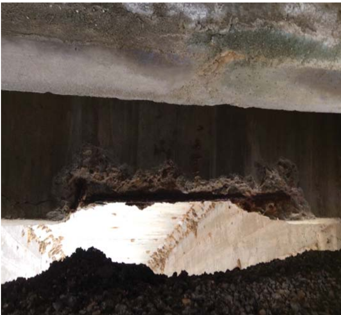
PHOTO 1 Description Spalls with rebar exposed to Concrete Diaphragms @ Spans 2, 4, 5, 6, 7 & 8.
