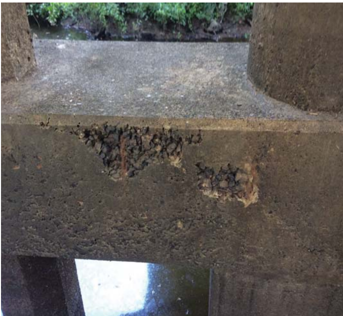
PHOTO 1 Description Bent 4 has Large honeycomb area with 6" rebar exposed to back side of Sub Cap between Pile 1 & 2.
