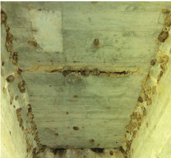
PHOTO 1 Description Spalls with rebar exposed to deck below at Spans 2, 6 & 10.
