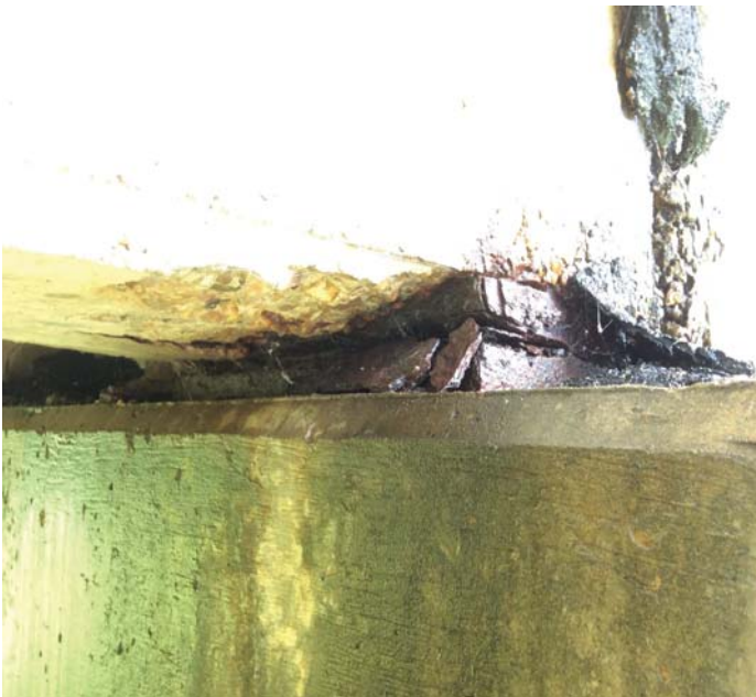
PHOTO 1 Description Rust & pitting with section loss to moveable Bearings 1 & 6 at Bents 2, 4, 6, 8, & 10.
