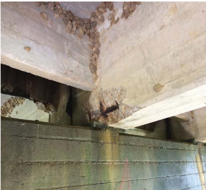
PHOTO 1 Description Spalls with rebar exposed to Girders at Spans 2, 3, 4, 5, 6, 7, 8, 9 & 11.
