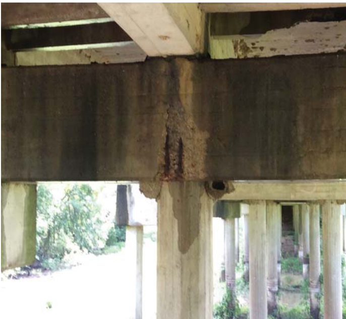
PHOTO 1 Description Spalls with rebar exposed to cap at Bents 4, 5, 6, 8, 9 & 10.
