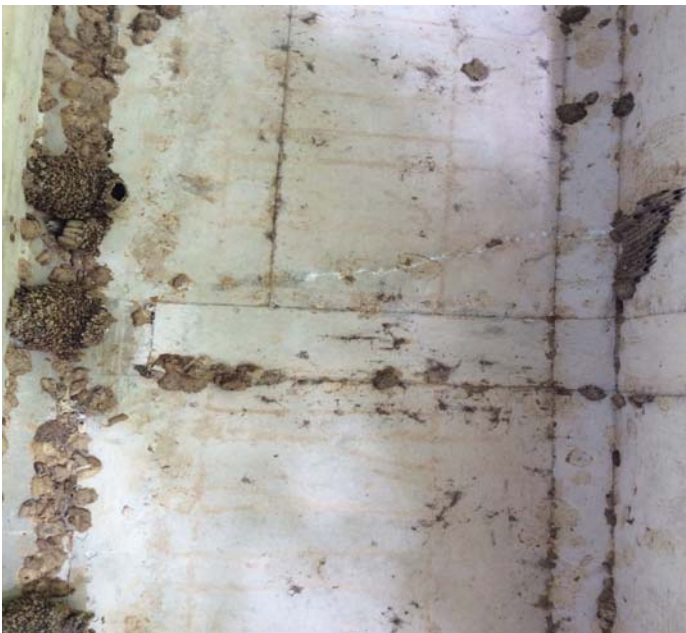
PHOTO 1 Description Transverse cracks, some with rust stains, to deck below & to girders at all Spans
