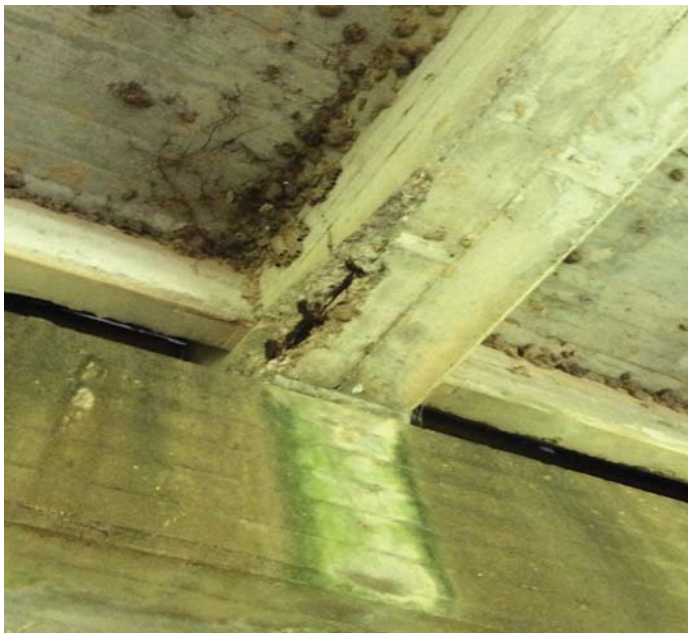
PHOTO 1 Description Cracking, delaminating &/or spalls with rebar exposed to end of girders & concrete diaphragms at all Spans.
