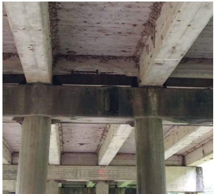
PHOTO 2 Description Cracking, delaminating &/or spalls with rebar exposed to ends of girders & concrete diaphragms.
