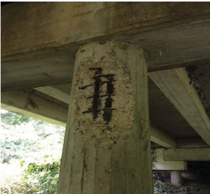
PHOTO 1 Description Large spall with 3.5' rebar exposed to Pile 4 at Bent 2.
