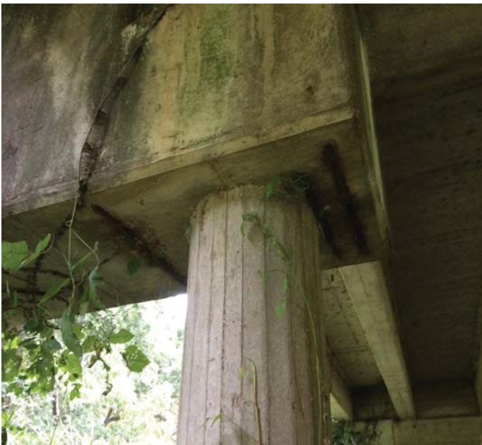
PHOTO 1 Description Spalls with rebar exposed to caps at Bents 2, 3, 6, 7, 8, 9, 10, 11, & 12.
