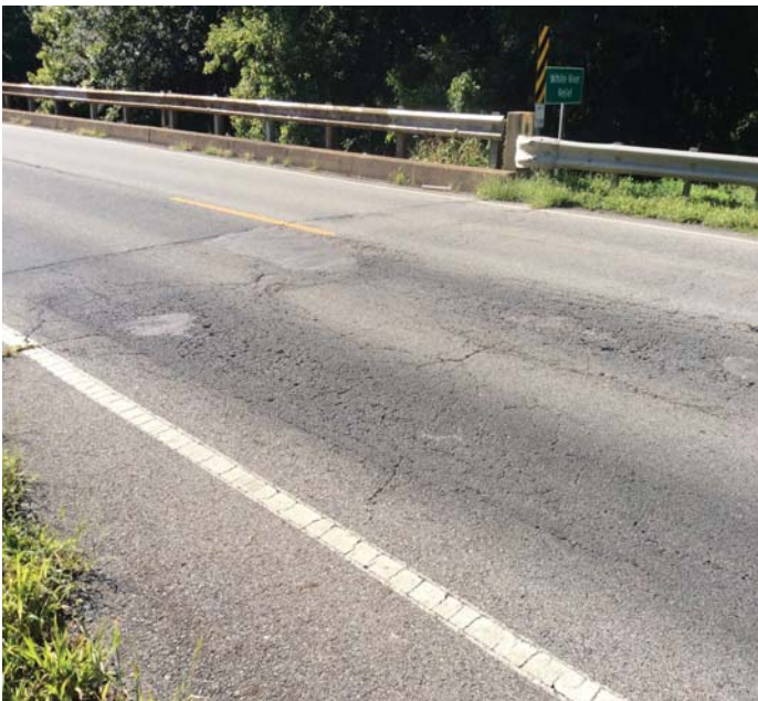
PHOTO 1 Description Visual settlement to approach roadway at Abutments 1 & 2.
