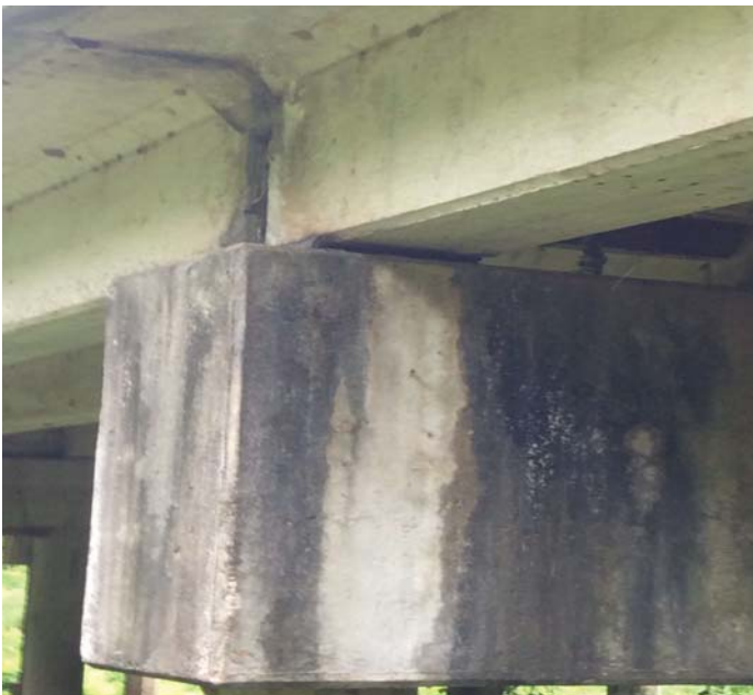
PHOTO 1 Description Rust & corrosion to Bearings 1 & 6 at Bents 2, 4, 6, 8, 10, & 12
