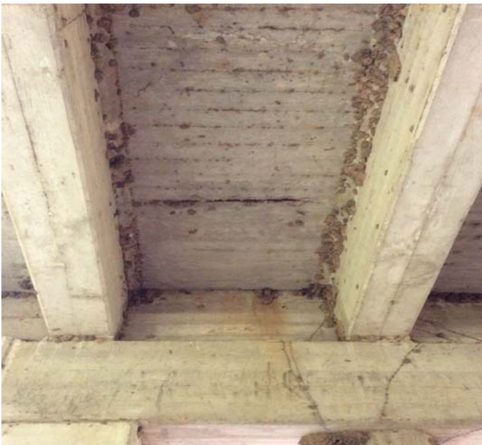
PHOTO 1 Description Spalls with rebar exposed to deck below at Spans 2, 3, 5, 6, 8, 9, 13, & 14.
