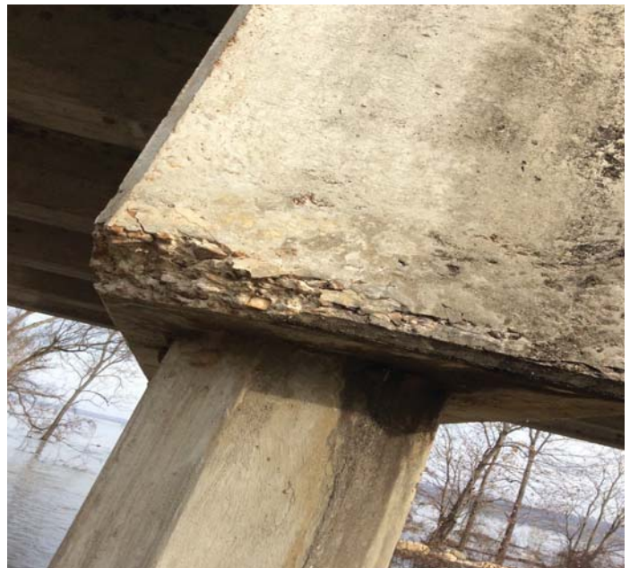
PHOTO 2 Description Typical spalls with Rebar Exposed or areas of delamination to some Caps @ Bents 1, 2, 4, 8, 10, 11 & 12. (Bent 3 @ Right end.)
