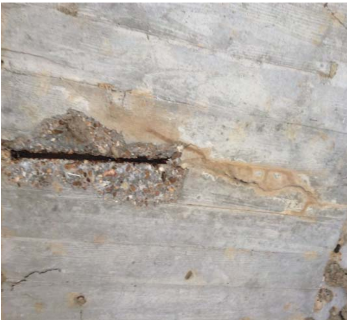
PHOTO 1 Description Typical spalls with Rebar Exposed to Soffit @ Spans 2, 8, 11 & 12.
