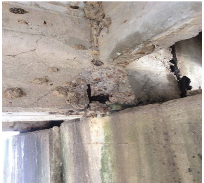
PHOTO 2 Description Spalls to Girders with Rebar Exposed @ Spans 1, 3, 4, 5, 6, 9, 10, 11 & 12. (Span 4 Girder 2 @ End of Span)
