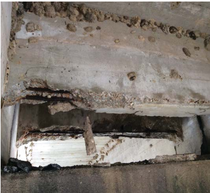
PHOTO 1 Description Spalls to Concrete Diaphragms with Rebar Exposed @ Spans 3, 4, 5, 8, 10 & 11. (Diaphragms between Girders 3 & 4 back & ahead side @ Bent 4.)
