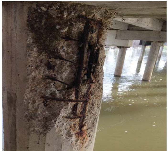
PHOTO 2 Description Typical spalls with Rebar Exposed to some Piles. (Bent 4 Pile 4 has large spall with 9' Rebar Exposed.)
