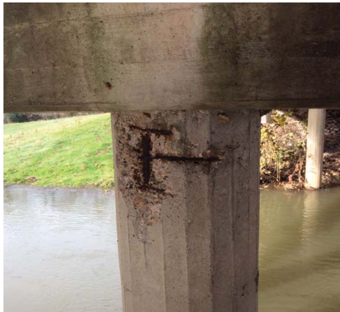
PHOTO 1 Description Typical spalls with Rebar Exposed to some Piles. (Bent 2 Pile 4)
