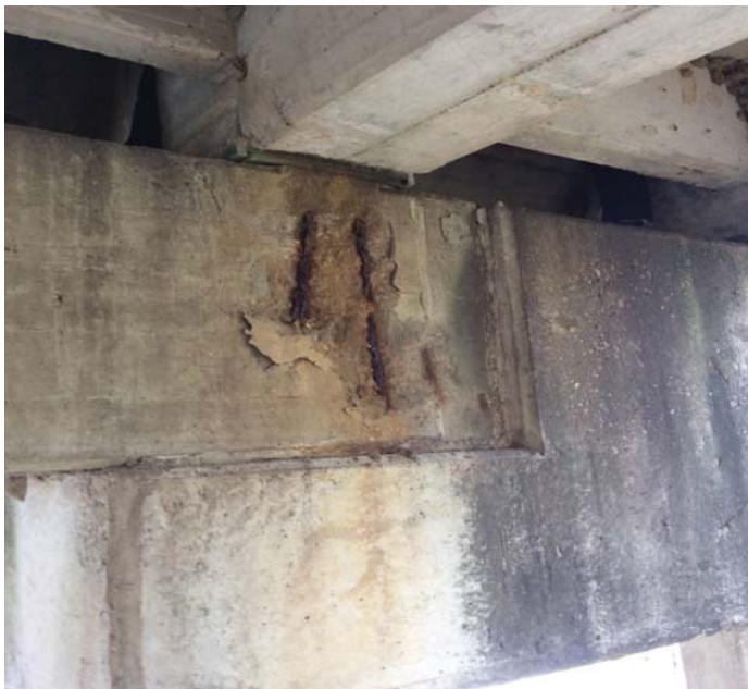
PHOTO 1 Description Typical spalls with Rebar Exposed or areas of delamination to some Caps @ Bents 1, 2, 4, 8, 10, 11 & 12. (Bent 2 back side)
