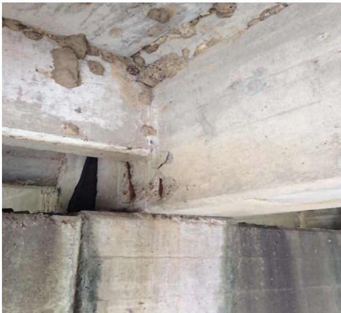
PHOTO 1 Description Spalls to Girders with Rebar Exposed @ Spans 1, 3, 4, 5, 6, 9, 10, 11 & 12. (Span 3 Girder 5 @ Beginning of Span)
