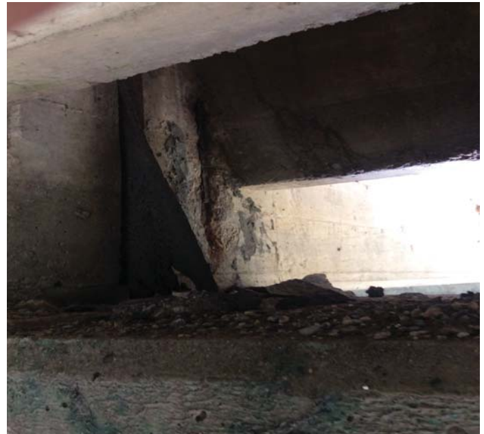
PHOTO 2 Description End of Girder 5 at Span 5. Cracking, delaminating &/or spalls with rebar exposed to girders at all spans.
