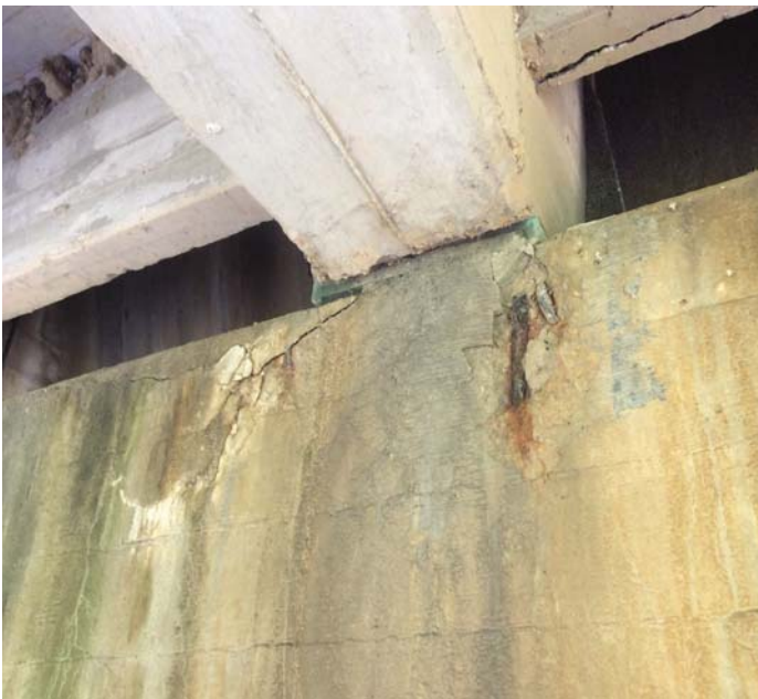
PHOTO 1 Description Cracks, delaminating &/or spalls with rebar exposed to caps at Bents 1 - 9.
