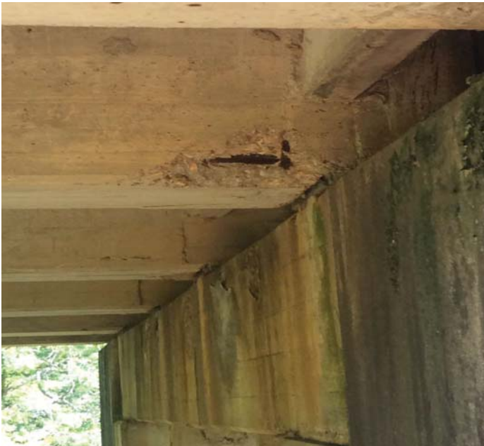
PHOTO 1 Description Bent 2 Girder 5 - Typical cracking, delaminating &/or spalls with rebar exposed to girders at all spans.
