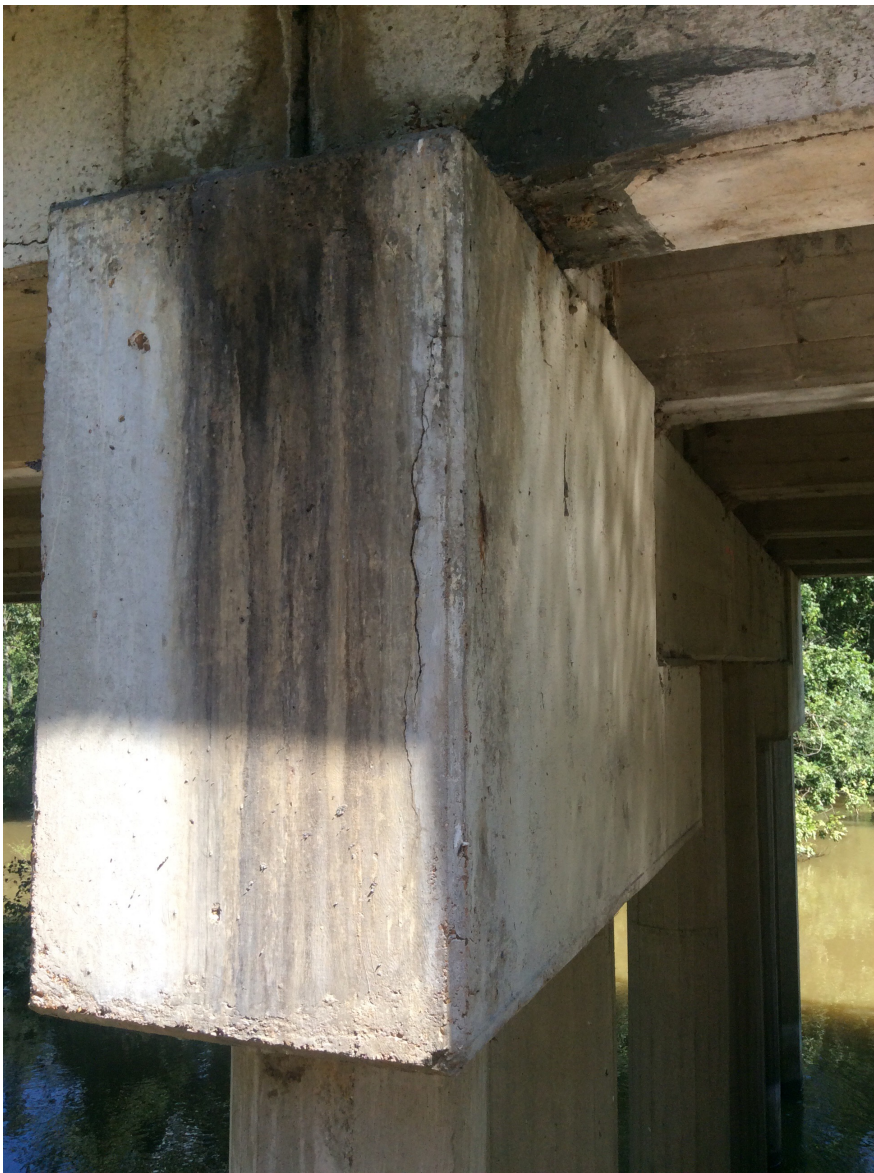
Bent 7 - typical of cracks, delamination, and spalls with rebar exposed to caps at Bents 1 through 9
