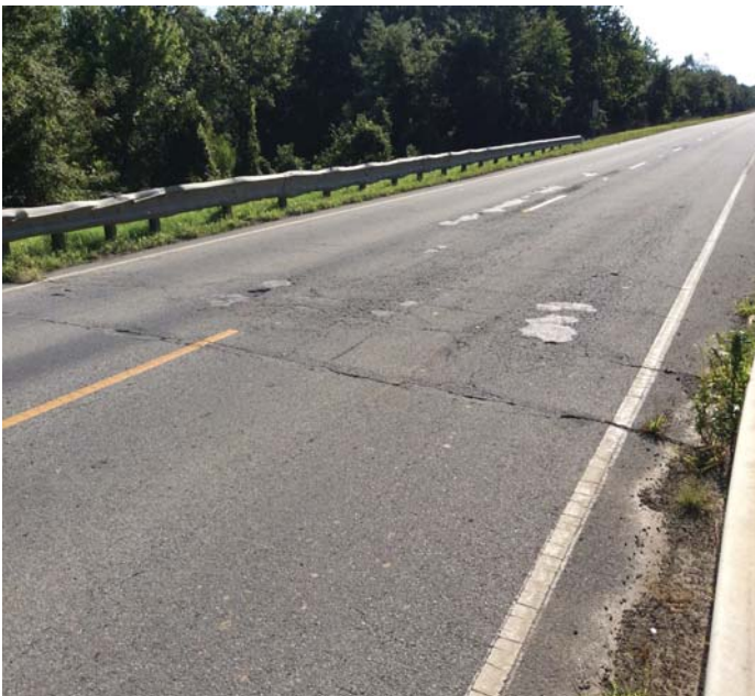
PHOTO 1 Description Visible settlement to roadway approaches at Abutments 1 & 2.
