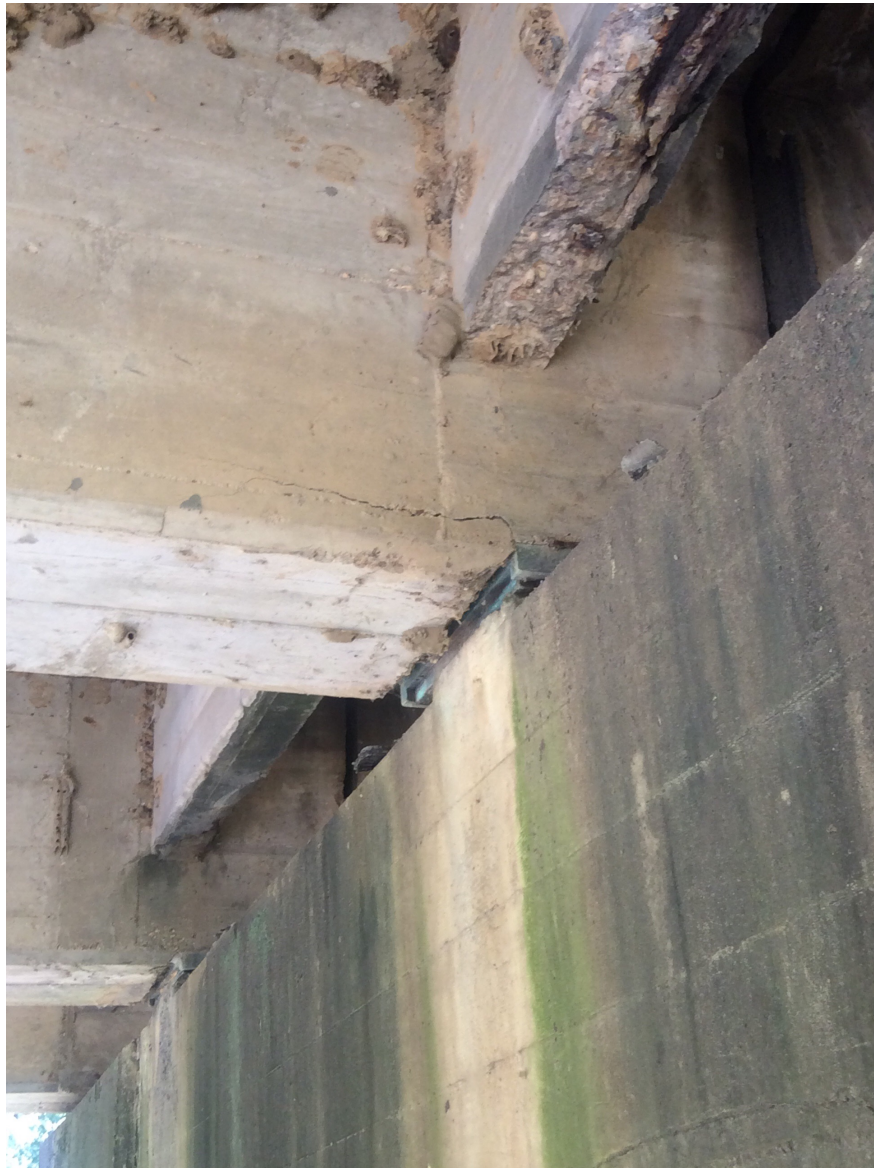
Typical cracking to bottom of girders at random areas.
