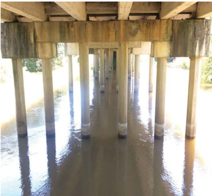
PHOTO 1 Description Minor scour to Bents 2, 3, 4, 5, and 7.
