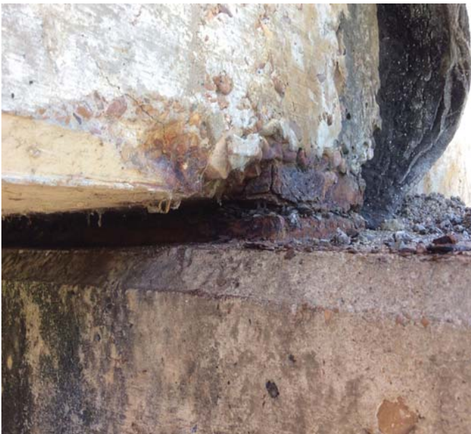
PHOTO 1 Description Span 4 Girder 6 - Typical of rust to Bearings 1 & 6 at Bents 2, 4, 6, & 8.
