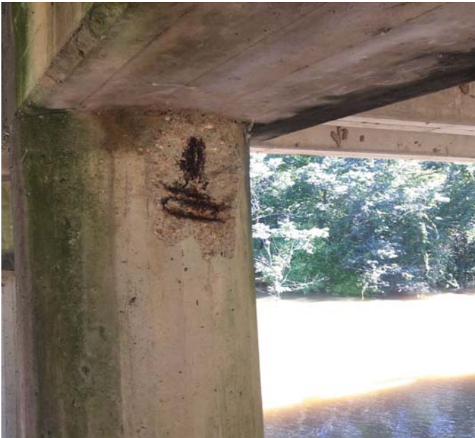
PHOTO 1 Description Bent 4 Pile 3 - Cracking, delaminating & spalls with rebar exposed at top of piles.
