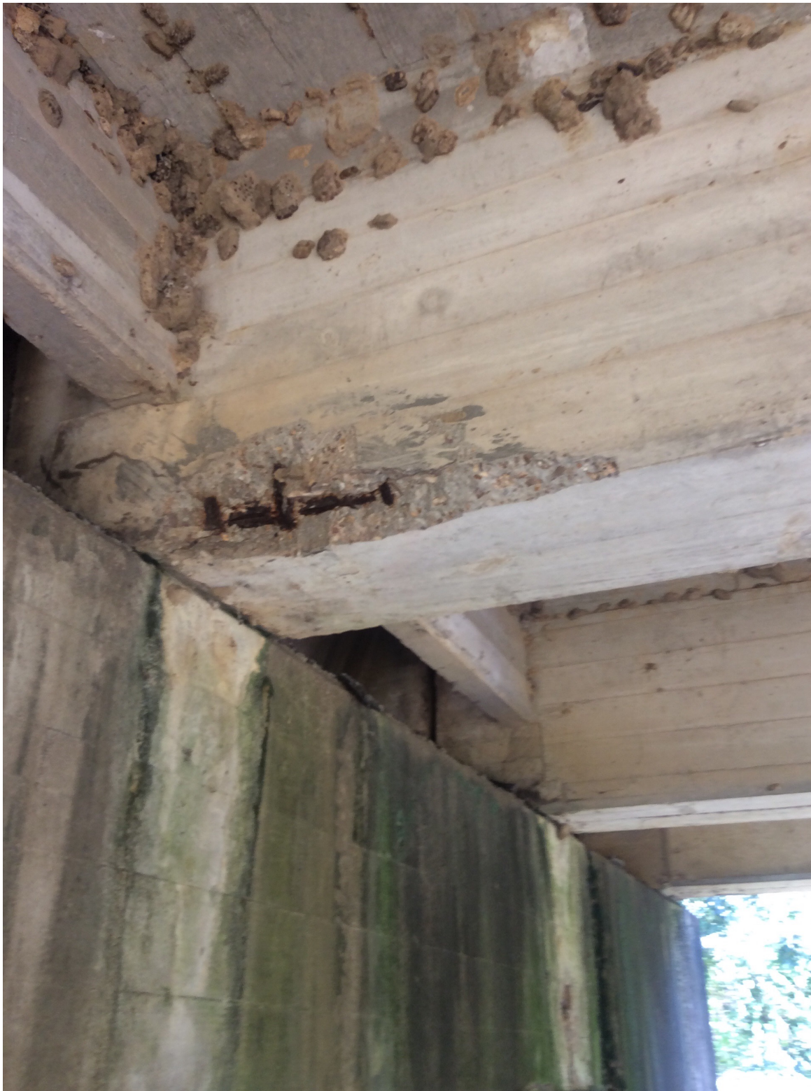
Span 6 Girder 3 - Typical cracking, delaminating, and spalling with rebar exposed to girders at all spans
