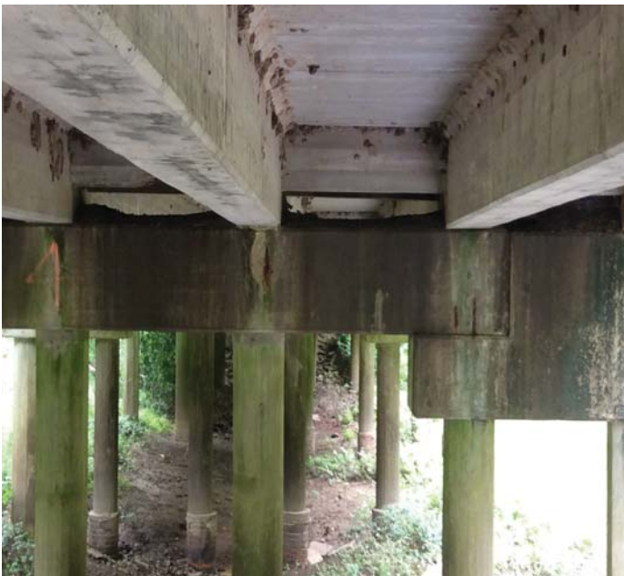
PHOTO 1 Description Bent 4. Spall with 2' rebar exposed.
