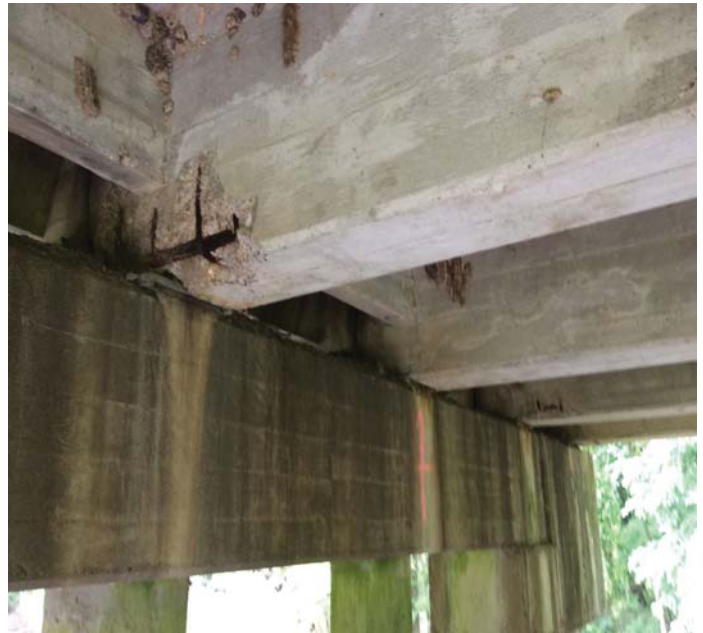
PHOTO 2 Description Span 4. Spall to Girder 3 with 3' rebar exposed & Girder 5 with 1' rebar exposed.
