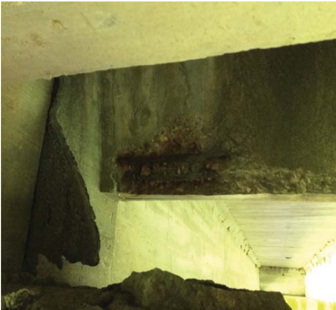
PHOTO 1 Description Typical spalls with rebar exposed to concrete haunches.
