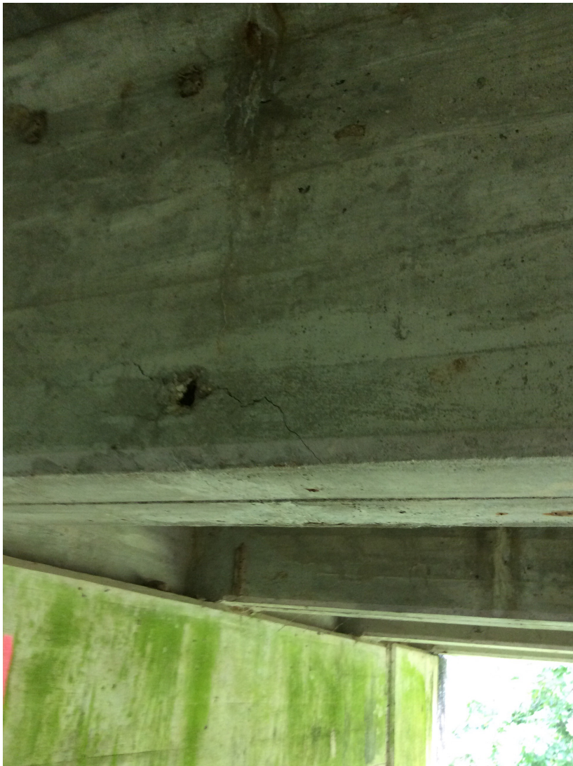
Span 2, Girder 4 - typical cracking to girder
