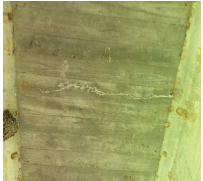
PHOTO 2 Description Typical efflorescent cracks to soffit.
