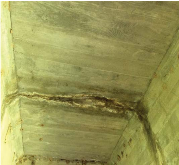
PHOTO 1 Description Typical efflorescent cracking & spall to soffit.
