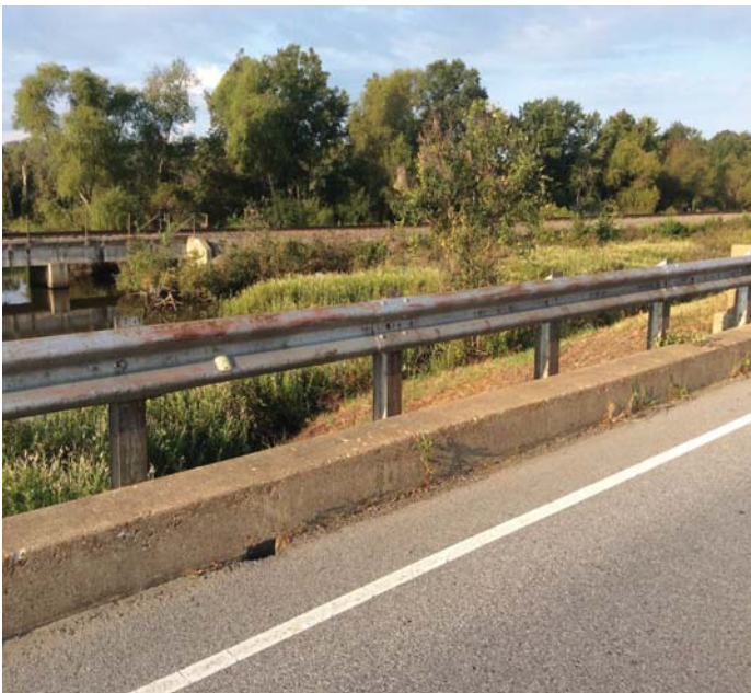
PHOTO 1 Description Paint peeling and rust forming to all post and guard rail.
