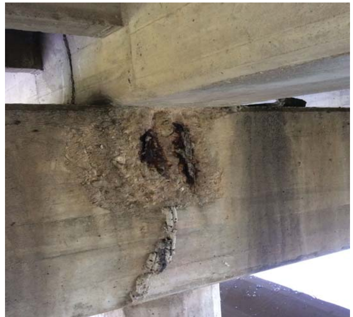
PHOTO 2 Description Spall with rebar exposed to cap @ Bent 2 back & ahead side. (Ahead side)
