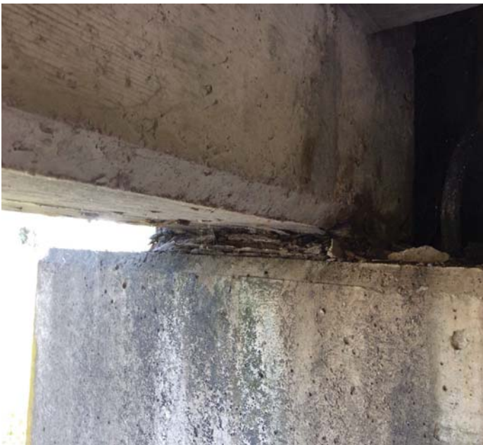
PHOTO 1 Description Bearings 1 & 6 @ Bent 2 have rust and section loss.
