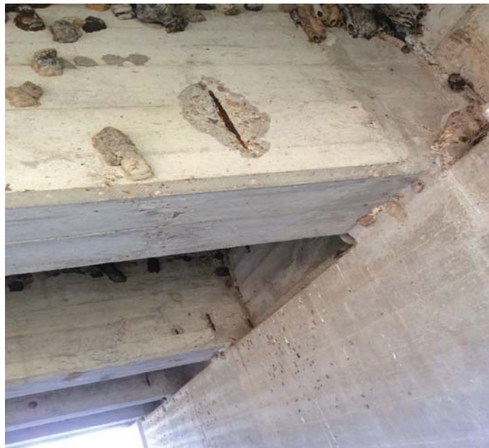
PHOTO 1 Description Girders at Spans 1 thru 3 have random spalls with rebar exposed at several locations. (Span 1)
