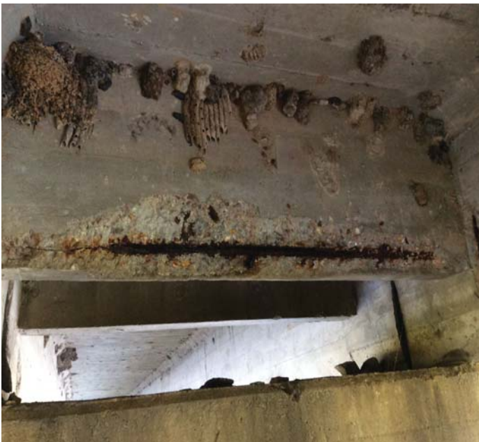
PHOTO 1 Description Spall to concrete Diaphragm's between Girders 2 & 3 @ beginning of Span 3.
