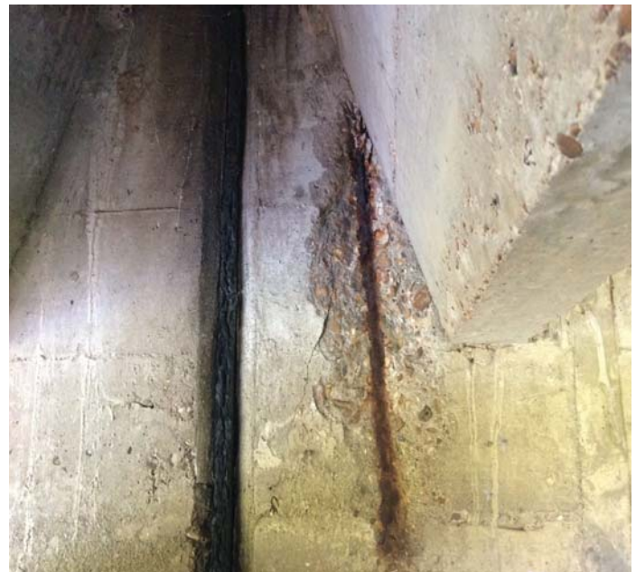
PHOTO 2 Description Girders at Spans 1 thru 3 have spalls with rebar exposed at several locations. (Span 3 girder 2 @ beginning of span)
