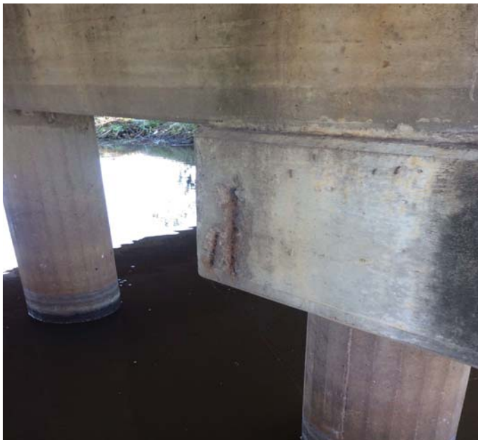
PHOTO 1 Description Spall with rebar exposed to cap @ Bent 2. (Back side)
