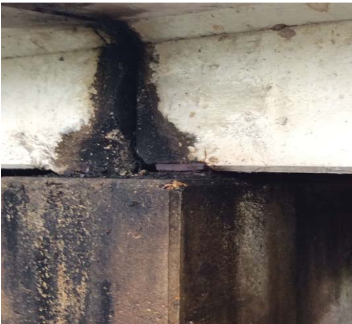
PHOTO 1 Description Typical rust to Bearings.
