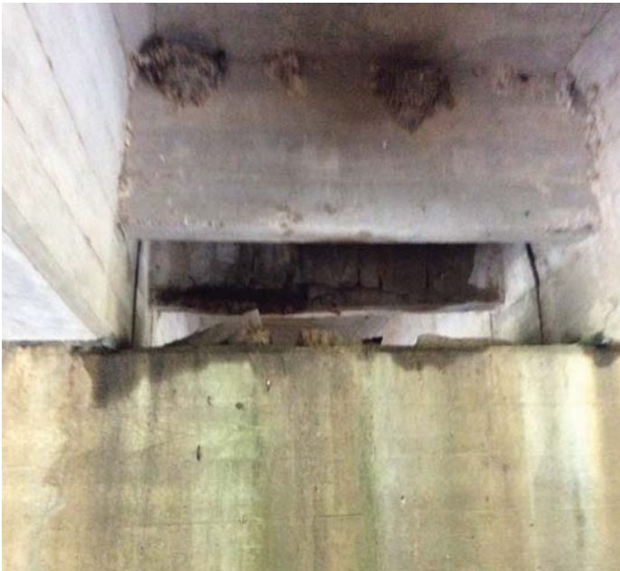
PHOTO 1 Description Typical spalls with rebar exposed to Concrete Diaphragm.
