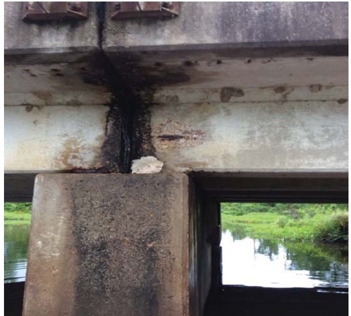
PHOTO 2 Description Span 3 Spall to Girder 6 with rebar exposed at Beginning of Span.
