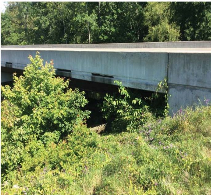
PHOTO 1 Description Small trees and vegetation are growing beside and under bridge at abutments.
