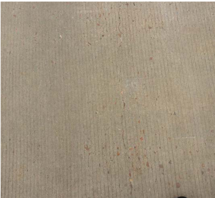
PHOTO 1 Description Typical transverse shoulder crack
