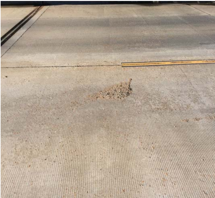
PHOTO 1 Description Abutment #2 approach slab right lane near chanter line has 1' spall no rebar exposed.
