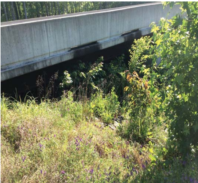
PHOTO 1 Description Abutments have small trees and vegetation growing beside and under bridge.
